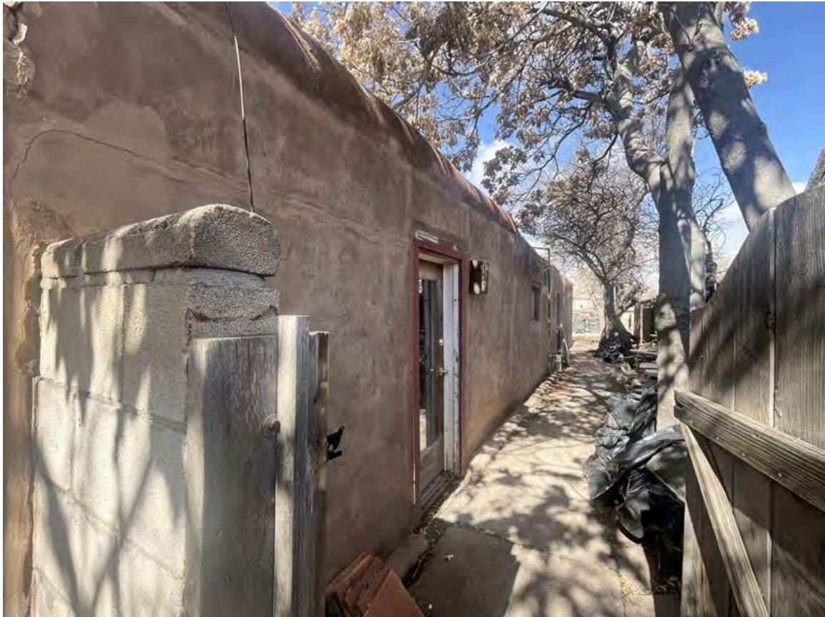
Photo 7: East elevation, south end. Camera facing north.
