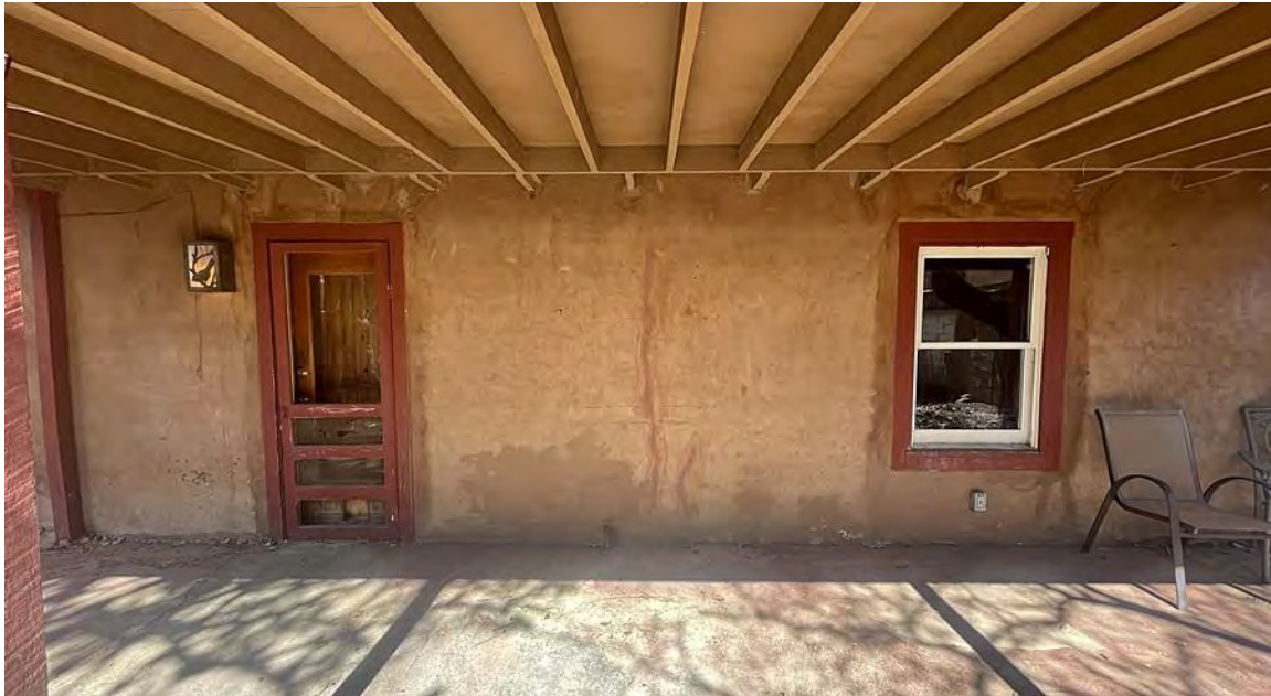
Photo 6: South elevation. Façade representing pre-1954 construction. Camera facing north.
