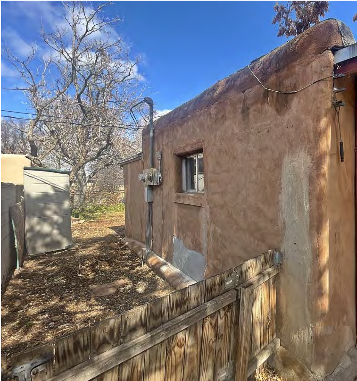
Photo 5: West elevation. South end representing pre-1954 construction. Camera facing northeast.
