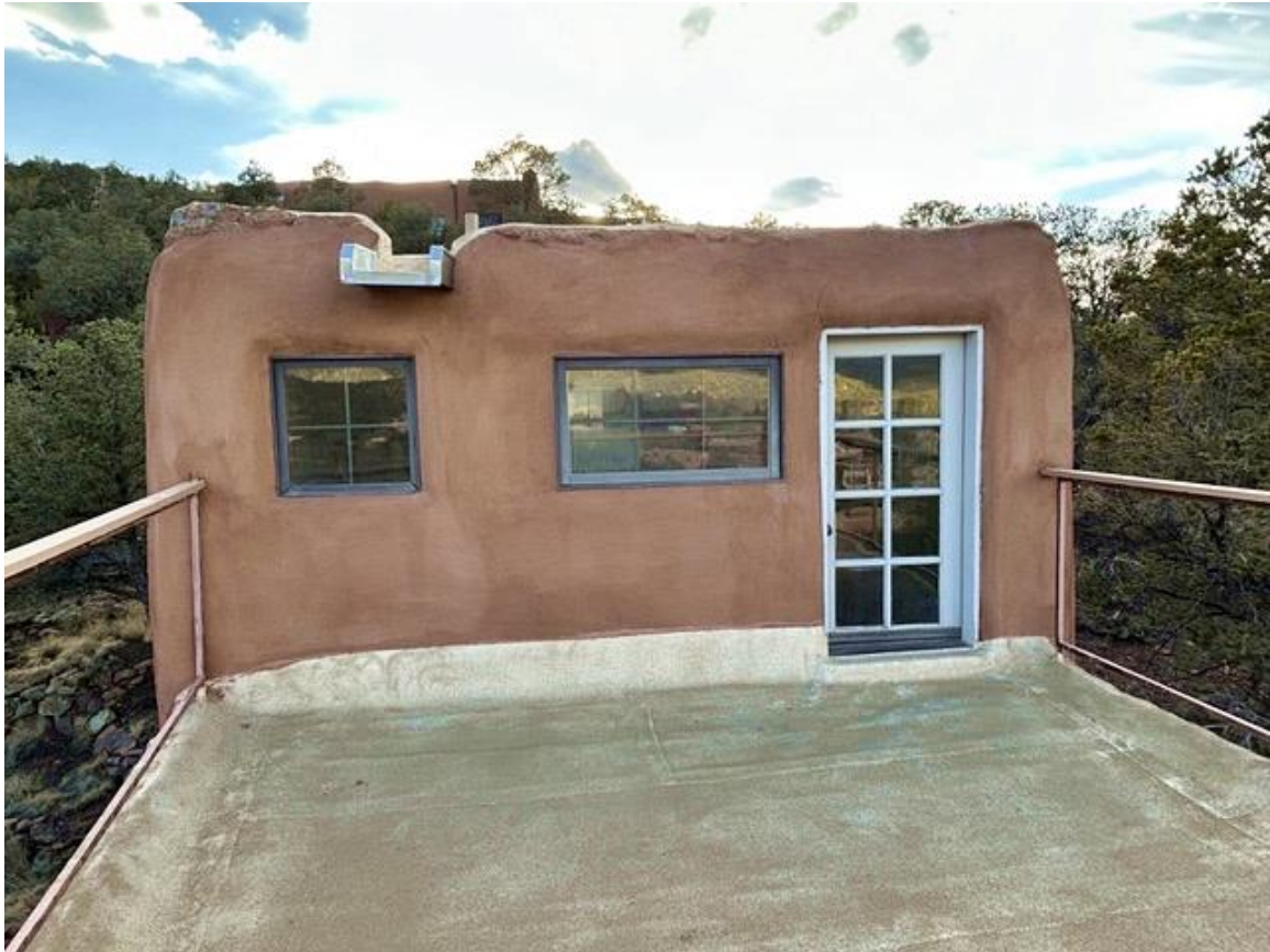
Photo 3: East elevation. Camera facing west.
