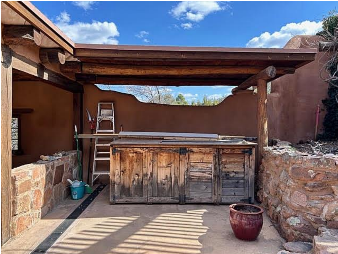
Photo 12: Patio portal area. Camera facing south.
