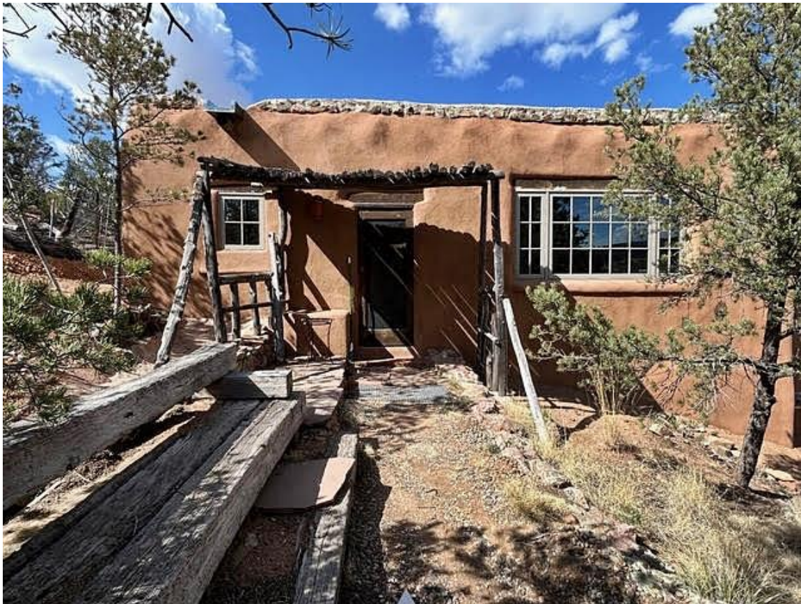
Photo 6: South elevation. Camera facing north.
