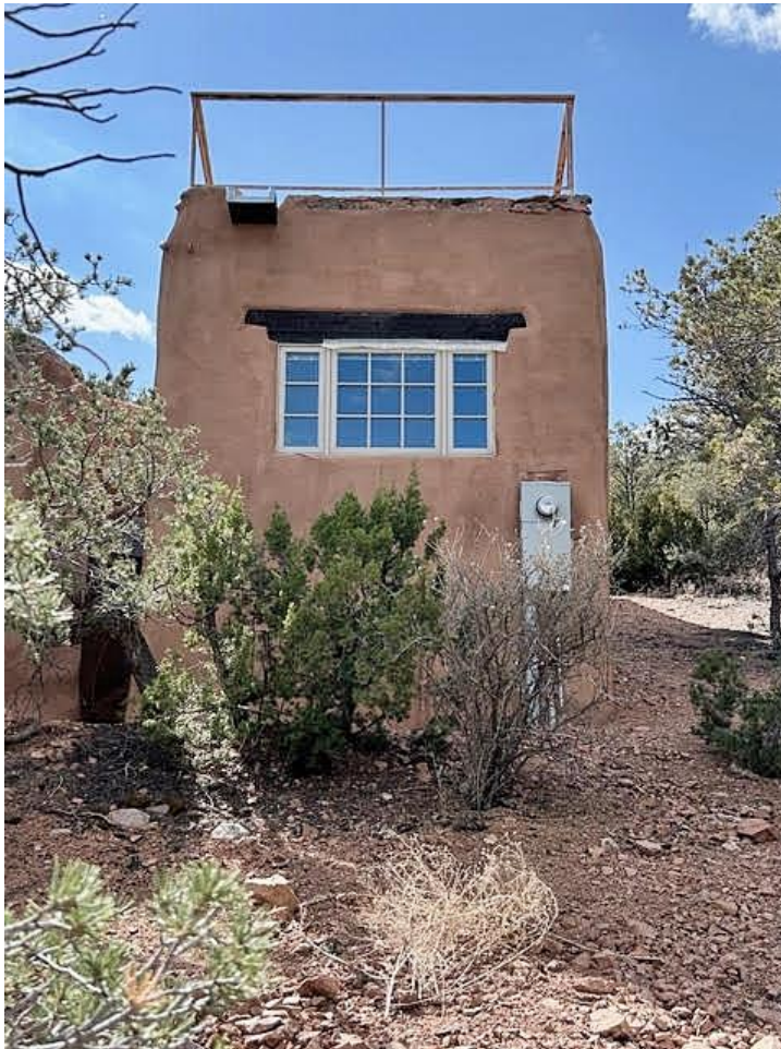
Photo 2: East elevation. Camera facing up.
