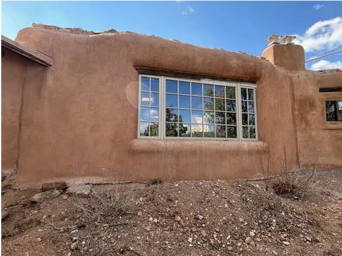
Photo 9: East elevation. Camera facing northwest.
