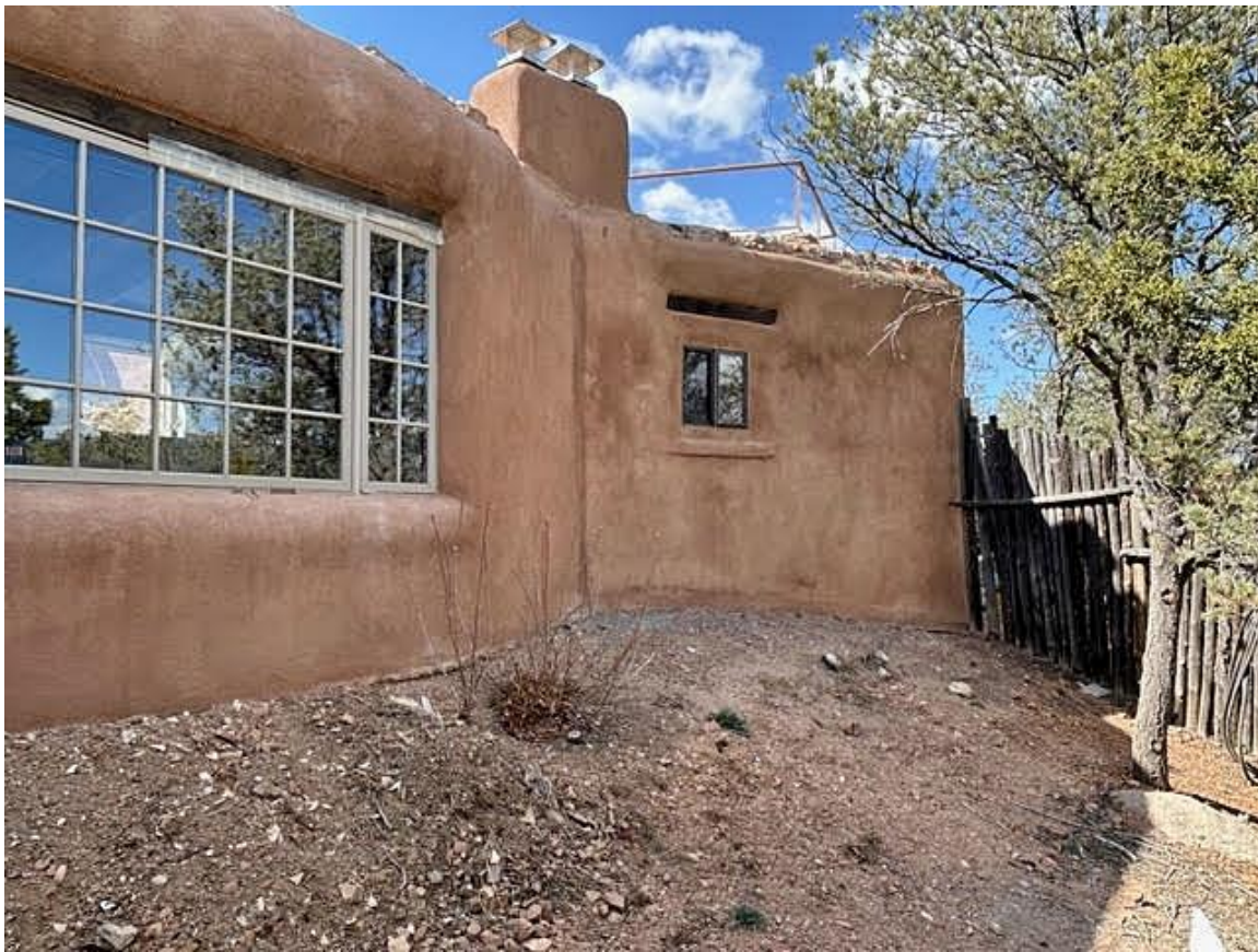
Photo 7: East elevation. Camera facing northwest.
