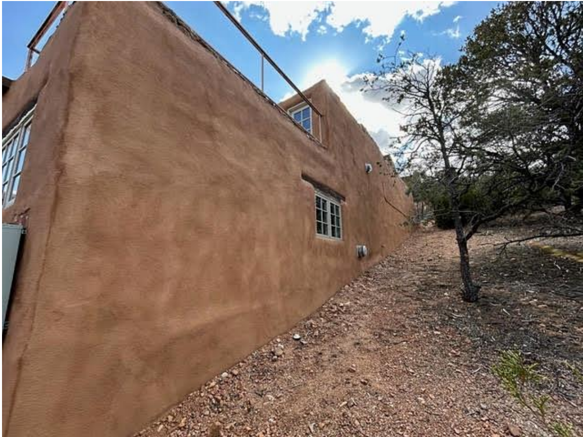
Photo 4: North elevation. Camera facing up.
