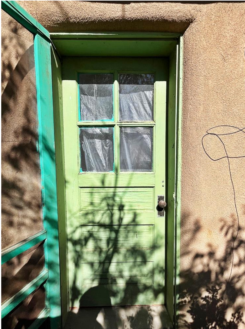
Photo 40: Rear entry door. Camera facing east.
