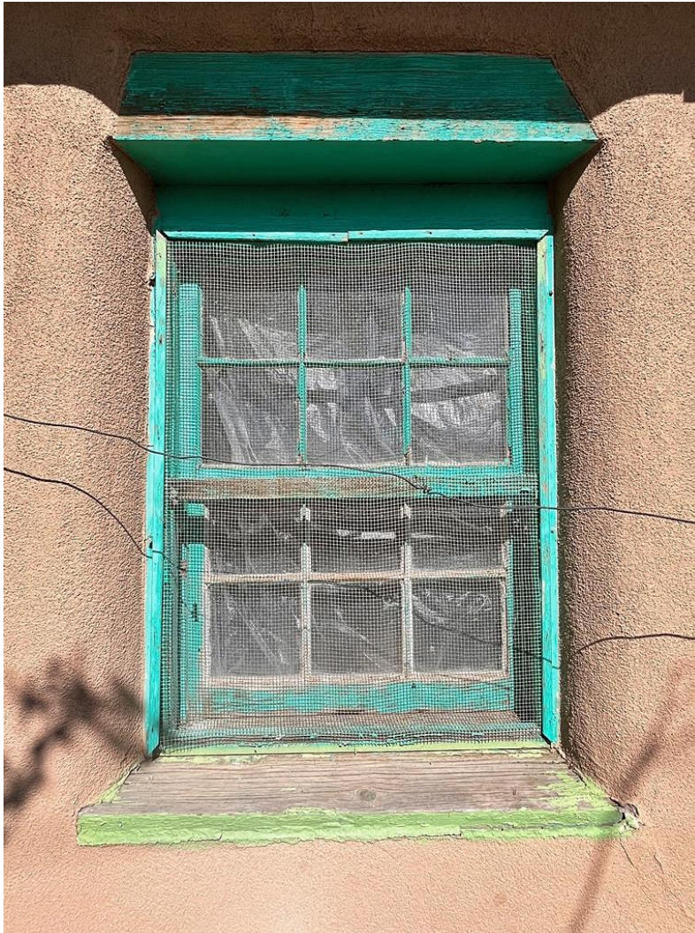
Photo 42: Window south of door. Camera facing east.
