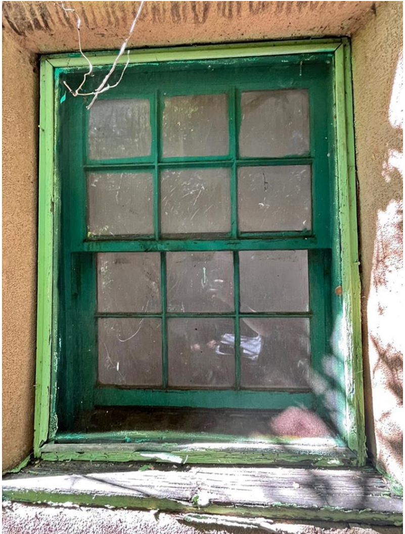
Photo 45: East end window. Camera facing north.
