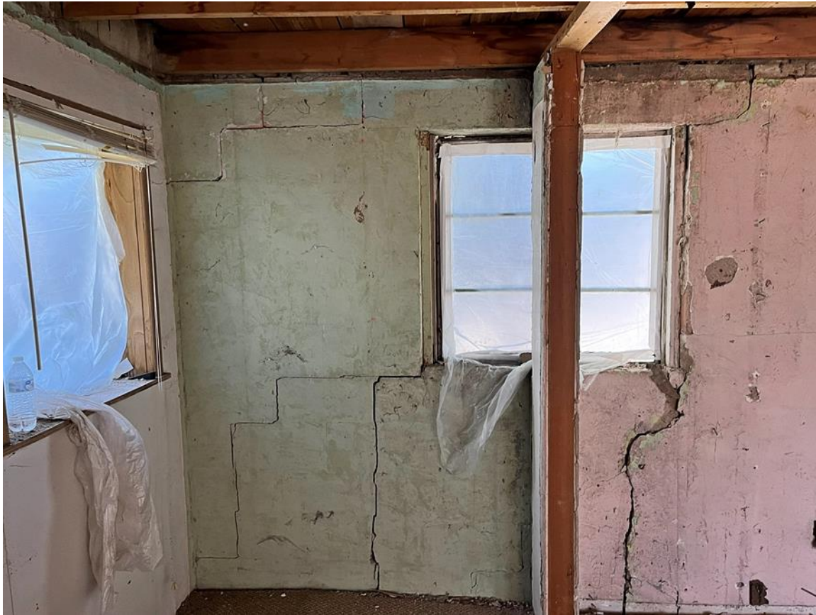
Photo 9: Windows at interior of CMU addition. Camera facing southeast.
