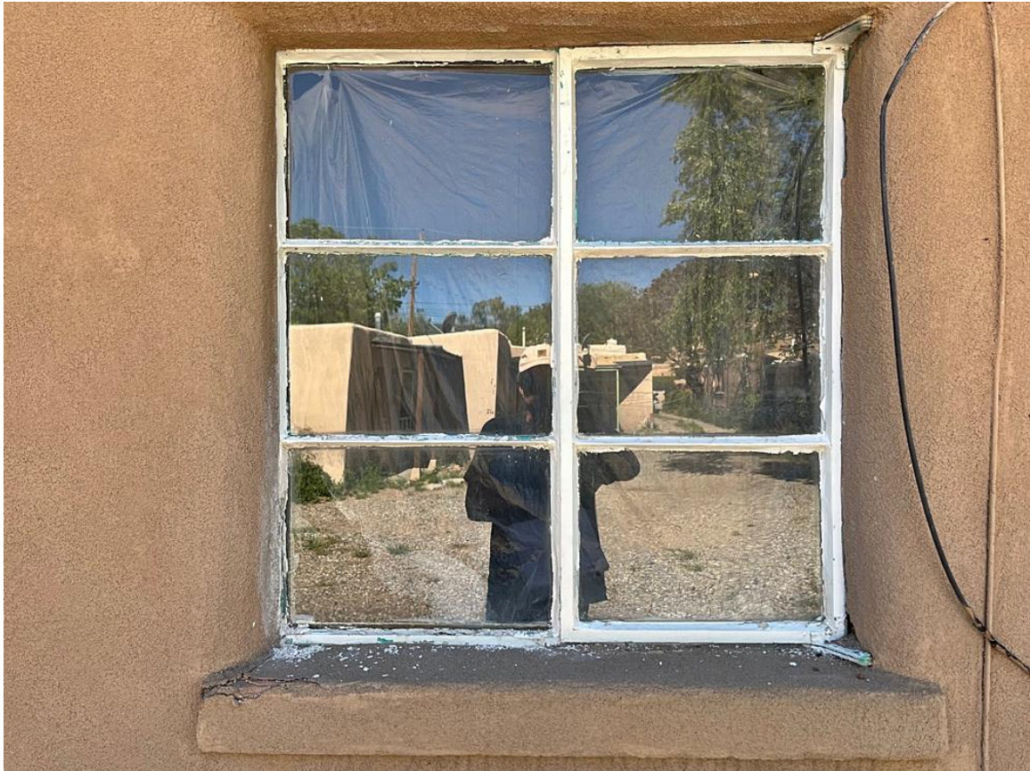
Photo 34: Camera north of entry. Camera facing west.
