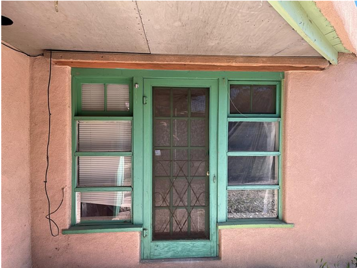
Photo 15: Entry to CMU addition. Camera facing south.
