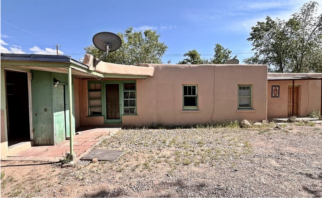
North elevation, west end, facing south.
