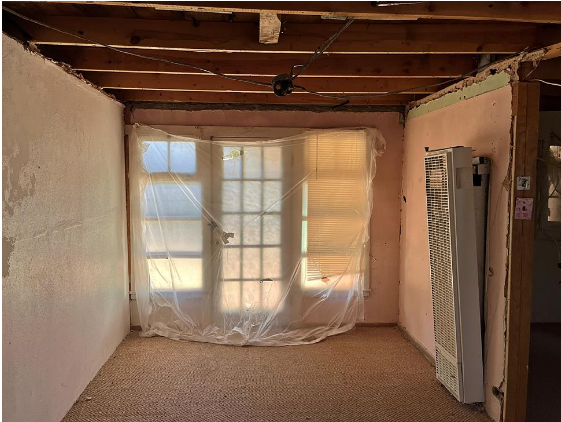
Photo 16: Interior of entry to CMU addition. Camera facing north.
