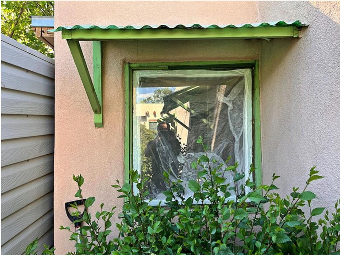
Photo 8: Window at CMU addition. Camera facing west.
