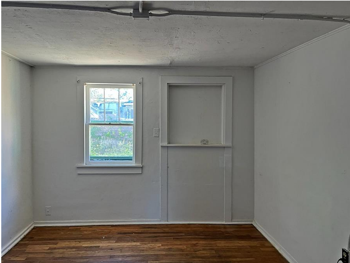
Photo 20: Interior of apartment showing window and deleted door. Camera facing north.
