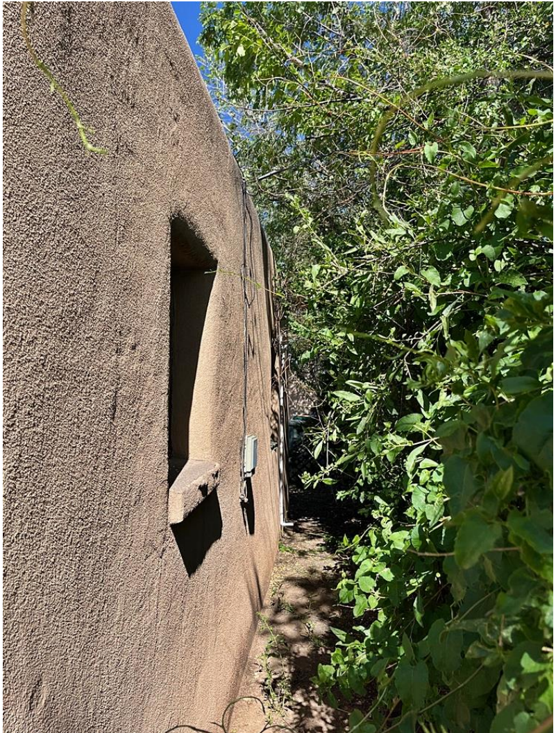
Photo 43: South elevation. Camera facing east.
