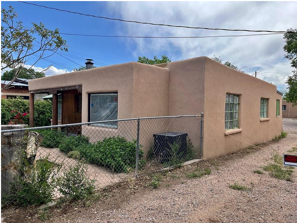
Photo 2: East (front) and north elevations of original home. Portal and entry added later. Camera facing southwest.
