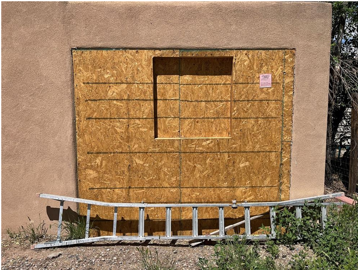
Photo 35: Infilled garage door. Camera facing west.
