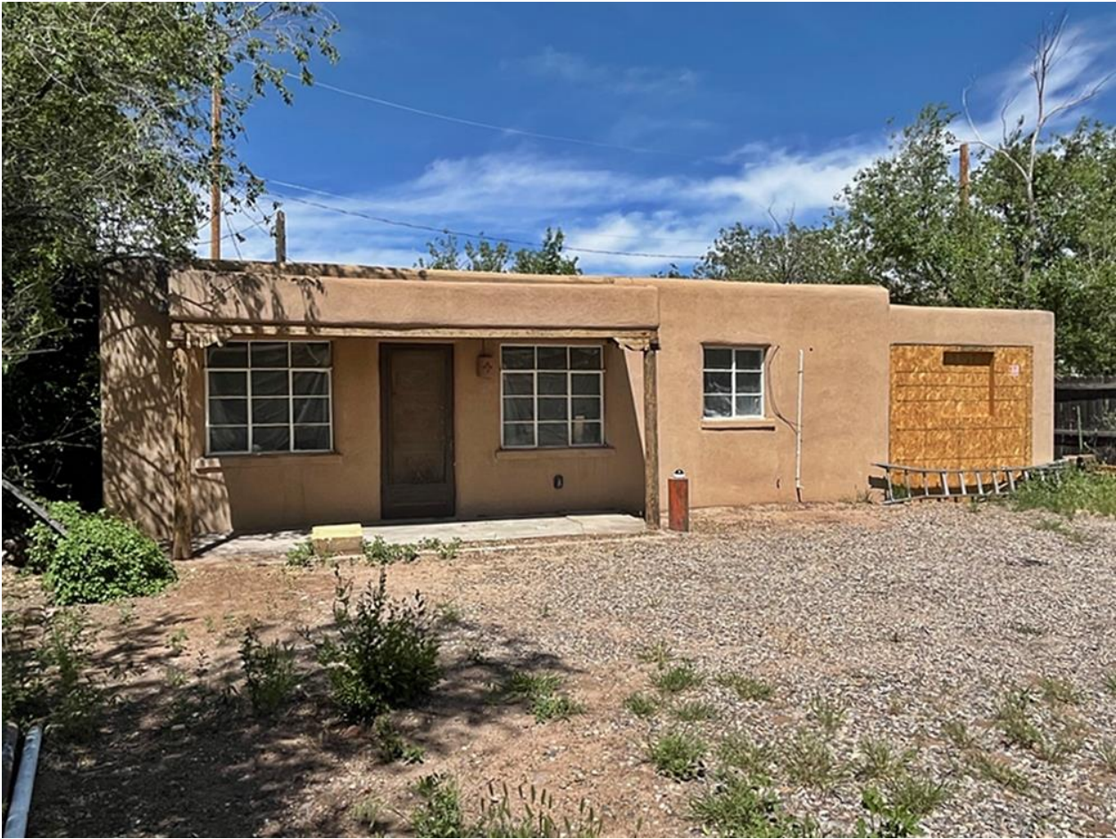
East (front) elevation, facing northwest.
