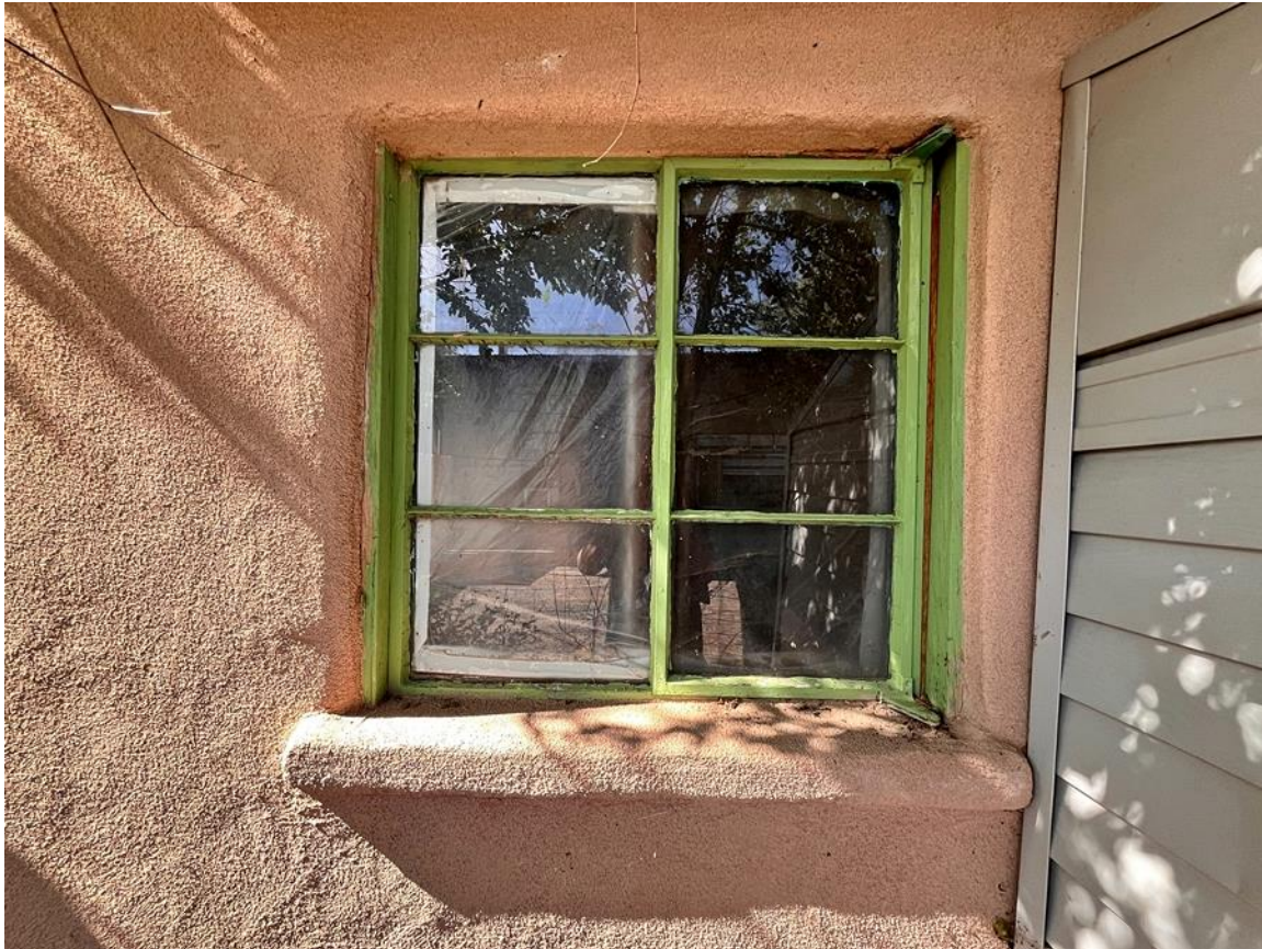
Photo 25: Window at CMU addition. Camera facing north.
