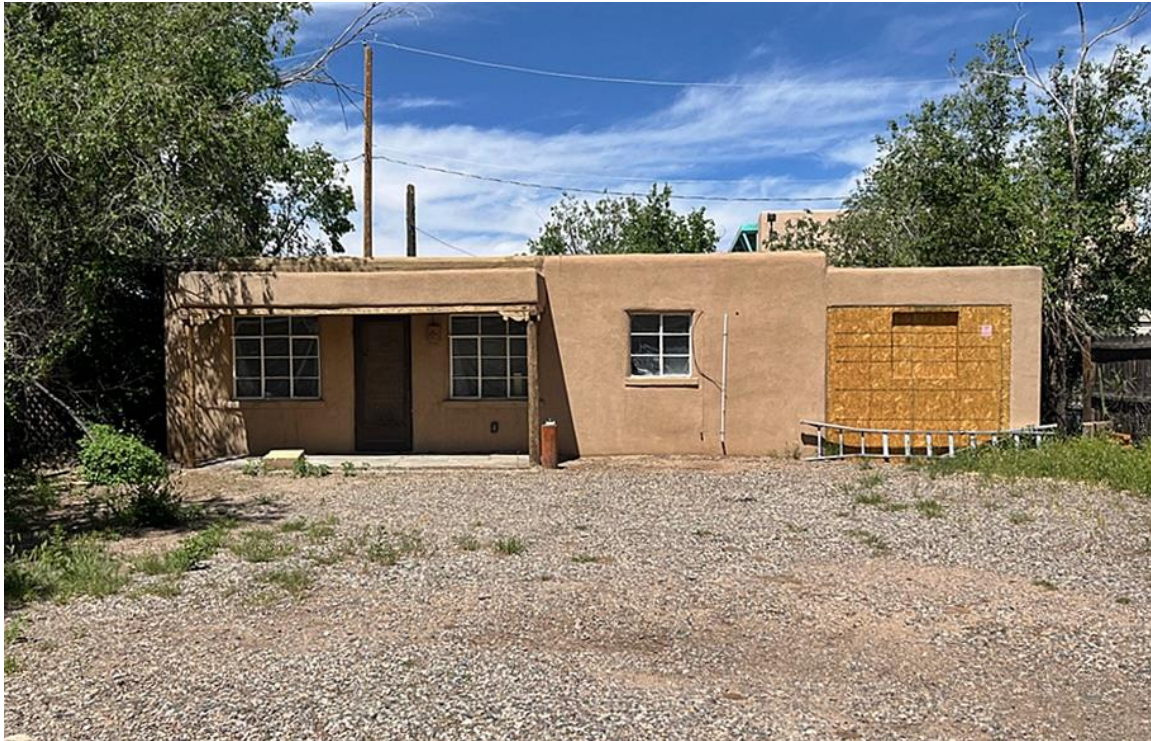
Photo 29: East façade and context. Camera facing west.
