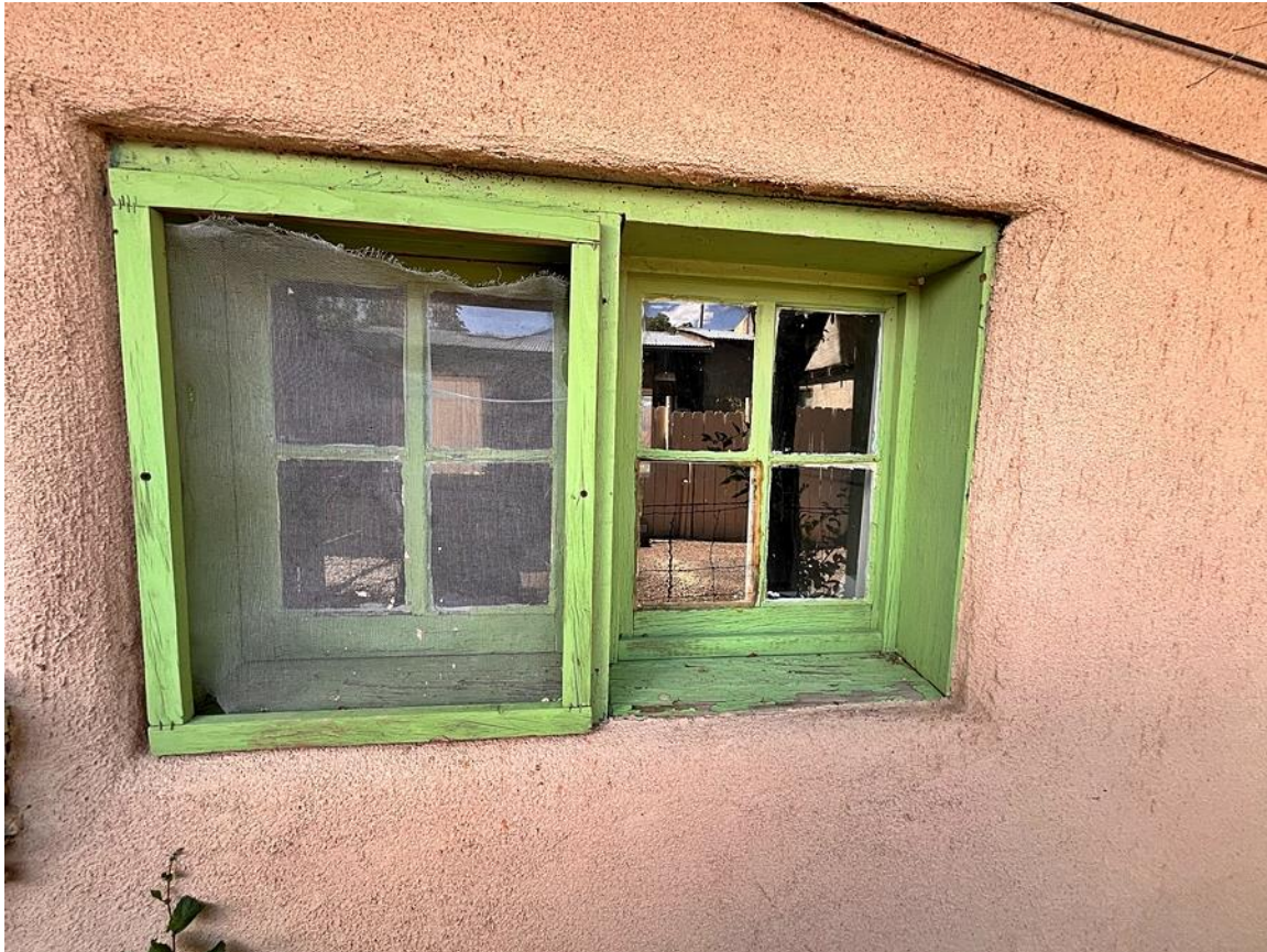
Photo 27: Window at apartment kitchen. Camera facing north.
