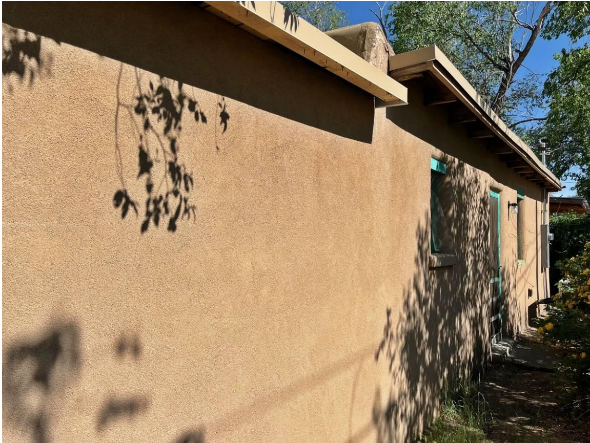
Photo 38: West elevation. Former garage on the left. Camera facing southeast.
