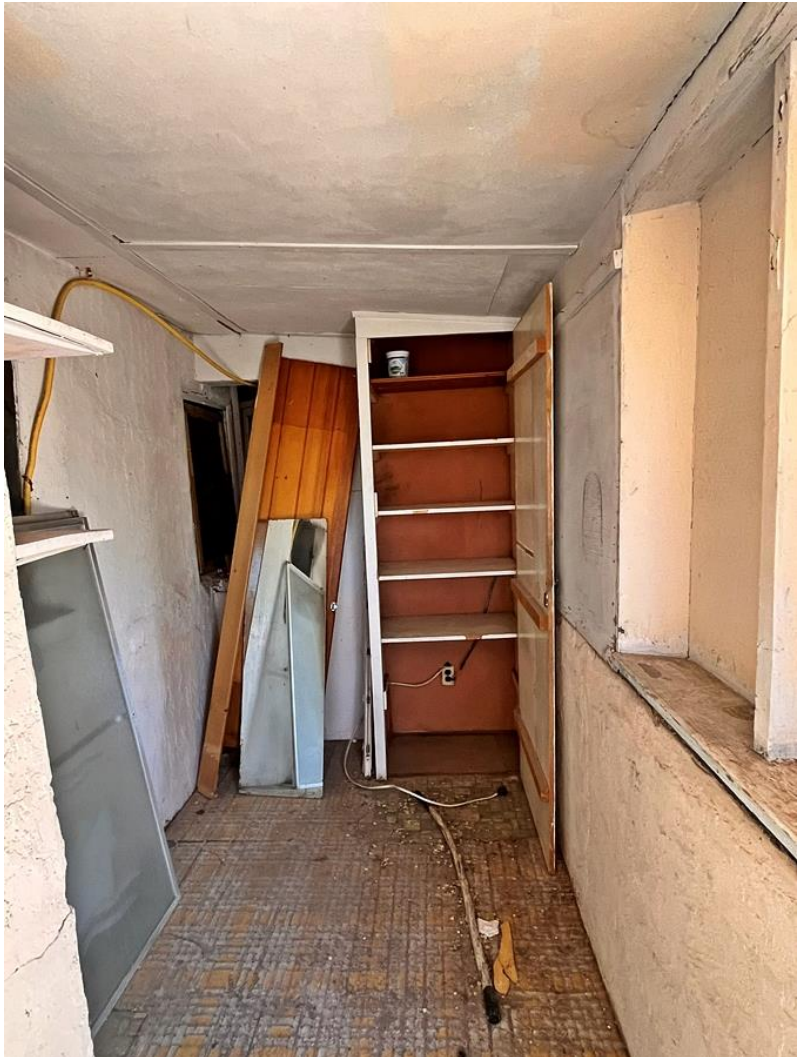
Photo 14: Interior of enclosed porch. Camera facing south.
