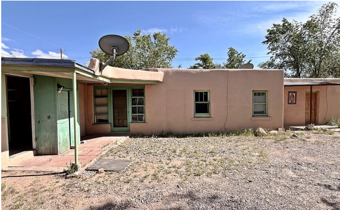
Photo 17: Apartment addition at center and right. Camera facing south.
