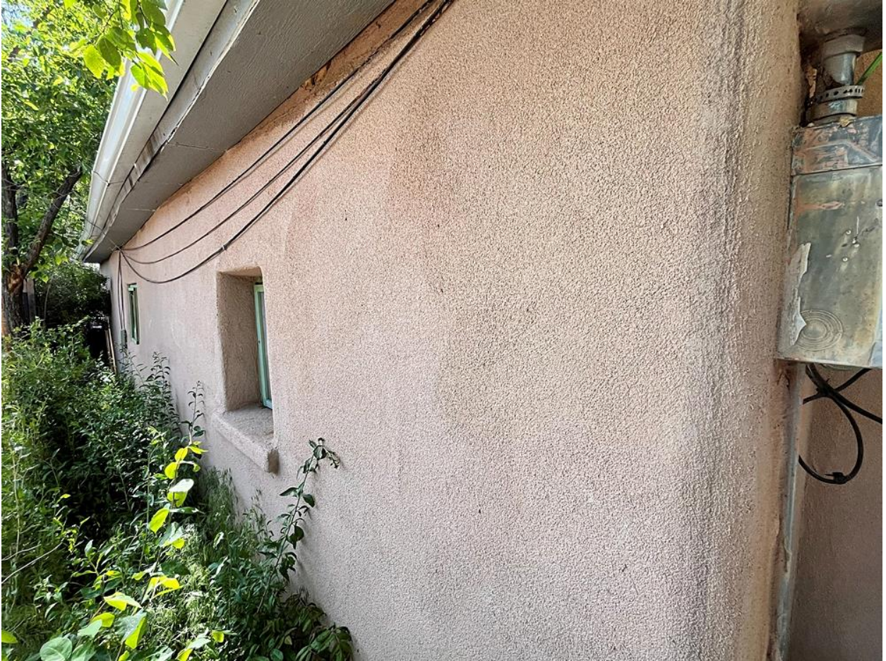
South elevation west end, facing west.
