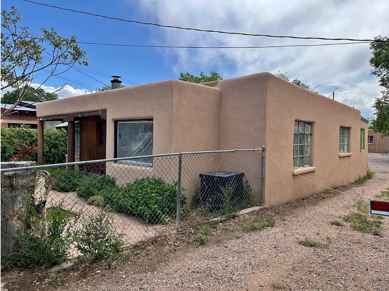
North elevation, east end, facing southwest.
