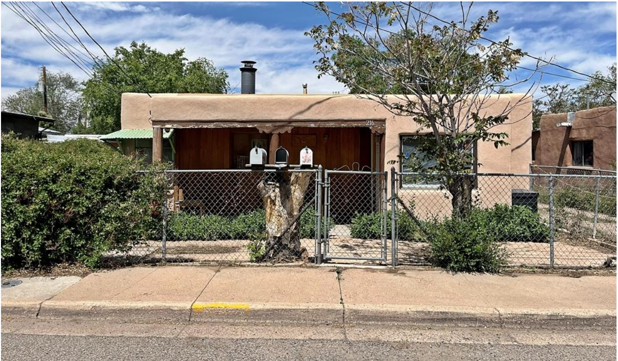
East (front) elevation, facing west.
