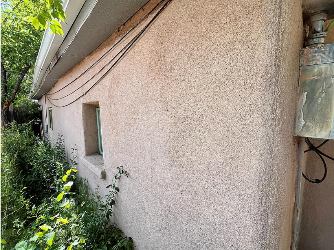
Photo 26: South elevation of apartment addition. Camera facing northwest.
