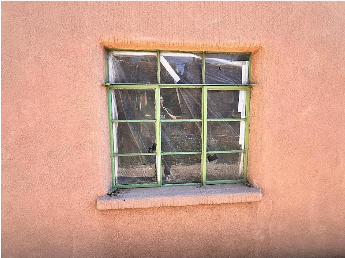
Photo 11: Window at north elevation of historic core. Camera facing south.
