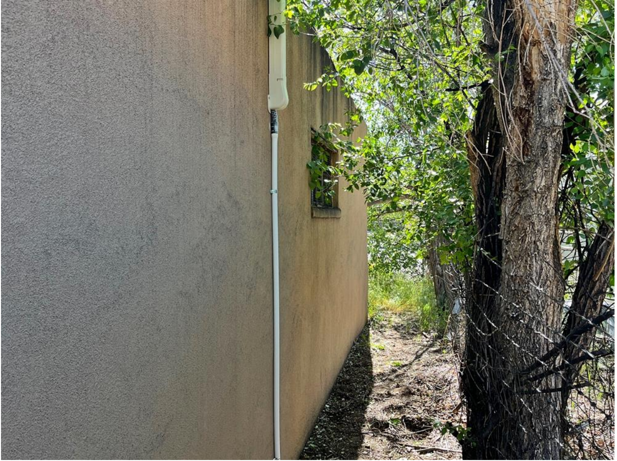
North elevation, facing west.
