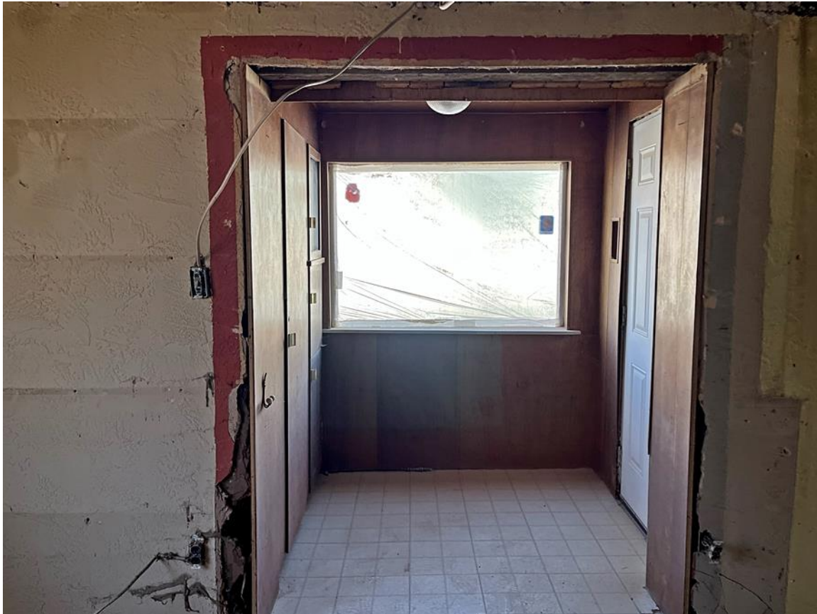
Photo 6: Entry vestibule. Camera facing east.
