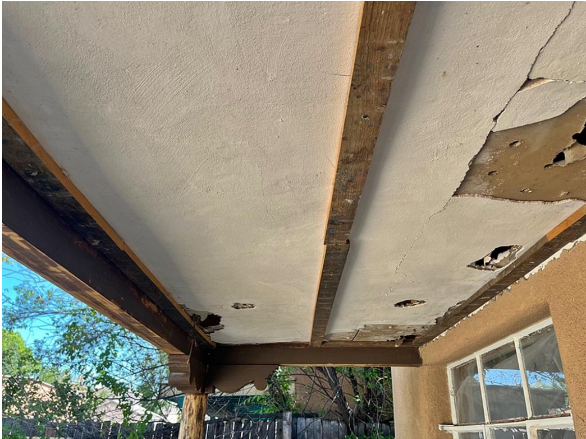
Photo 31: Porch ceiling. Camera facing up.
