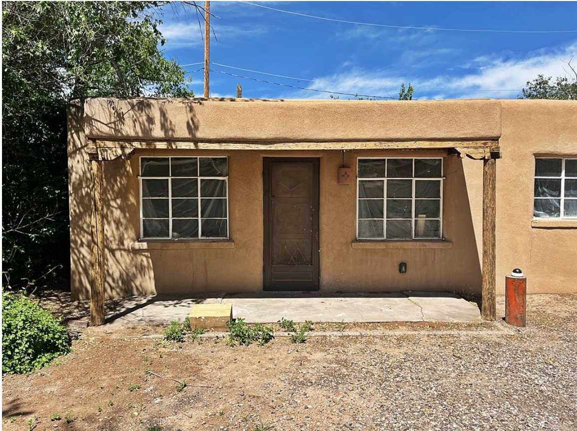
Photo 30: Porch. Camera facing west.
