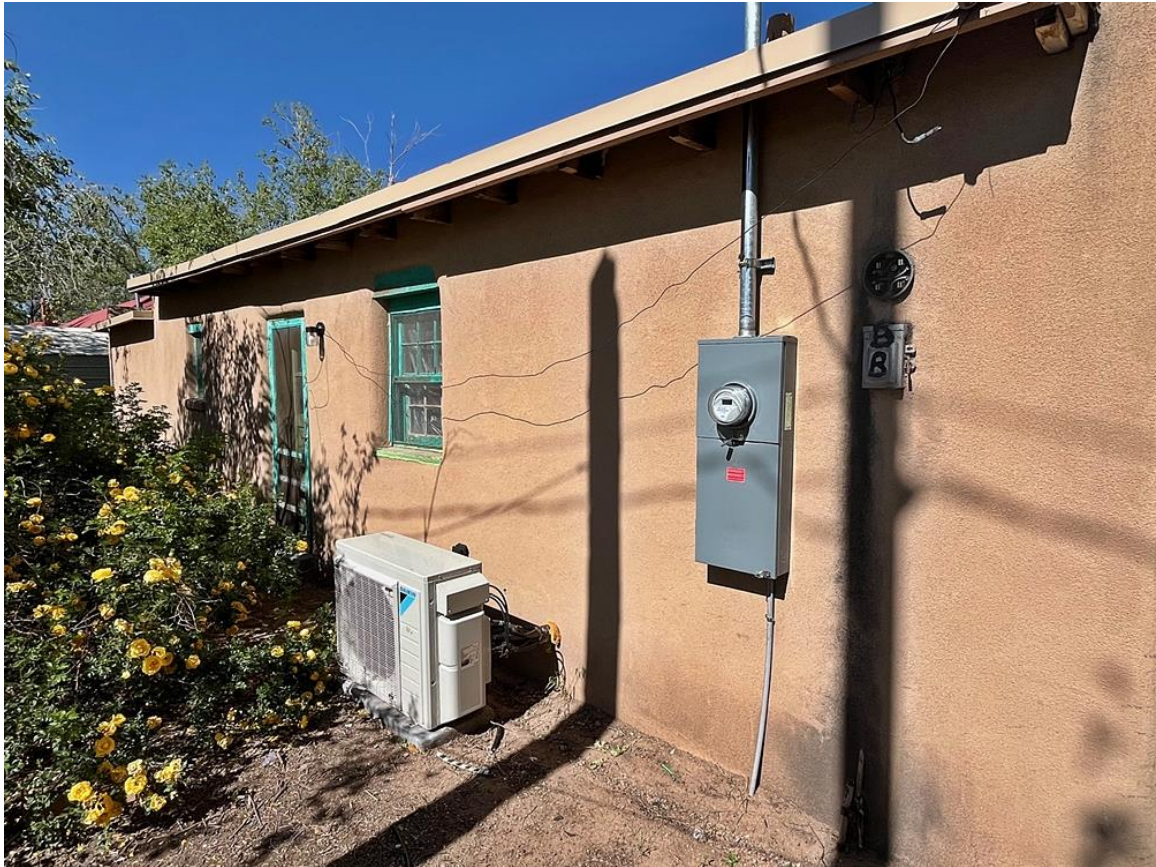
Photo 39: West elevation. Camera facing northeast.
