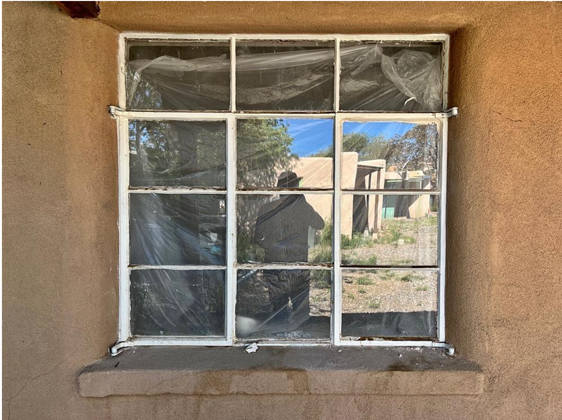
Photo 33: Window south of entry. Camera facing west.
