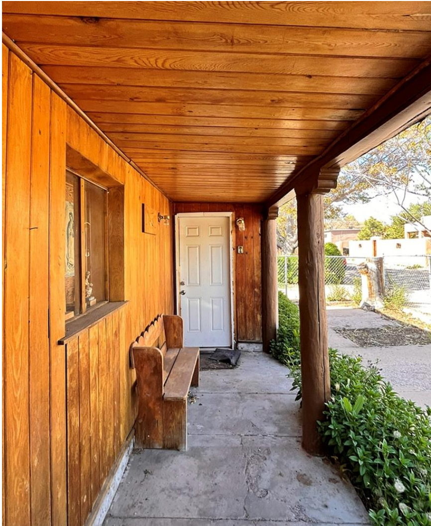
Photo 3: Portal and entry vestibule. Camera facing north.
