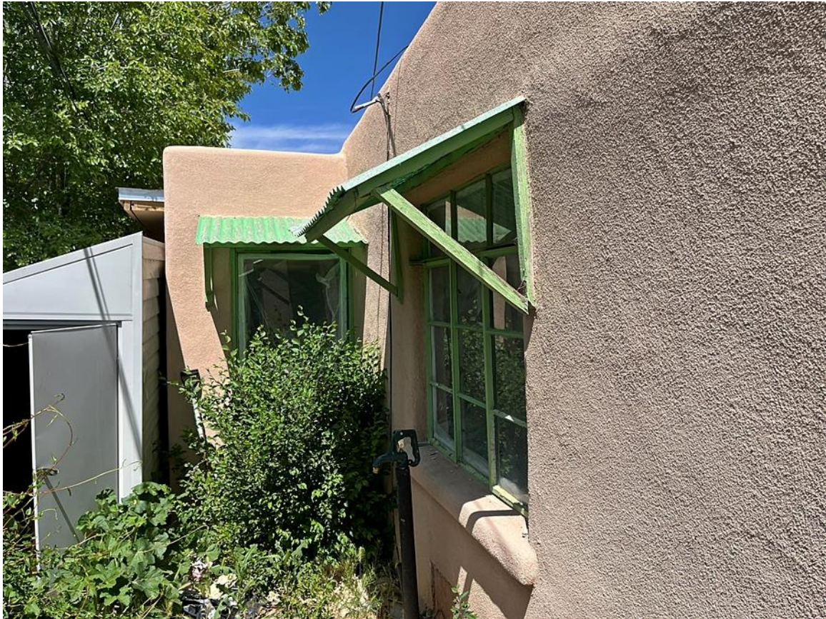
Photo 23: South elevation, original historic core at right. Camera facing west.
