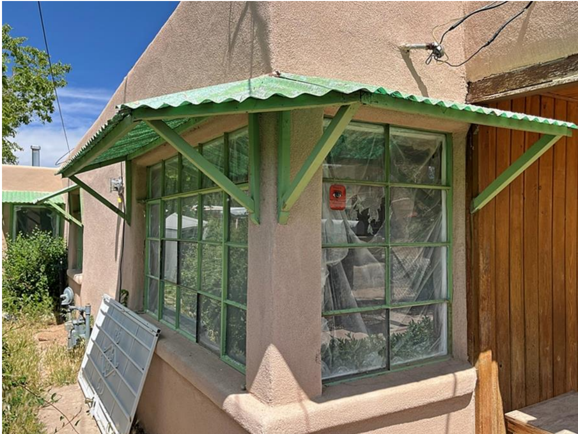
Photo 7: Windows at southeast corner. Camera facing northwest.
