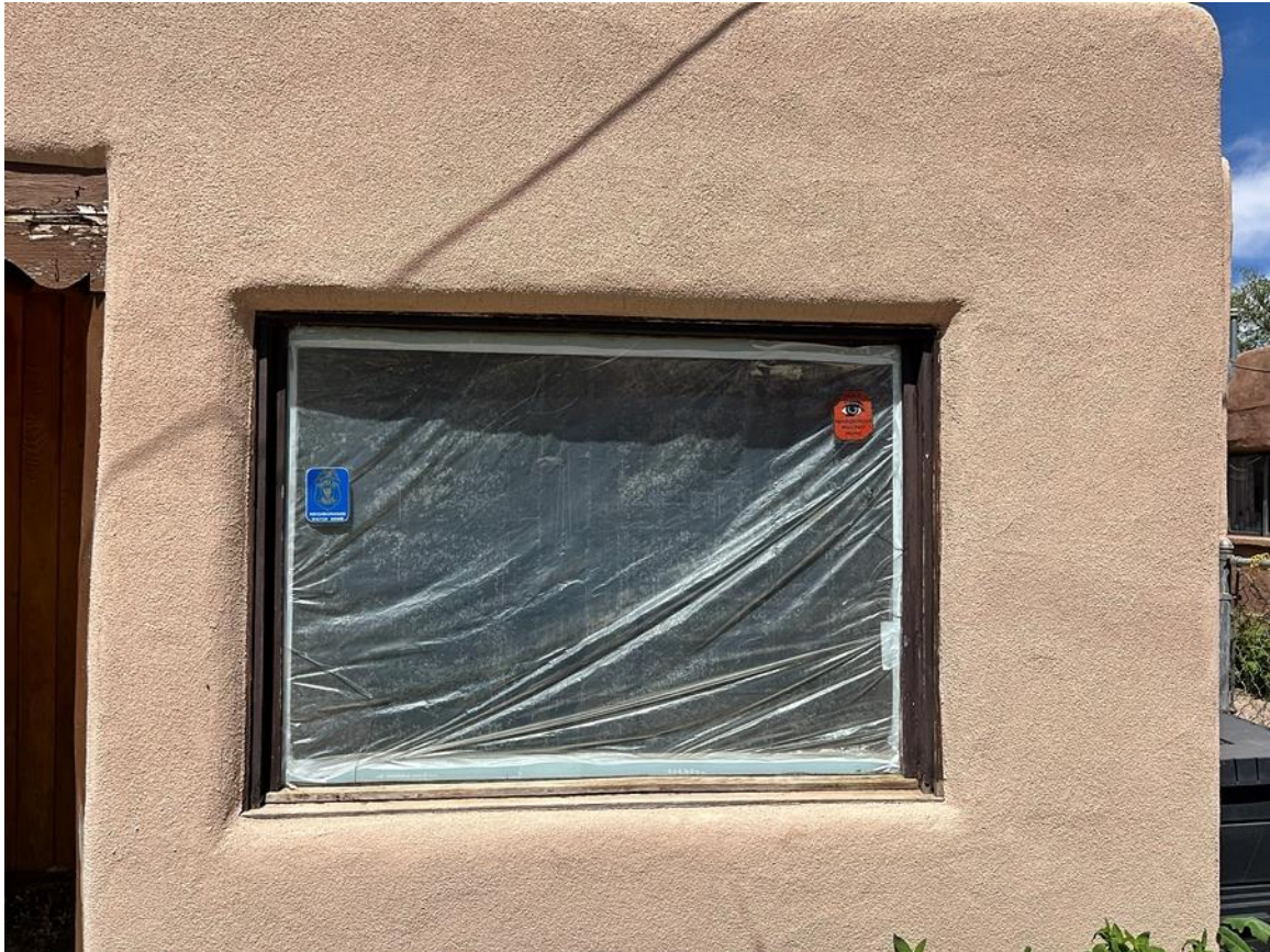
Photo 5: Window at entry vestibule. Camera facing west.
