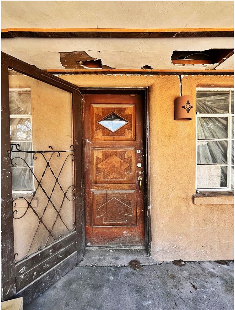
Photo 32: Entry door. Camera facing west.
