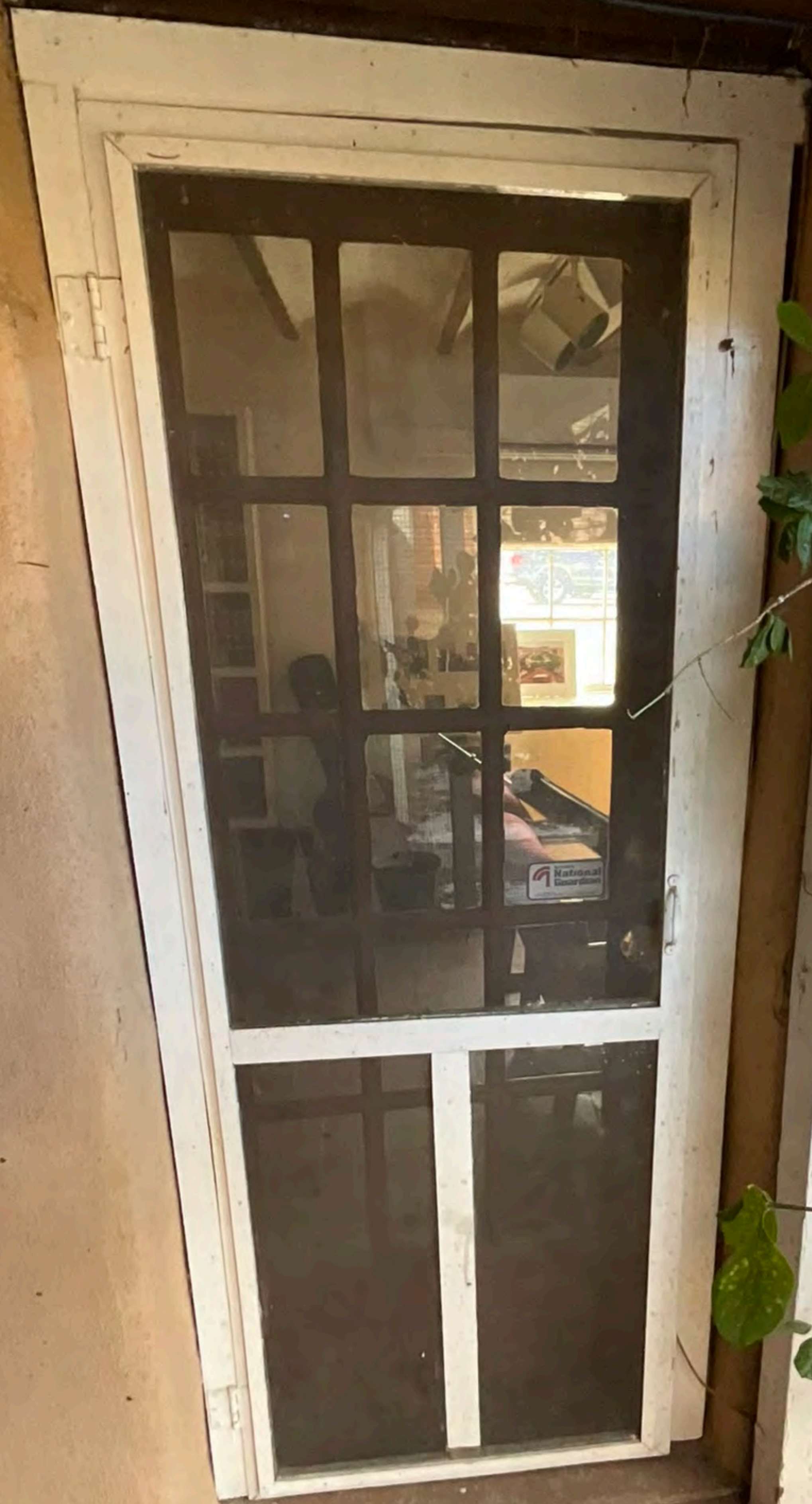
Courtyard North Elevation Door #9
