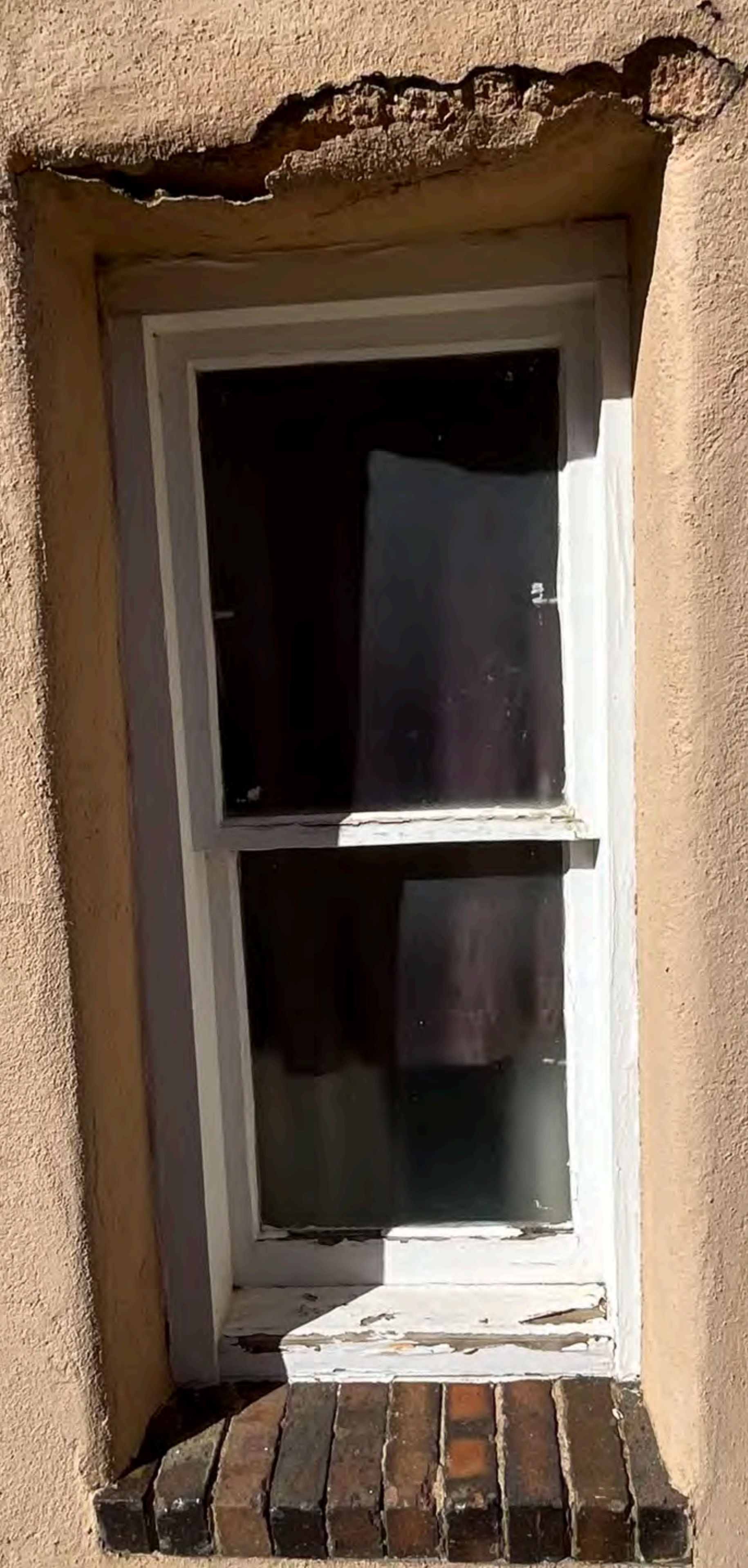
East Elevation Window F
