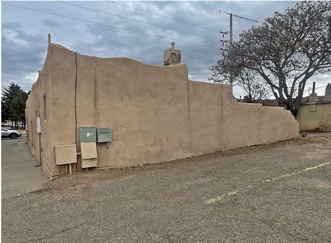
Photo 32: South elevation. Camera facing northeast.
