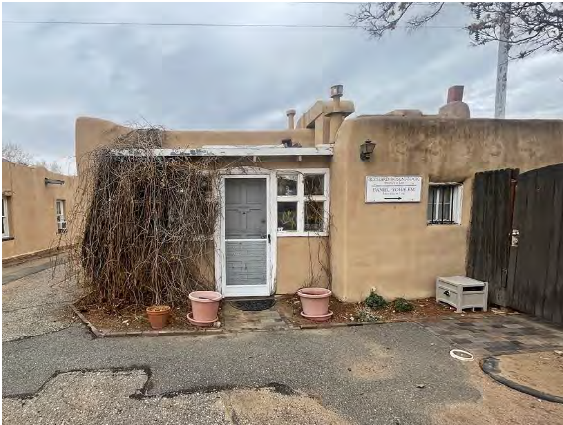
Photo 13: South elevation, west end. Closeup of enclosed porch. Camera facing north.
