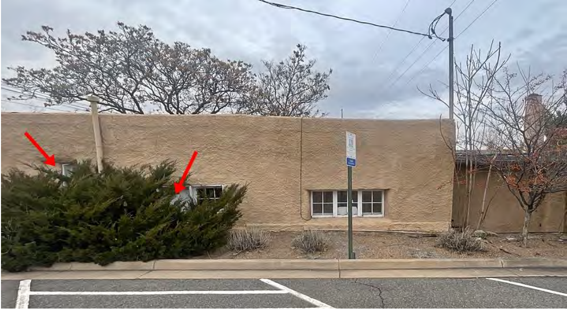
Photo 19: East elevation. Location of obscured windows. Camera facing west.
