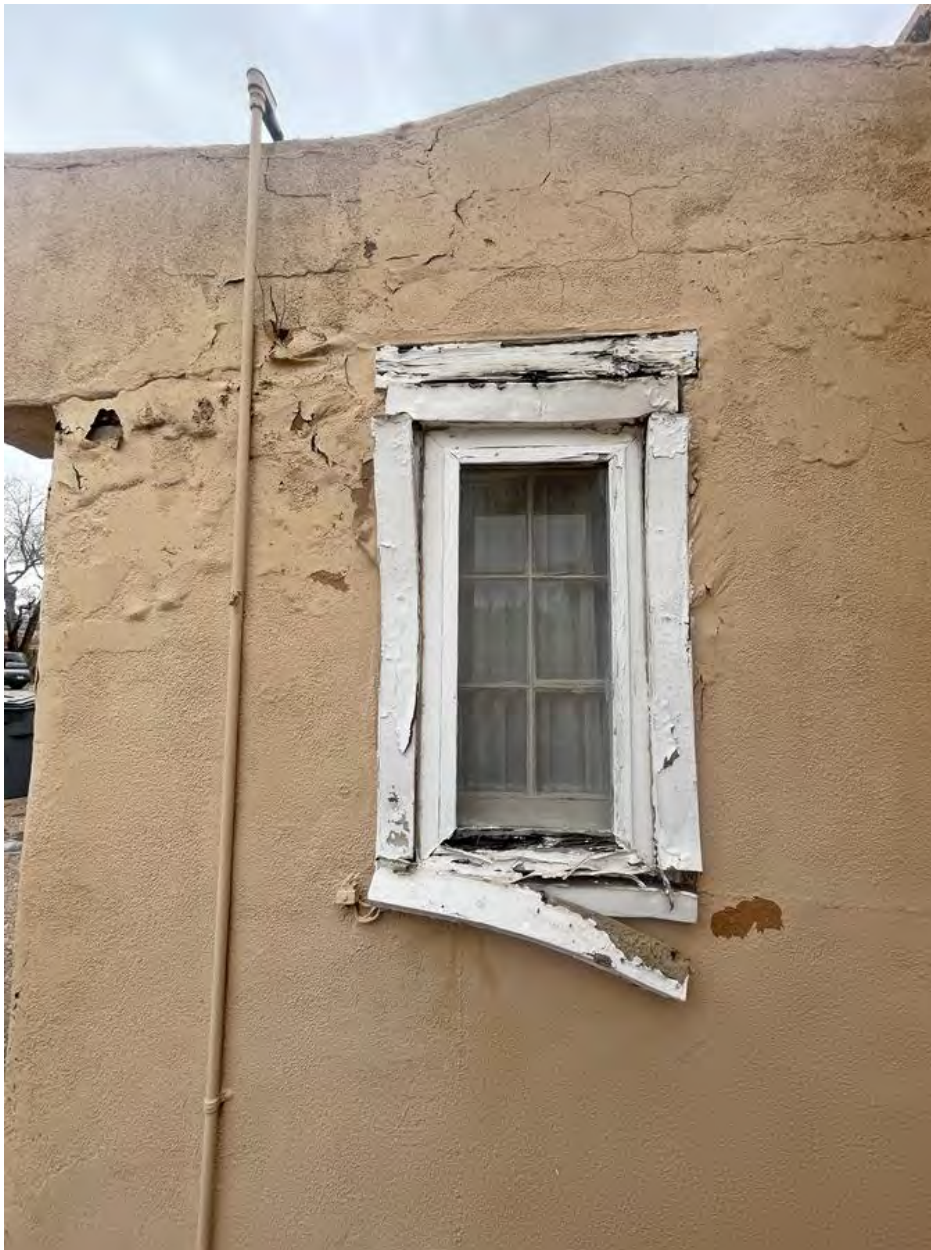
Photo 30: East elevation. Addition and window detail. Camera facing south.
