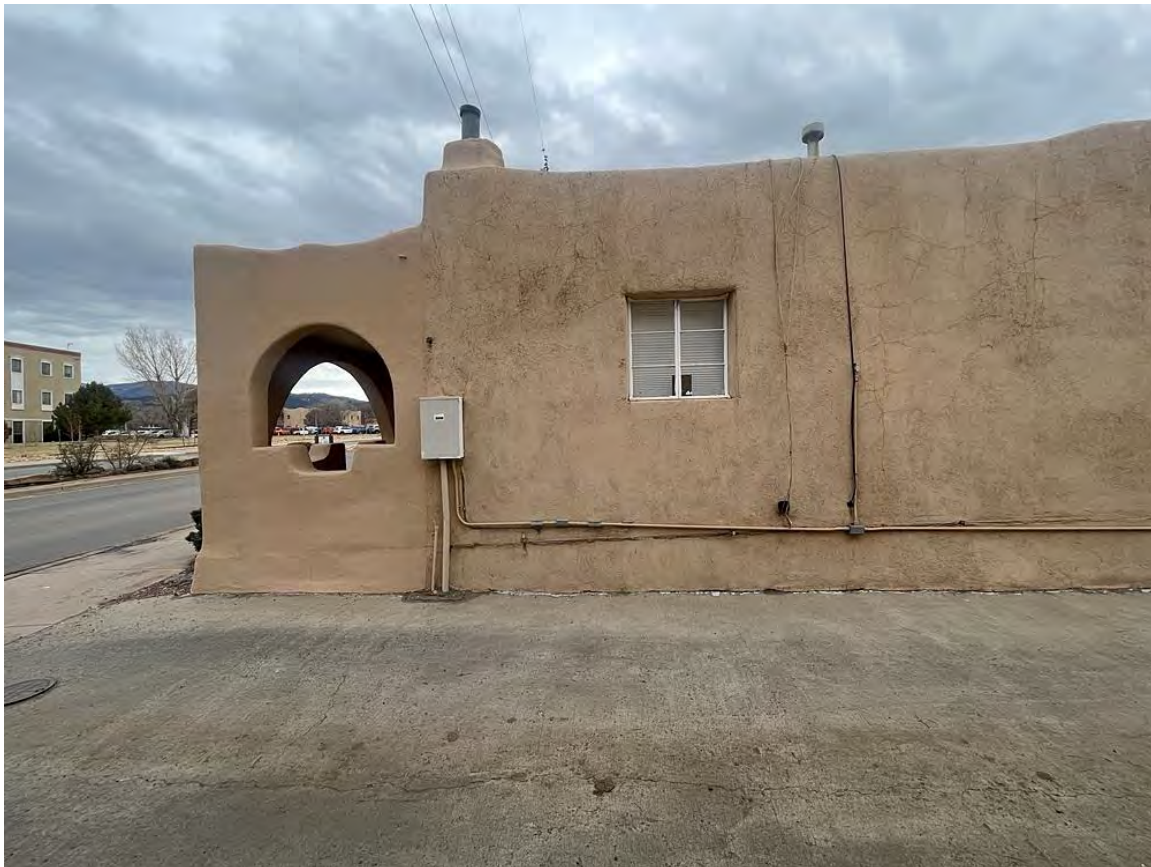
Photo 34: Camera facing east. North end. Camera facing east.
