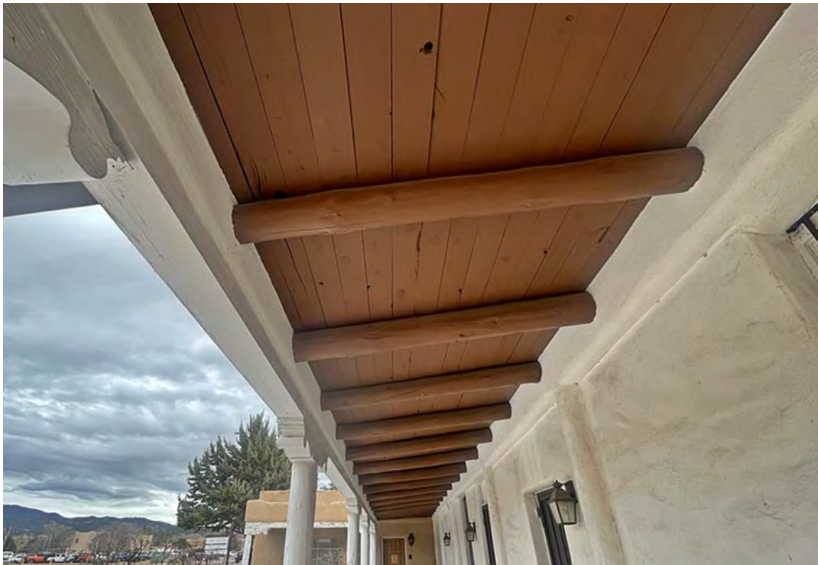
Photo 5: North elevation, portal decking. Camera facing up.
