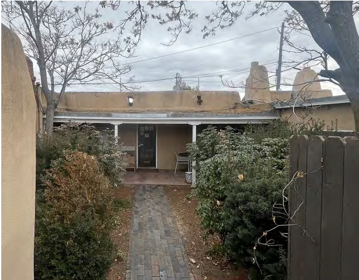
Photo 15: West elevation, post-1948 portal. Camera facing east.
