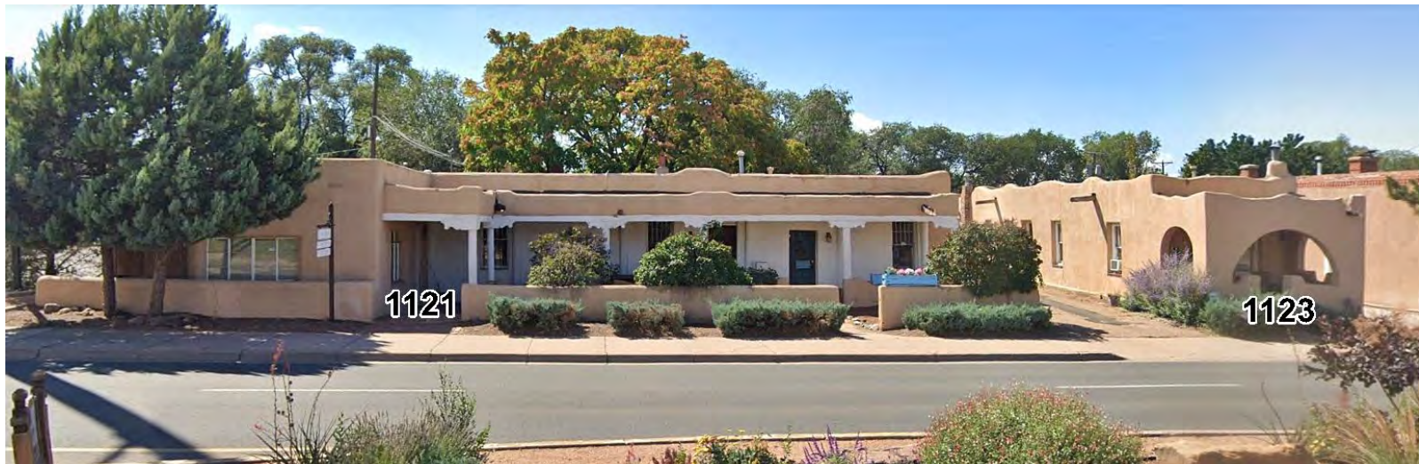
Photo 2: Setting of the Alarid Property. Google Street View, September 2022.
