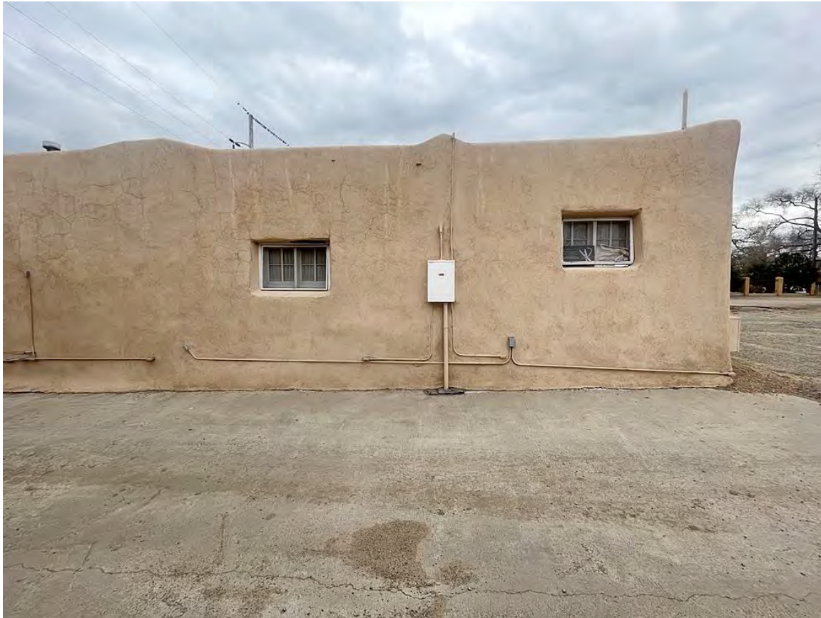
Photo 33: West elevation. South end. Camera facing east.
