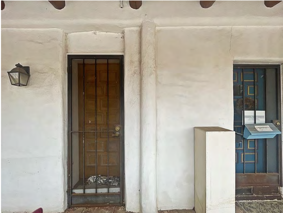
Photo 9: North elevation, portal north wall. Camera facing south.
