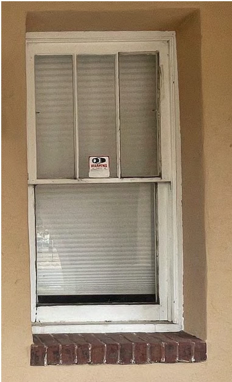
Photo 26: North elevation. Window detail. Camera facing south.
