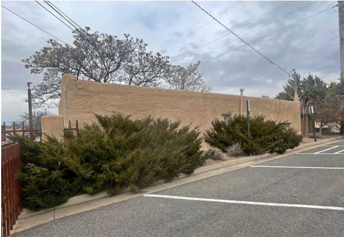
Photo 18: East elevation. Camera facing northwest.
