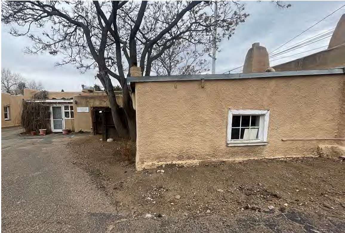
Photo 16: South elevation, pre-1930 addition. Camera facing north.
