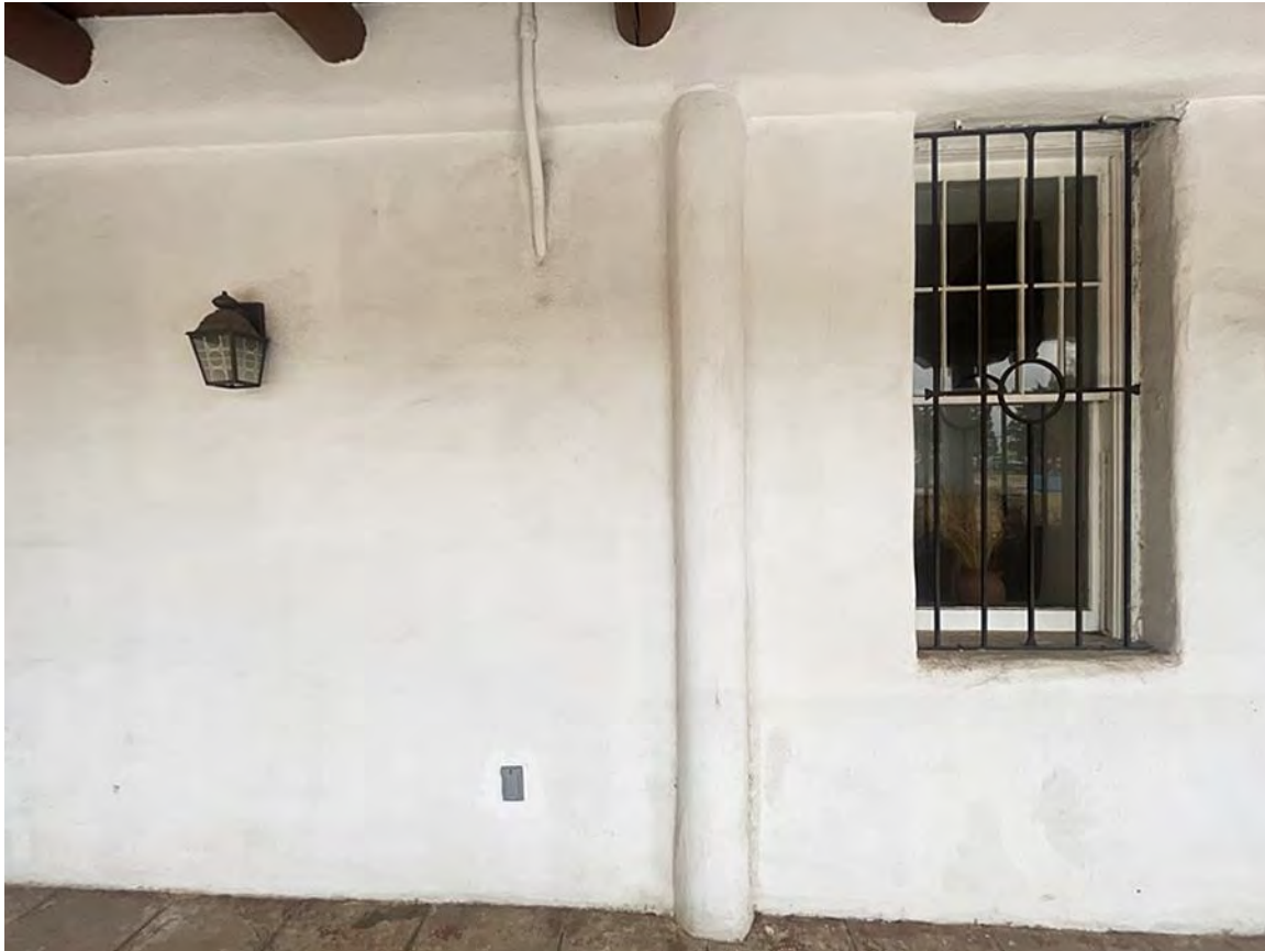
Photo 8: North elevation, portal north wall. Camera facing south.
