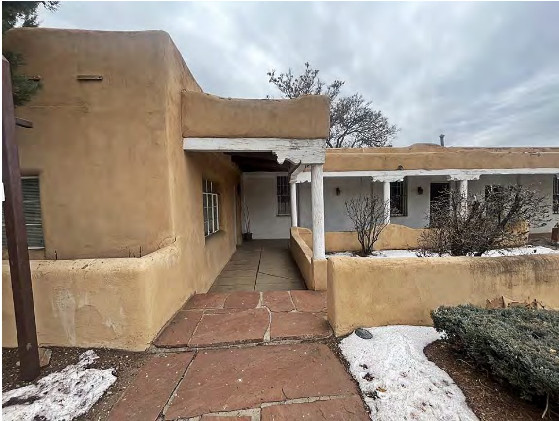
Photo 4: North elevation, portal. Camera facing south.
