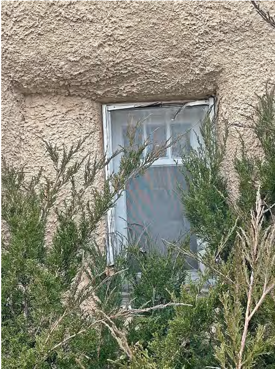
Photo 22: East elevation. Window detail. Camera facing west.
