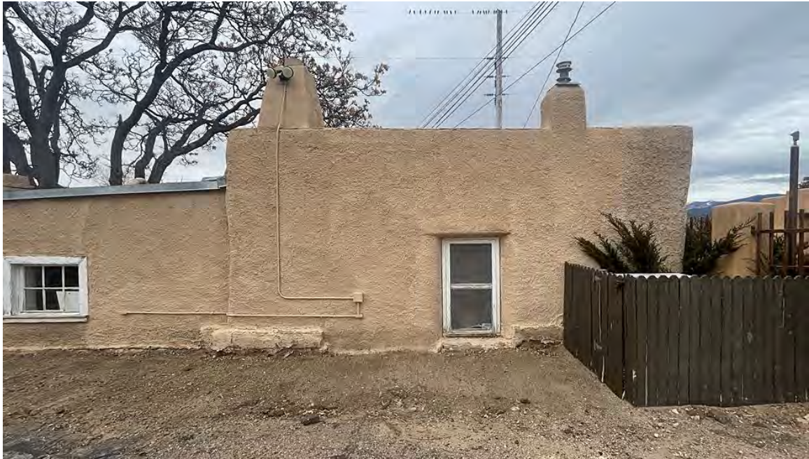
Photo 17: South elevation, original building or pre-1930 addition. Camera facing north.
