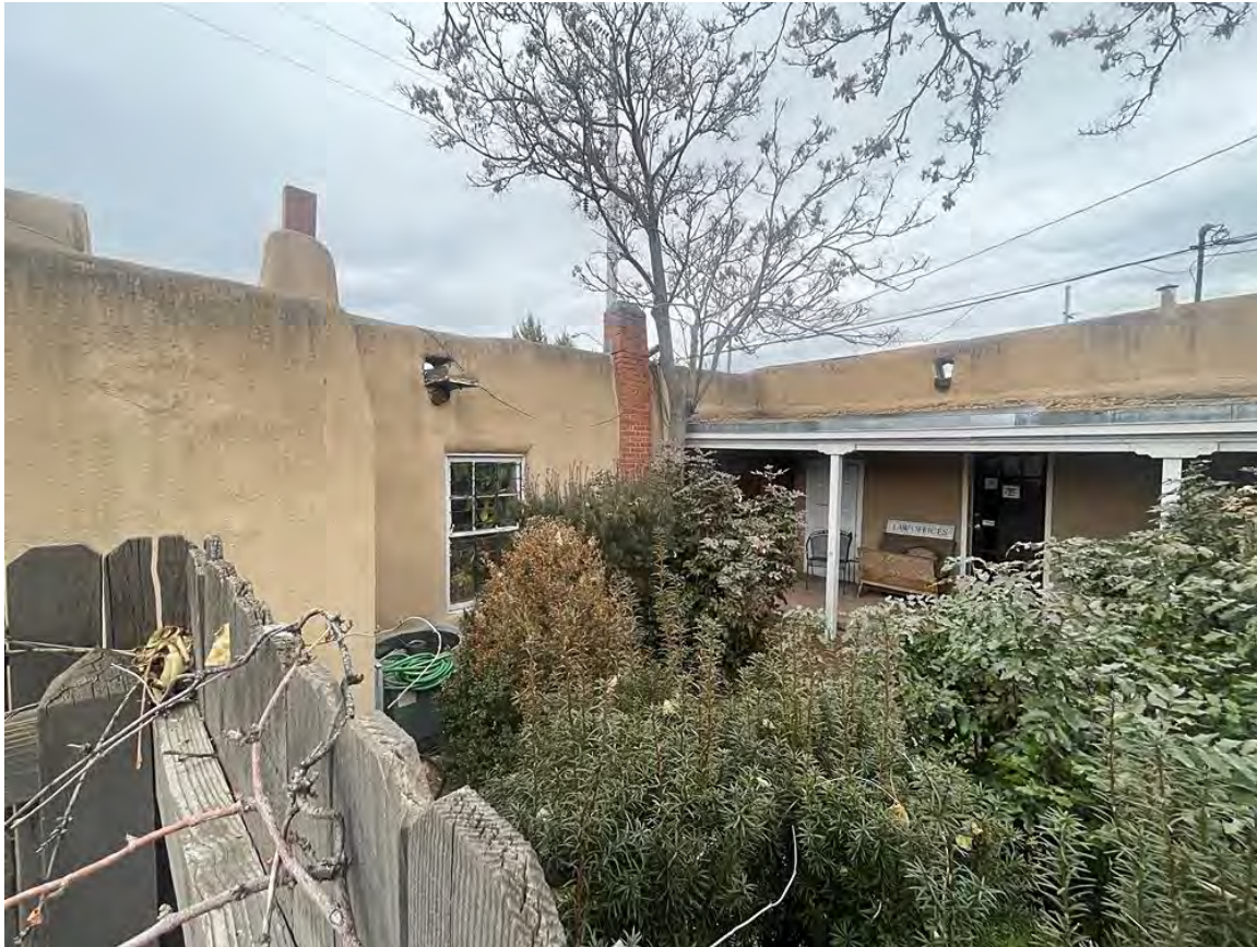
Photo 14: South elevation, east and post-1948 portal. Camera facing northeast.
