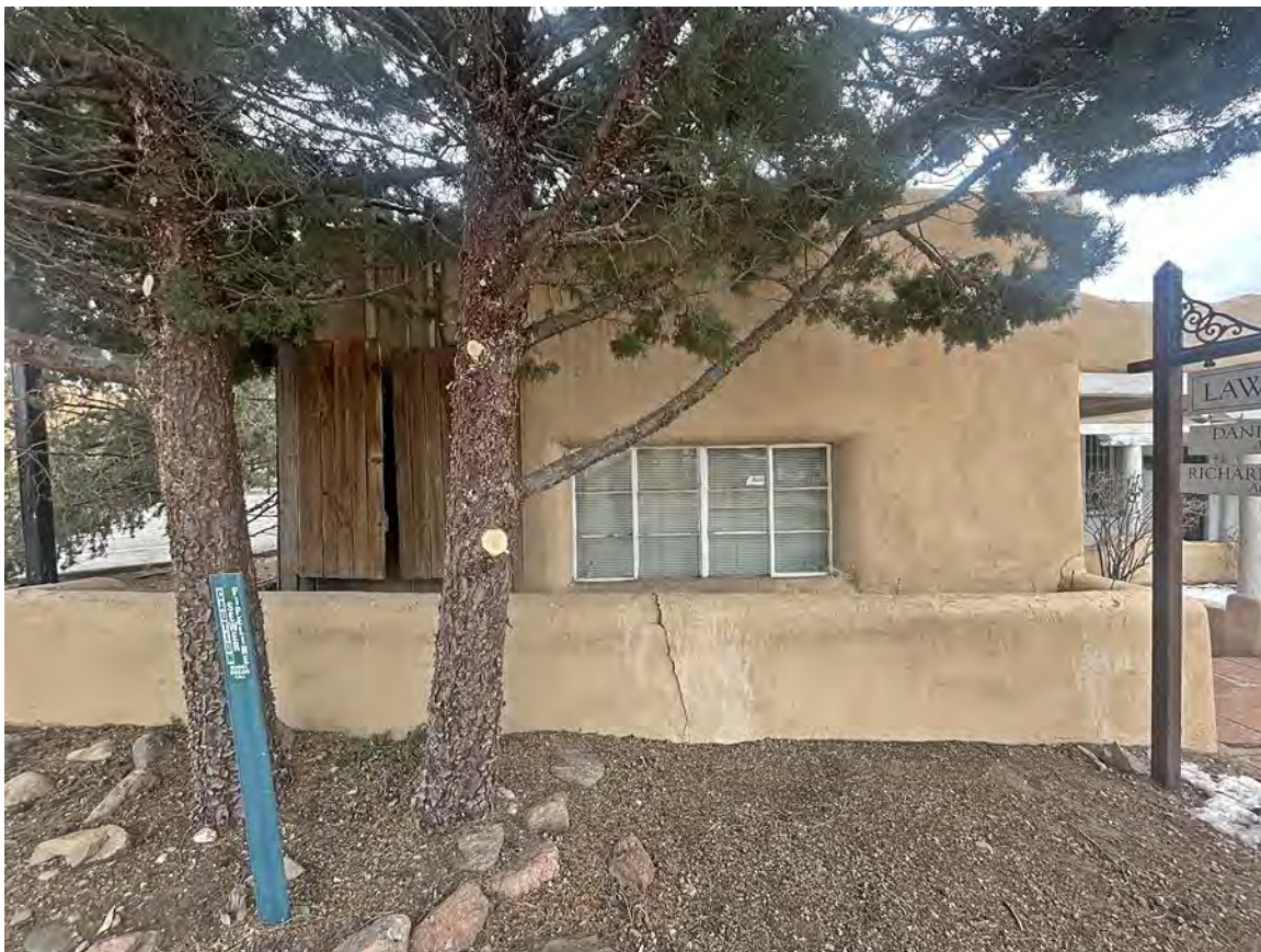
Photo 3: North elevation, east end. Camera facing south.
