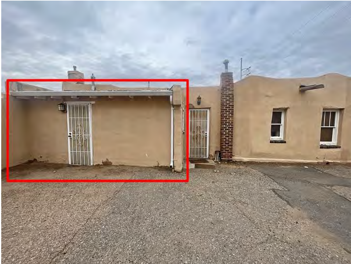
Photo 31: East elevation. Post-1978 addition. Camera facing west.
