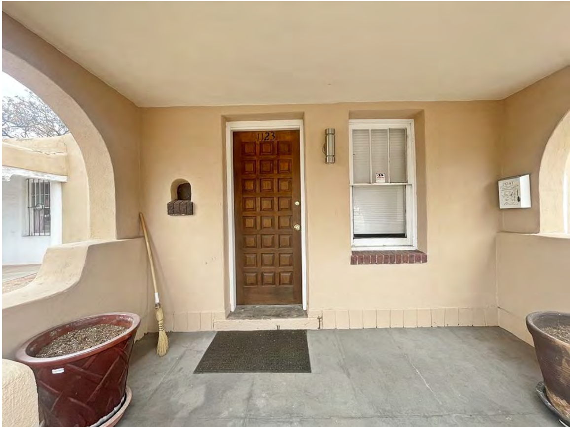
Photo 25: North elevation. Porch. Camera facing south.
