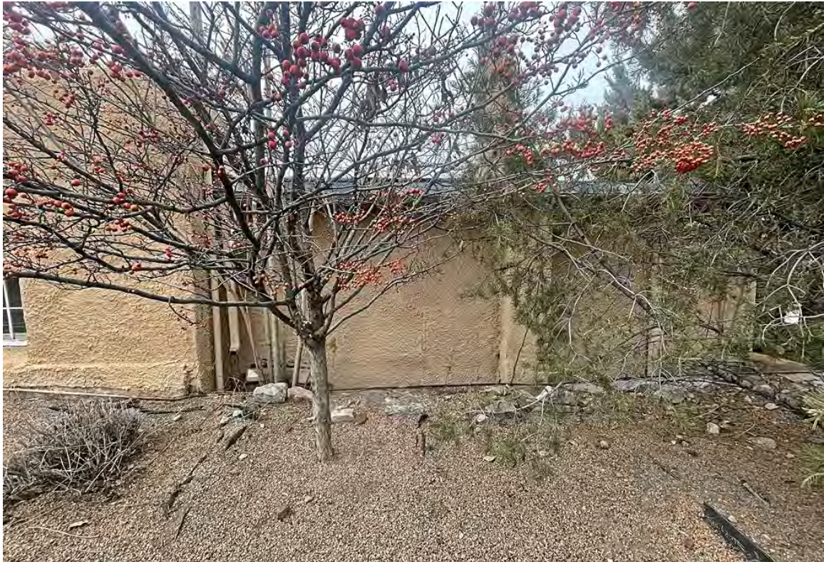
Photo 23: East elevation, pre-1930 addition. Camera facing west.
