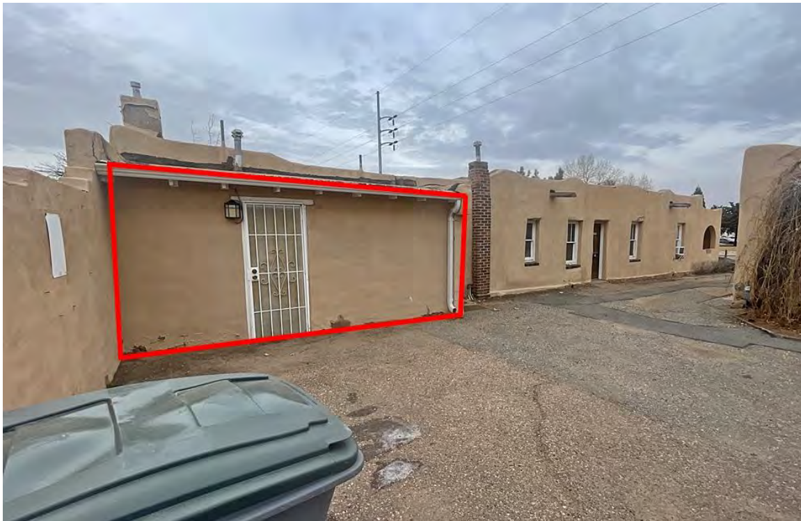
Photo 27: East elevation. Camera facing northwest.
