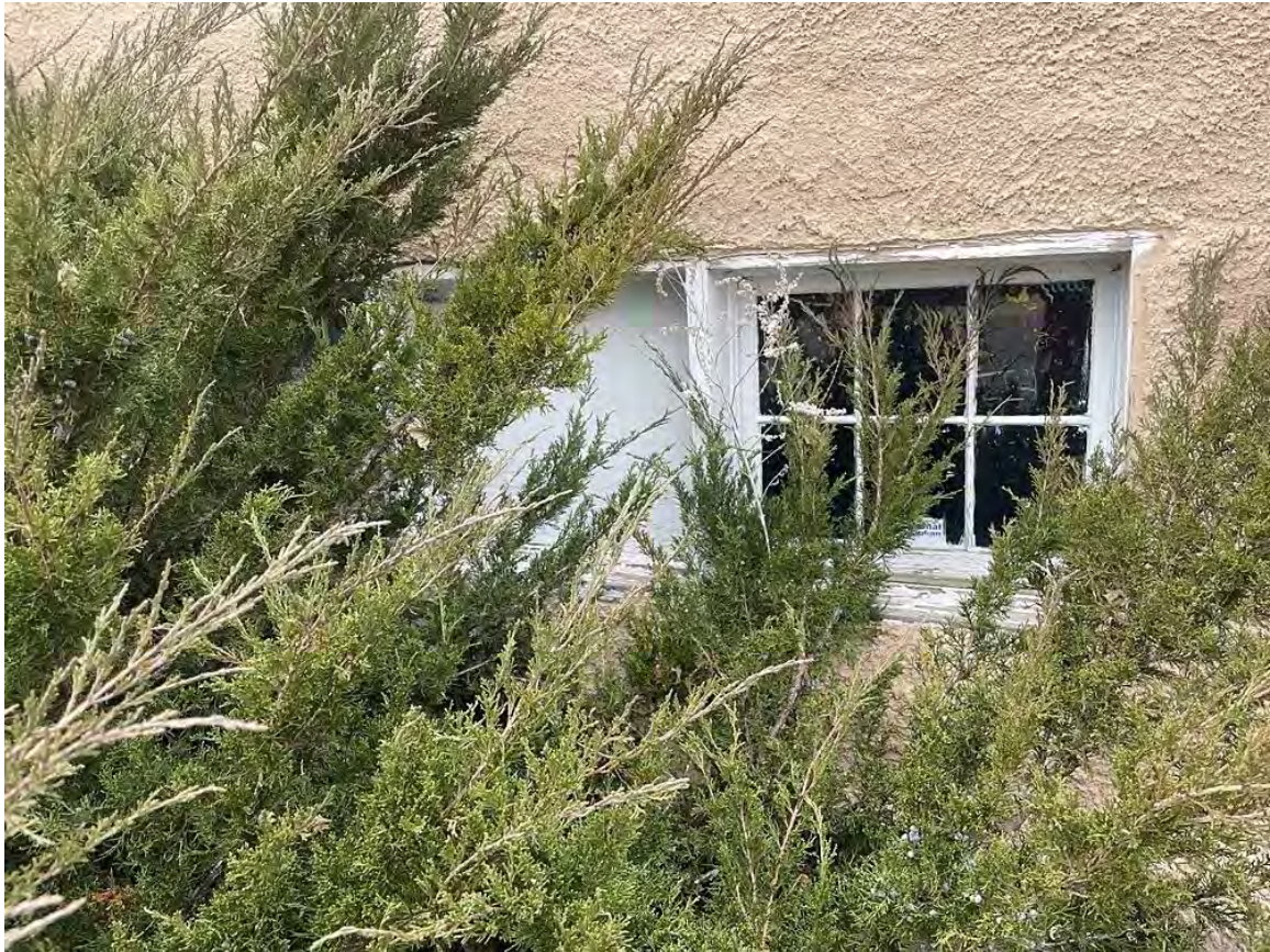
Photo 21: East elevation. Window detail. Camera facing west.
