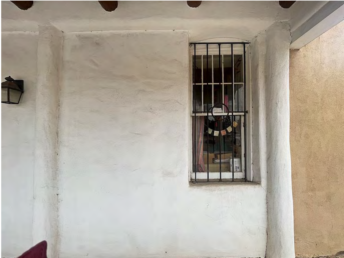
Photo 10: North elevation, portal north wall. Camera facing south.
