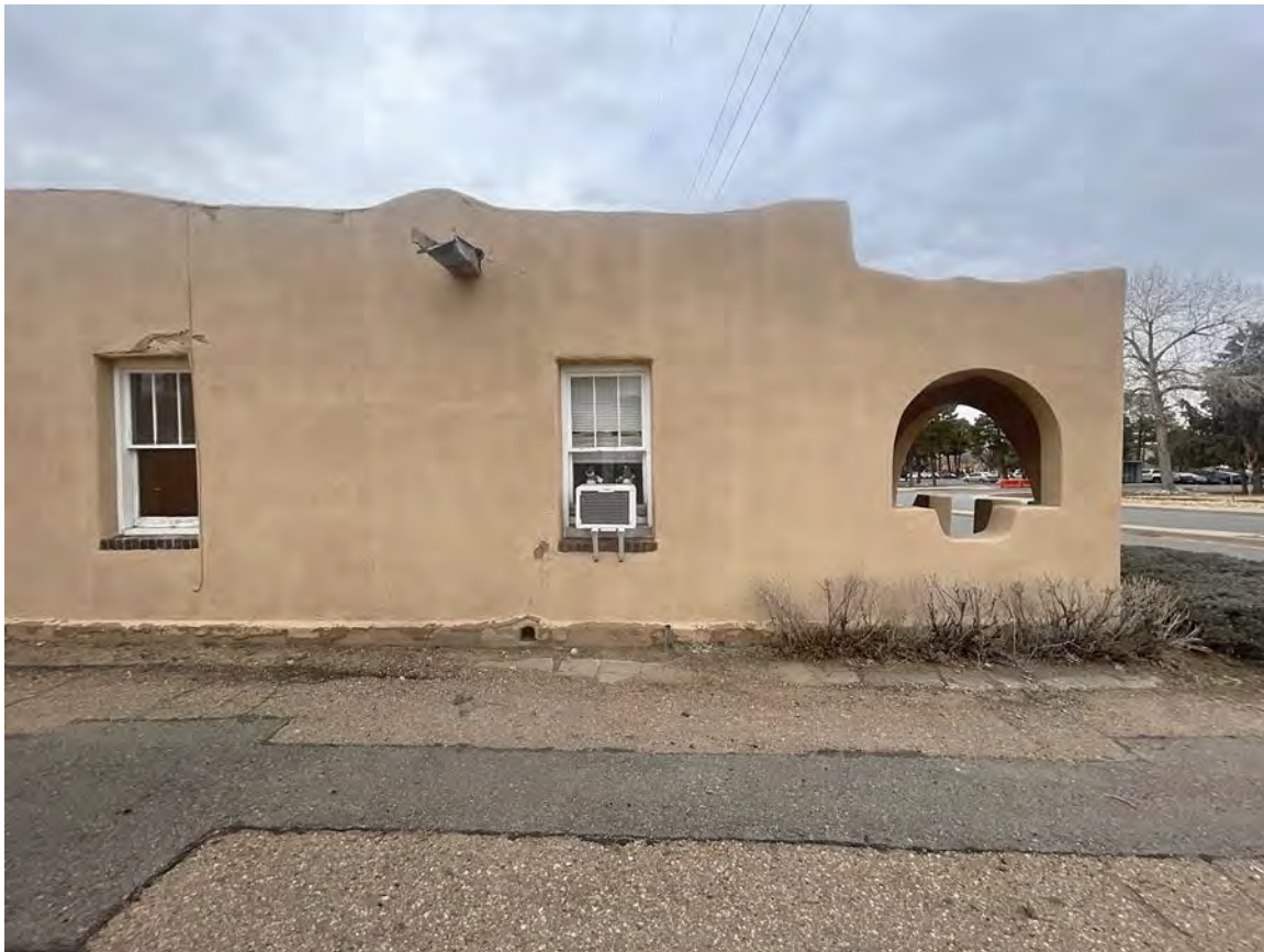
Photo 28: East elevation. North section. Camera facing west.
