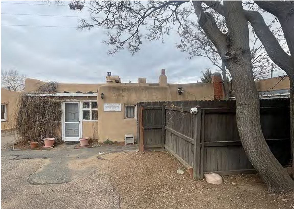
Photo 12: South elevation, west end. Camera facing north.
