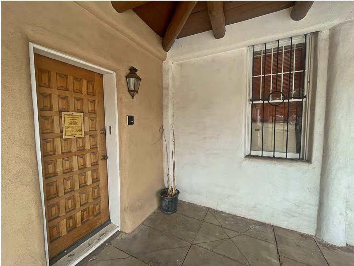
Photo 7: North elevation, portal southeast corner. Camera facing southeast.
