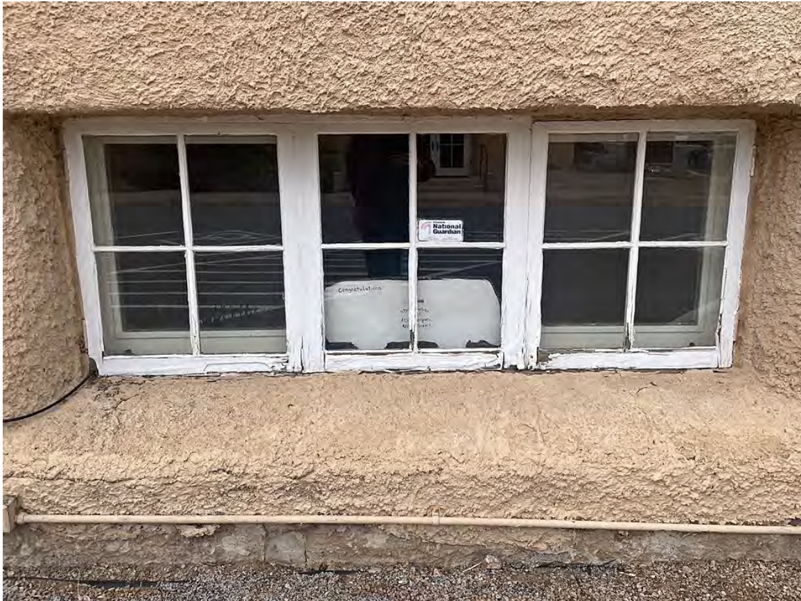
Photo 20: East elevation. Window detail. Camera facing west.
