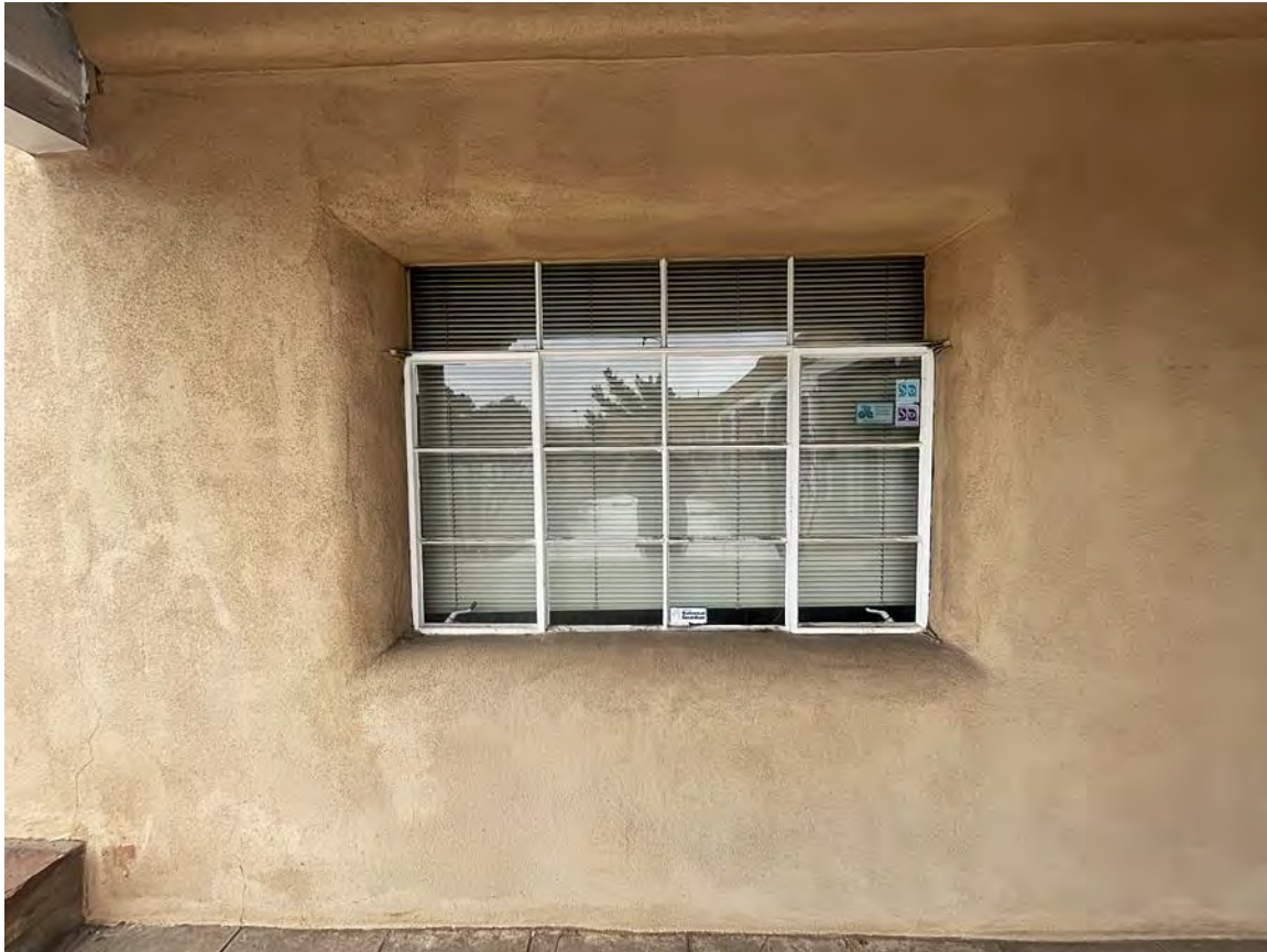
Photo 6: North elevation, portal west wall. Camera facing east.
