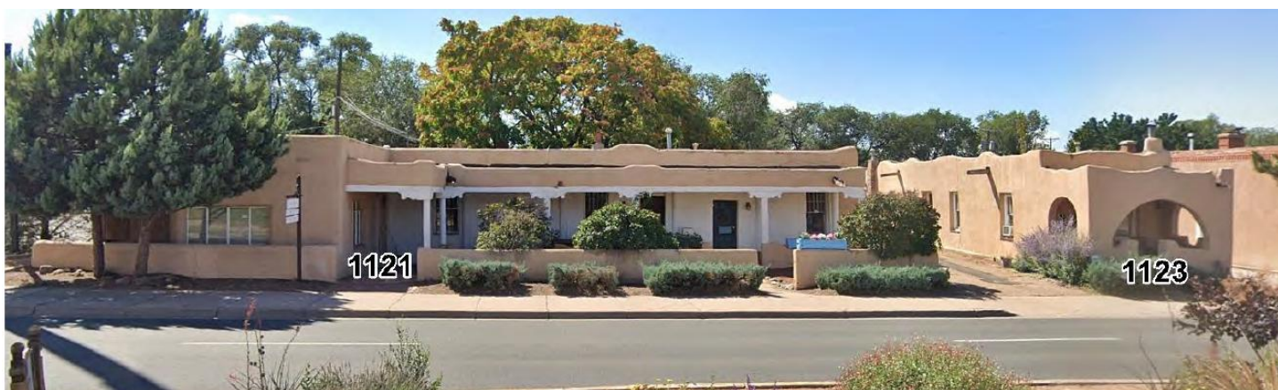
Figure 2: 1121 and 1123 Paseo de Peralta
