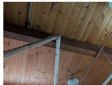
6) Metal Bracing in Shop
