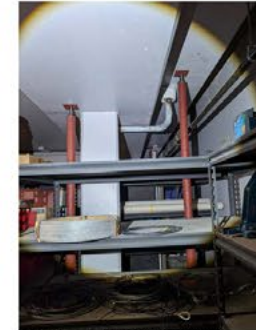
2) Basement Bracing
