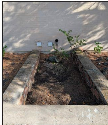
3) Roof Water Catchment Area
