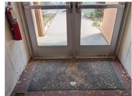
6) Exit Doors in Corridor 115
