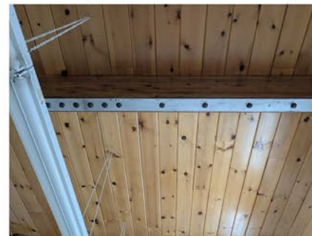
4) Metal Bracing in Classrooms
