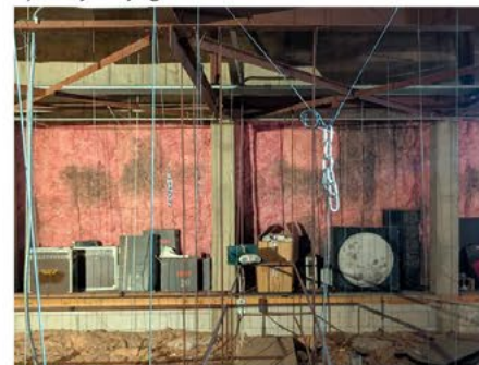
5) Wall Insulation in Attic Level
