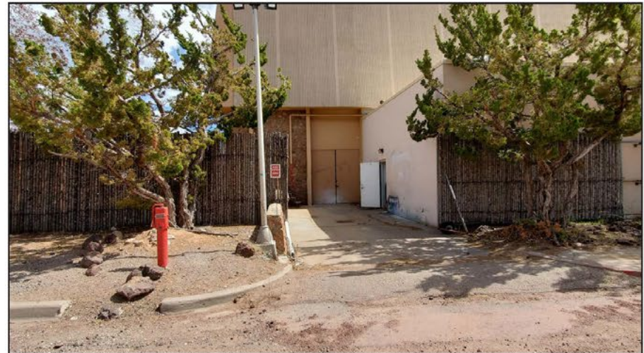
4) View of loading area
