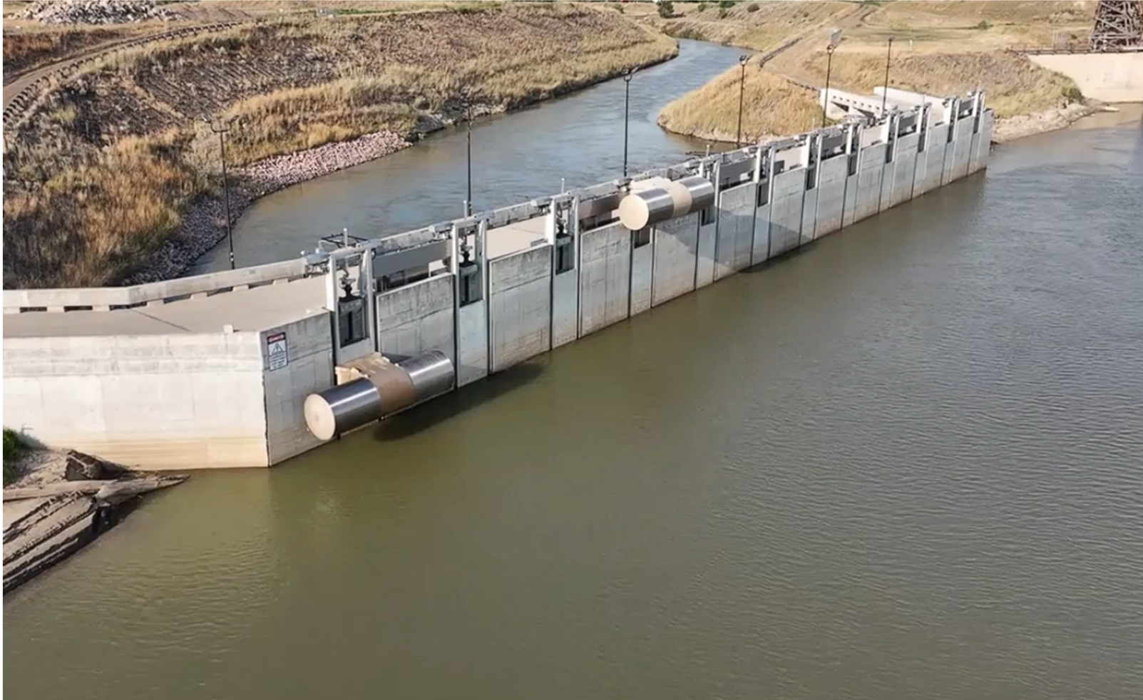
LOWER YELLOWSTONE DIVERSION DAM, MT
