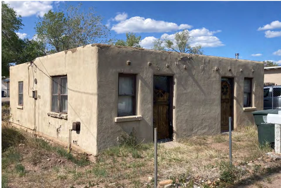
Southwest corner – looking northeast – May 2025
