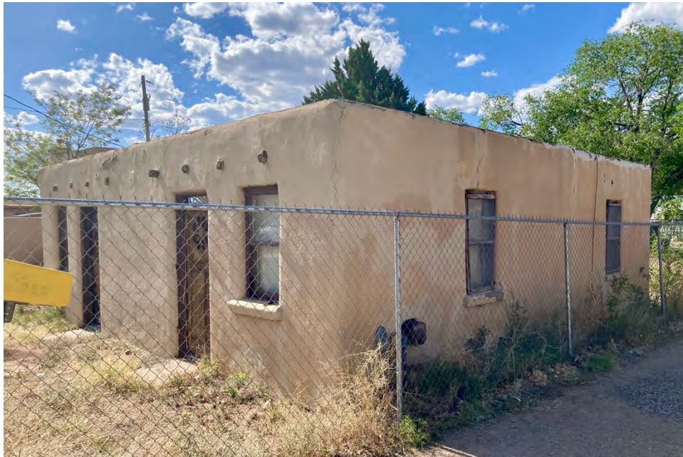
Southeast corner- looking northwest - May 2025
