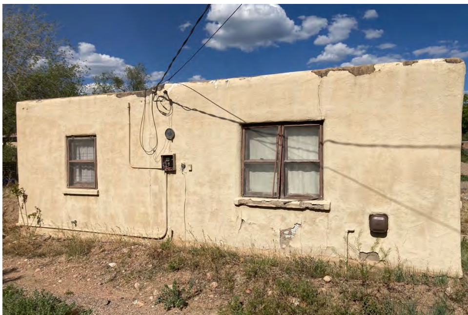
West façade – looking east – May 2025
