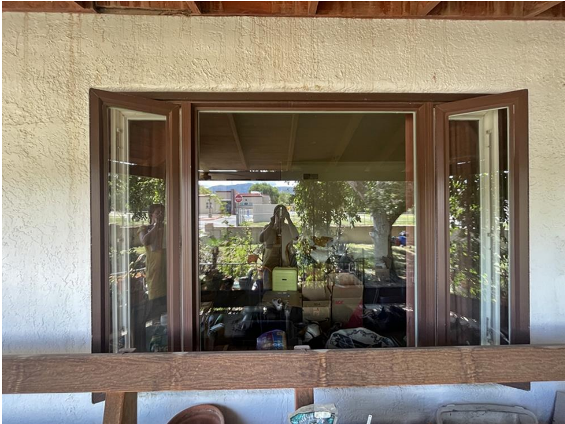
Photo 7: Porch. East elevation window. Camera facing west.
