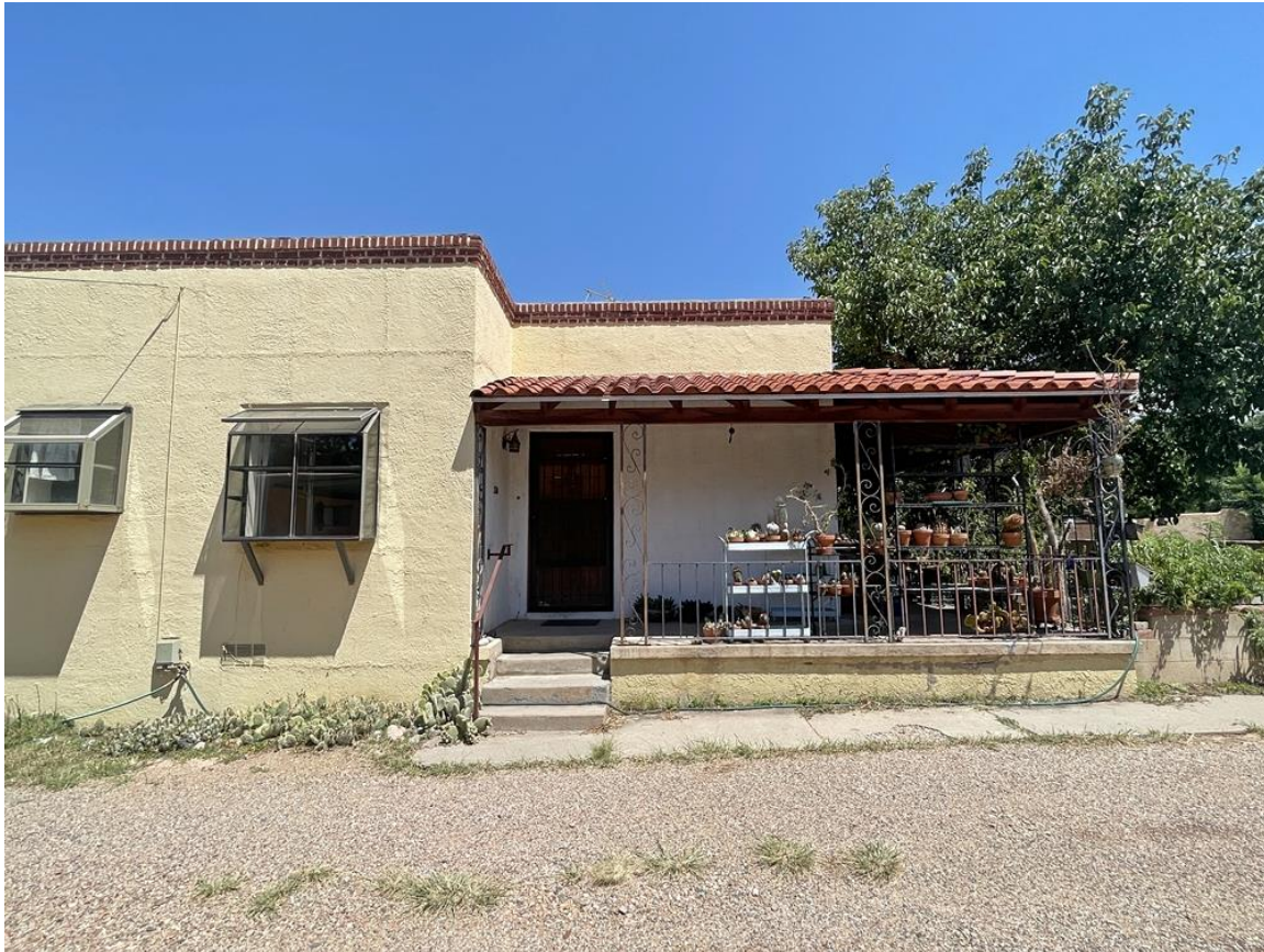
Photo 10: South elevation, east end. Camera facing north.
