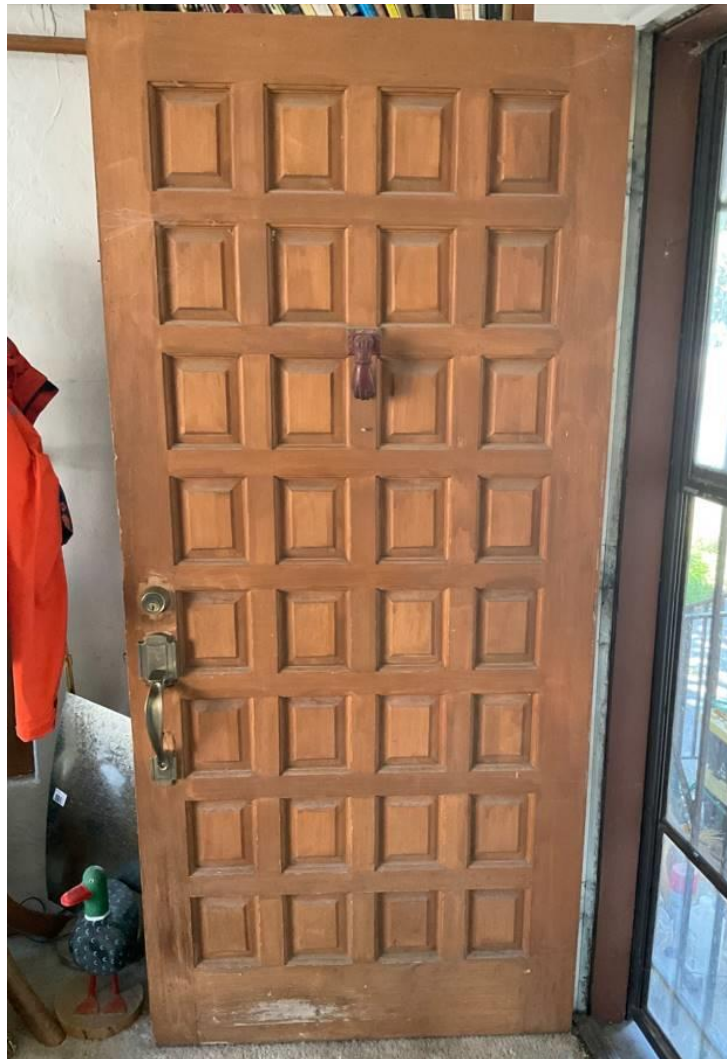
Photo 8: Porch. East elevation entry door to apartment. David Kozlowski, August 5, 2025.
