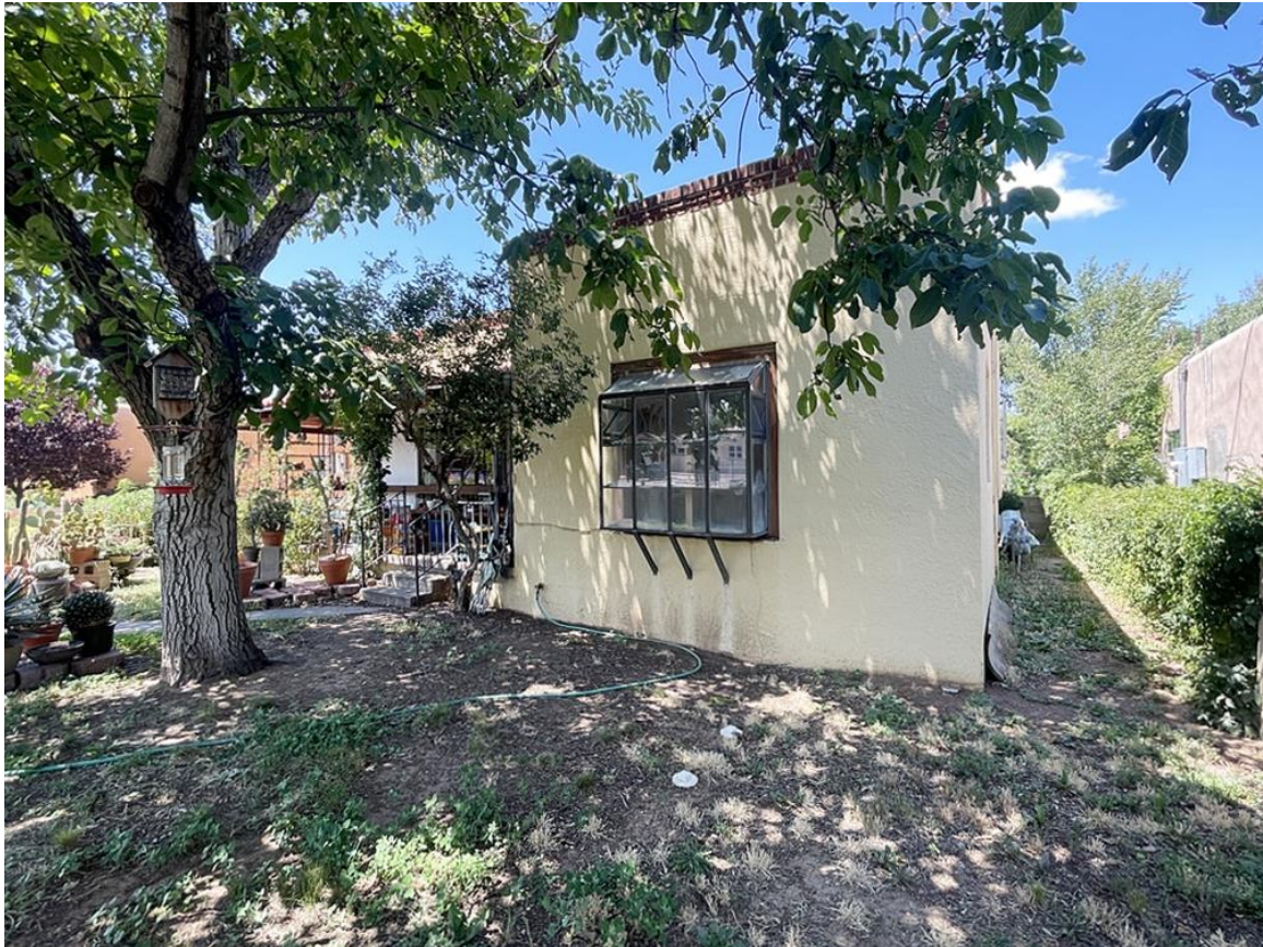
Photo 9: East elevation. Camera facing southwest.
