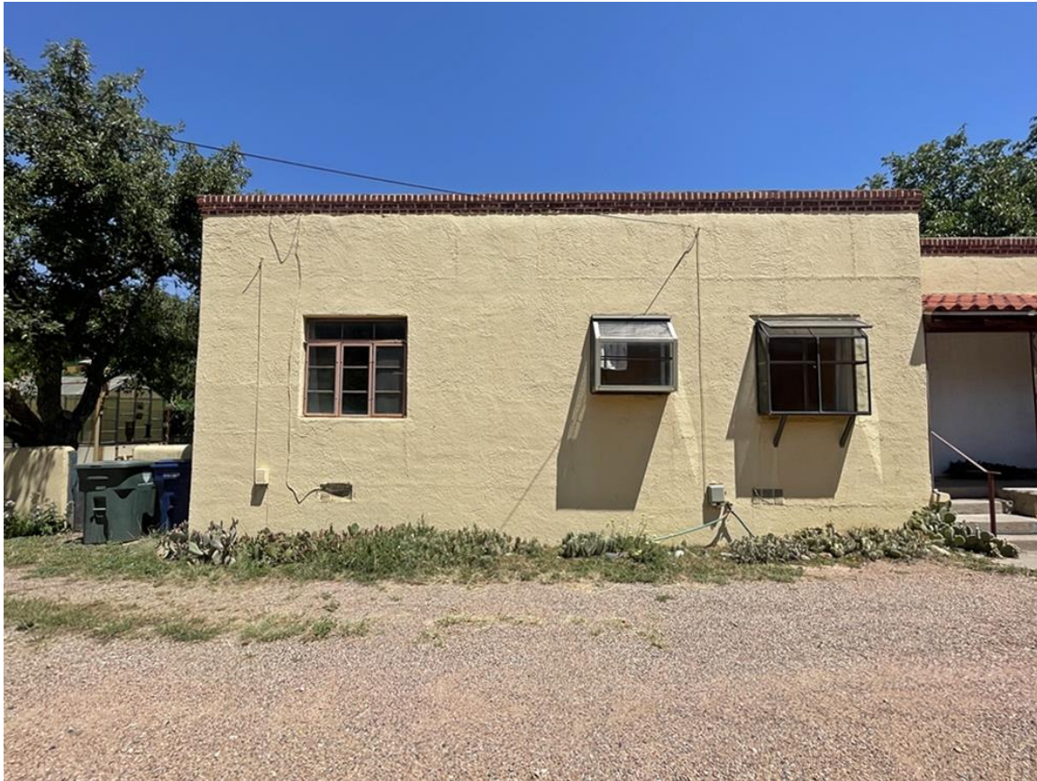
Photo 11: South elevation, west end. Camera facing north.
