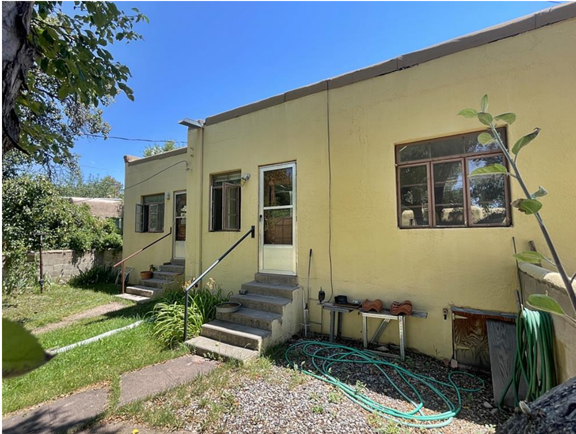
Photo 12: West elevation. Camera facing northeast.
