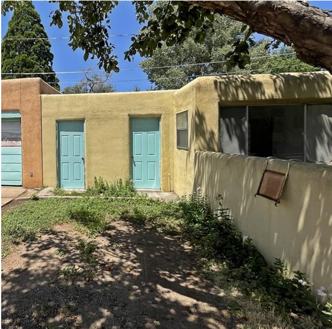
Photo 16: Former garage. Camera facing west.
