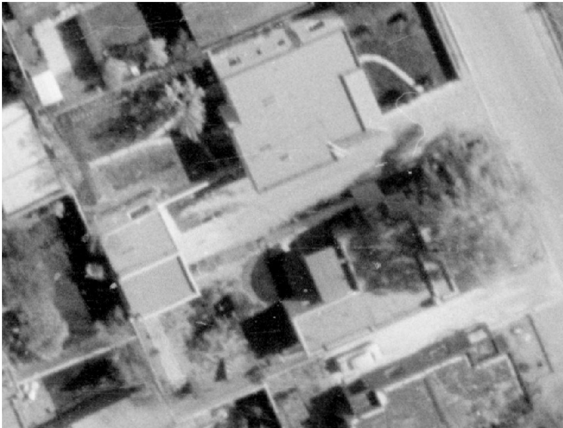
Figure 4: May 1, 1973, aerial photograph. Note garage has no attachment, and large window across its north elevation.
