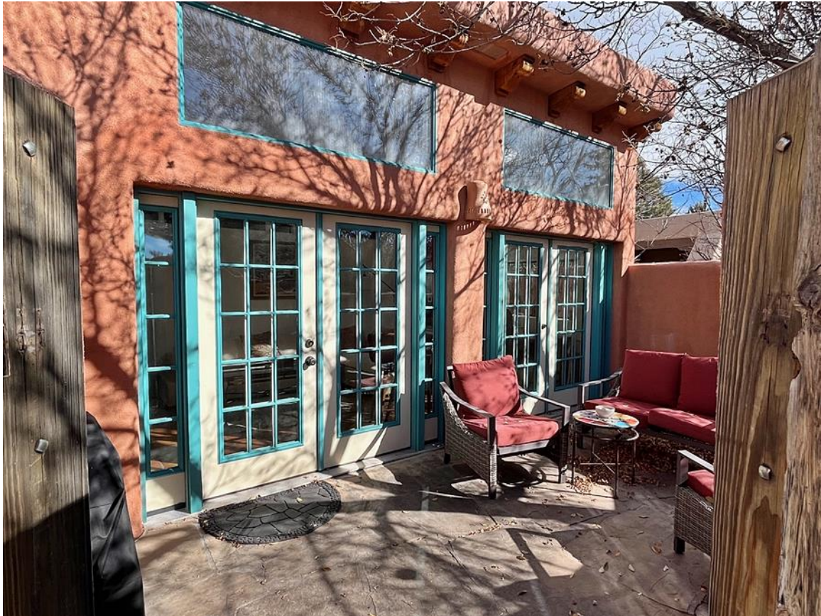
Photo 21: South elevation. Camera facing northeast.
