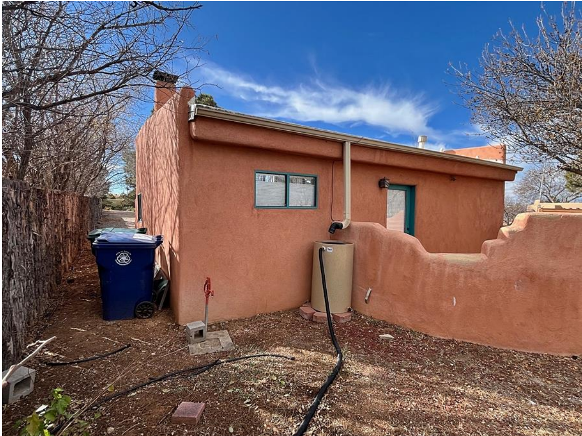
Photo 20: East and north elevations. Camera facing southwest.
