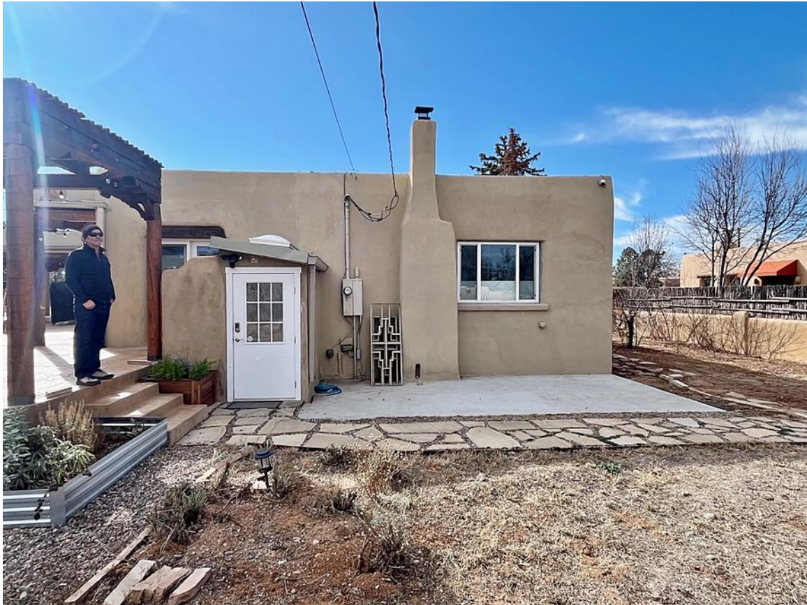
Photo 15: North elevation. Camera facing southwest.
