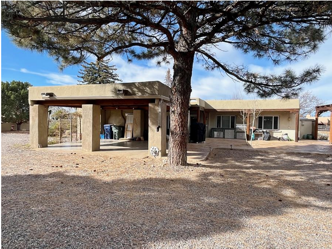
Photo 12: East elevation. Camera facing northwest.
