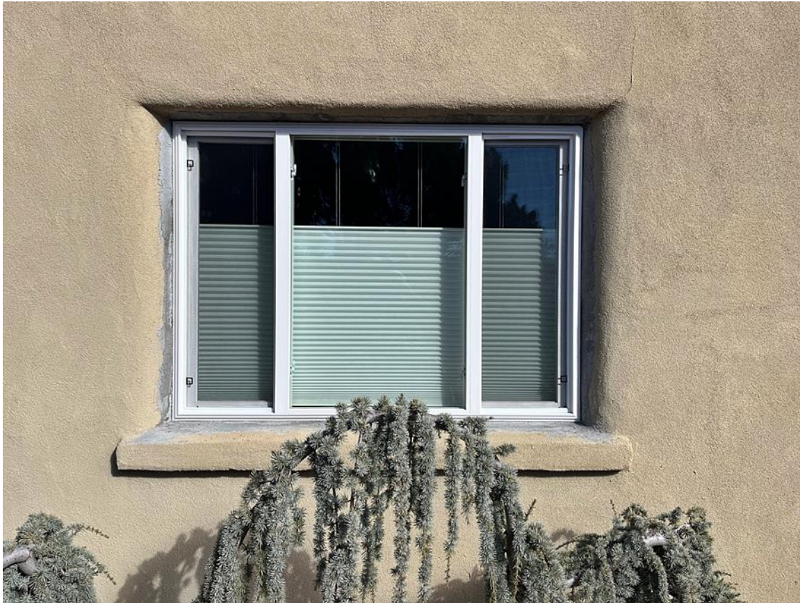
Photo 10: South elevation. Window at living room. Camera facing northeast.
