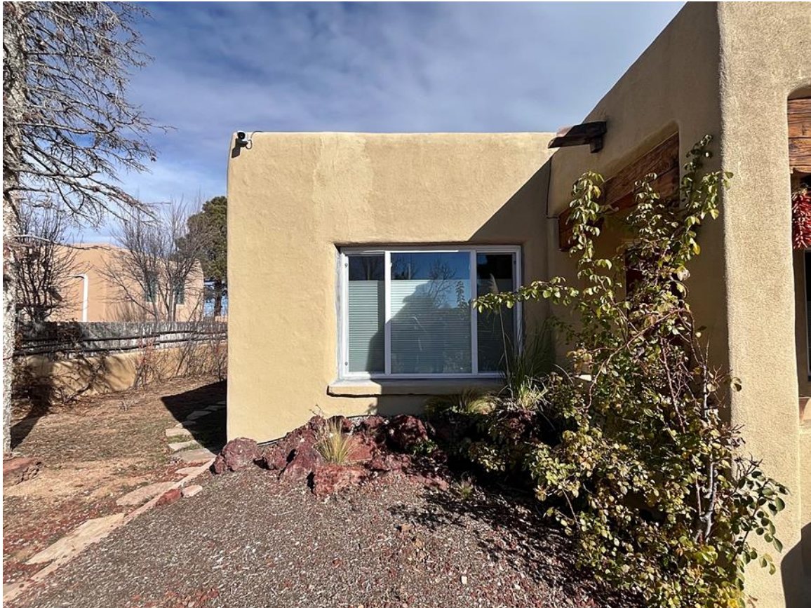
Photo 7: South elevation. West section at sitting room. Camera facing northeast.
