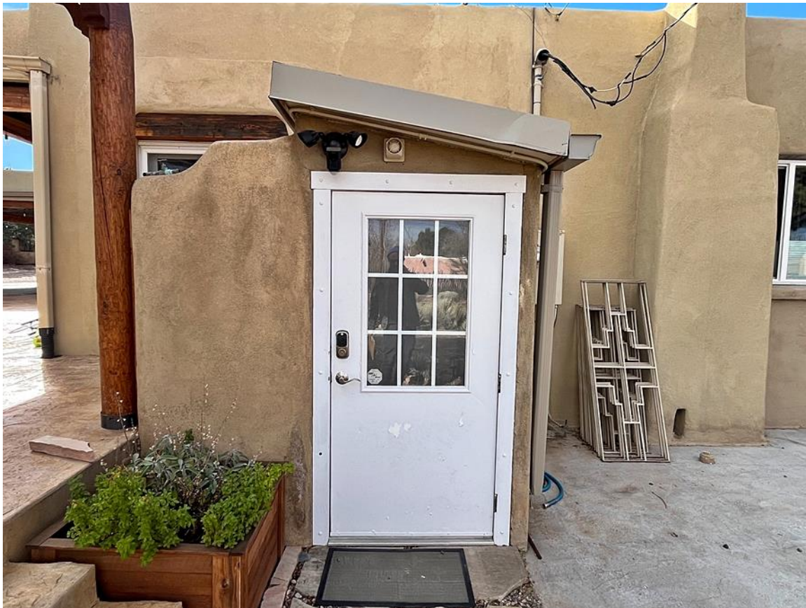
Photo 17: North elevation. Non-historic basement entry.
