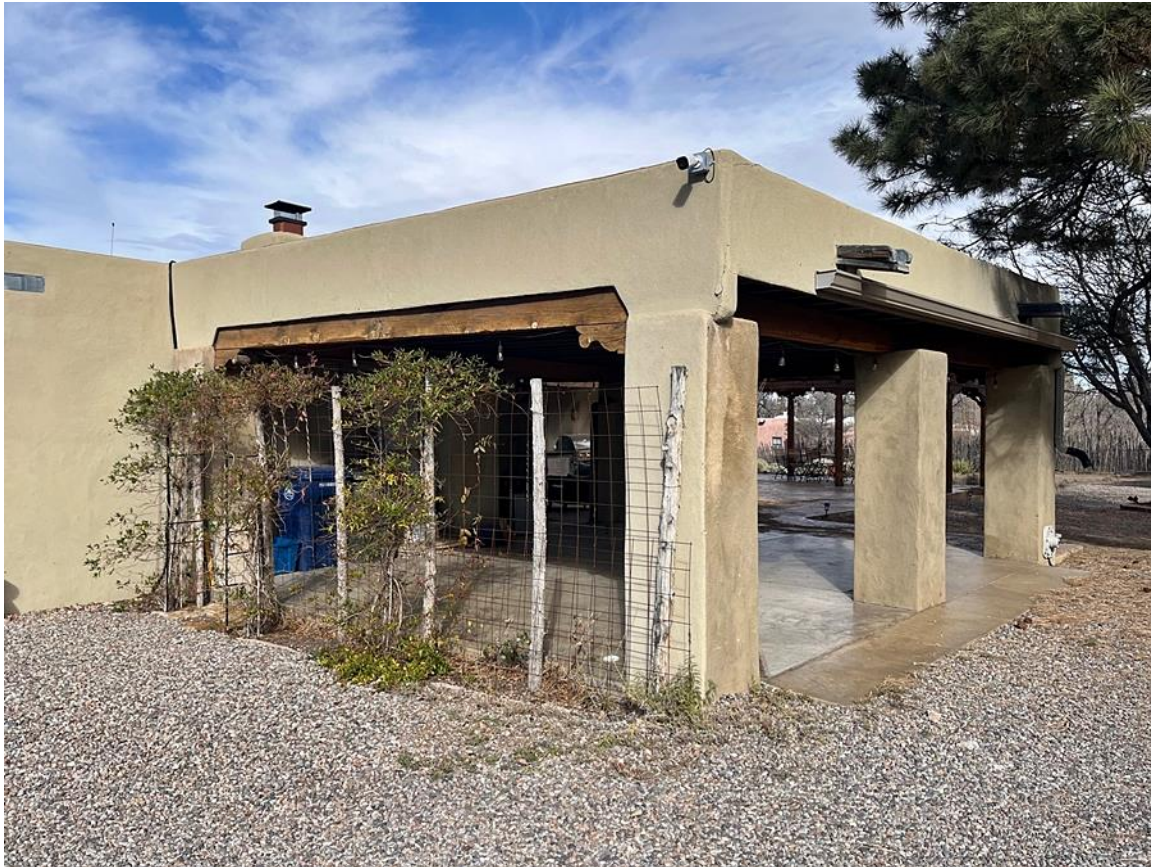
Photo 11: South and east elevations. Carport. Camera facing northwest.
