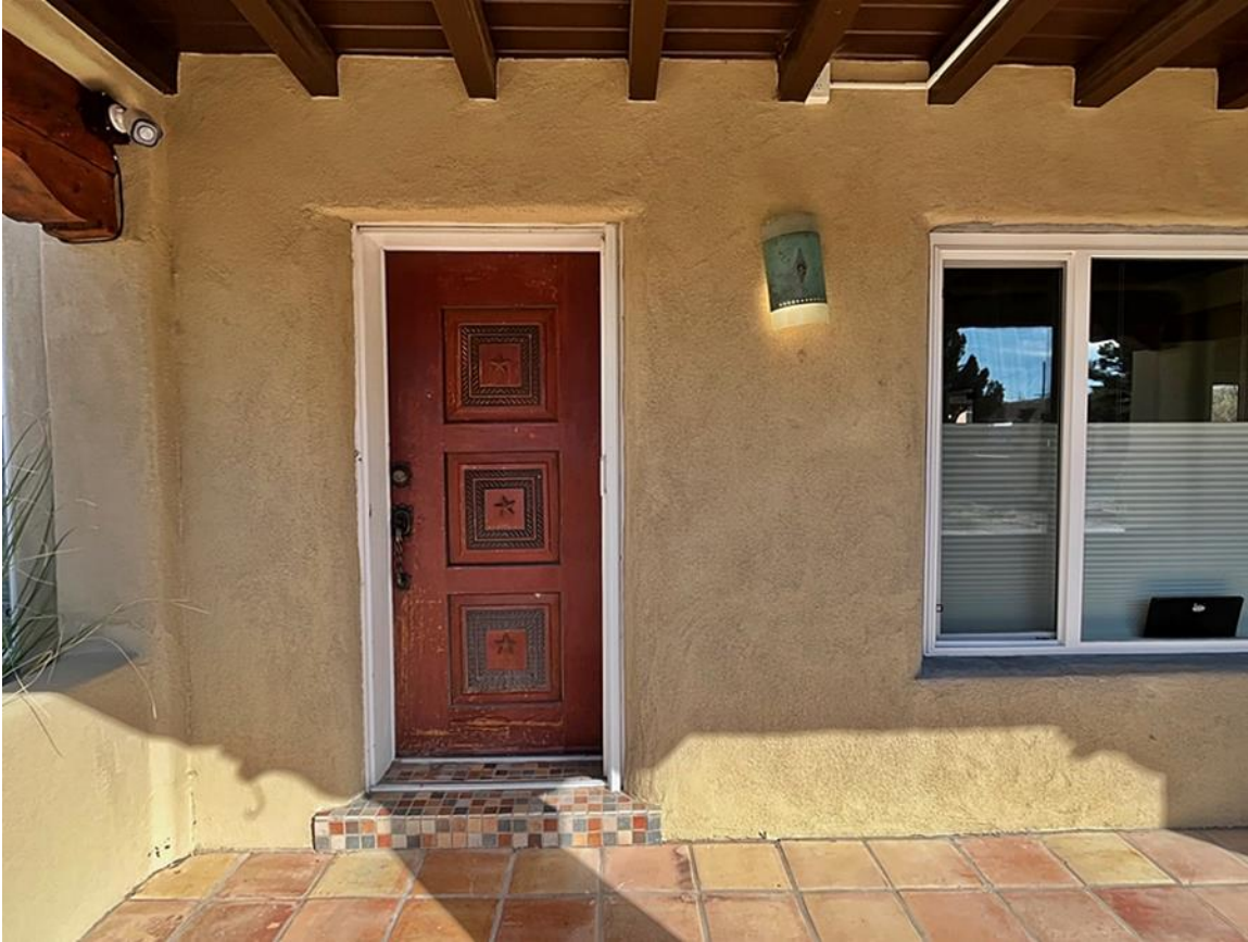
Photo 9: South elevation. Entry door. Camera facing northeast.
