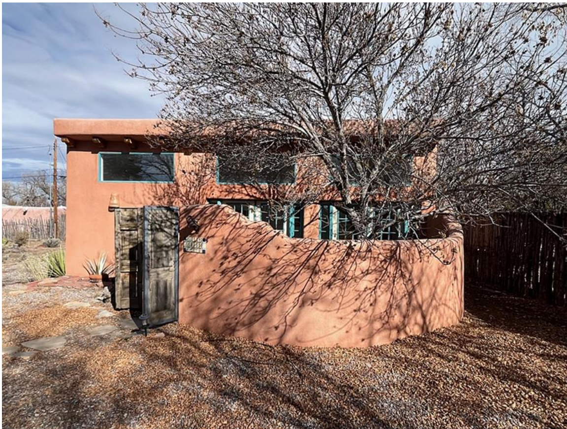
Photo 19: South elevation. Camera facing northeast.
