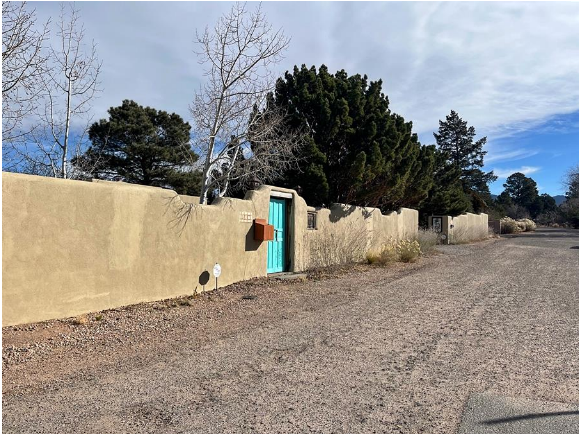
Photo 5: Front privacy wall. Camera facing northeast.
