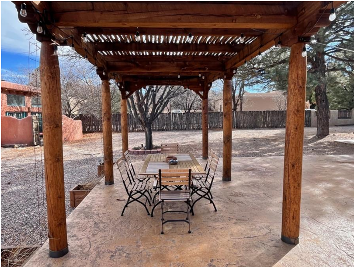
Photo 4: Pergola. Camera facing southeast.
