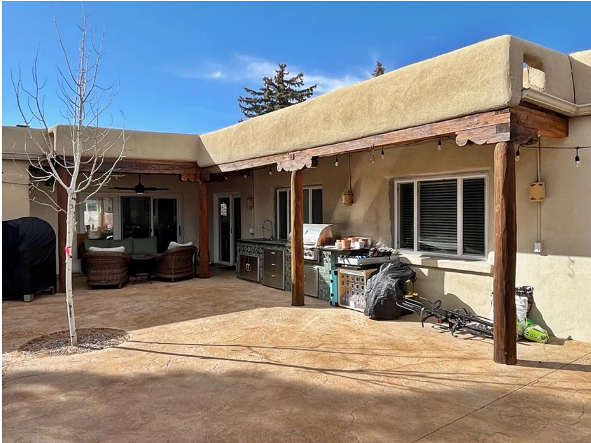
Photo 14: East elevation. Non-historic portal. Camera facing southwest.
