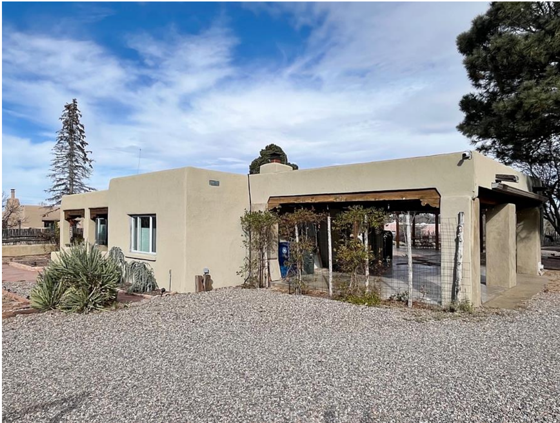
Photo 6: South elevation. Camera facing northwest.
