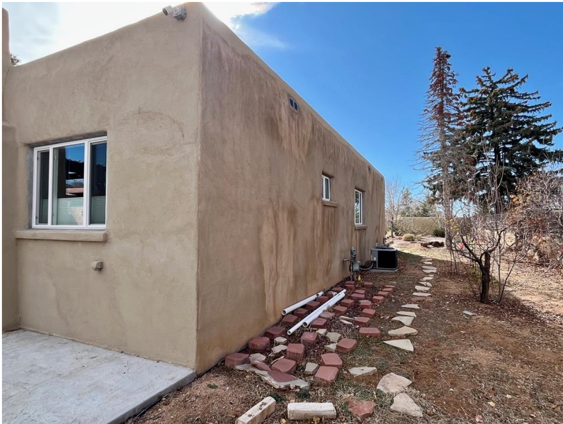
Photo 18: West elevation. Camera facing southeast.
