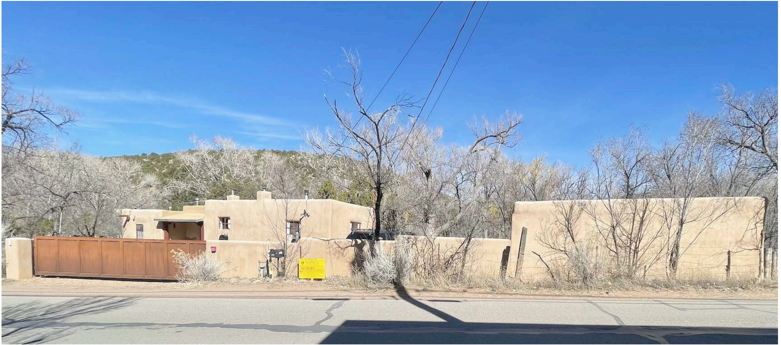
WALL AND GATE SOUTH SIDE 1489 CANYON ROAD
