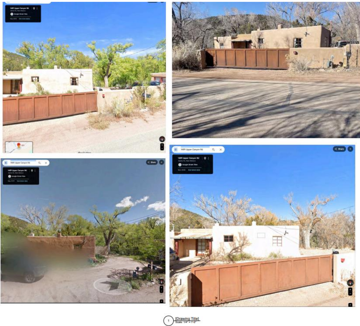
Figure 6. Overview of 1489 Canyon Road.
