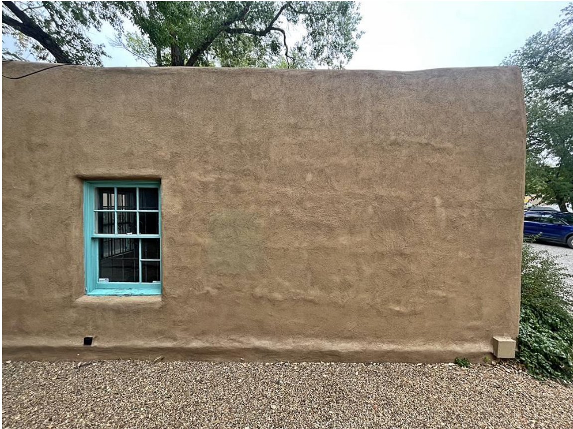
Photo 19: South elevation. Camera facing north.
