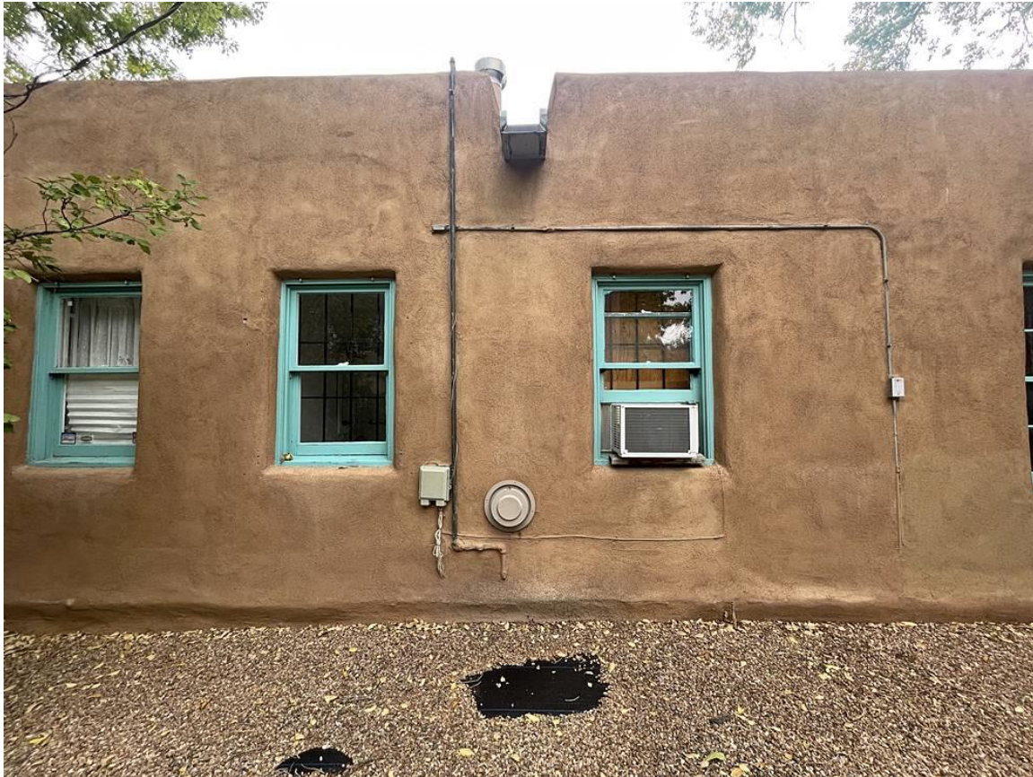
Photo 21: West elevation, middle section. Camera facing east.
