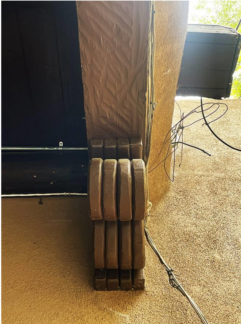
Photo 11: West elevation. Camera facing up.
