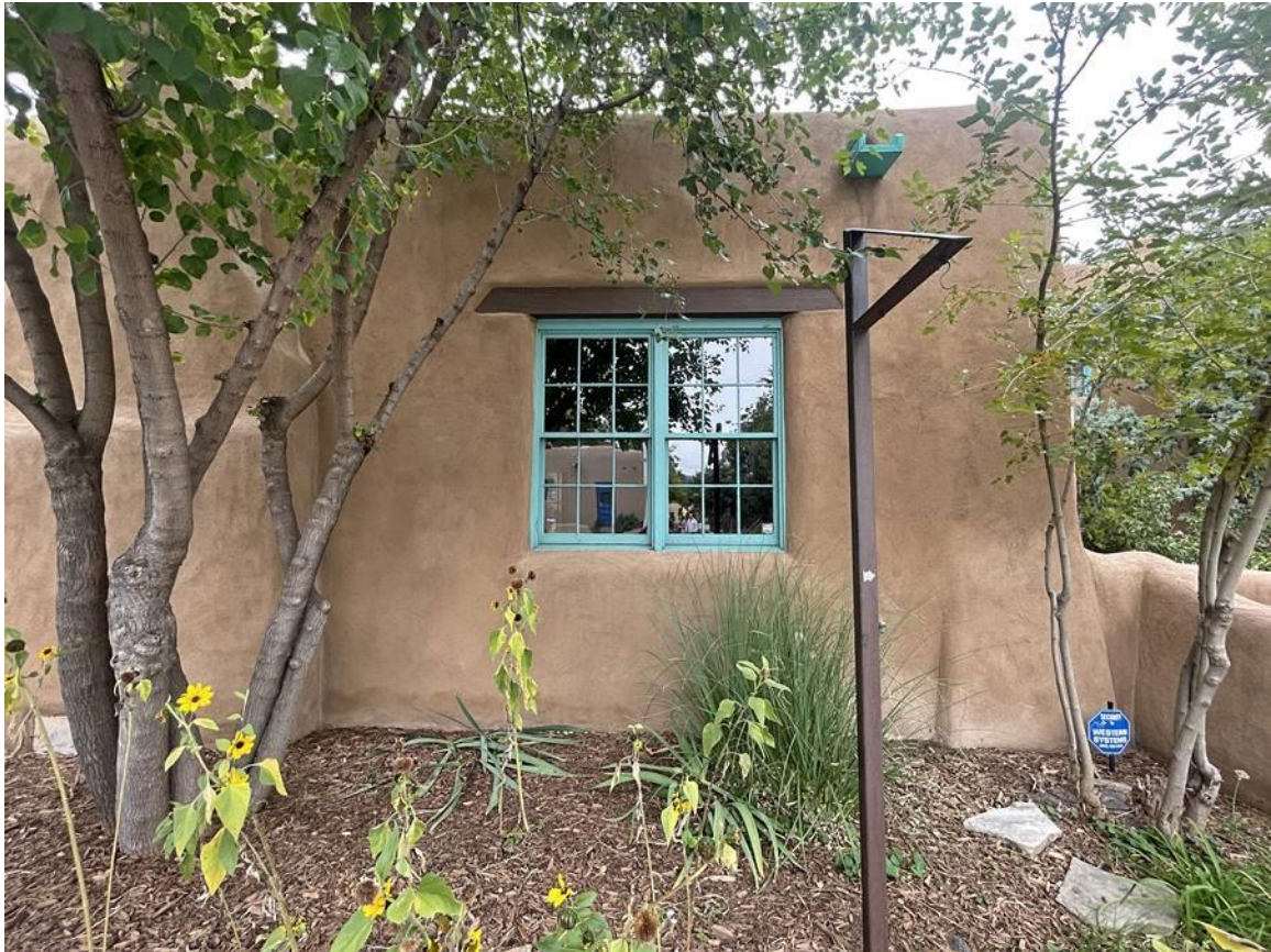
Photo 4: East elevation, one-story section. Camera facing west.
