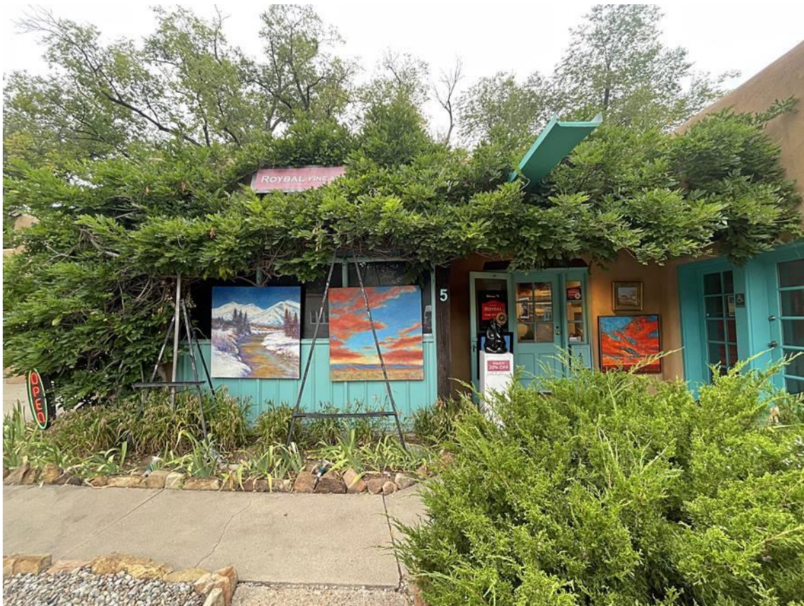
Photo 14: East elevation. Infilled portal. Camera facing west.
