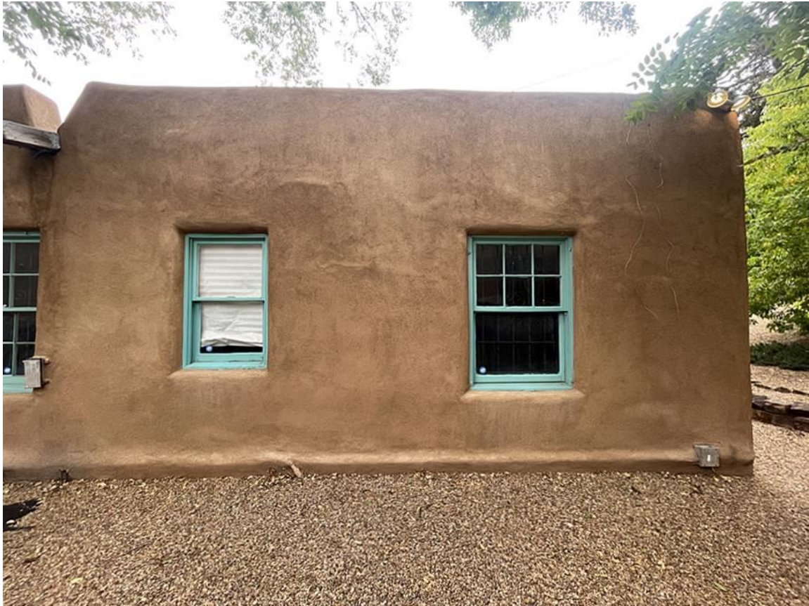
Photo 22: West elevation, south section. Camera facing east.
