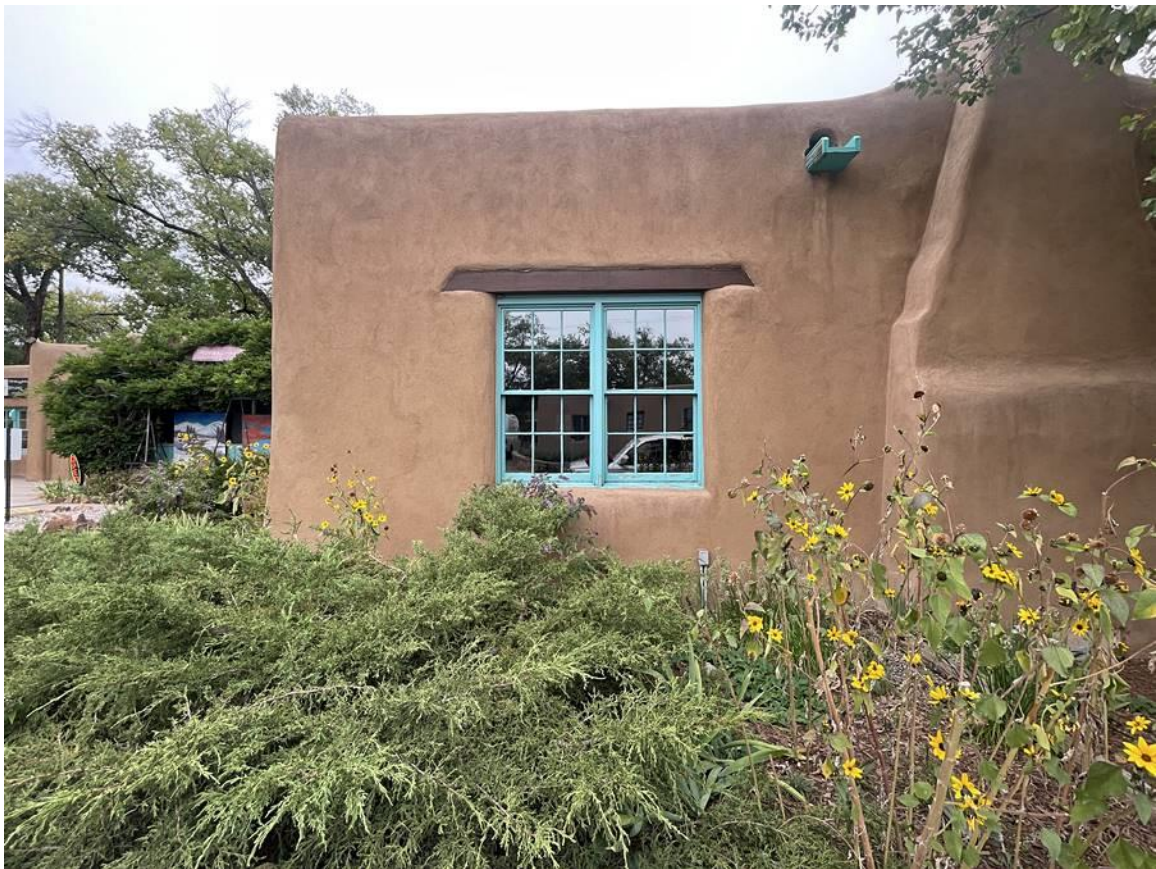
Photo 3: East elevation, one-story section. Camera facing southwest.
