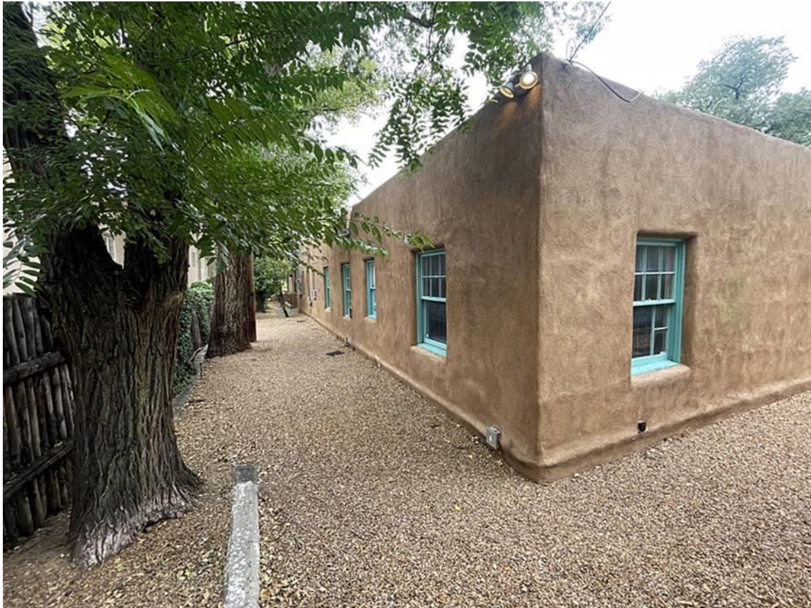
Photo 23 West elevation oblique. Camera facing northeast.
