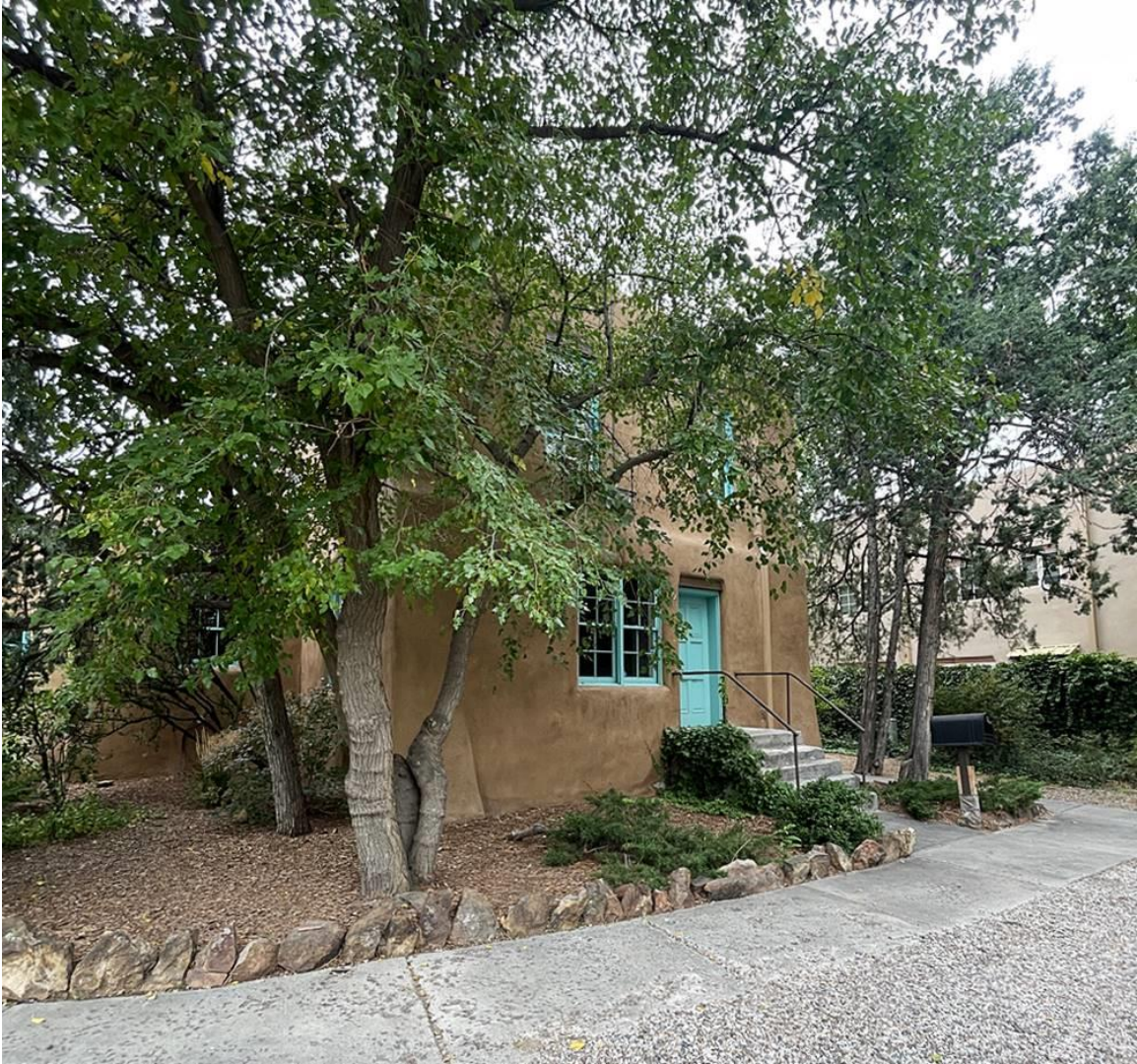
Photo 7: East and north elevations. Camera facing southwest.
