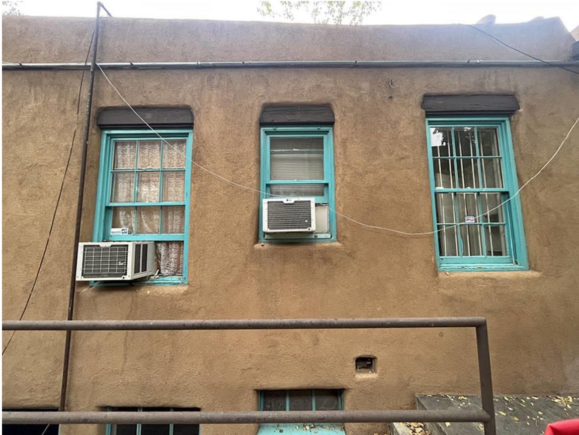
Photo 15: West elevation. Basement apartment below. Camera facing east.
