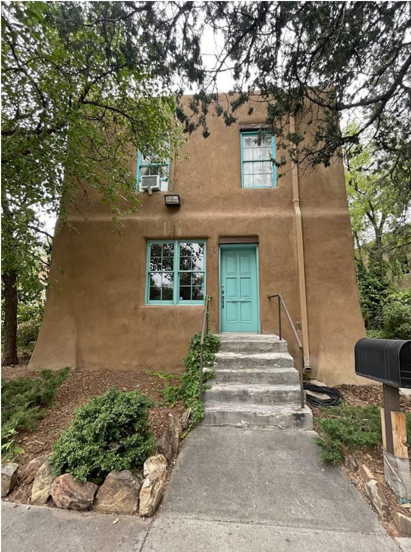
Photo 8: North elevation. Camera facing south.
