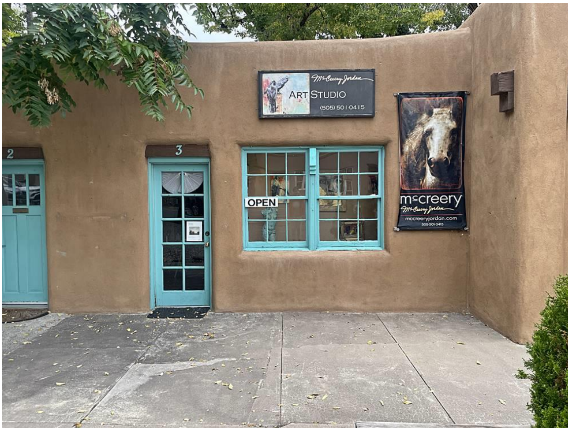
Photo 16: East elevation, north section. Camera facing west.
