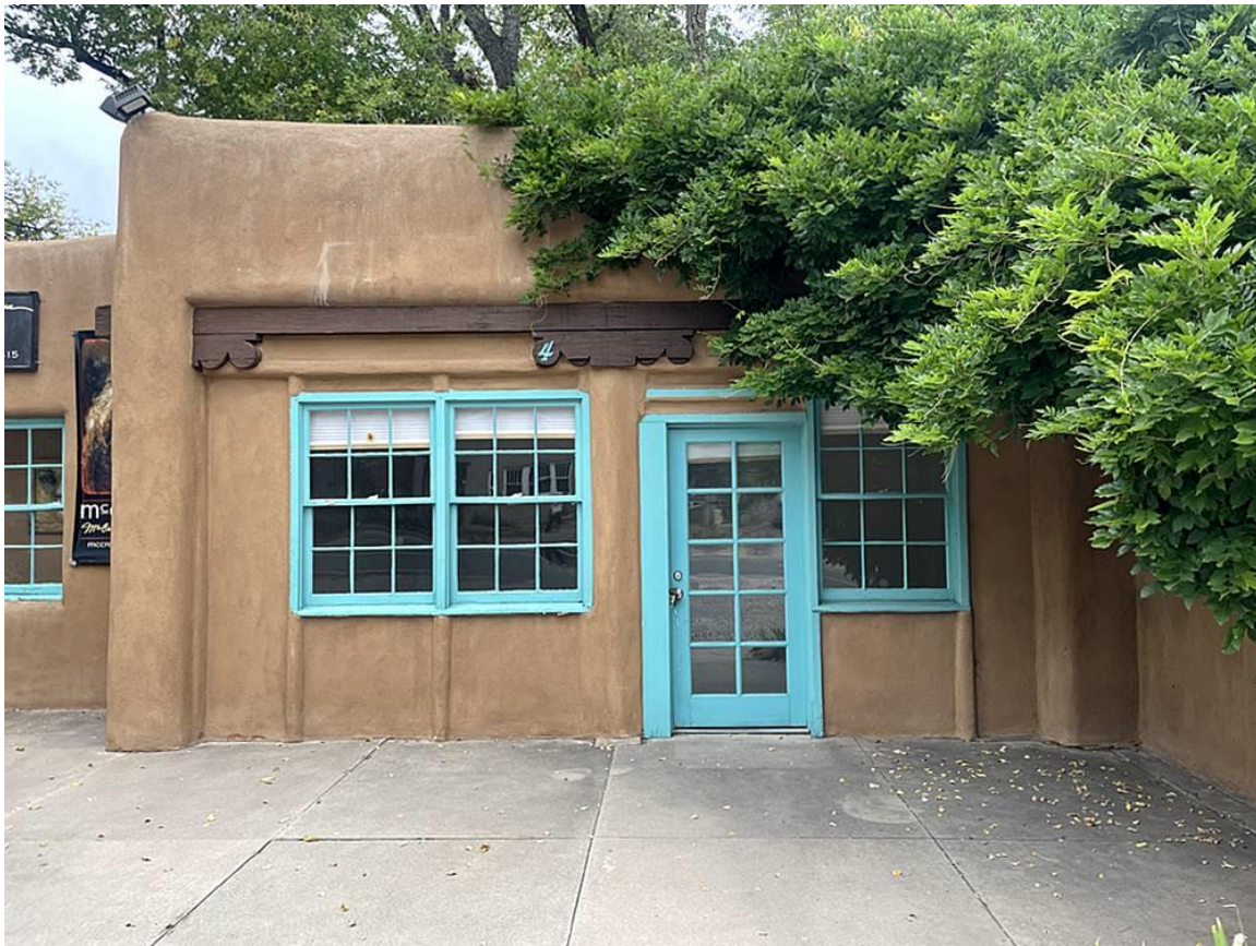
Photo 13: East elevation. Infilled garage. Camera facing west.
