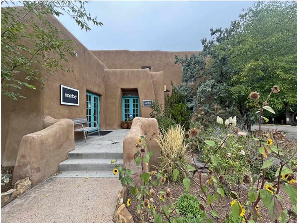
Photo 5: East elevation. Entry. Camera facing west.
