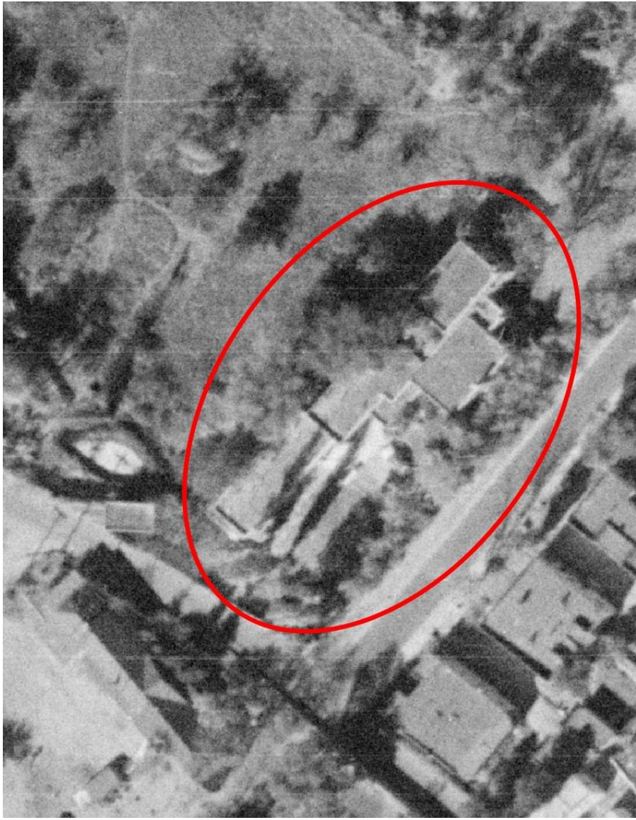
Figure 9: November 10, 1958, aerial photograph.
