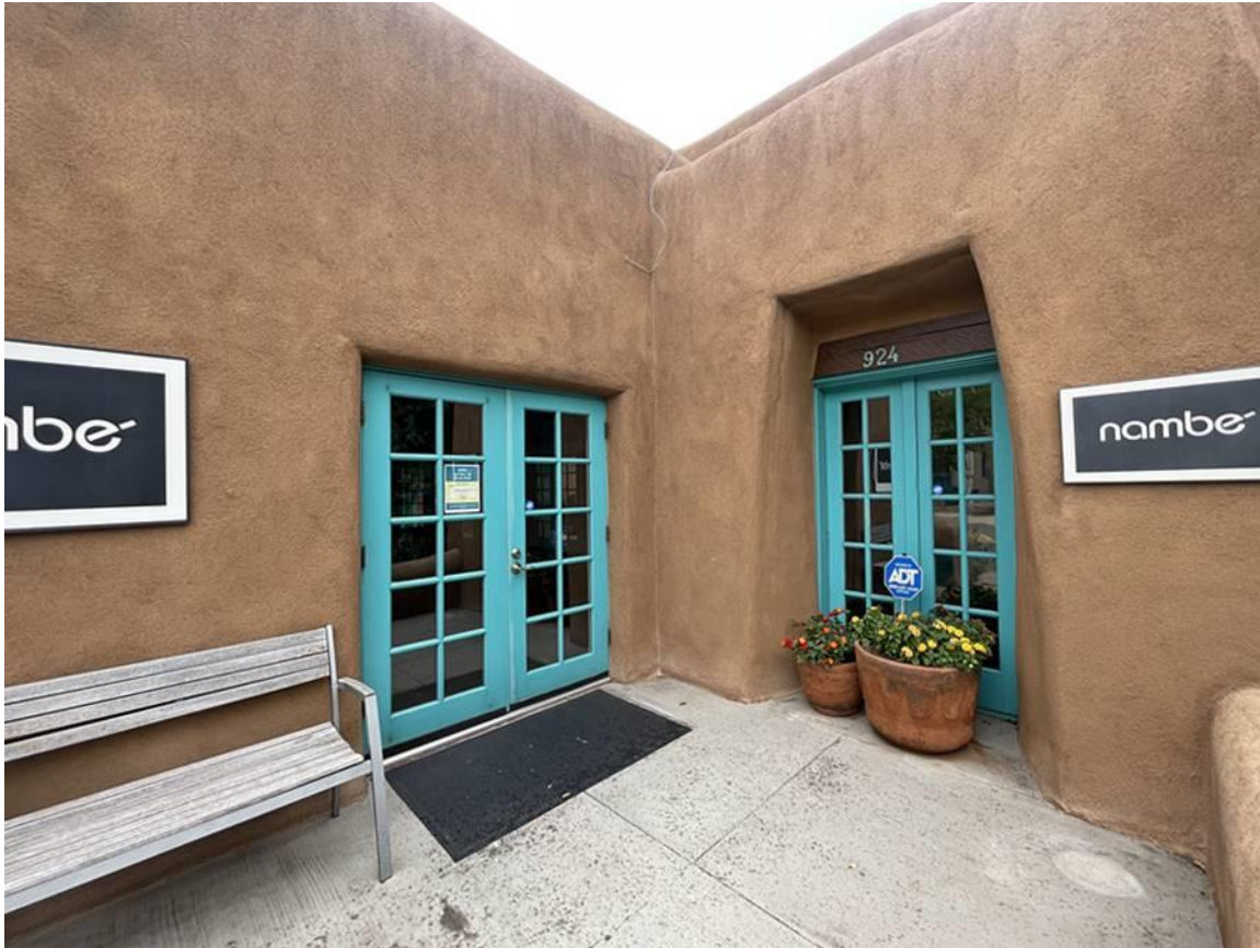
Photo 6: East elevation. Entry. Camera facing southwest.
