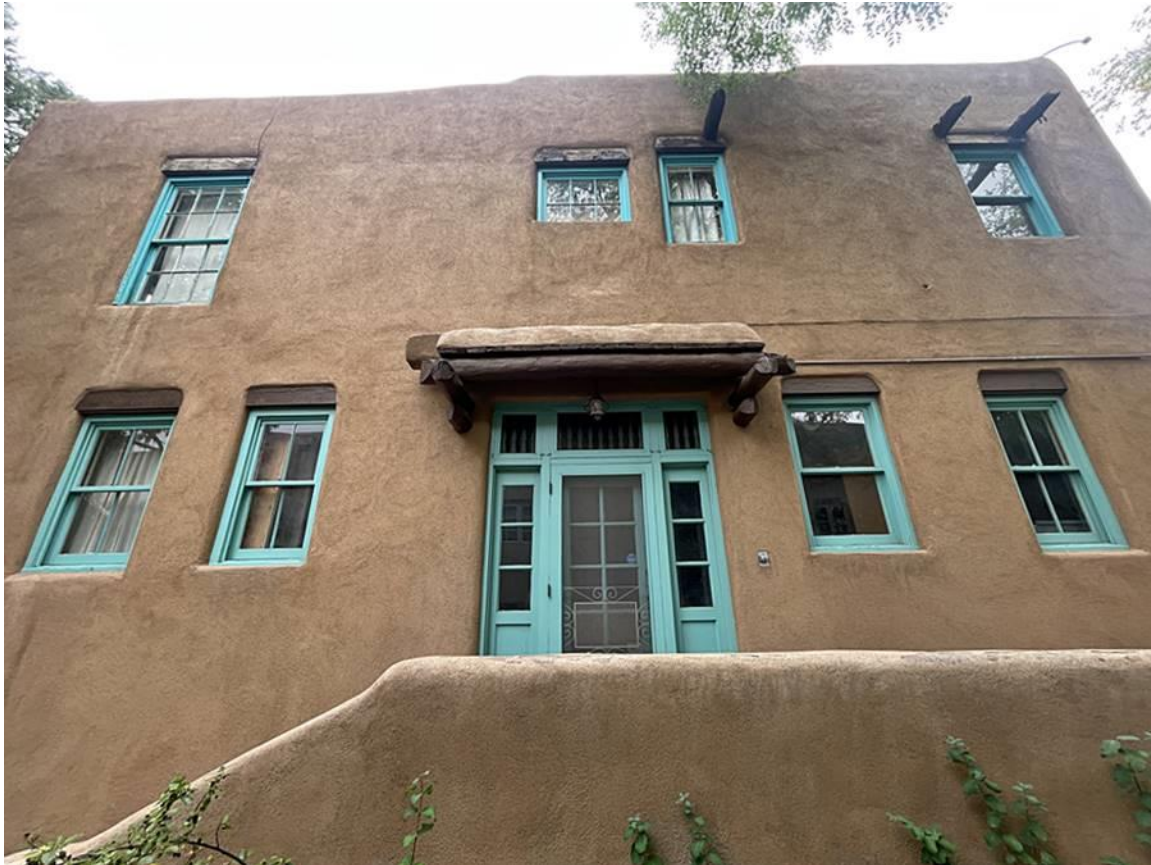
Photo 9: West elevation. Camera facing up.
