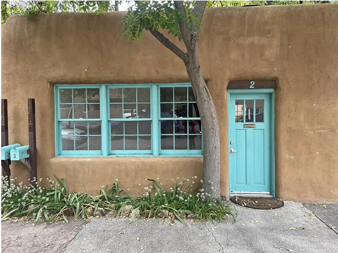
Photo 17: East elevation, middle section. Camera facing west.
