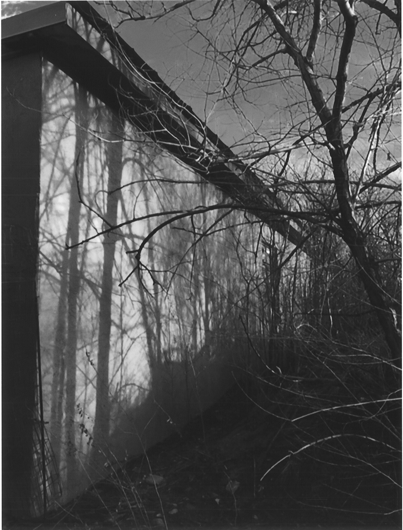
West side of garage
