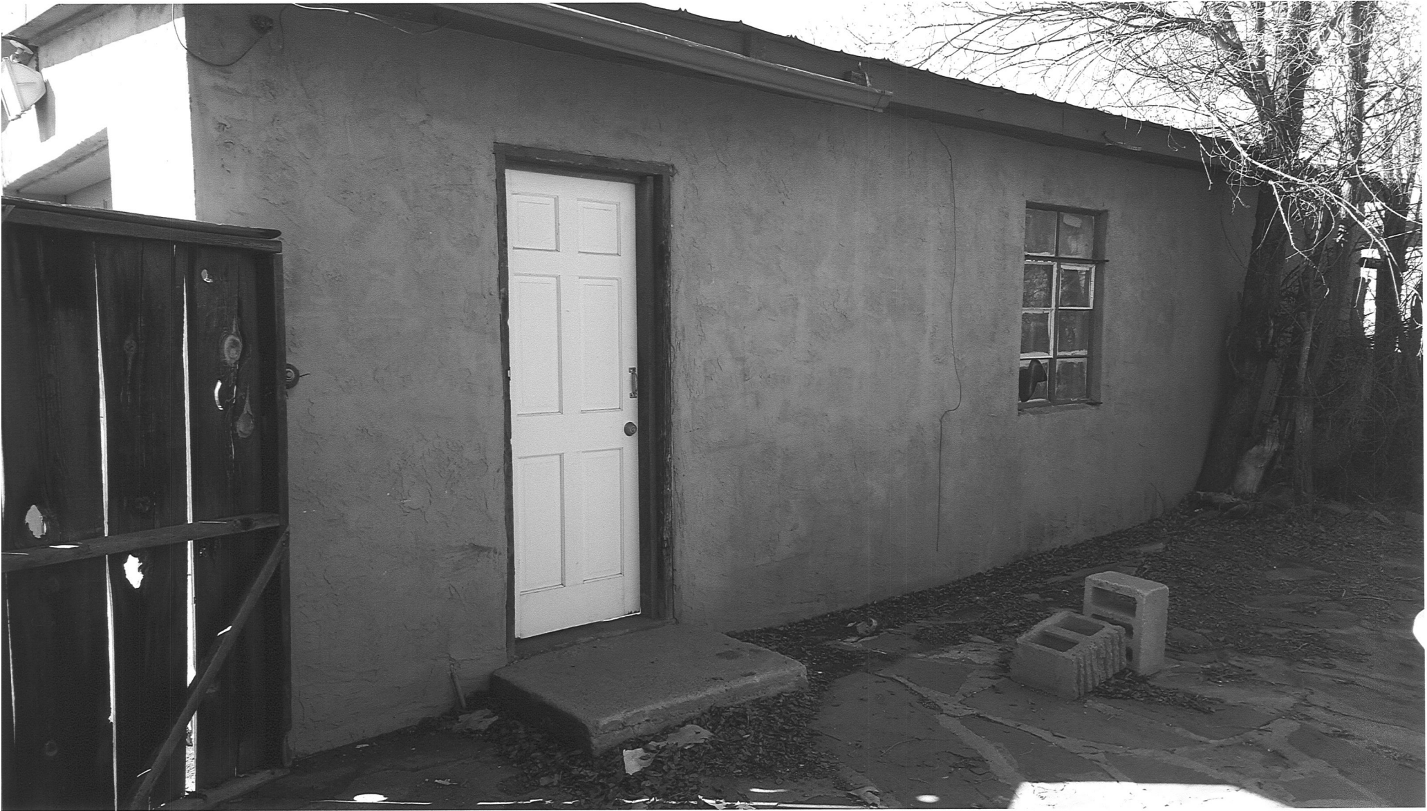
East side of garage
