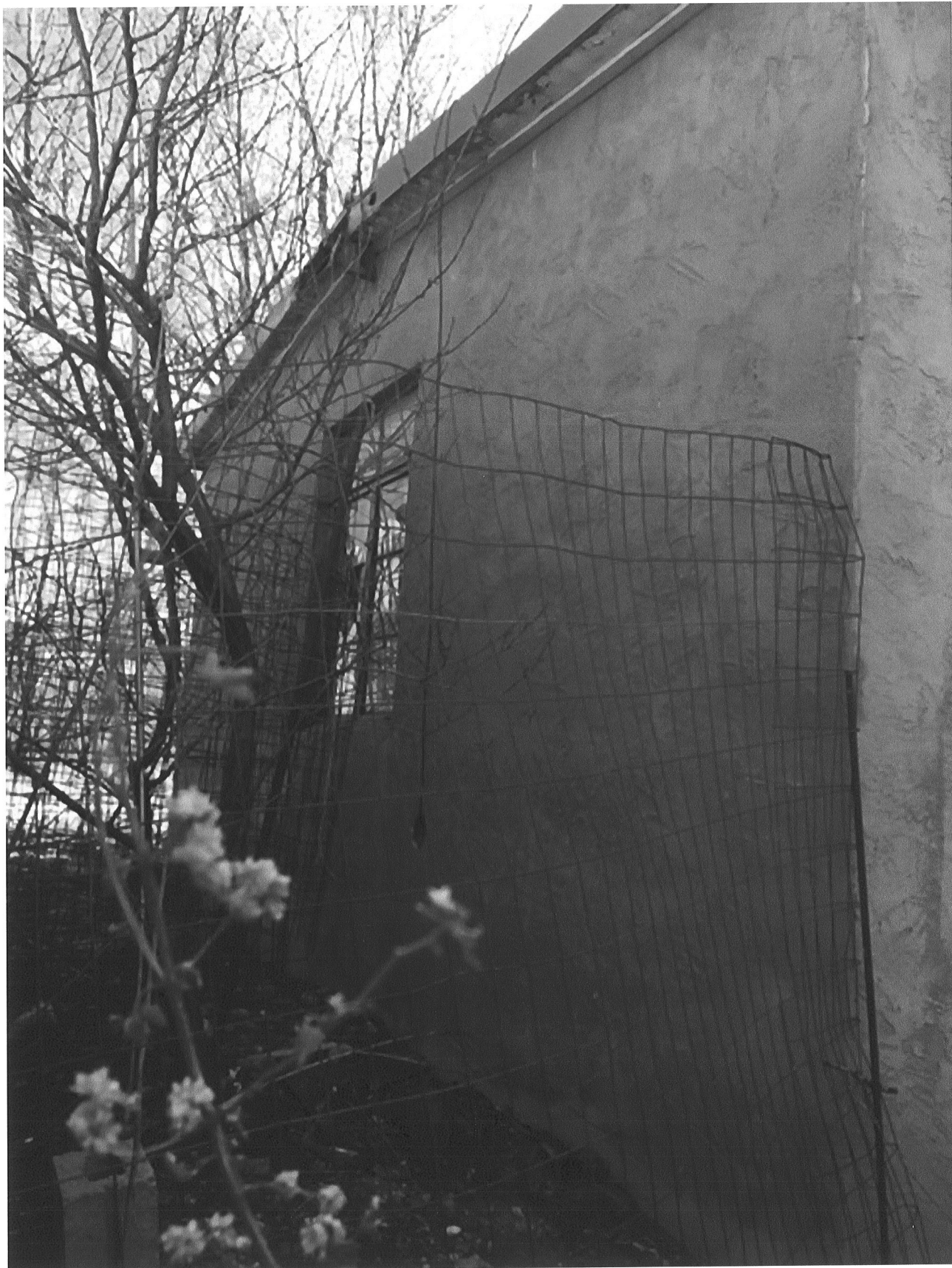
North side of garage
