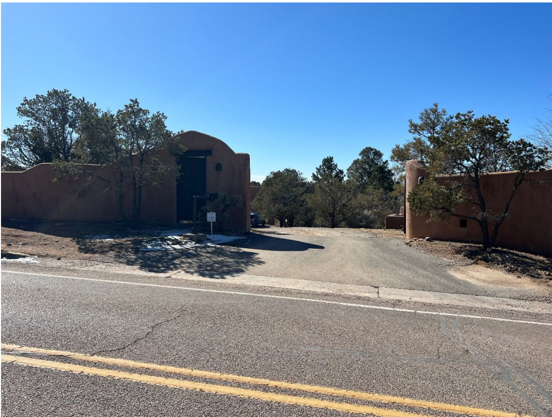
Looking West Across Garcia St. – SAR Delivery Vehicle Entrance
