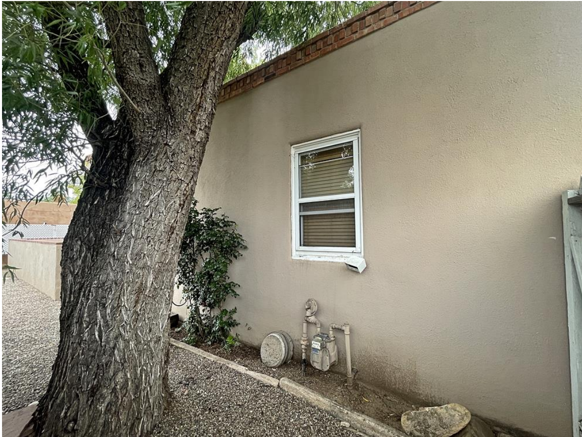
Photo 10: West elevation. Camera facing northeast.
