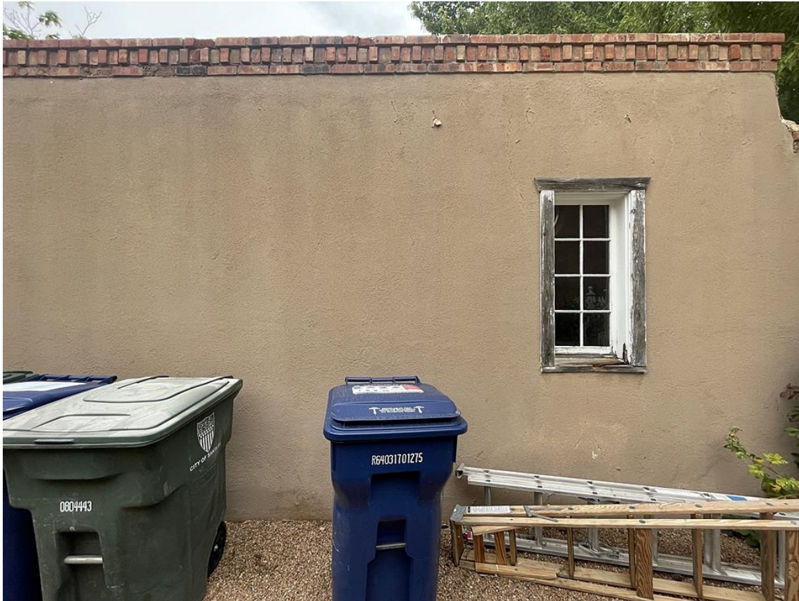
Photo 6: West elevation. Camera facing northwest.
