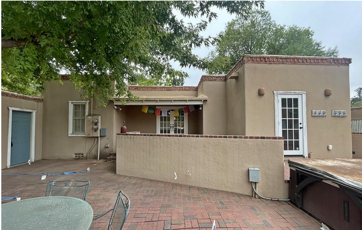
Photo 8: North (rear) elevation, center and west sections. Camera facing southwest.
