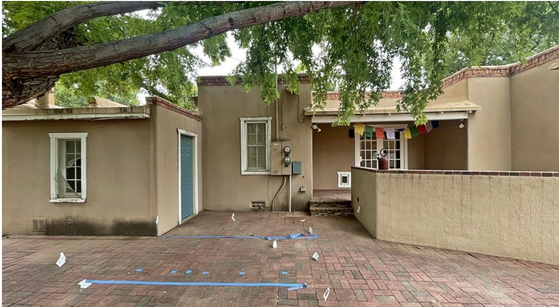
Photo 7: North (rear) elevation, east and center sections. Camera facing southwest.
