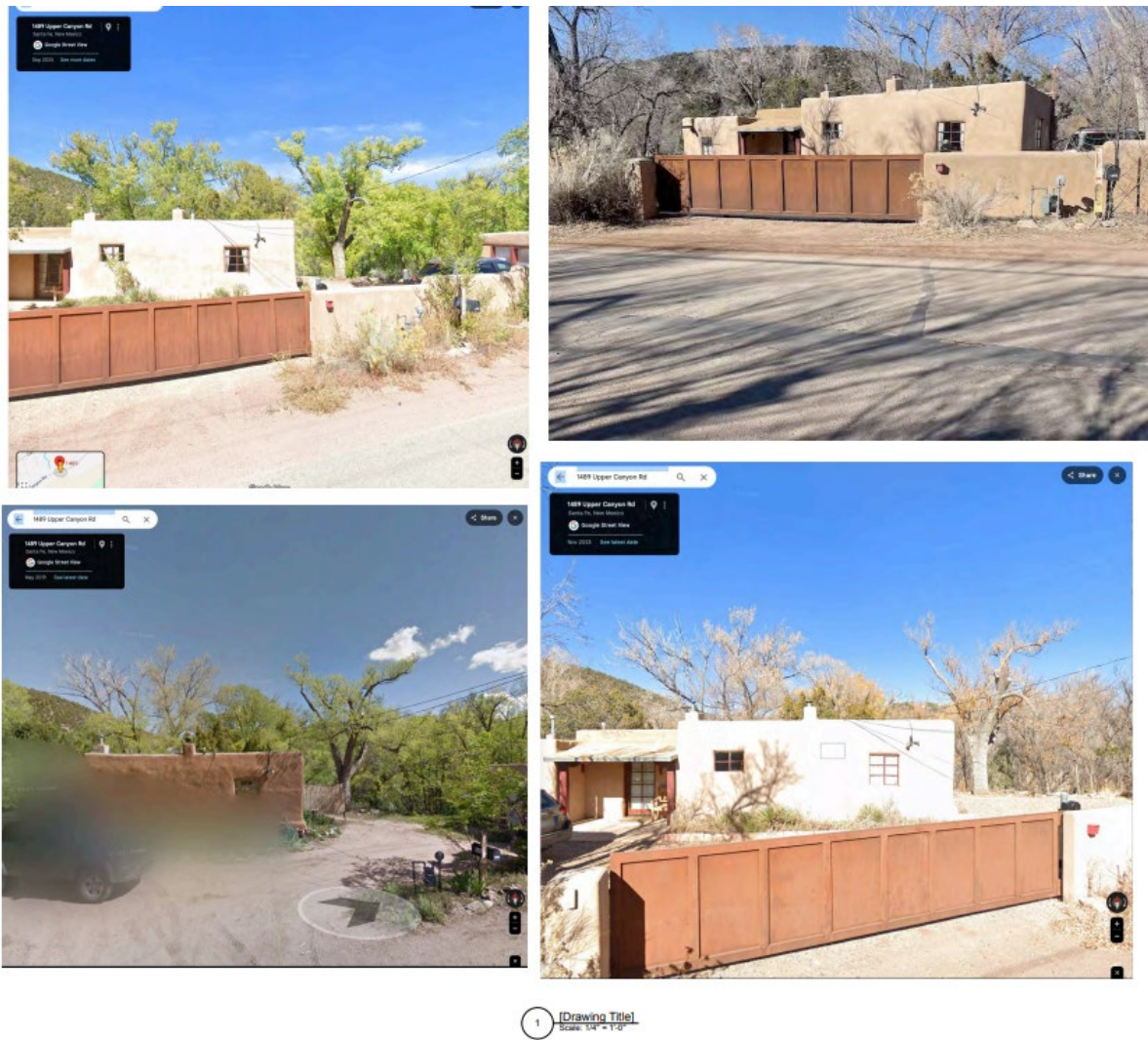
Figure 7. Overview of 1489 Canyon Road.
