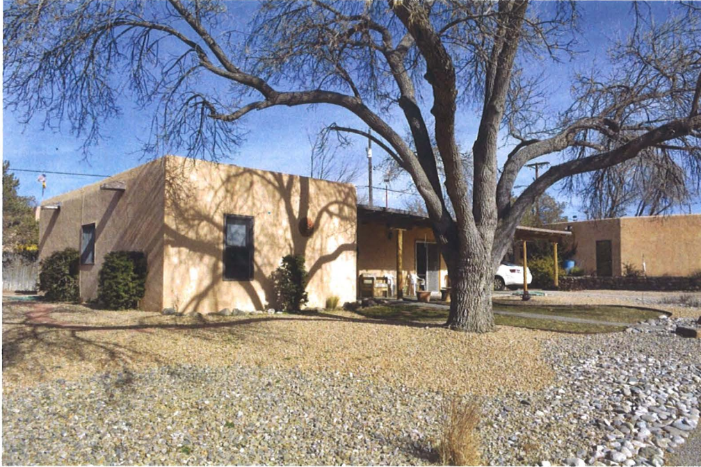
Photo 2: Street and west elevations, facing northeast.
