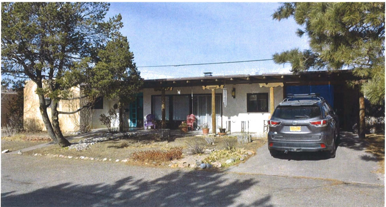
Photo 1: Street and east elevations, facing northwest.
