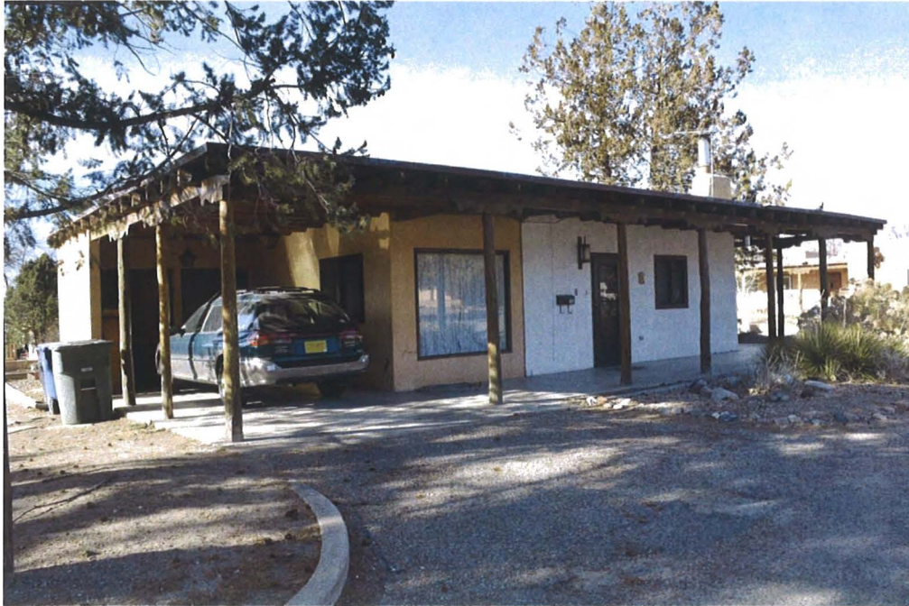
Photo 2: South and east elevations, facing northwest.
