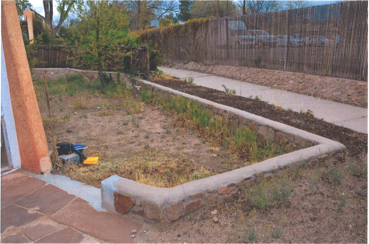
Figure 2: 124 Camino Santiago, rear retaining wall, May 3, 2018.
