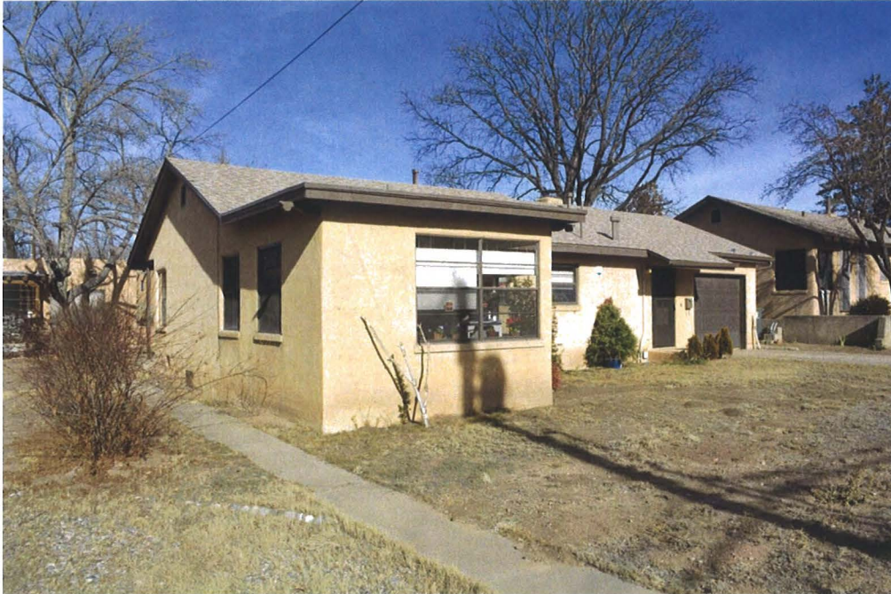
Photo 2: Street and west elevations, facing northeast.
