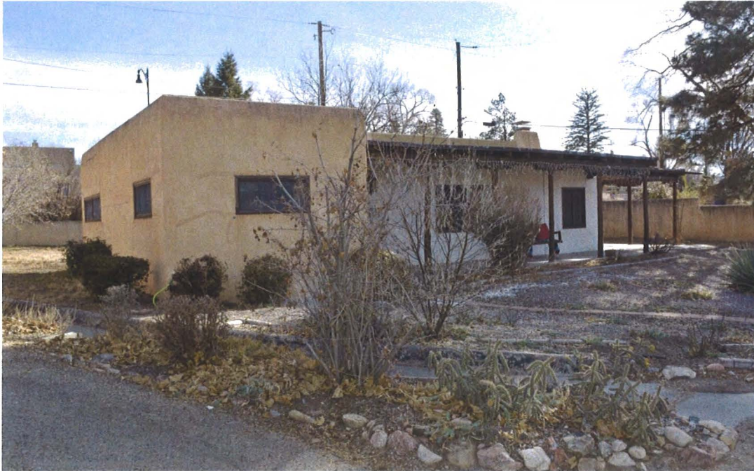
Photo 2: Street and north elevations, facing southeast.
