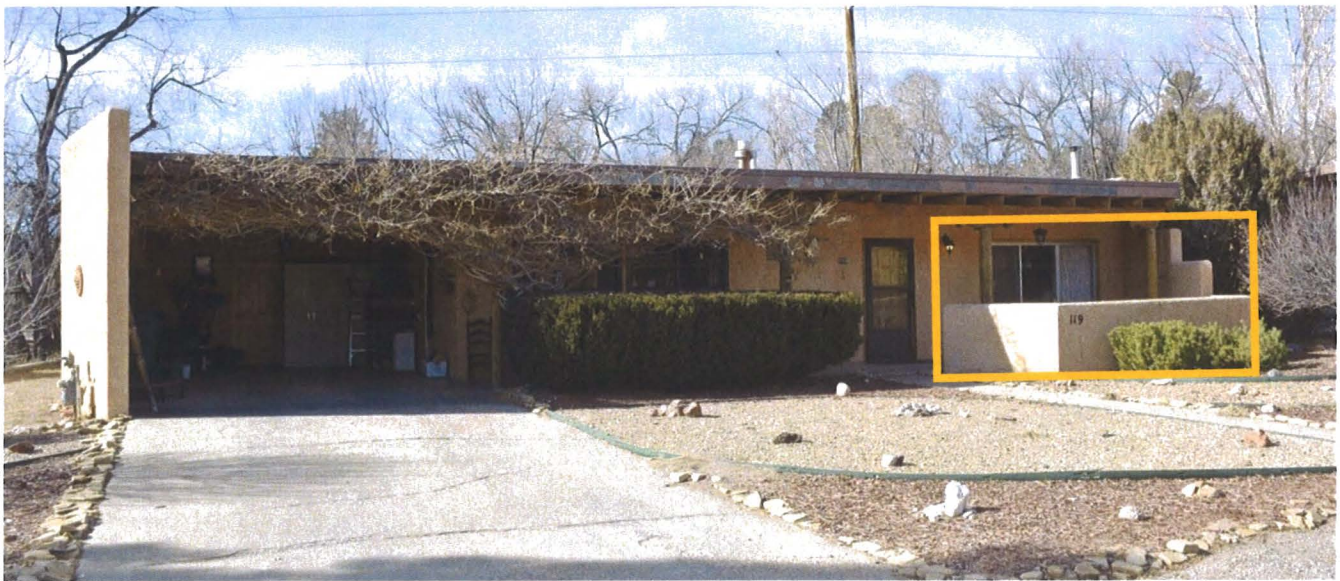
Photo 1: Street and south elevations, facing northwest. Box indicates removed portion of angled patio wall.
