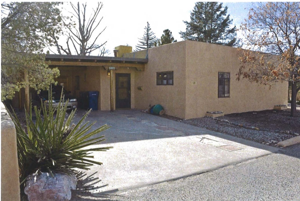
Photo 1: Street and east elevations, facing southwest.
