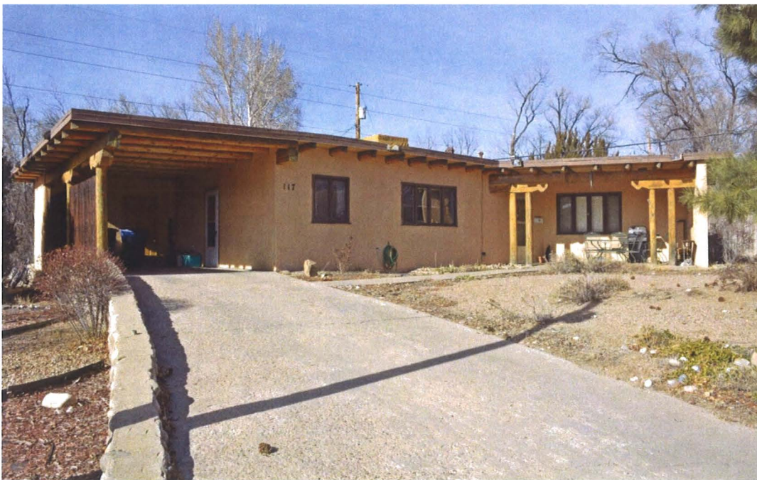
Photo 1: Street, west and south elevations, facing northeast.
