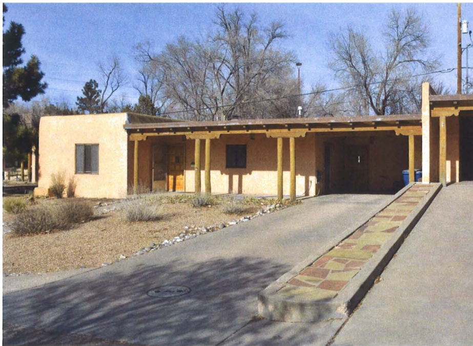
Photo 1: Street and east elevations, facing northwest.
