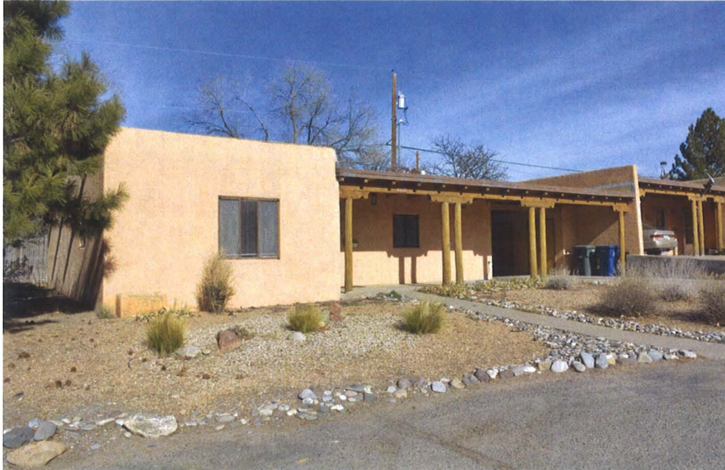
Photo 2: Street and west elevations, facing northeast.
