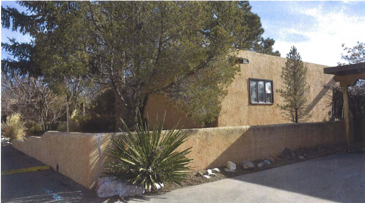
Photo 2: West elevation, facing southeast.
