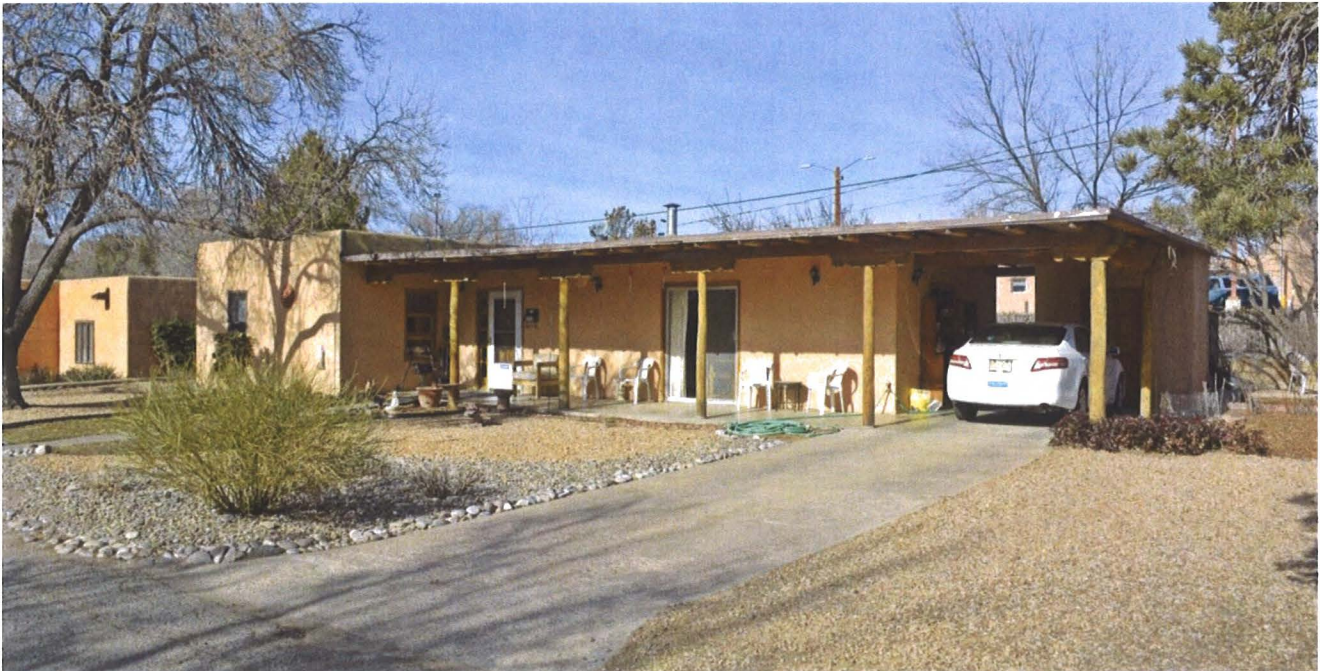
Photo 1: Street and east elevations, facing northwest.
