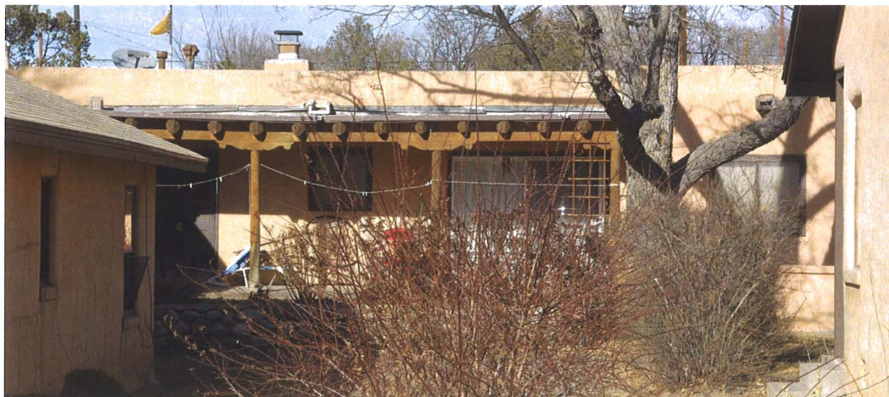
Photo 4: South elevation, facing north.
