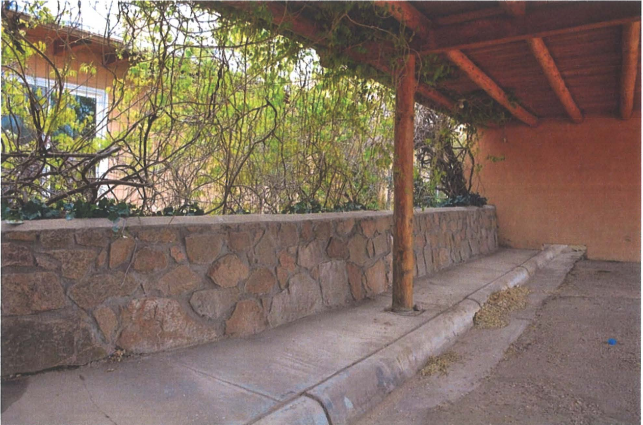
Figure 1: 126 A Camino Santiago, Garage/Carport Structure, retaining wall, May 3, 2018.
