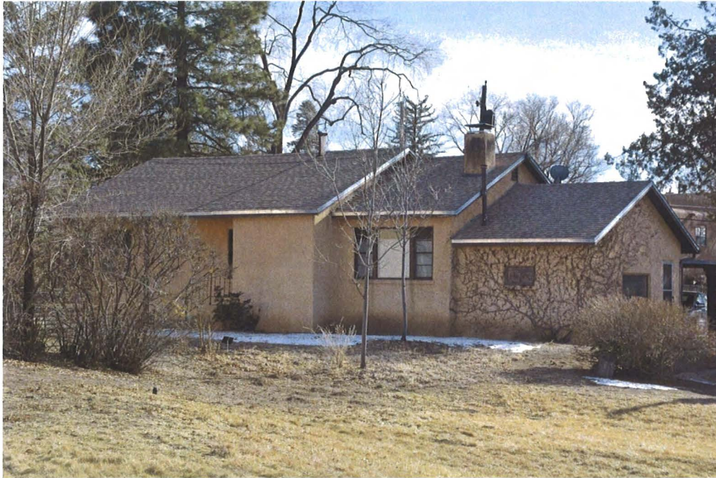
Photo 3: North elevation, facing southeast.
