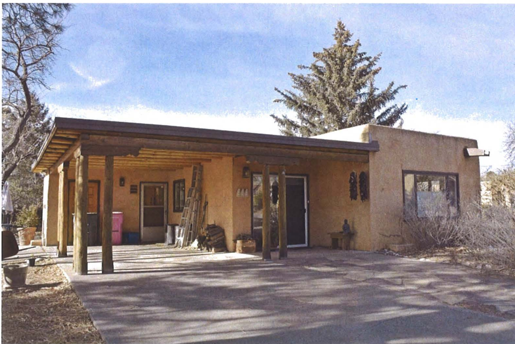
Photo 1: East and south elevations, facing northeast.
