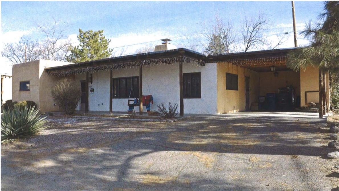
Photo 1: Street and south elevations, facing southeast.
