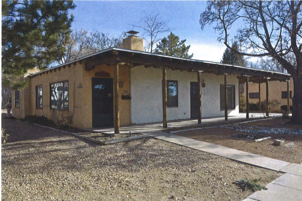
Photo 2: North and street elevations, facing southeast.
