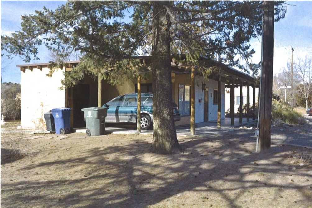
Photo 1: South and east elevations, facing northwest.
