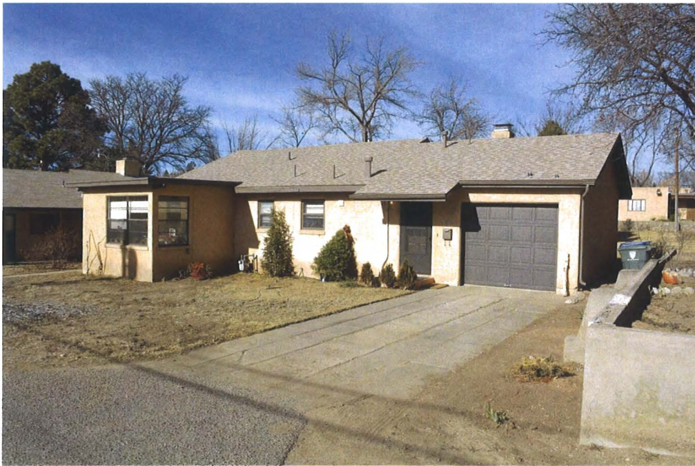
Photo 1: Street and east elevations, facing northwest.
