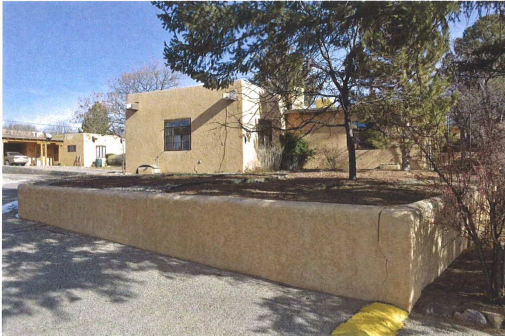
Photo 3: West and south elevations, facing northeast.
