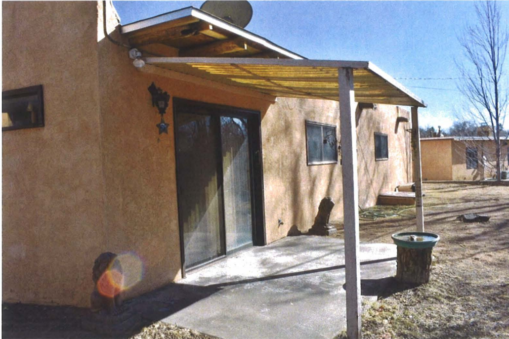
Photo 2: West elevation, facing south (Sharon Joyce, February 23, 2018).
