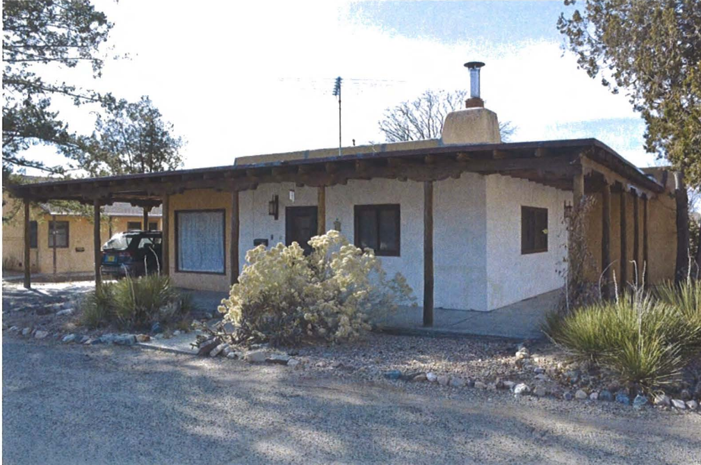
Photo 3: Street and west elevations, facing southeast.
