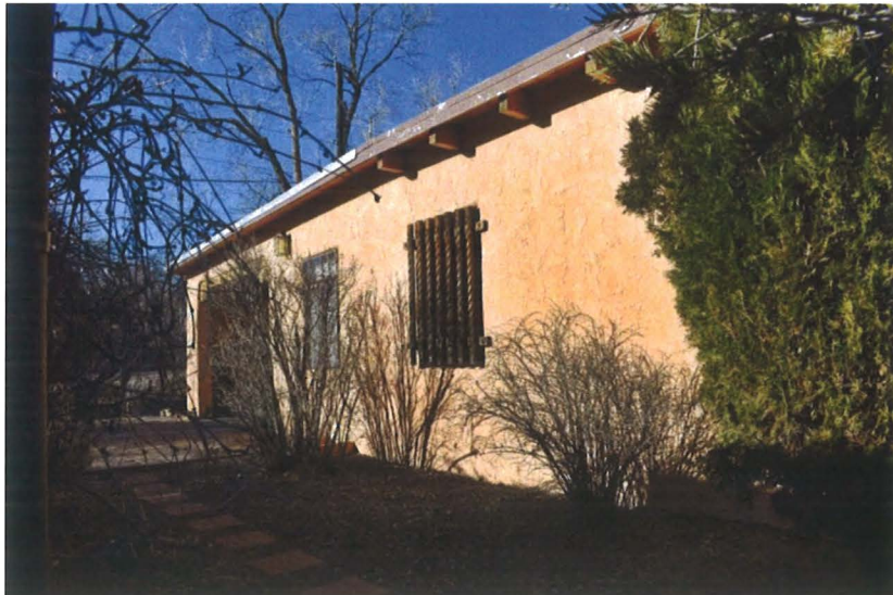
Photo 1: South elevation, facing northeast and northwest (Sharon Joyce, February 23, 2018).
