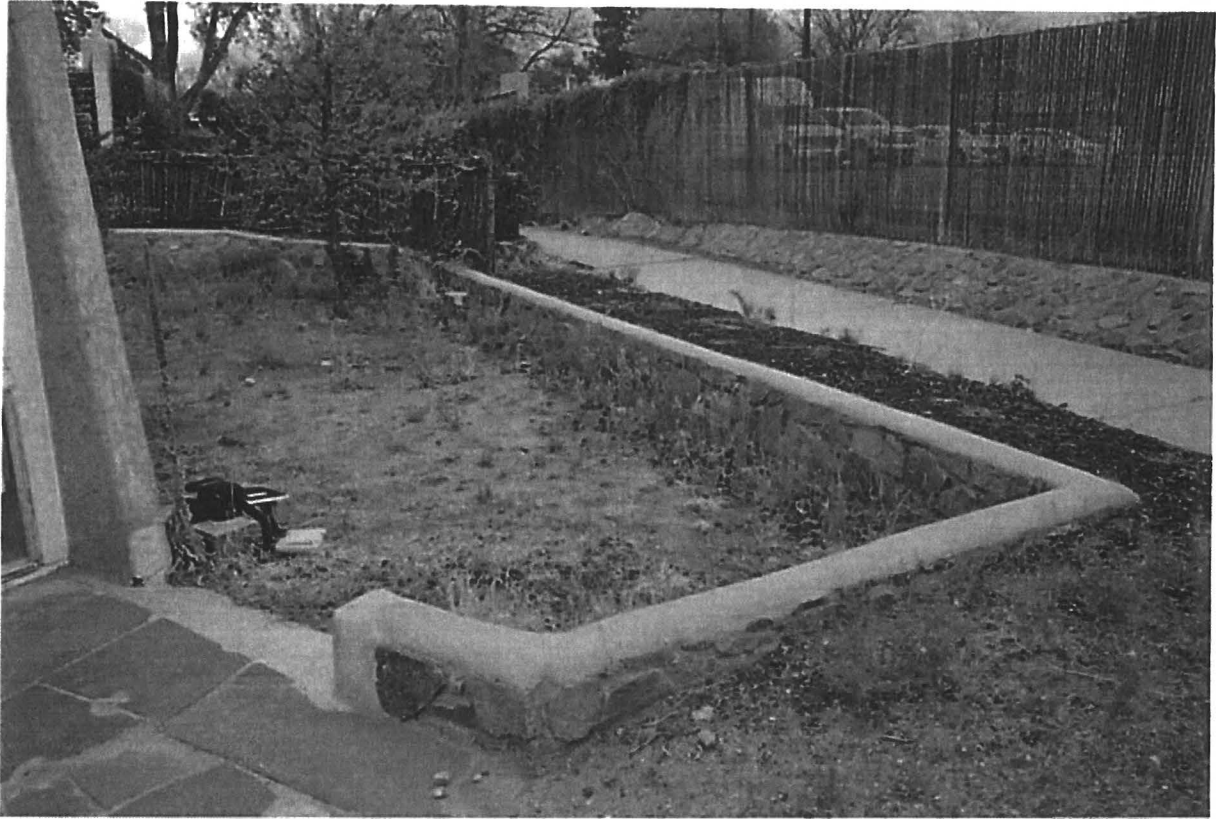
Figure 2: 124 Camino Santiago, rear retaining wall, May 3, 2018.
