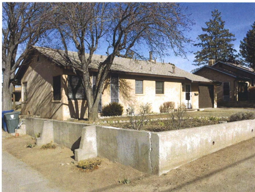
Photo 2: Street west elevations, facing northeast.
