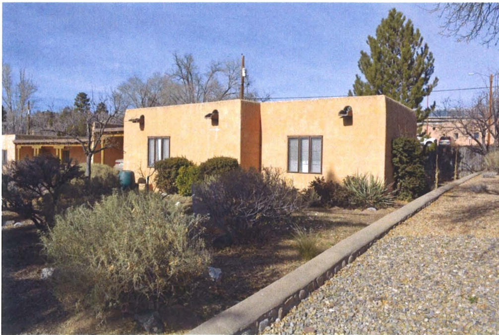
Photo 1: Street and east elevations, facing northwest.
