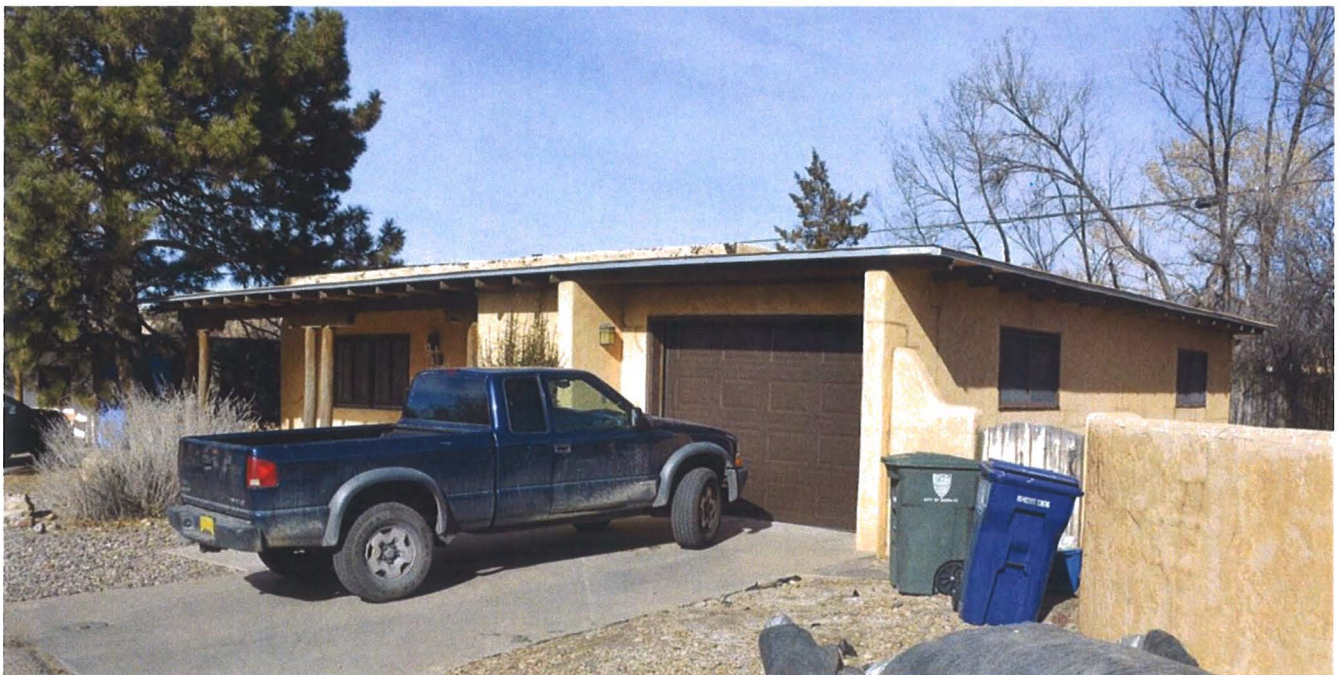
Photo 1: Street elevation and north elevations, facing northwest.
