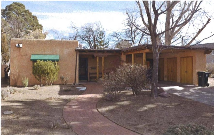
Figure 12: 120 Camino Santiago, constructed in c. 1971.
