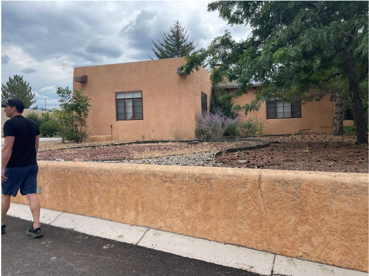
118 Camino Santiago (west side of house, looking east)
