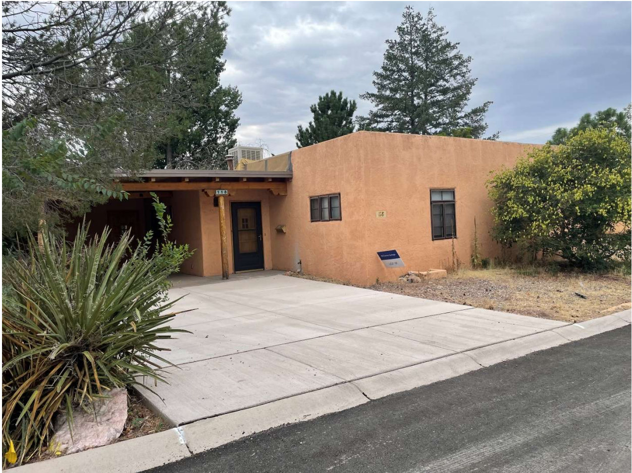
118 Camino Santiago (Front of house - north side, looking southwest)
