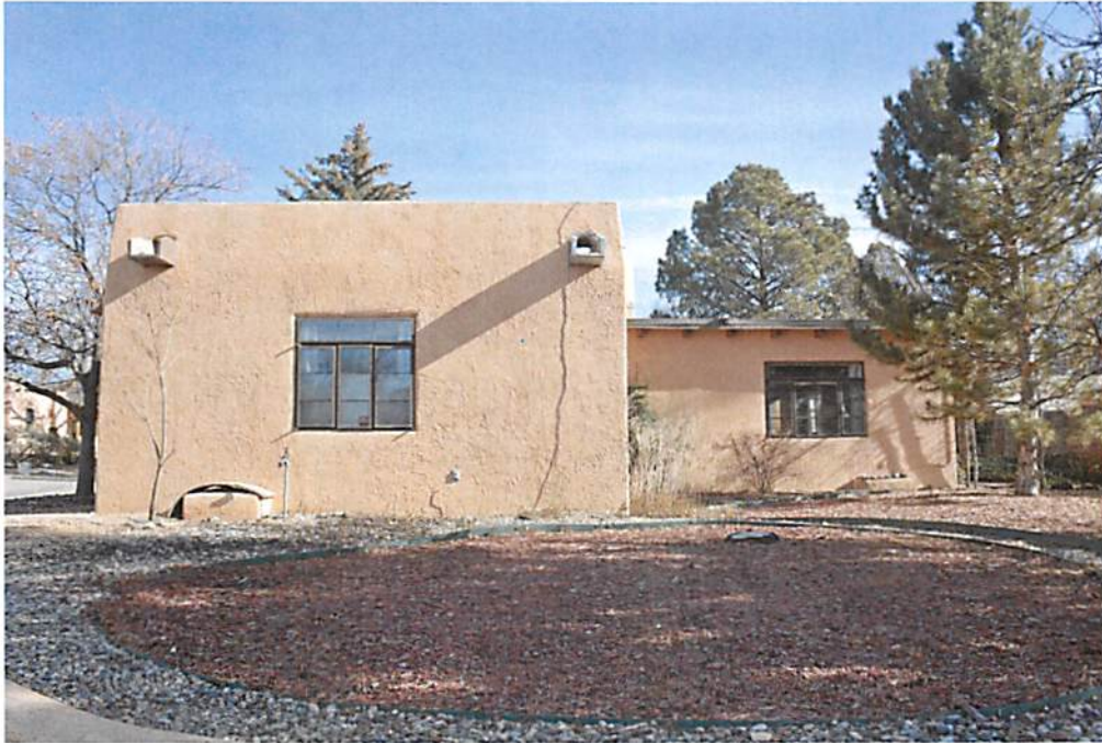
Photo 2: West elevation, facing east.
