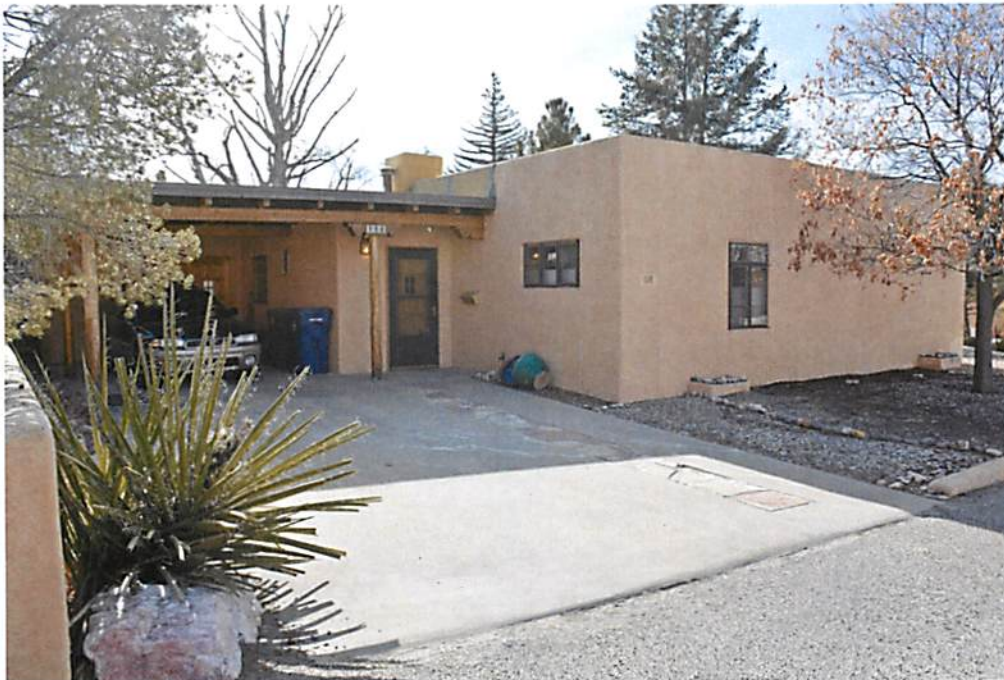
Photo 1: Street and east elevations, facing southwest.
