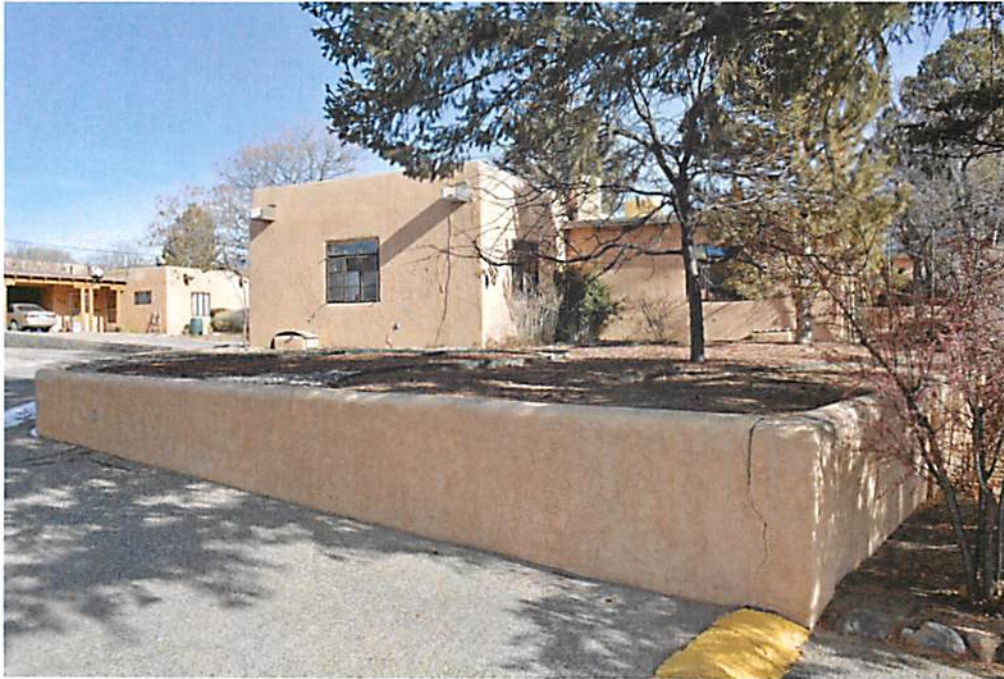
Photo 3: West and south elevations, facing northeast.
