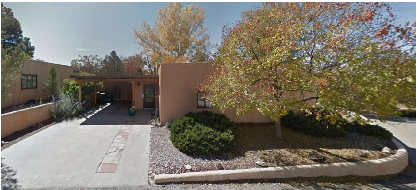
Figure 2: Subject Property North Street Facing Elevation
