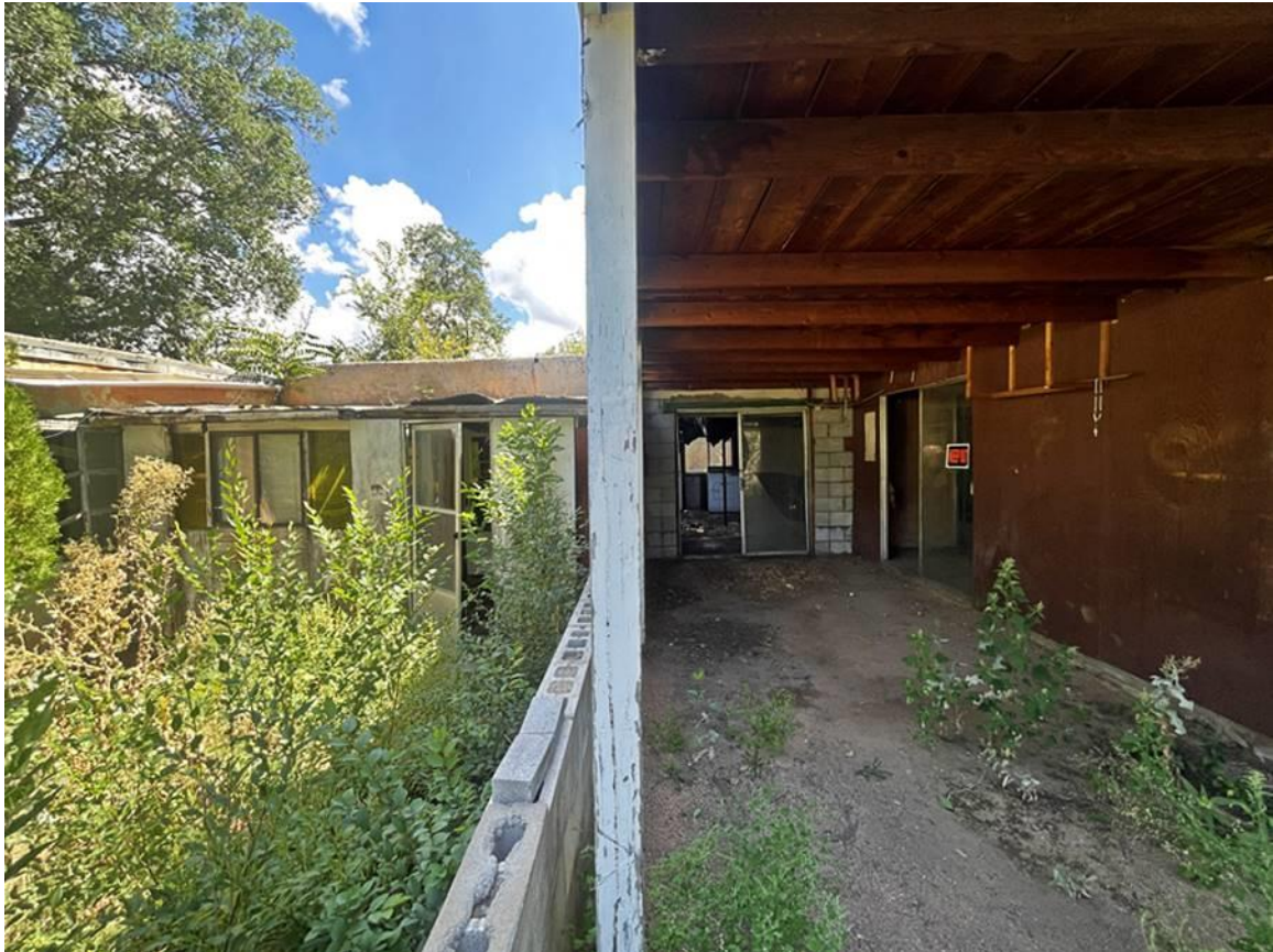
Photo 8: West elevation. Addition and carport structure. Camera facing east.
