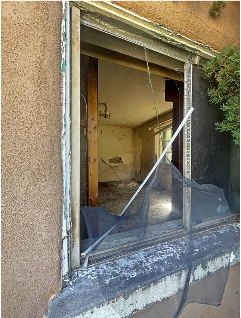
Photo 5: West elevation. Condition of windows. Camera facing southeast.
