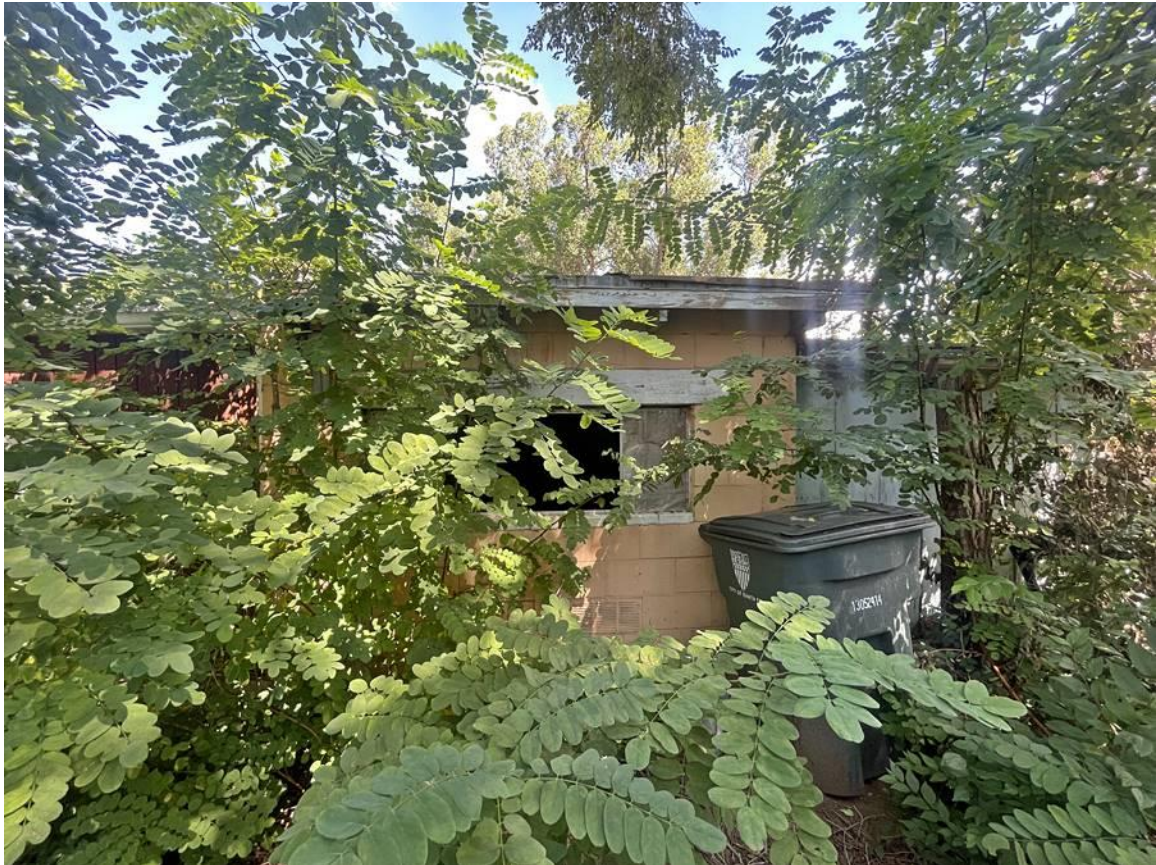
Photo 12: South elevation. CMU storage area. Camera facing northeast.
