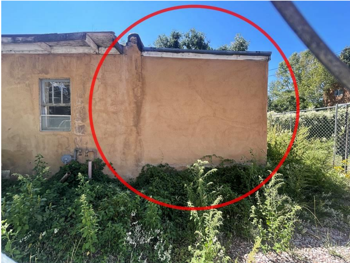
Photo 3: North elevation. Enclosed porch or patio area circled. Camera facing south.
