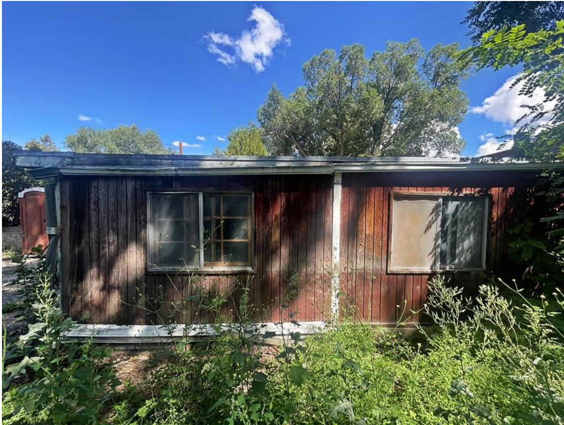
Photo 11: South elevation. Workshop. Camera facing north.
