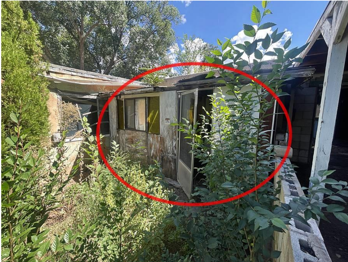
Photo 6: West elevation. 1960s addition. Plywood porch enclosure circled. Camera facing northeast.
