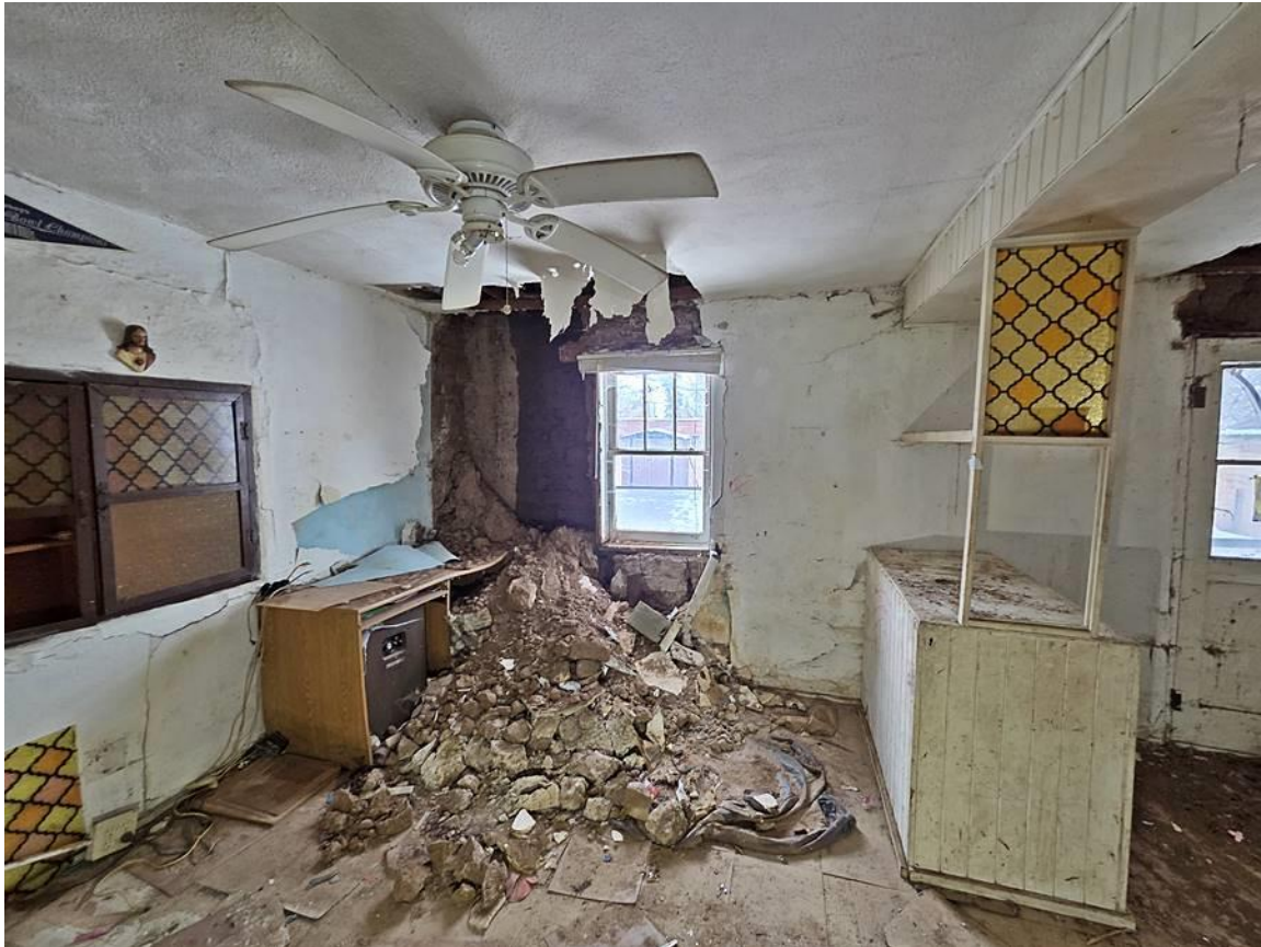
Photo 14: Interior. Room at northwest corner of older building. March 9, 2025, John Padilla.
