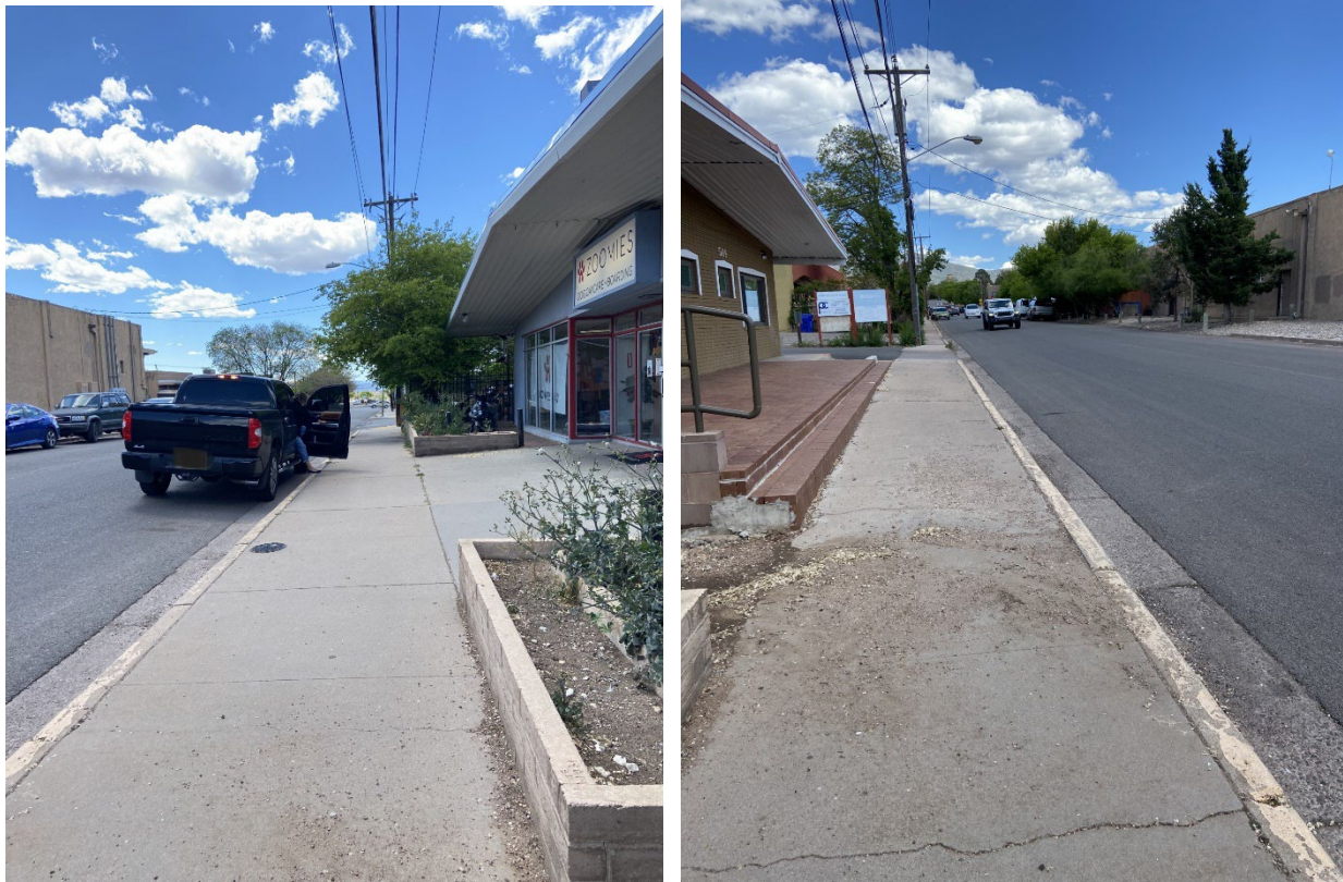
Figure 1. Improper Parking Pickup & Fire Lane
