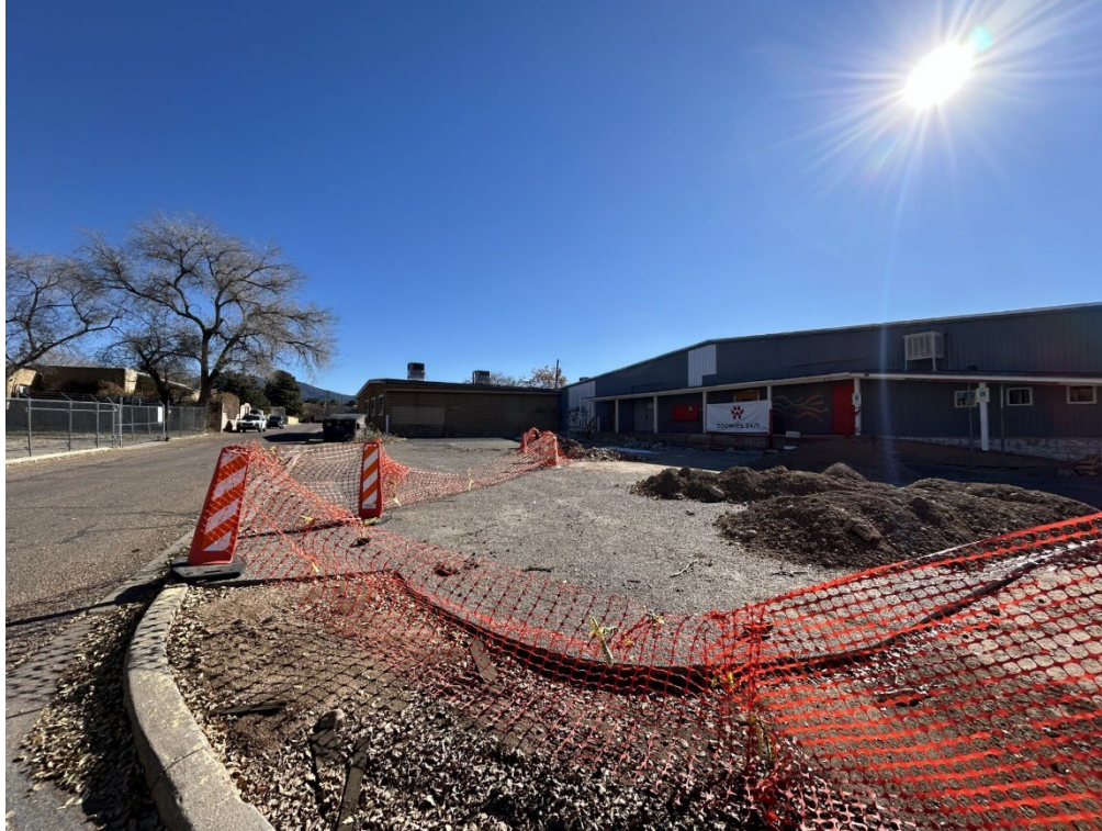
Figure 3: Rear Parking Lot Infrastructure (December 5, 2024)
