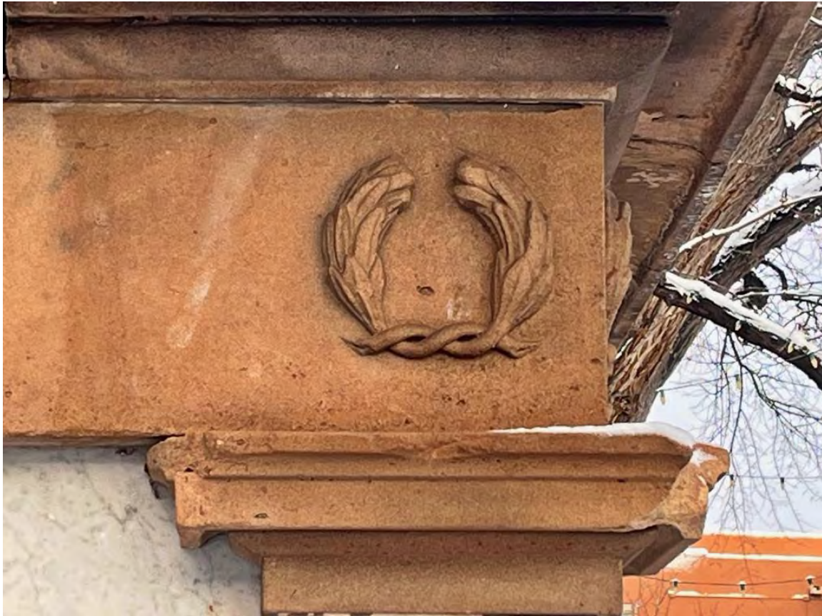
Photo 10: East elevation. Wreath motif. Camera facing east. March 7, 2025.
