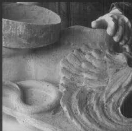
Figure 20. (top) After cast stone from the field is cast, a new surface texture is used to replicate the original surface texture. (middle) Cast stone units and joints on a new window pediment. (bottom) Cast stone units on the surface of a new window pediment. The surface of the casting is filled with a mortar similar to the concrete mix used to cast the element.
