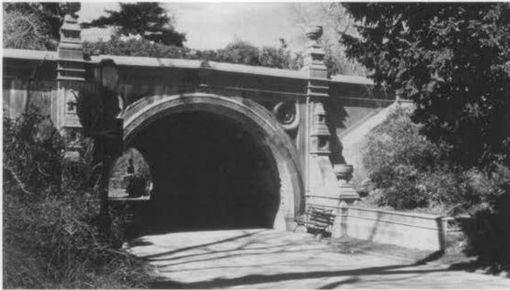
Figure 5. Constructed in 1868 of Beton Coignet, the Cleft Ridge Span in New York City's Prospect Park is one of the earliest extant cast stone structures in the United States.
