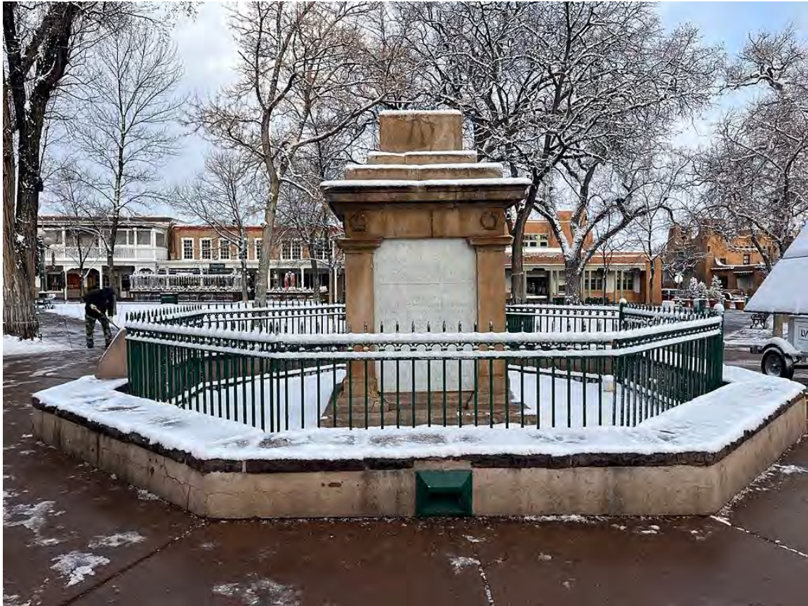
Photo 5: East elevation and picket fence. Camera facing west. March 7, 2025.
