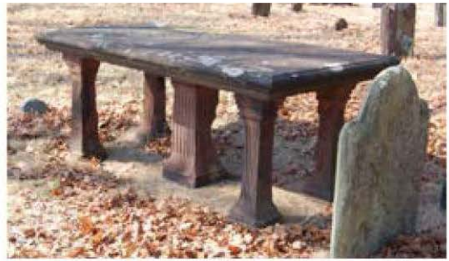
Figure 4. This sandstone table tomb, located in Cedar Grove Cemetery, New London, CT, is an engineered grave marker structure consisting of a horizontal stone tablet supported by four vertical table “legs” with a central column,. Photo: Jason Church.
