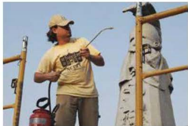
Figure 24. A severely deteriorating monument or grave marker can be treated with a stone consolidant. The treatment is usually applied using a spray system. The consolidant soaks into the stone and replaces mineral binders that hold the stone together. On-site and laboratory testing and evaluation are performed prior to using this non-reversible type of treatment. Photo: Lucas Flickinger.
