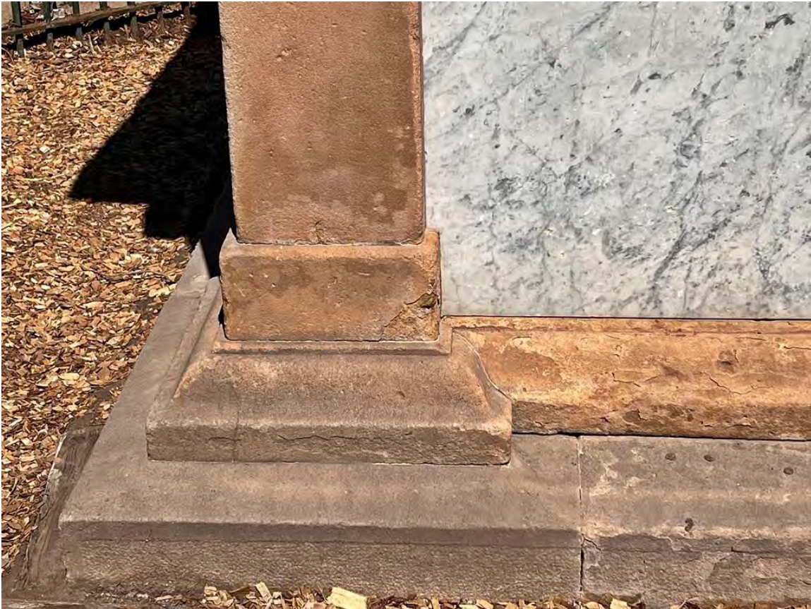
Photo 7: South elevation. Base. Camera facing down. March 16, 2025.
