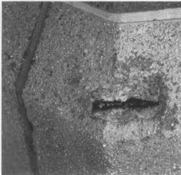
Figure 13. Rusting of reinforcement near the surface of the stone may result in spalling. Sections of reinforcement, such as this, may be cut out and the spall repaired with a matching composite mortar.
