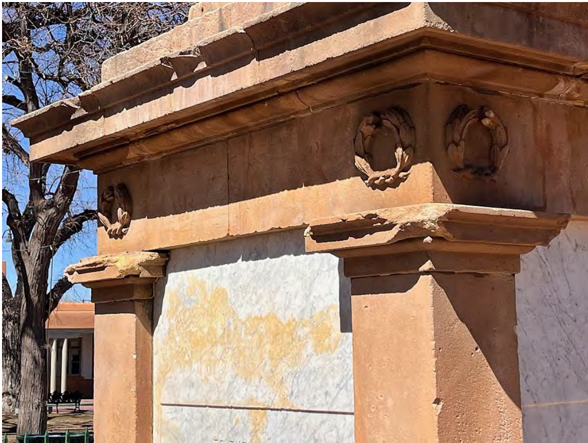
Photo 9: South elevation. Architrave. Camera facing northwest. March 16, 2025.
