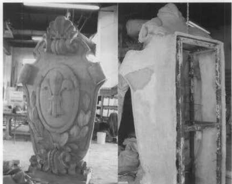
Figure 25. Glass Fiber Reinforced Concrete (GFRG) is sometimes used to replicate deteriorated elements of cast or fine grained natural stone. Because the GFRG element is a rigid, but relatively thin shell, it must be supported and attached with an interior framework of steel. The attachment hardware inside this GFRG cartouche (left) will not be visible when the unit is installed (armature visible at right). Photos: Towne House Restorations, Inc.
