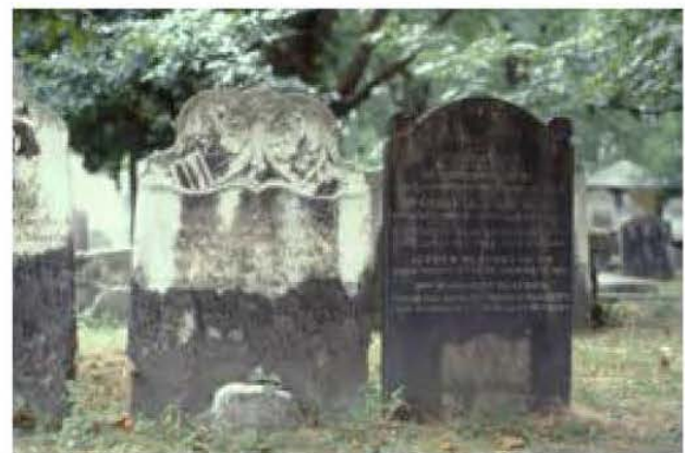
Figure 9. The limestone and sandstone grave markers in this historic cemetery have different weathering processes. On the left, the limestone shows surface loss in areas exposed to rainwater and gypsum crust formation below. The sandstone marker on the right displays uniform soiling, but surface hardening may be occurring. Photo: Fran Gale.
