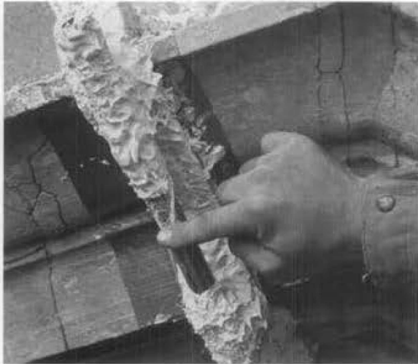
Figure 19. Molds for the replication of cast stone may be made on site using rubber materials and reinforcement. The molded profile of this window pediment will be used to run a plaster mockup, from which a production mold will be made. Photo: Michael Devonshire.
