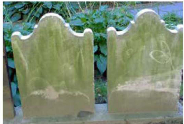
Figure 14. High-pressure water washing can damage grave markers. The photograph shows "wand marks" on the headstones produced by inappropriate pressure washing. Photo: Jason Church.
