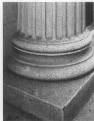
Figure 7. A combination of crushed white marble and black smelting slag was frequently used to give the appearance of a "white granite". The hammered finish on this early twentieth century cast stone would have been produced with a pneumatic chisel.
