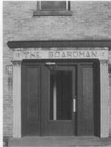
Figure 6. Cast stone was commonly used for molded trim in conjunction with brick or natural stone. This brick building in Rochester, New York, uses cast stone for the entry surround, and natural stone for unornamented window sills, thresholds, and water table units.
