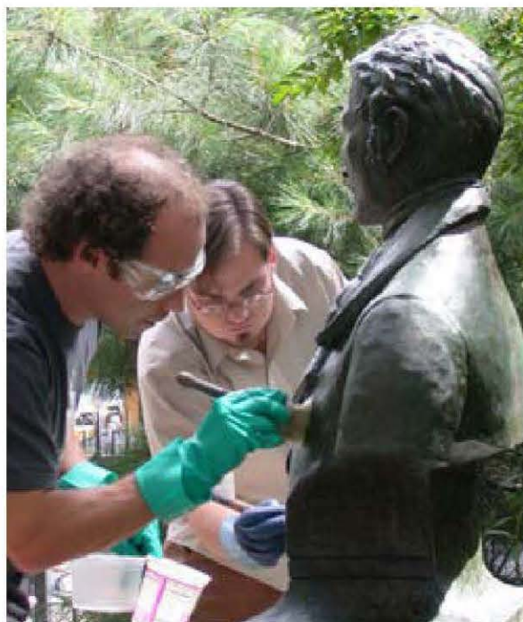
Figure 22. A protective coating must be maintained on metal elements. Wax or lacquer coatings help preserve the bronze patina and slow corrosion. Conservators apply a microcrystalline wax to this bust at St. Mark's Church in the Bowery, New York, NY. Photo: John Scott.
