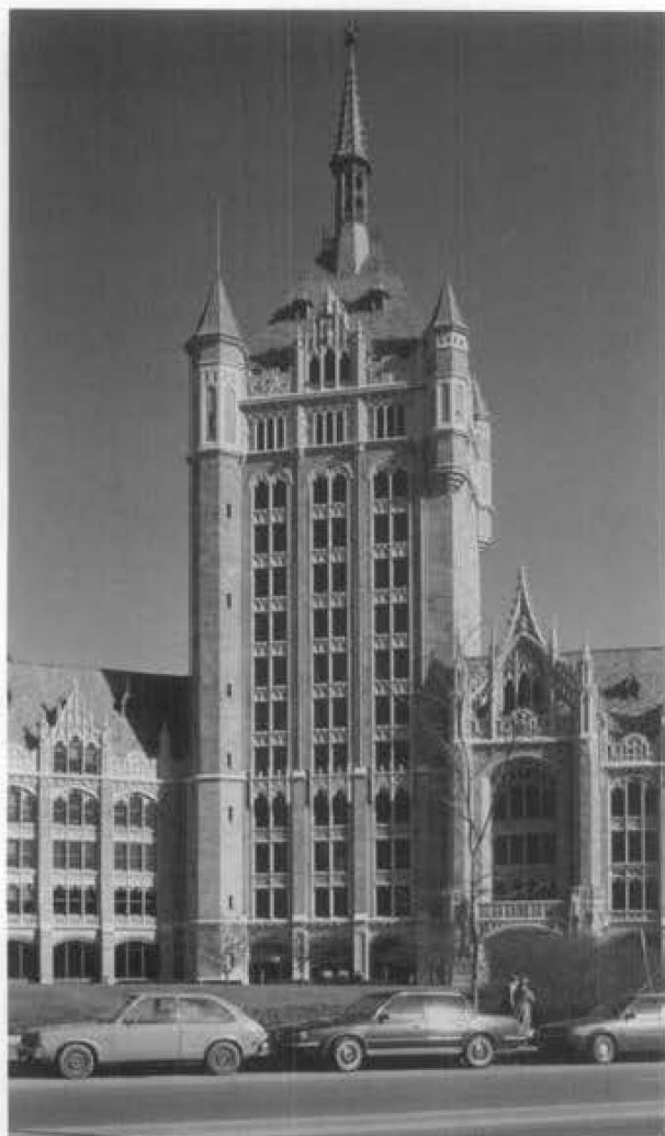
Figure 2. The prominent Delaware and Hudson Building in Albany, New York (1916) made extensive use of cast stone as trim combined with a random ashlar facing of natural granite. The elaborate gothic trim was produced by the Onondaga Litholite Company of Syracuse, New York.
