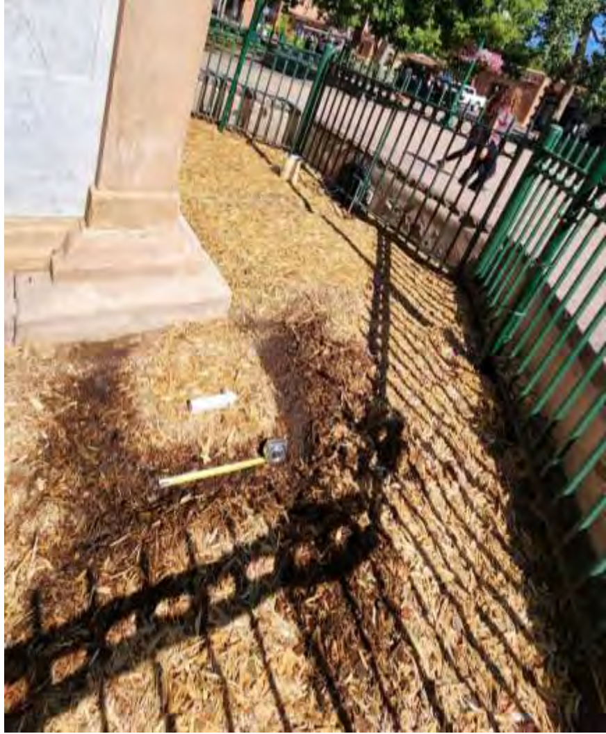
Figure 3. Begin assessment in the NE Corner.
