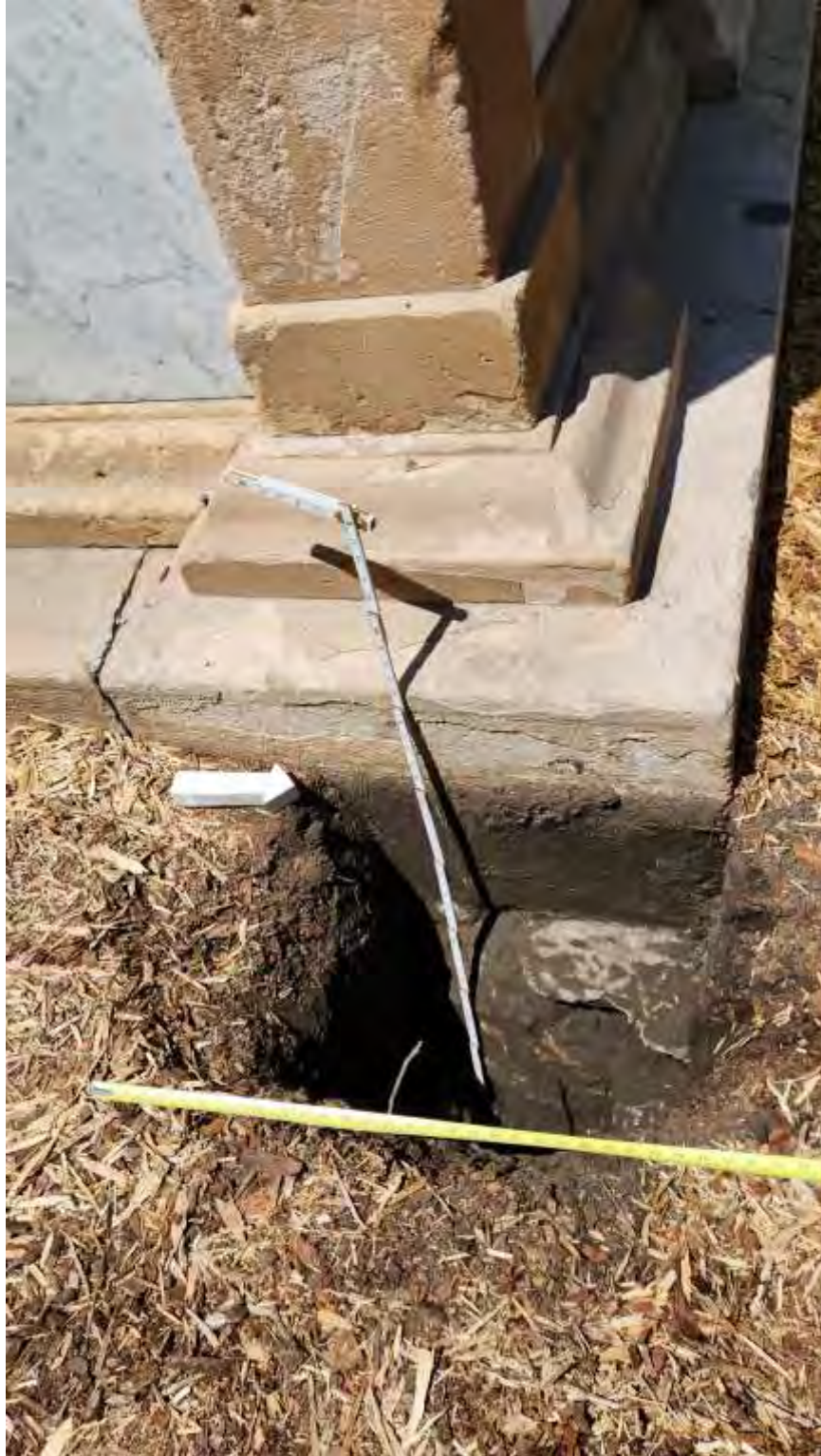
Figure 6. Bottom of excavation.
