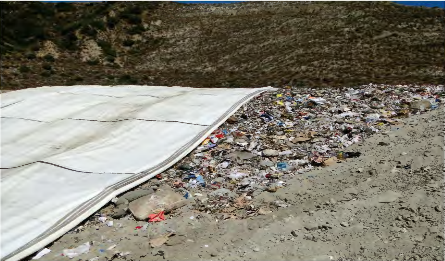
Photo 2: Tarp Laid Over Trash
