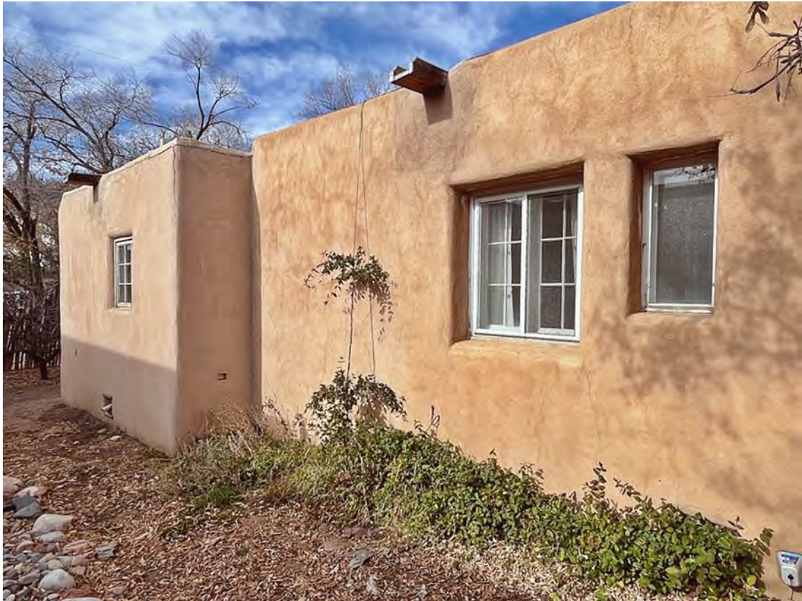
Photo 13: South elevation, west end. Camera facing northwest.
