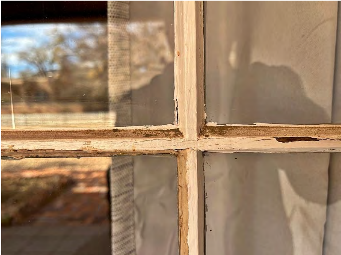
Photo 5: East (front) façade. Muntin profile. Camera facing west.
