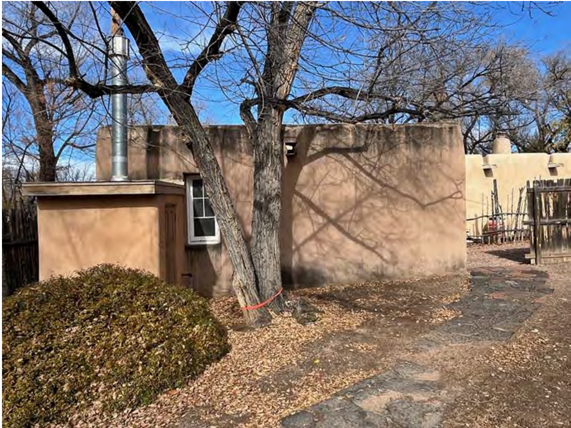
Photo 16: Garage. South elevation. Camera facing north.
