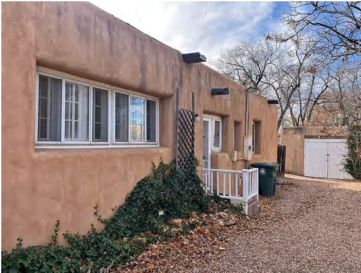
Photo 9: North elevation. Camera facing southwest.
