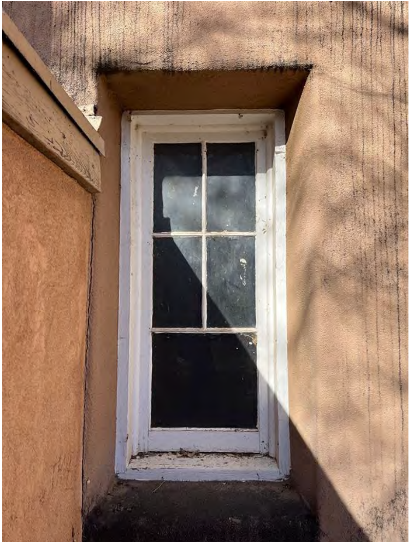
Photo 15: Garage. South elevation window. Camera facing north.
