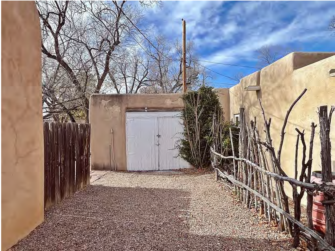
Photo 14: Garage. East elevation. Camera facing west.
