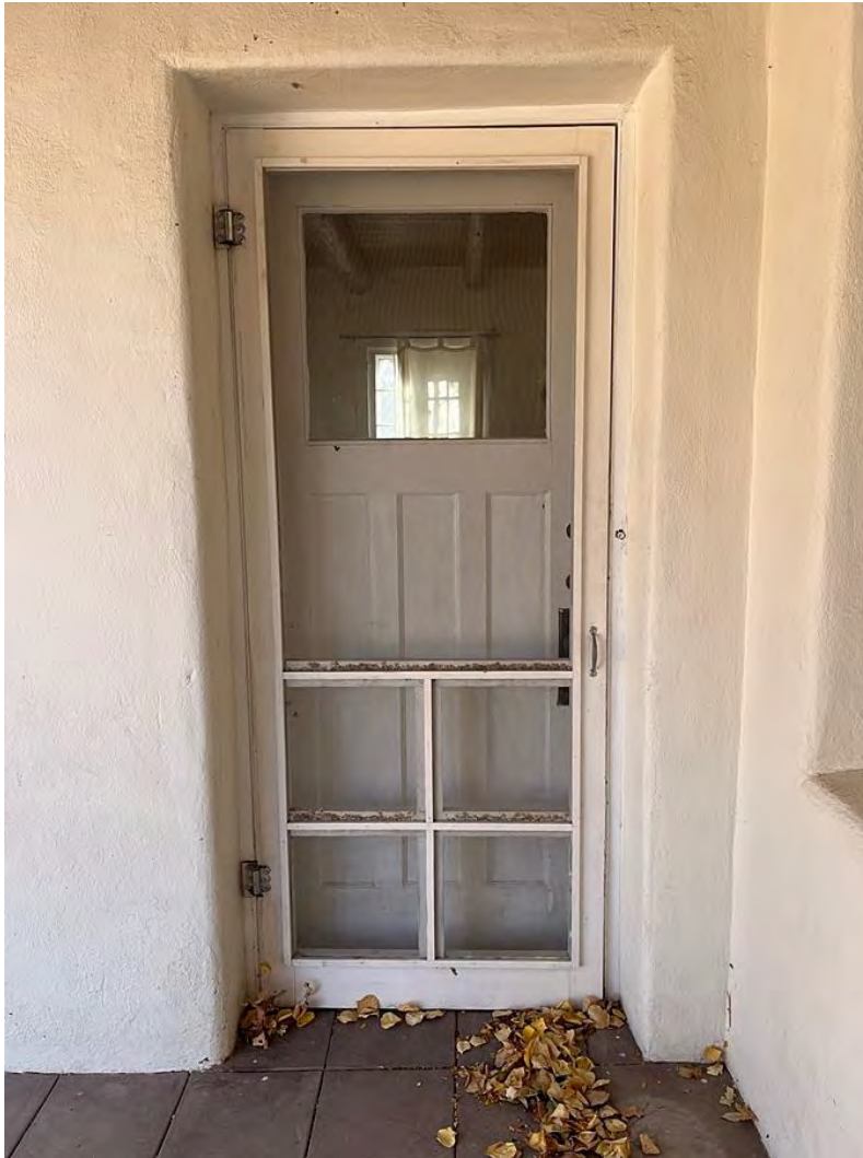
Photo 8: East (front) façade. Portal, entry door. Camera facing south.
