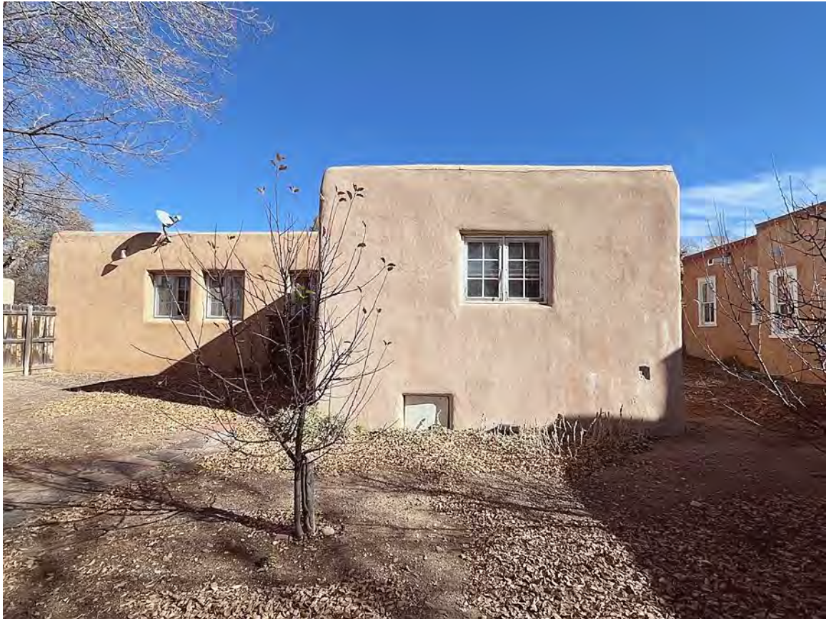
Photo 11: West elevation. 1995 addition at right. Camera facing east.
