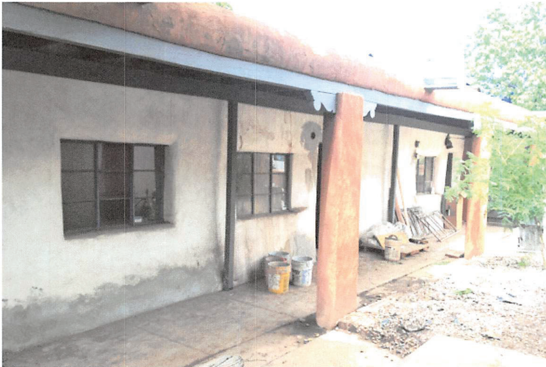
Portal at East Elevation
