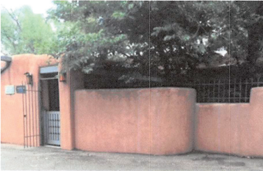
Entrance at West Elevation
