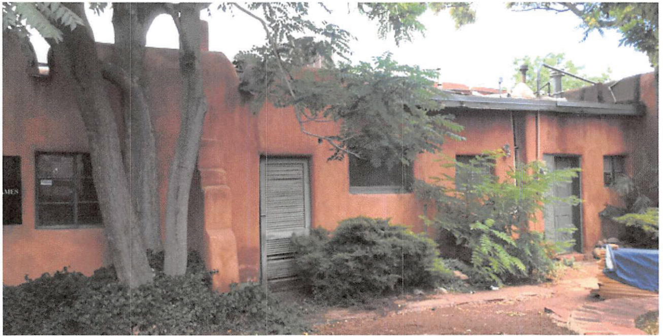
South elevation of patio
