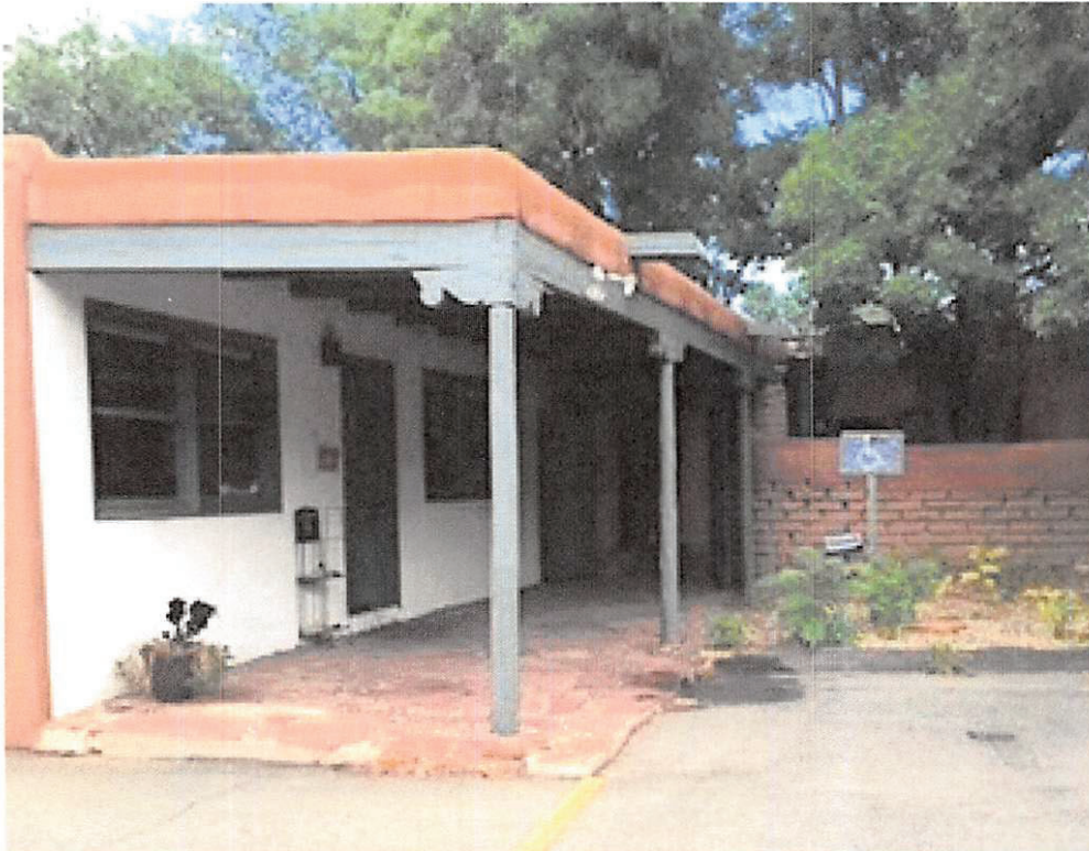
Portal and east elevation
