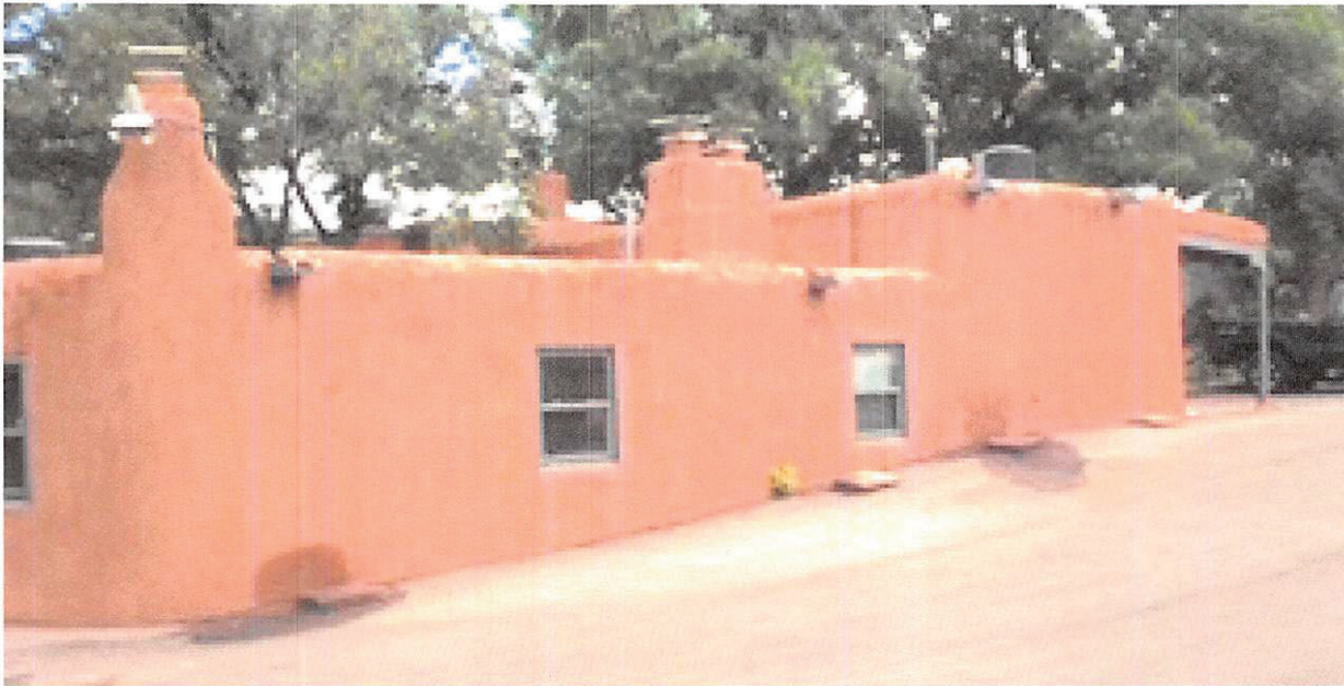
Southwest corner and south elevation
