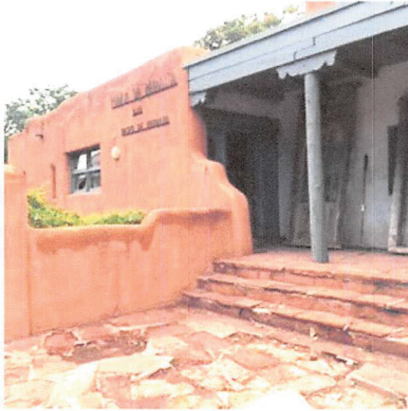
Detail of north entrance
