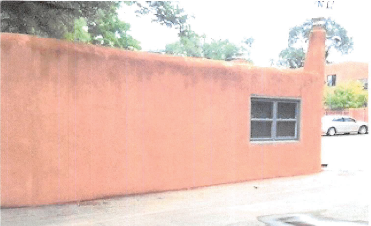
South end of West Elevation
