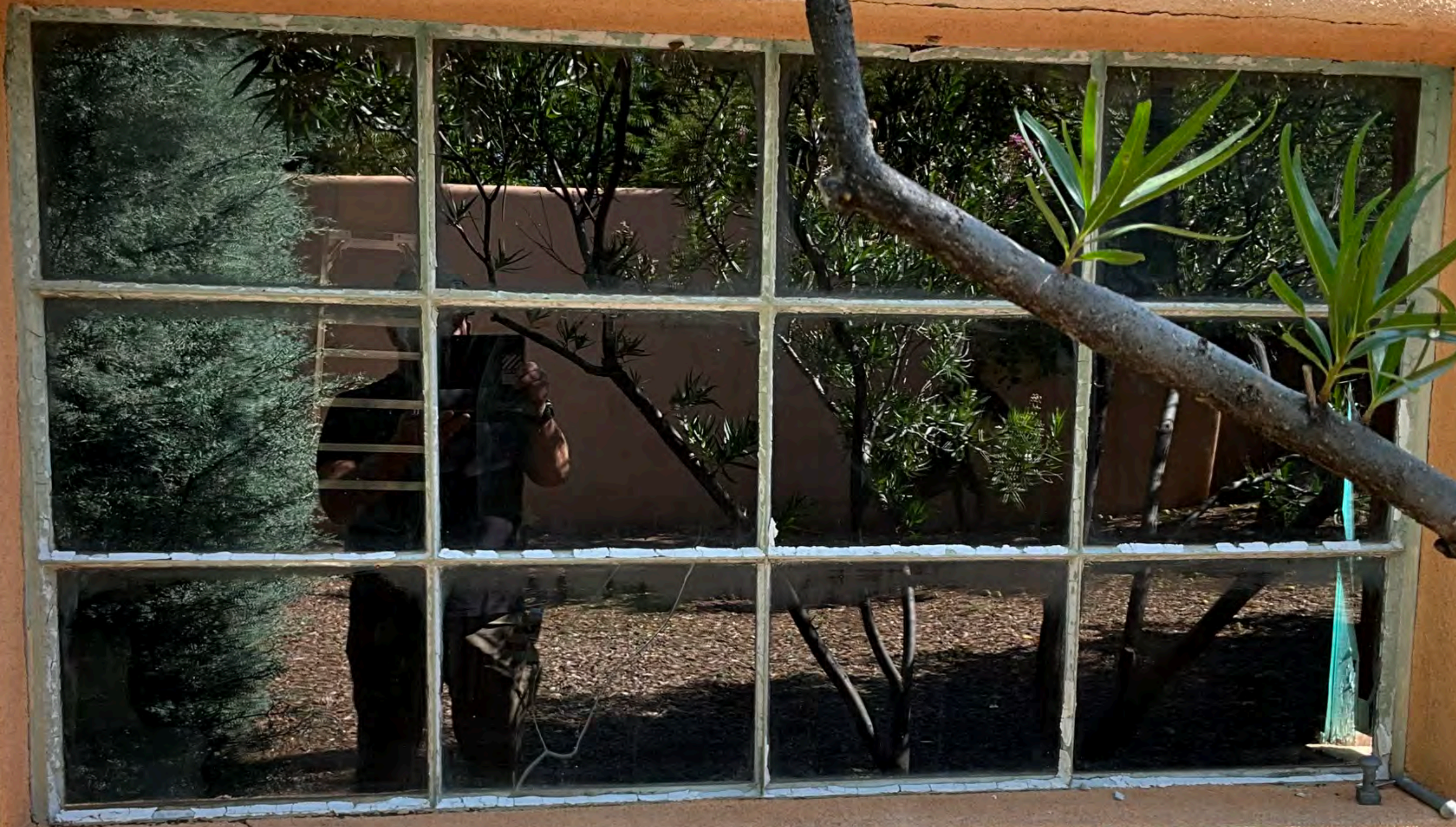
Garage South Elevation Window G-N
