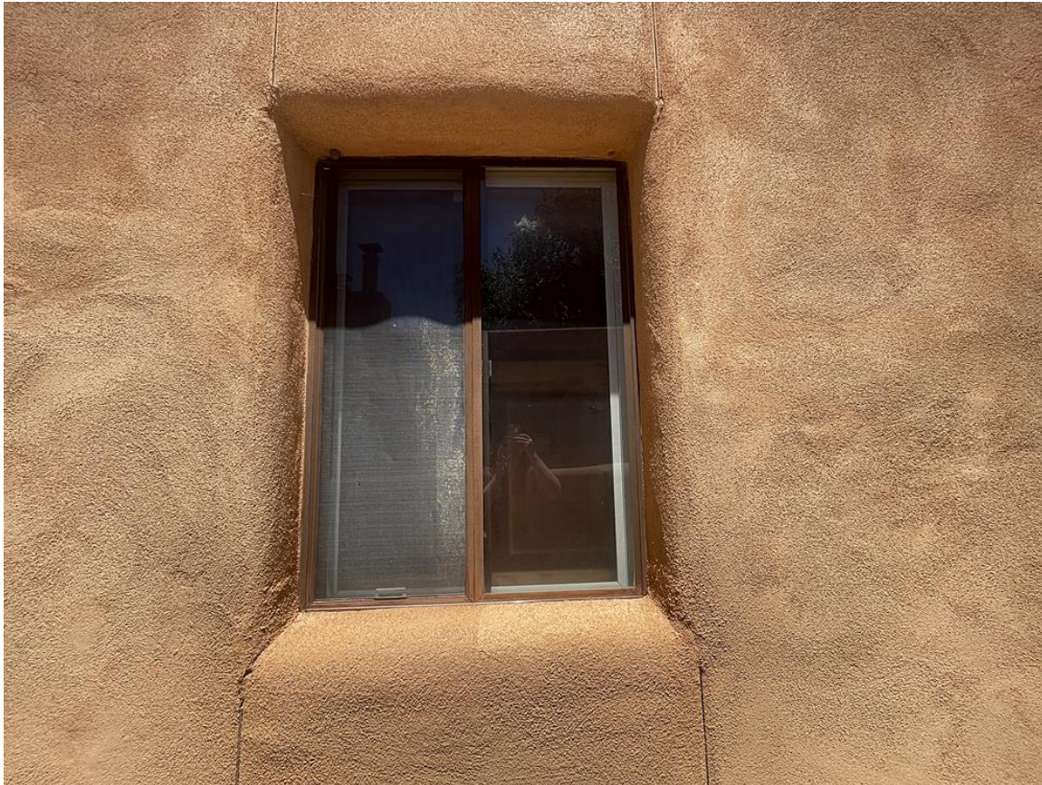
Photo 14: South elevation. Original section. Window detail. Camera facing north.
