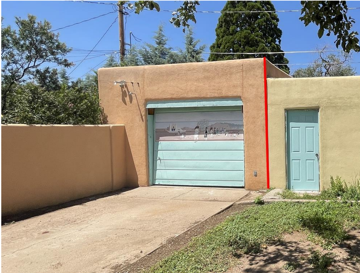
Photo 15: Garage (left of red line). Camera facing southwest.
