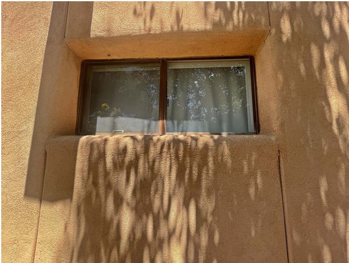
Photo 13: South elevation. Privacy window at primary bedroom addition. Camera facing north.
