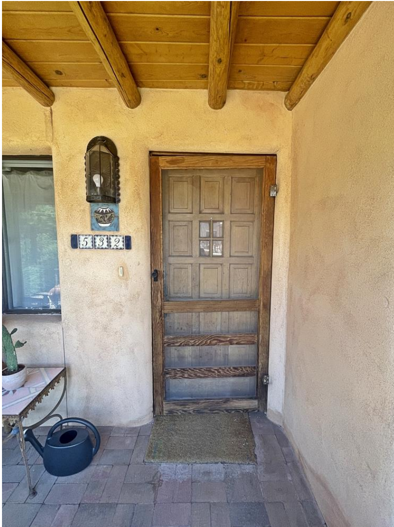
Photo 4: East (front) façade. Front entry door. Camera facing west.
