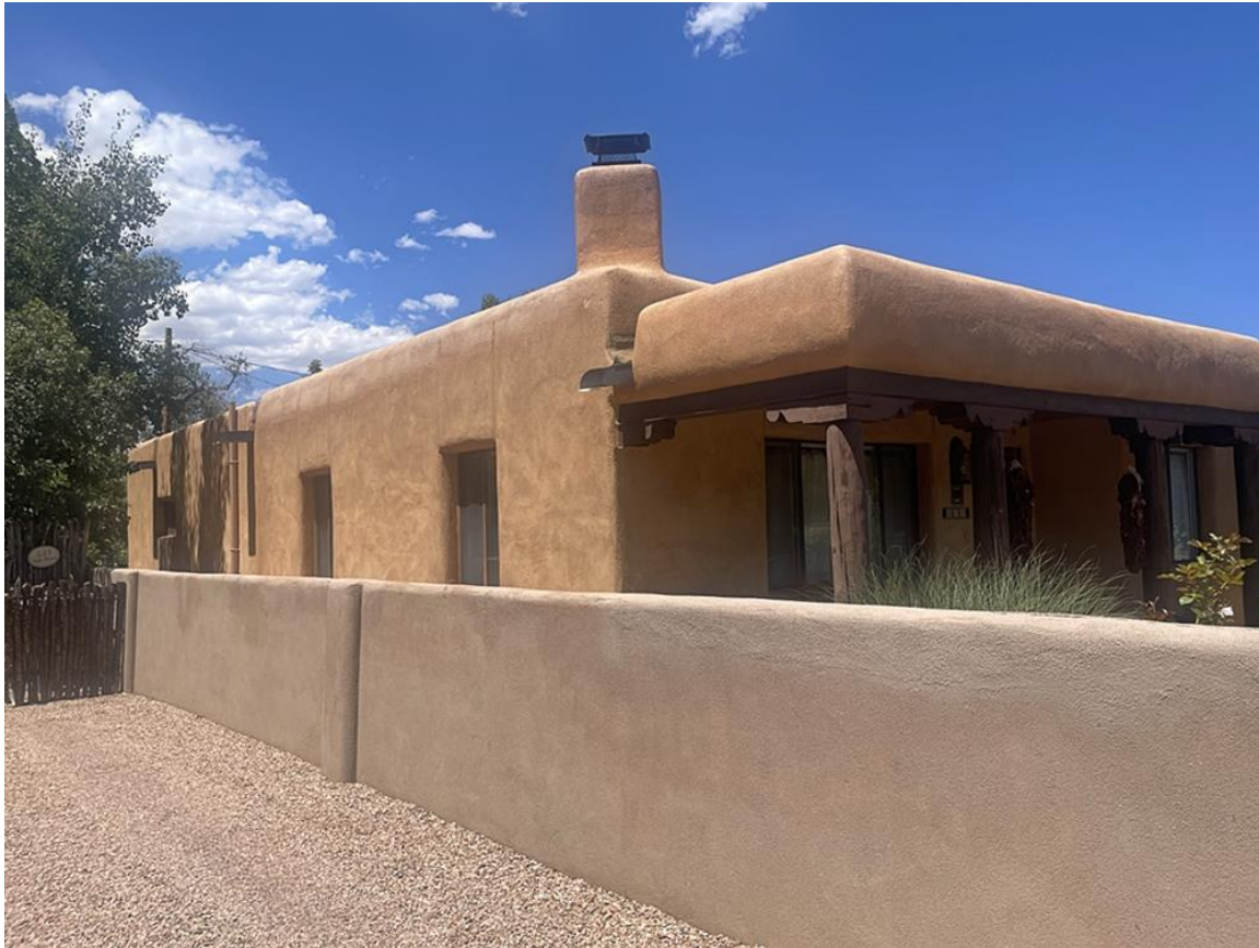
Photo 12: South elevation and property wall. Camera facing northeast.
