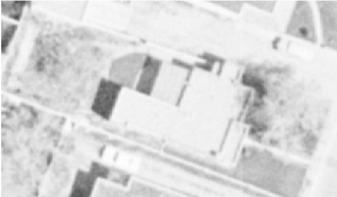
Figure 5: June 6, 1966, aerial photograph. Note presence of primary bedroom addition, roofed patio, and canopy over laundry room entry.
