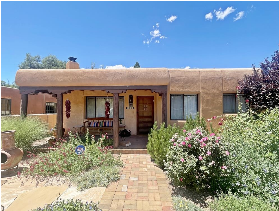
Photo 2: East (front) façade. Camera facing west.
