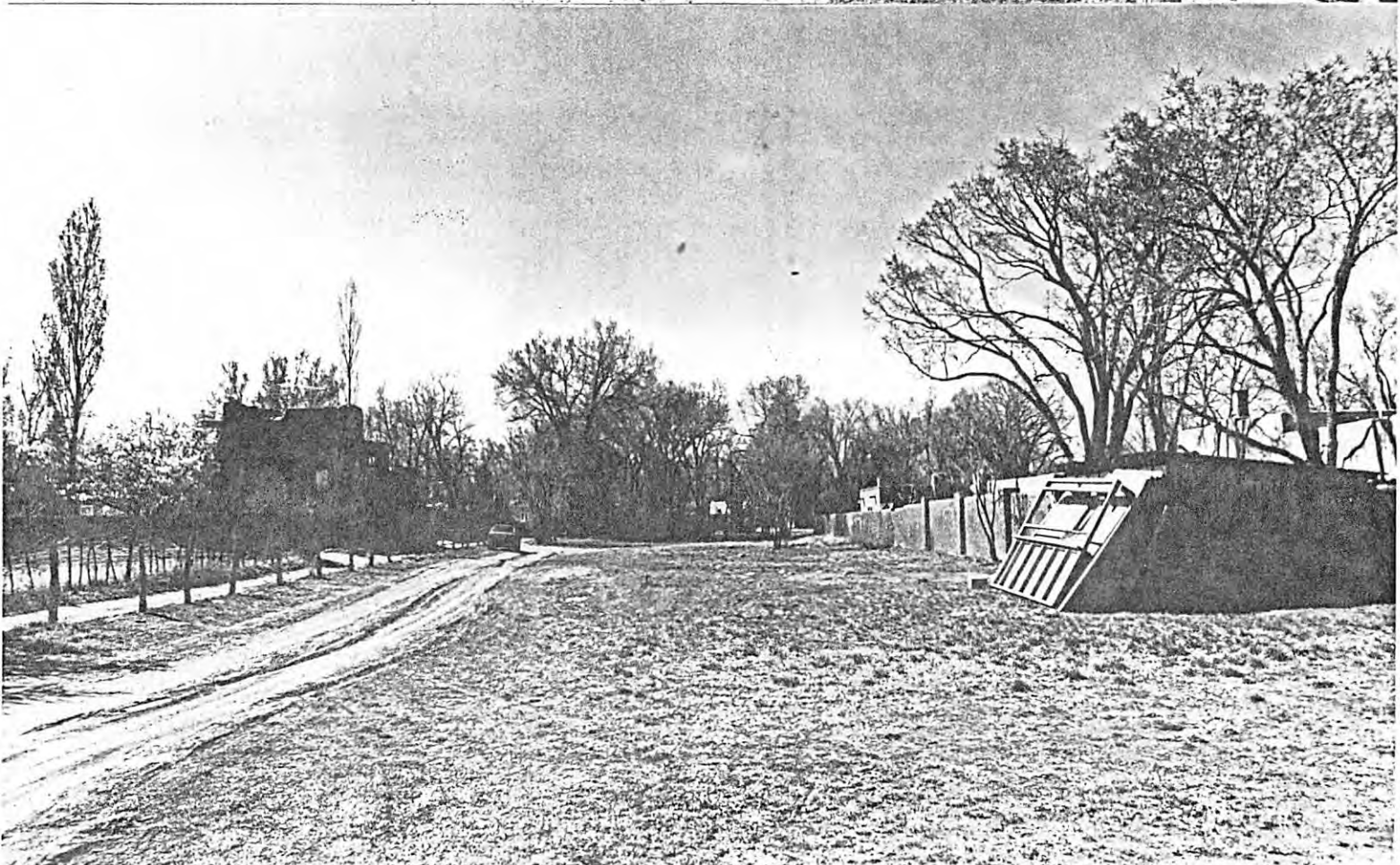
NORTH ELEVATION FROM GORMLEY ACCESS 160' OFF CANYON ROAD
