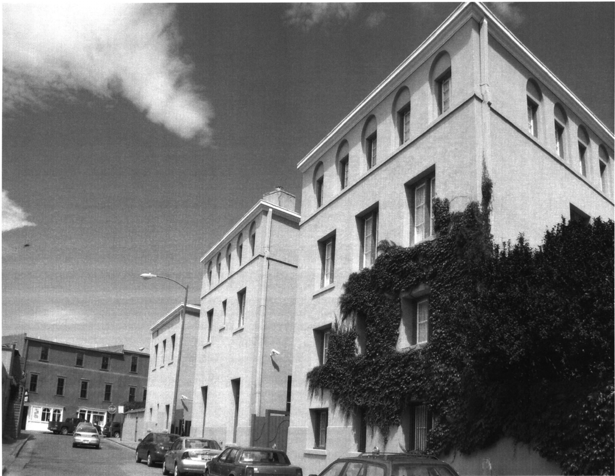
THE VIEW FROM ORTIZ STREET THE EXISTING BOLLER FIVE IS VISIBLE.
