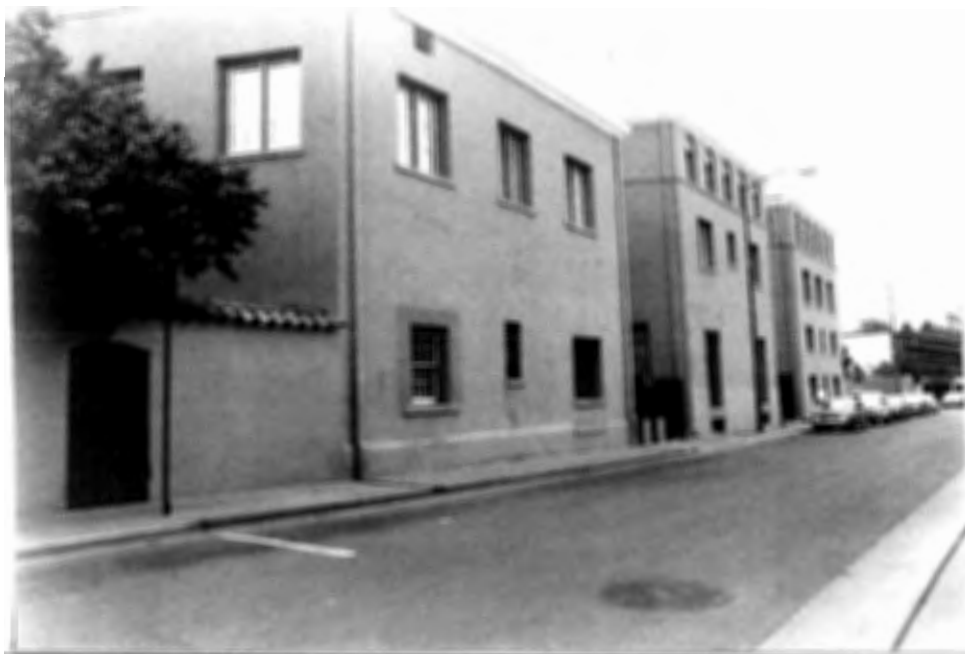
#14 west elevation, N end
