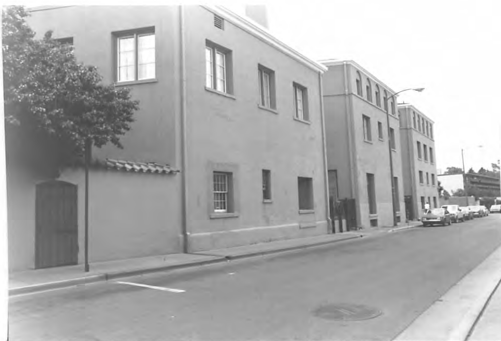
#14 west elevation, N end
