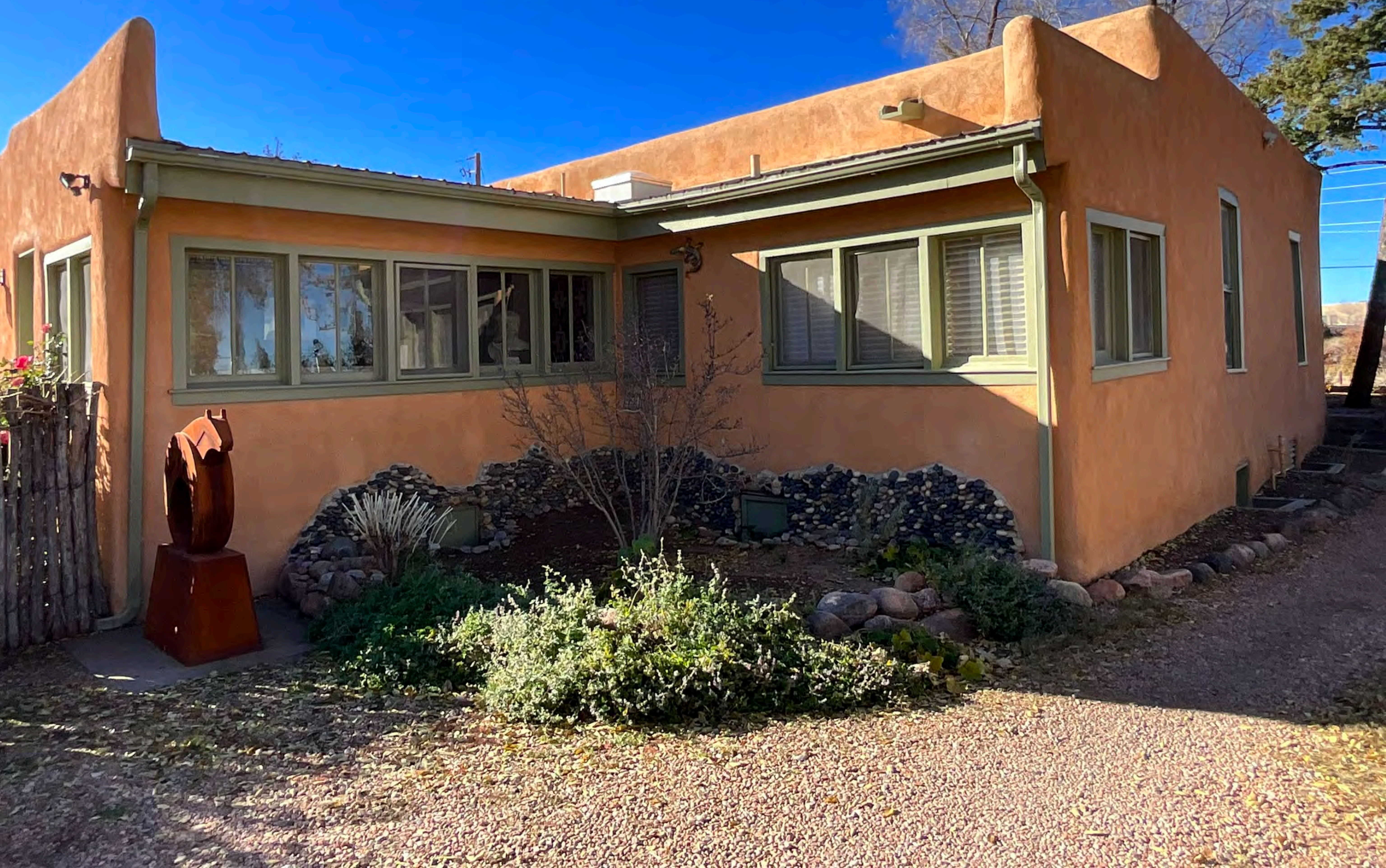
801 Old SF Trail NorthEast Elevation
