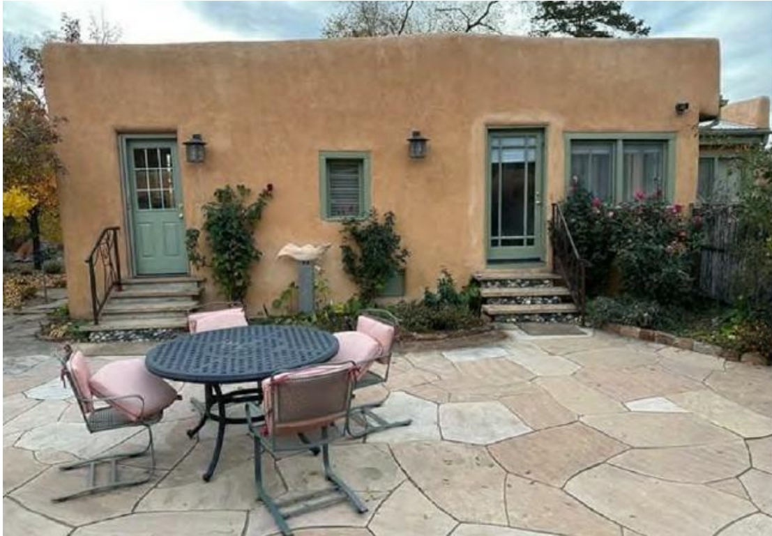
Figure 3: East Elevation of Residence
