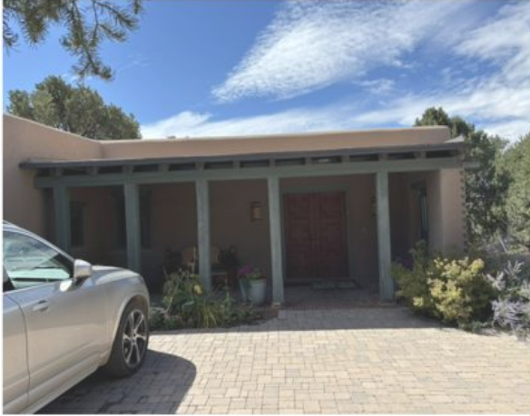
EAST ENTRY PORTAL STREET SIDE
