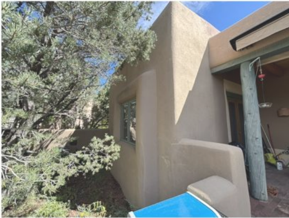
WEST SIDE PATIO AND PORTALS
