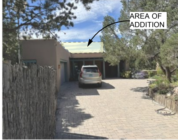
EAST ENTRY PORTAL STREET SIDE
