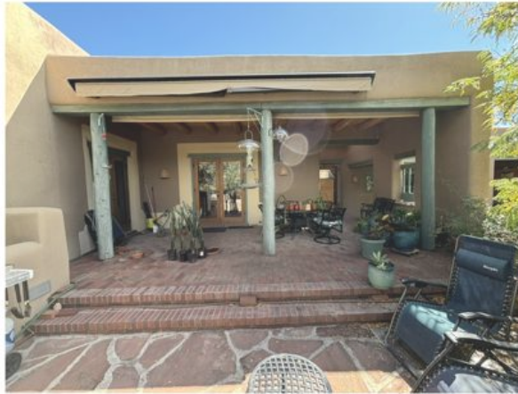
WEST SIDE PATIO AND PORTALS
