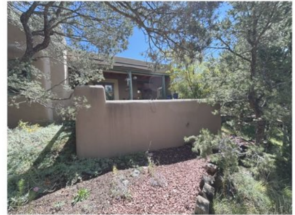
WEST SIDE PATIO AND PORTALS
