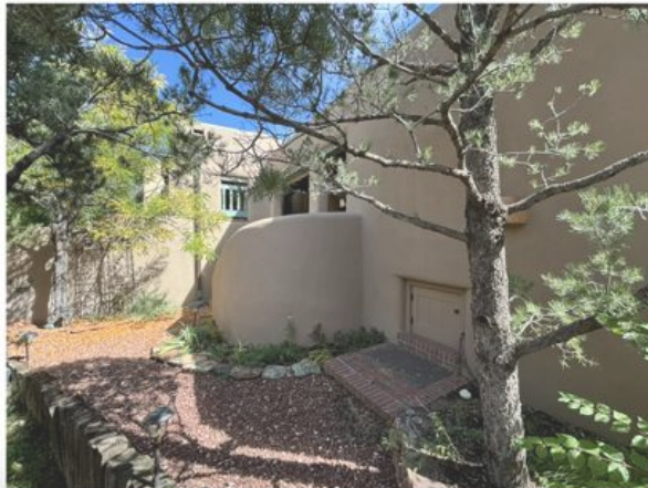
WEST SIDE STAIRS / PATIO WALLS
