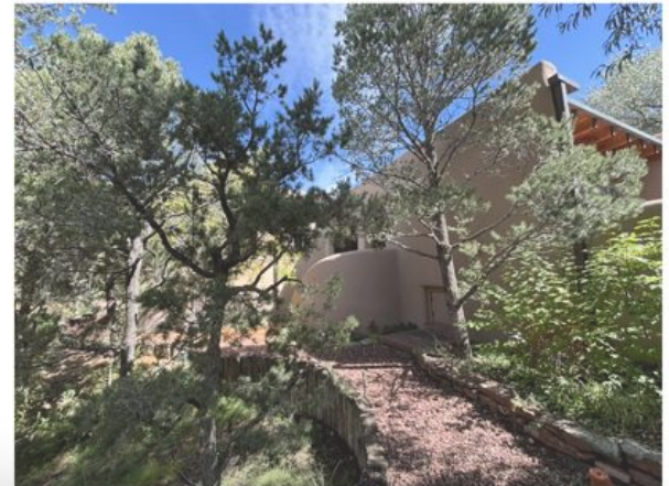
WEST SIDE STAIRS / PATIO WALLS
