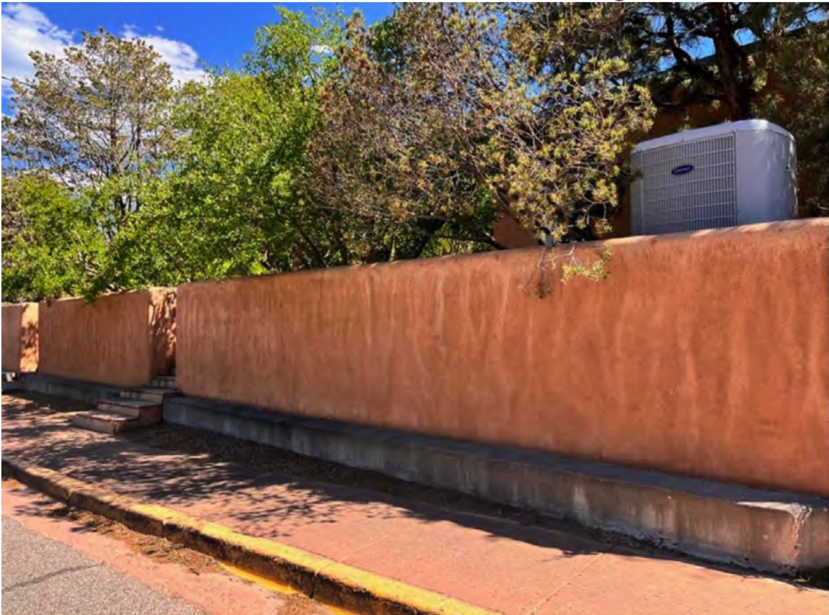
Alto Street retaining wall. Camera facing southeast.
