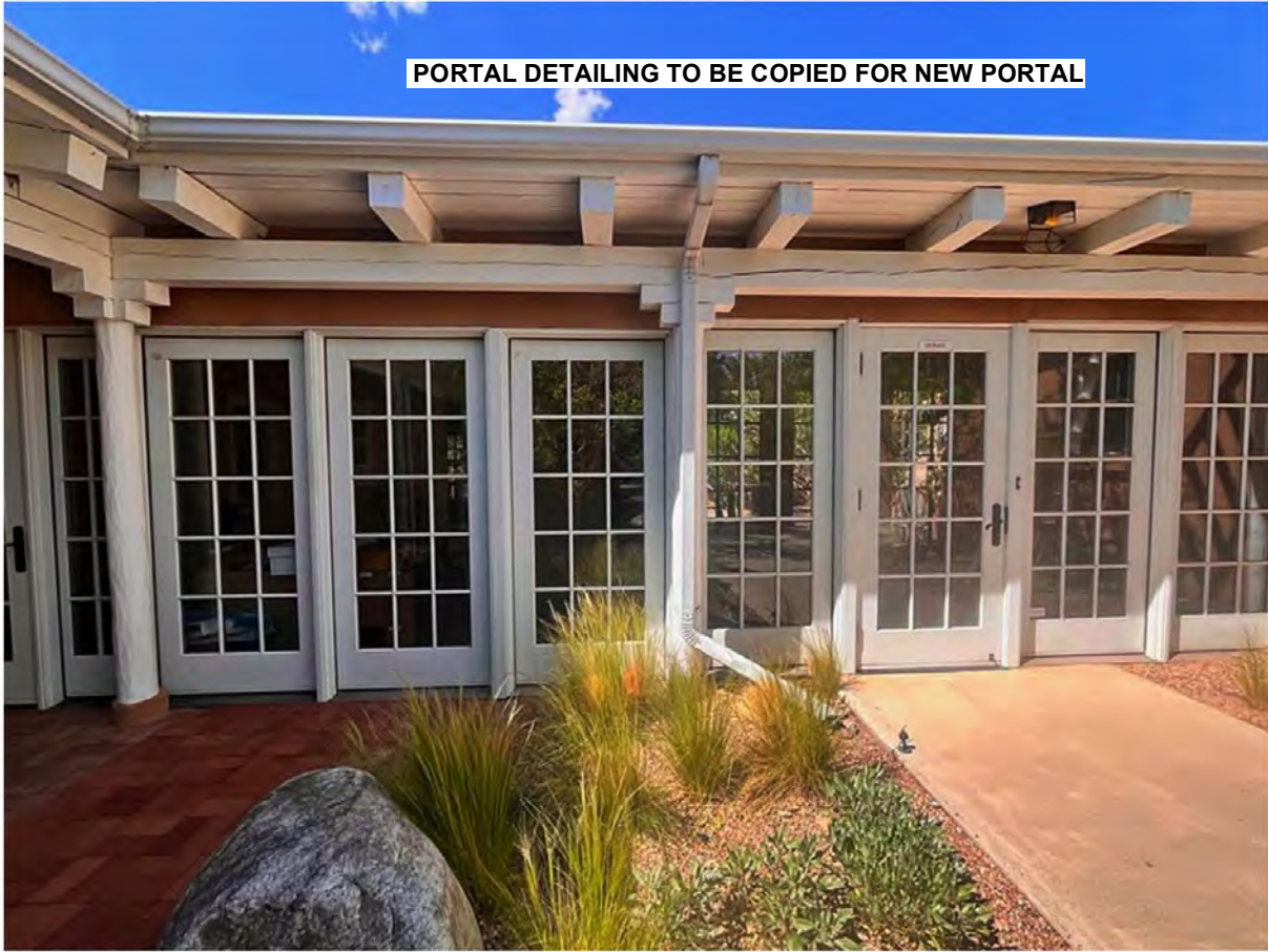
Glazed corridor between 516 and 516 ½. Camera facing north.
