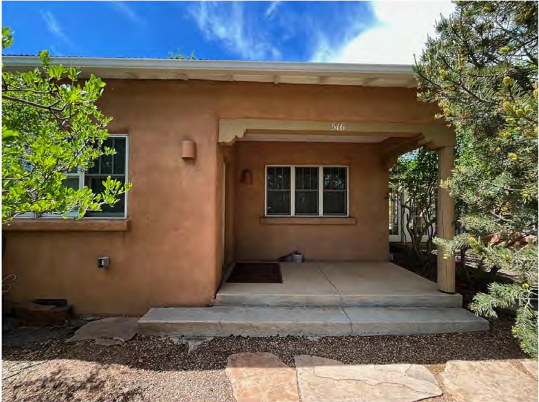
North façade of 516. Camera facing south.
