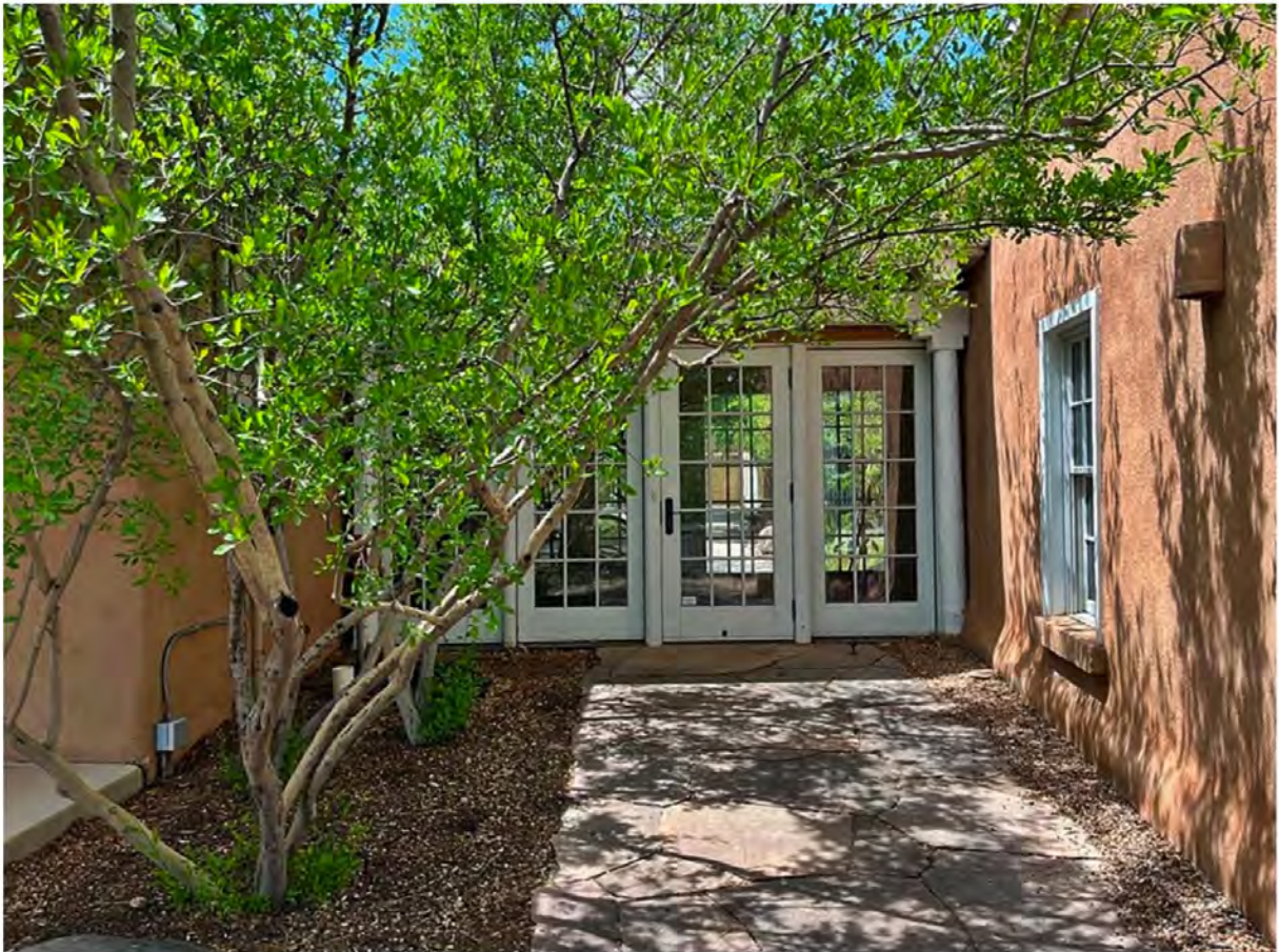
: Glazed corridor between 516 and 516 ½. Camera facing south.
