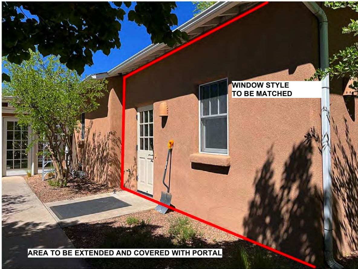
West (courtyard) elevation of c.1996 addition to 516. Camera facing northeast.
