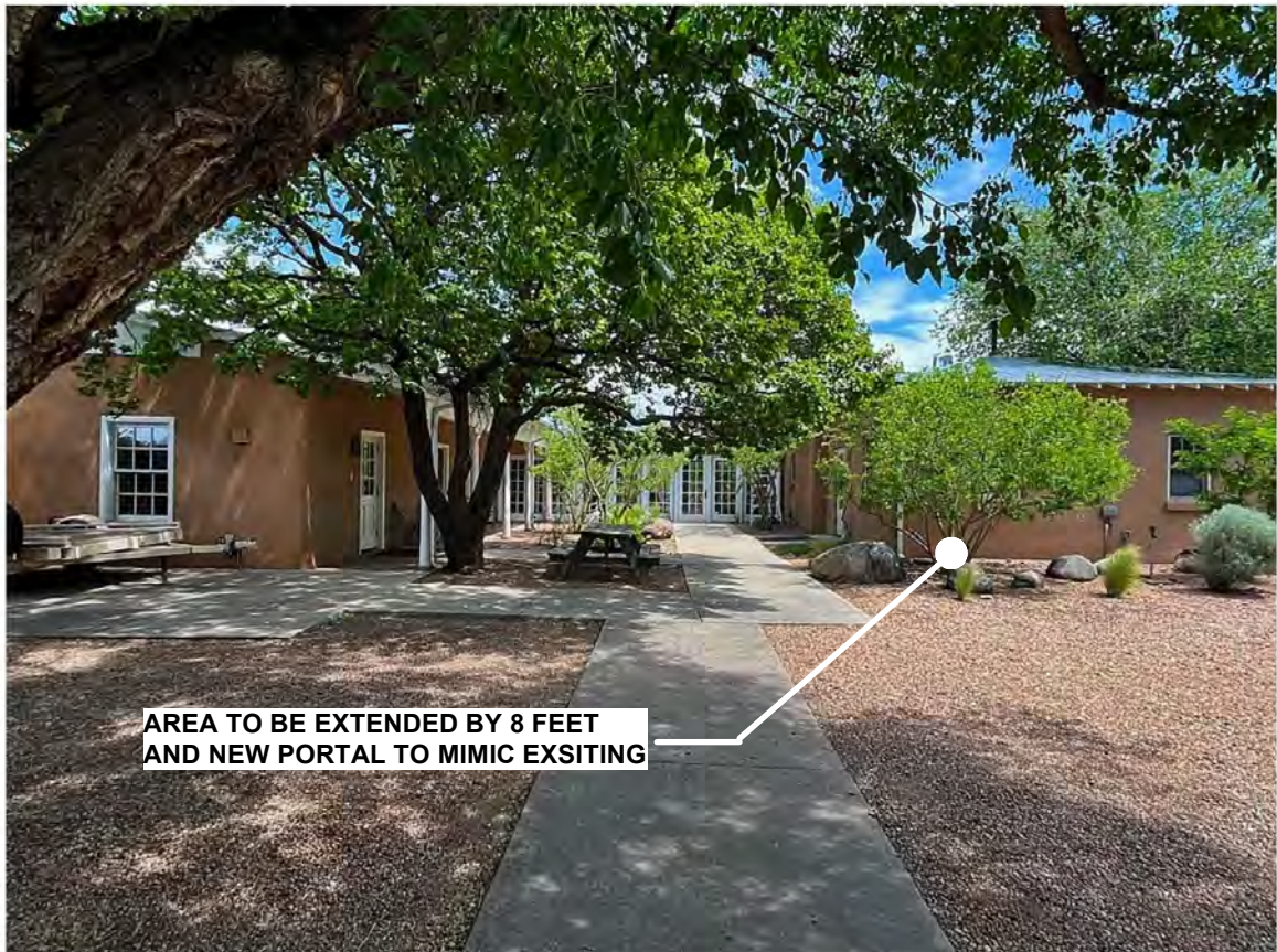
Courtyard elevation. Camera facing north.
