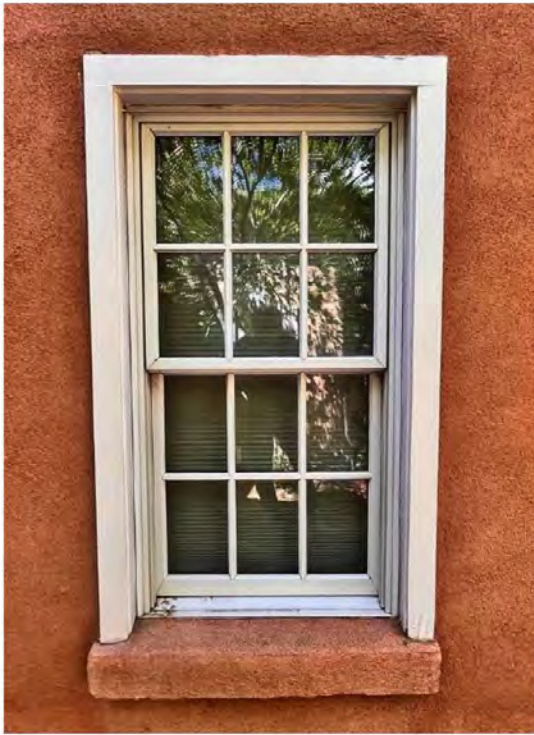
Reconstructed window openings with 1990s Pella vinyl clad units.
