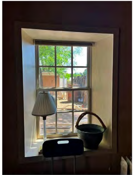
Reconstructed window openings with 1990s Pella vinyl clad units.
