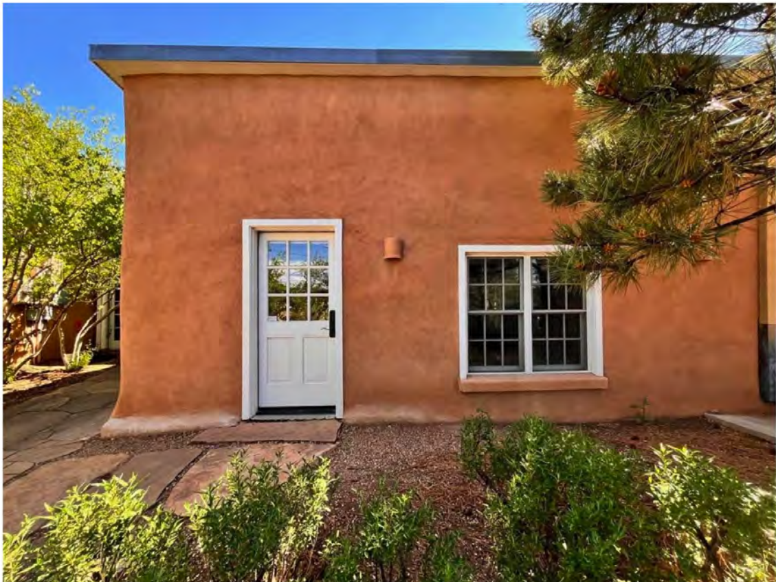
North façade of 516 ½. Camera facing south.
