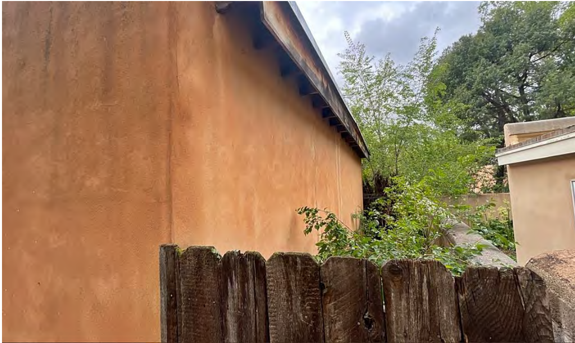
Photo 24: Garage. North elevation. Camera facing west.
