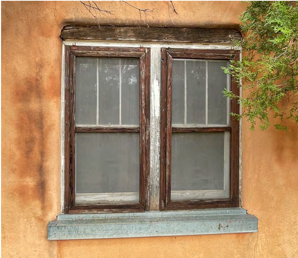
Photo 8: South elevation. Window at bedroom detail. Camera facing north.
