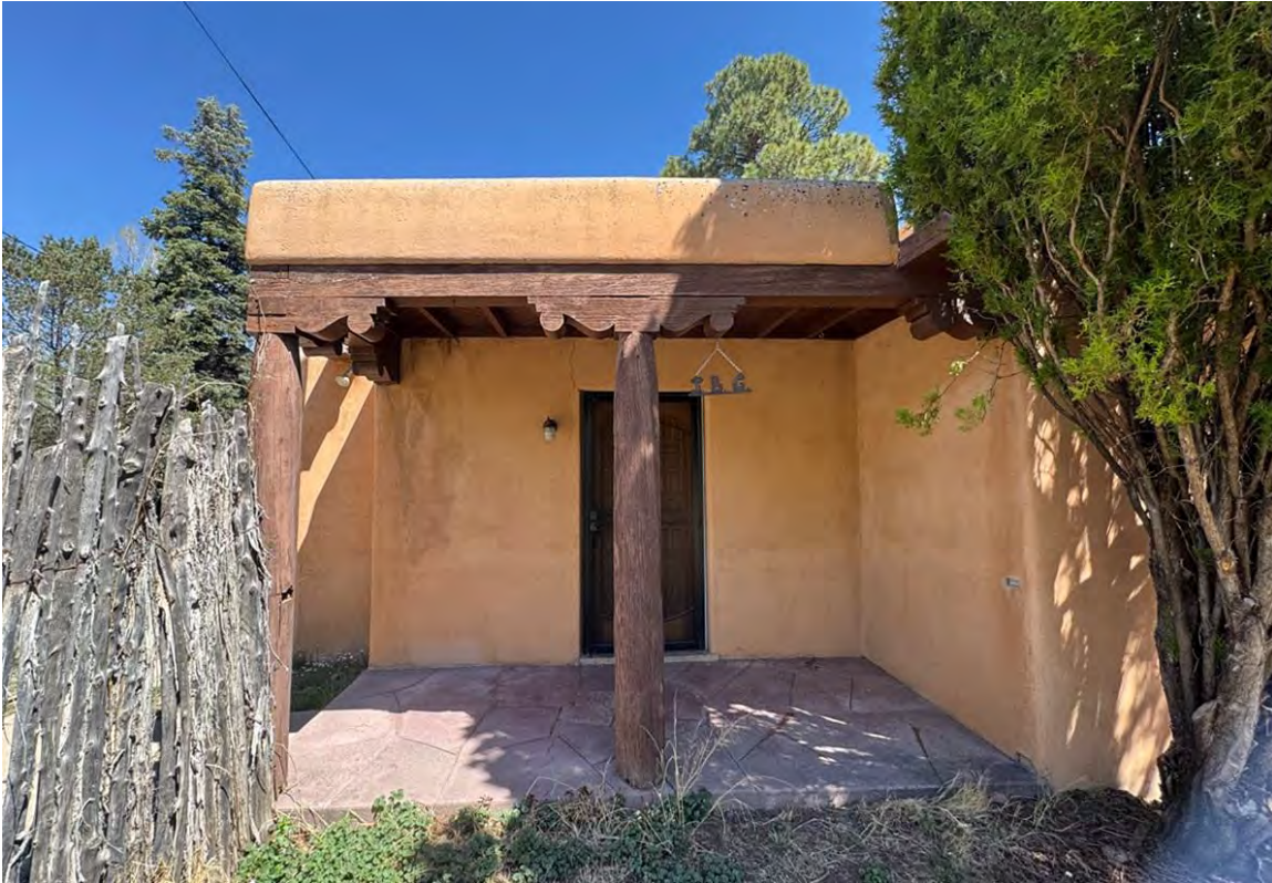
Photo 5: South elevation. Portal. Camera facing north. Aviva Baumann, April 23, 2025.
