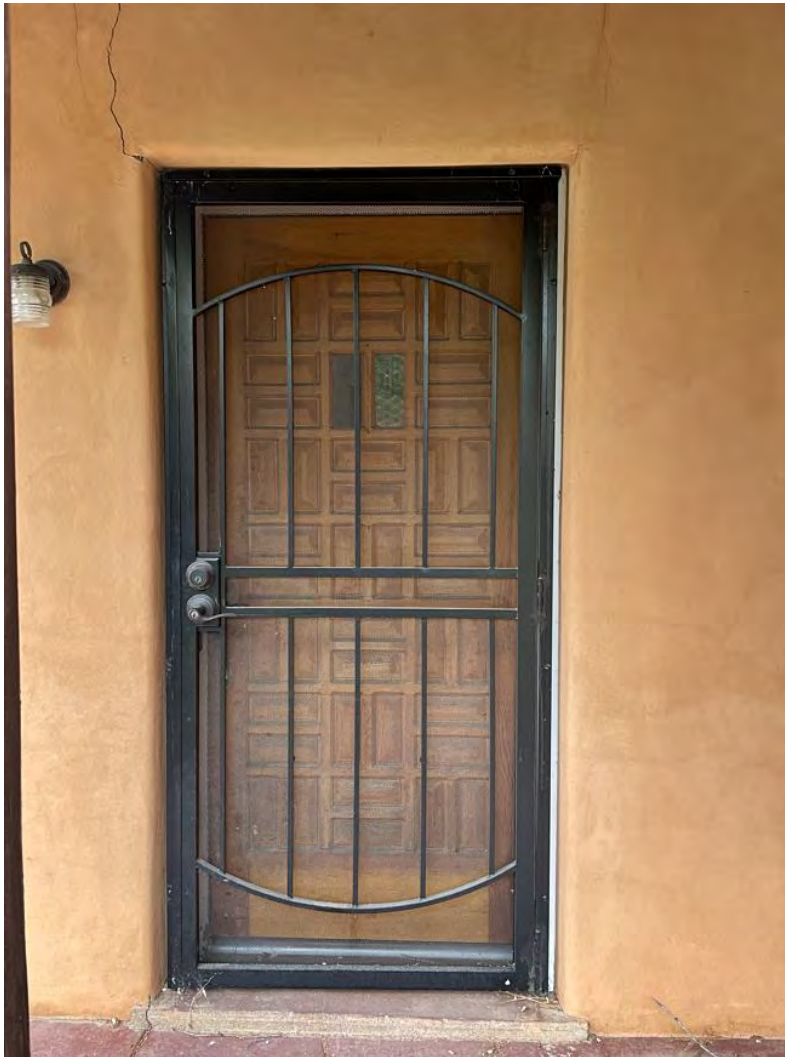
Photo 6: South elevation. Entry door. Camera facing north.
