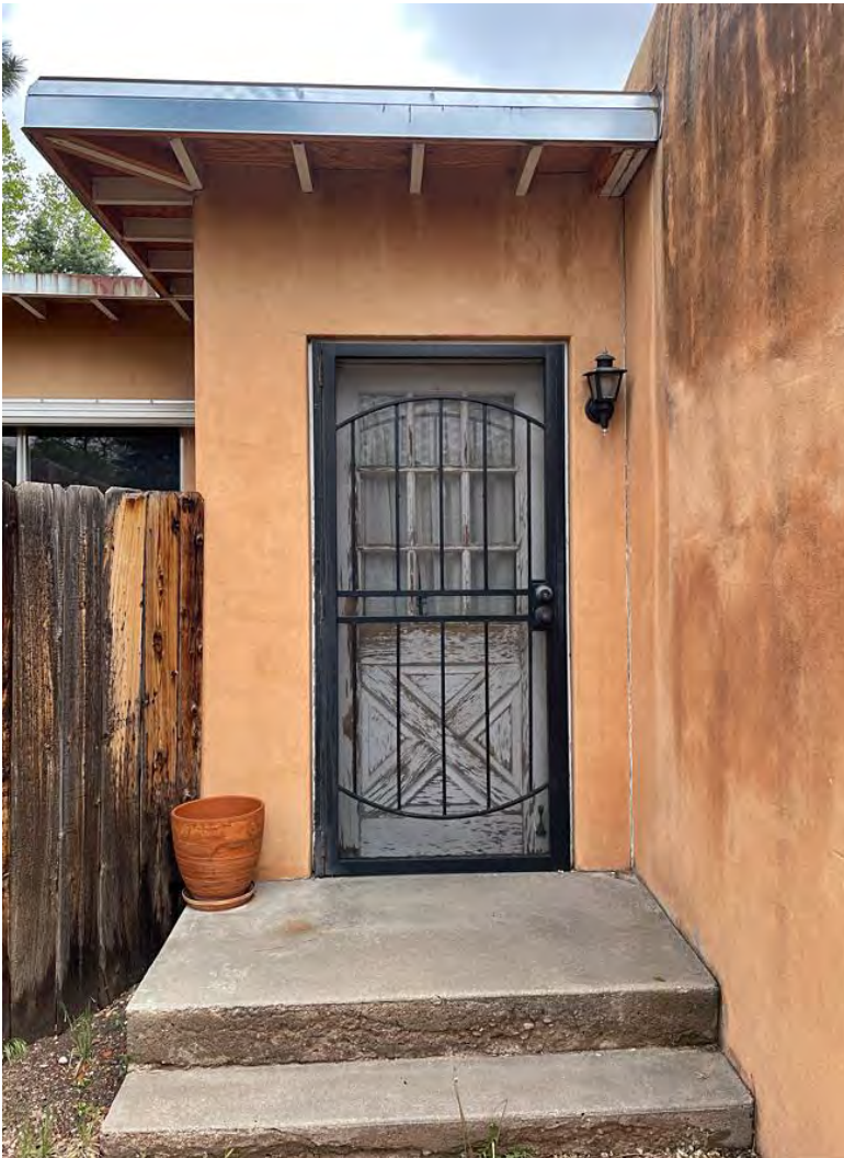
Photo 13: West elevation. Addition. Detail of entry door. Camera facing east.
