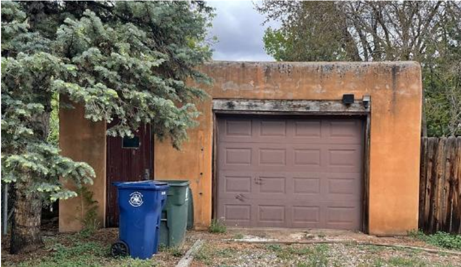
Figure 3: South Elevation of Accessory Structure
