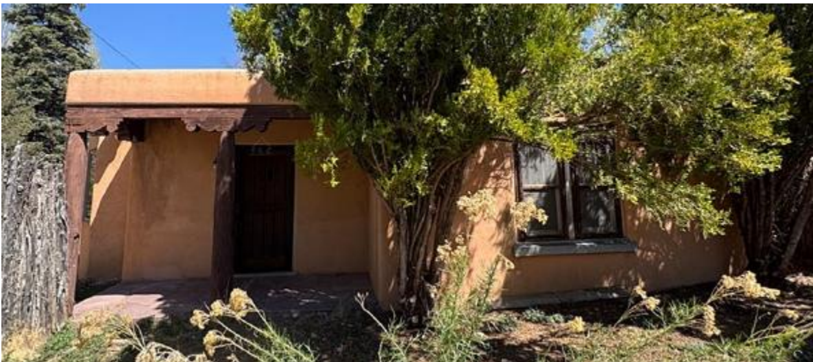
Figure 2: South Elevation of Residential Structure
