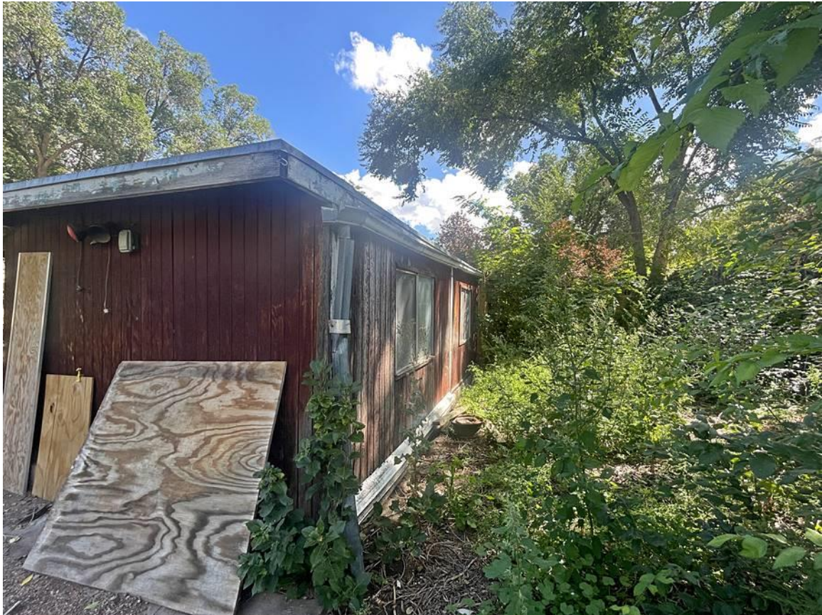
Photo 10: West elevation. Workshop. Camera facing northeast.
