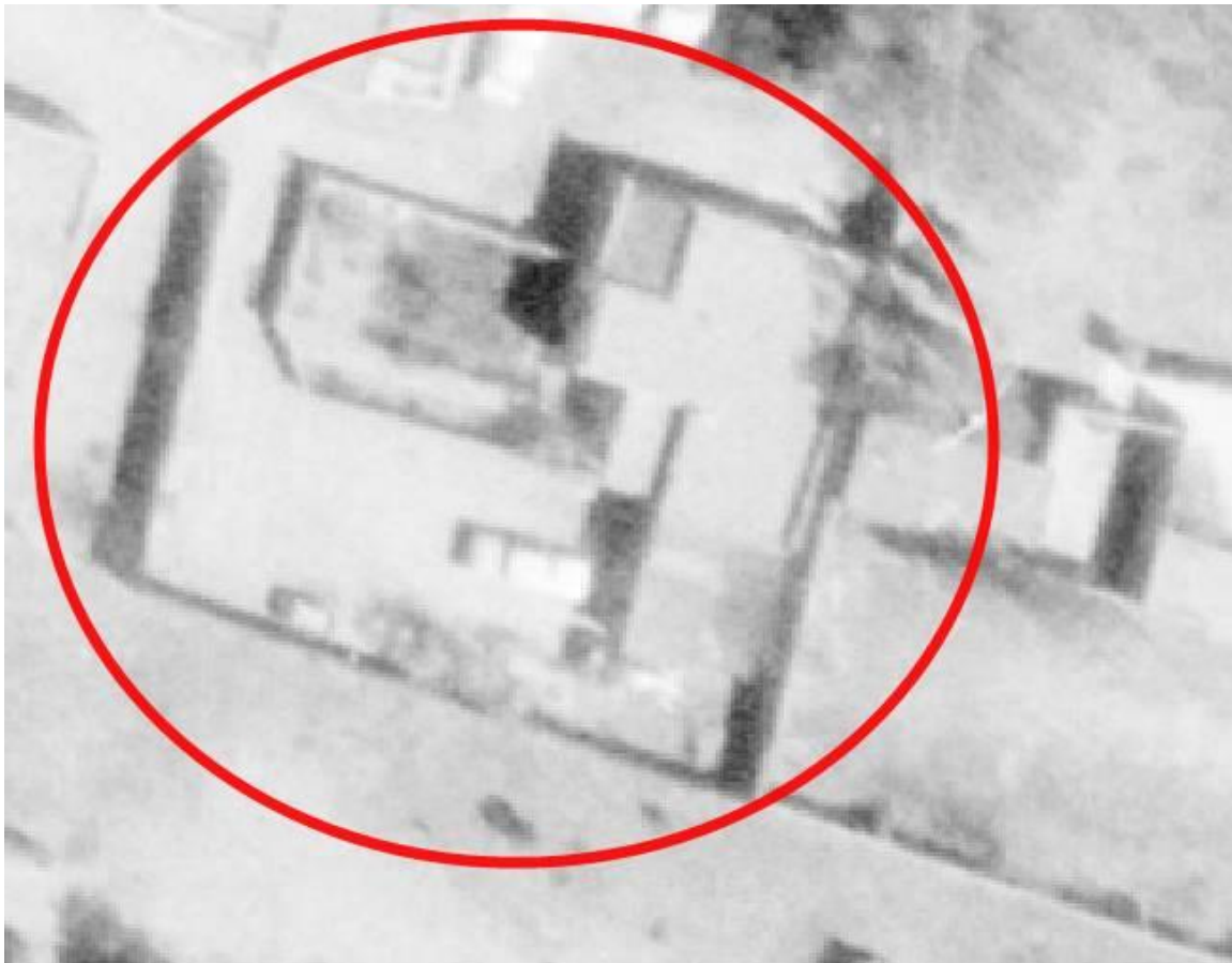
Figure 4: May 2, 1966, aerial photograph. Note the patio or open porch at the northwest has been enclosed and several additions to the rear have been built.
