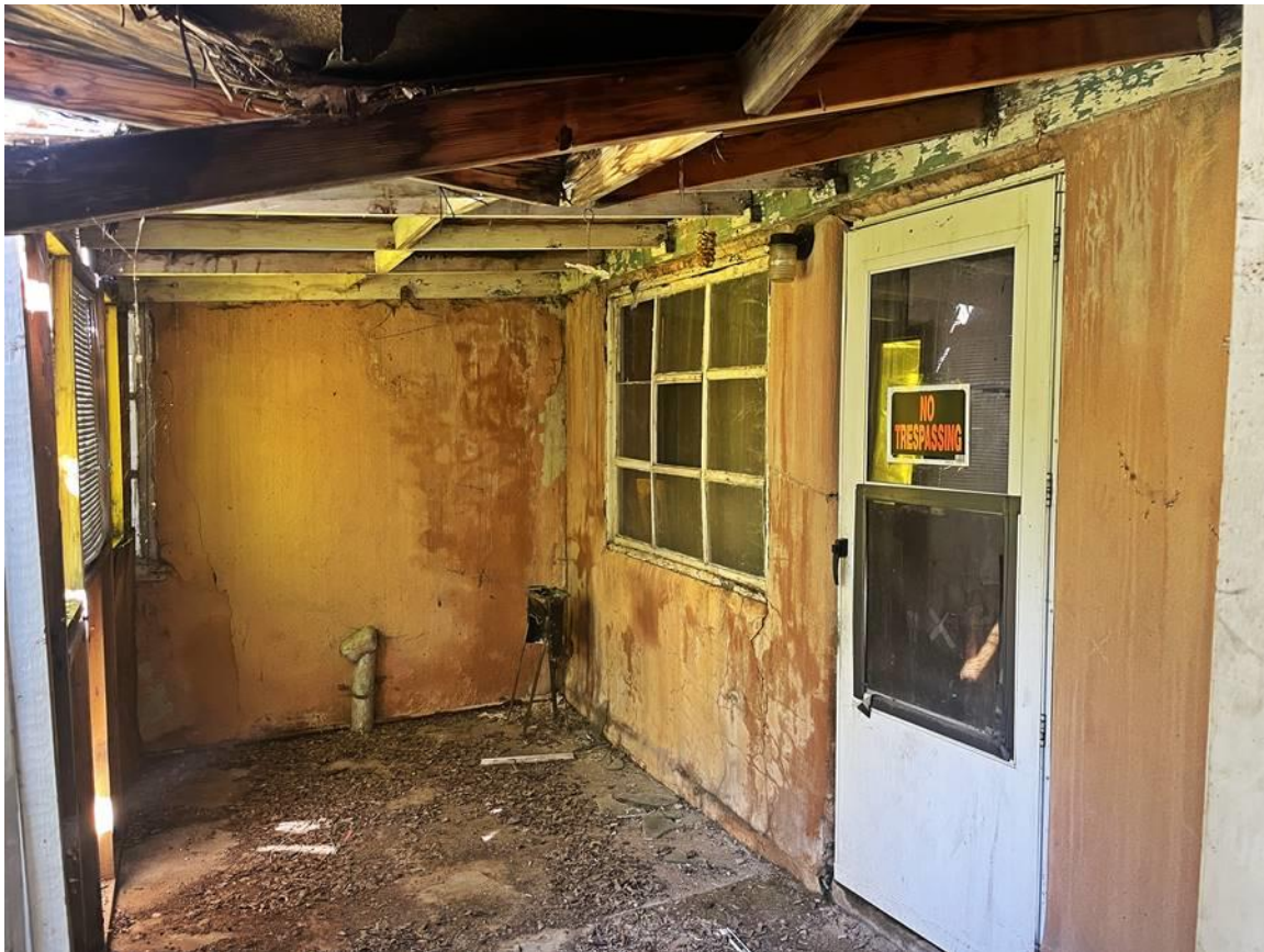
Photo 7: West elevation. Entry inside plywood porch enclosure. Camera facing northeast.
