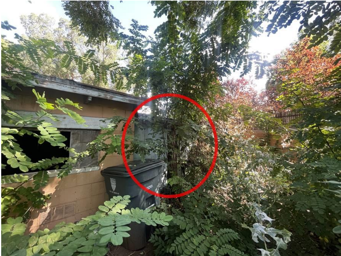
Photo 13: South elevation. Wood board storage room circled. Camera facing northeast.
