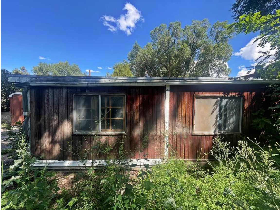
Photo 11: South elevation. Workshop. Camera facing north.
