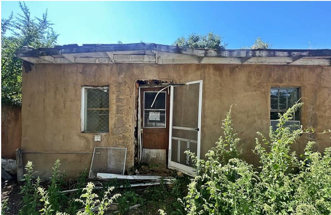
Photo 2: North elevation. Older part of home. Camera facing south.
