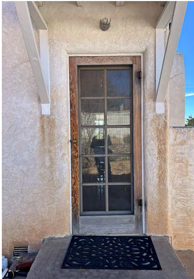
Photo 9: North elevation. Kitchen entry door. Camera facing south.
