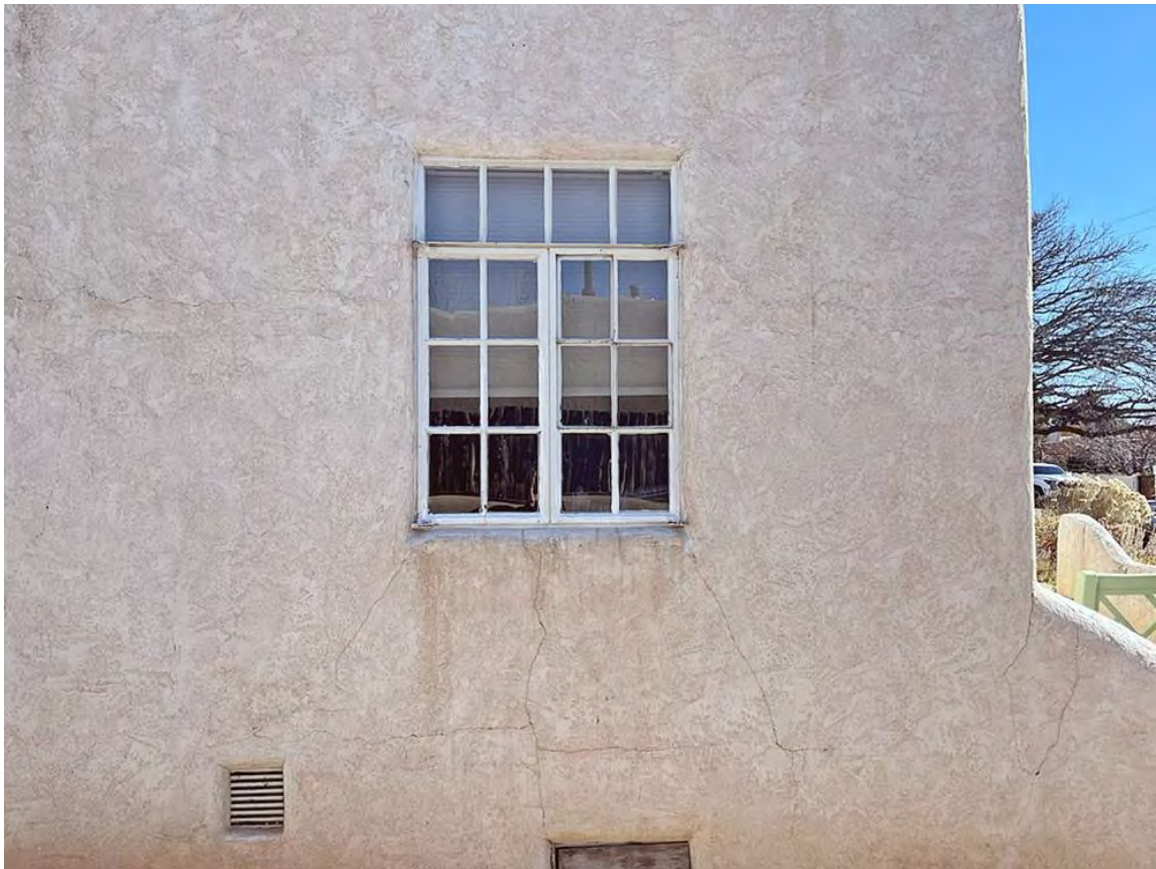
Photo 11: West elevation, south end. Camera facing east.
