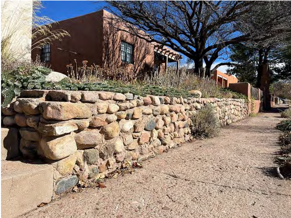
Photo 13: Stone retaining wall. Camera facing northeast.
