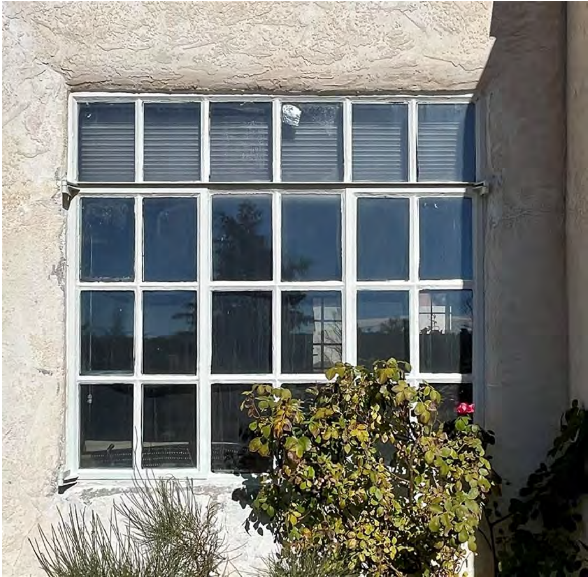
Photo 4: South (front) façade. Living room window. Camera facing north.
