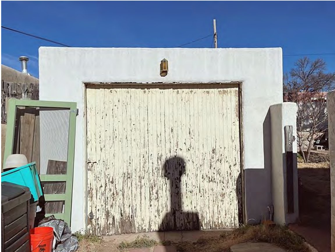
Photo 12: Garage. South elevation. Camera facing north.
