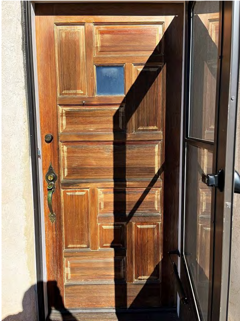
Photo 5: South (front) façade. Camera facing north.
