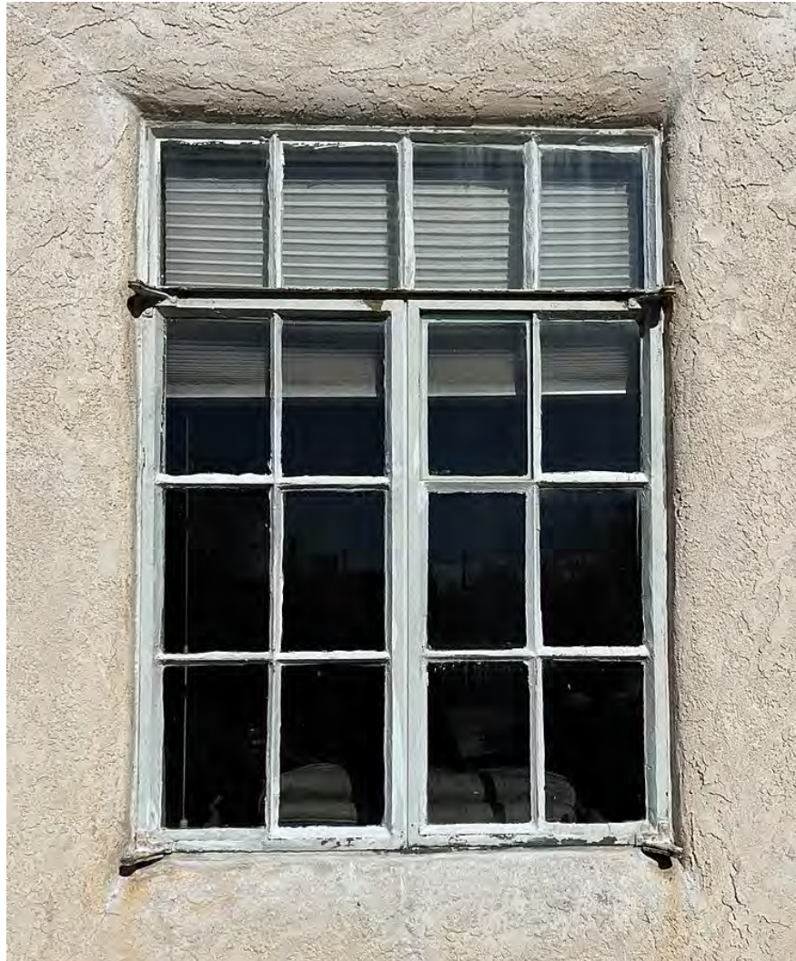
Photo 6: South (front) façade. Front bedroom window. Camera facing north.
