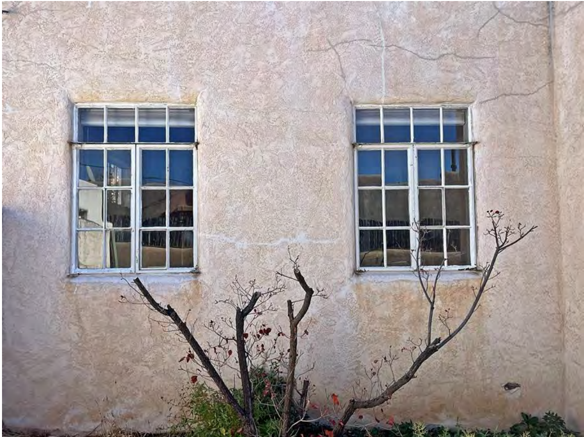
Photo 10: West elevation, north end. Camera facing east.
