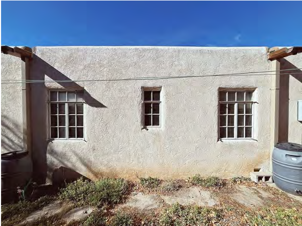
Photo 7: East elevation. Camera facing west.
