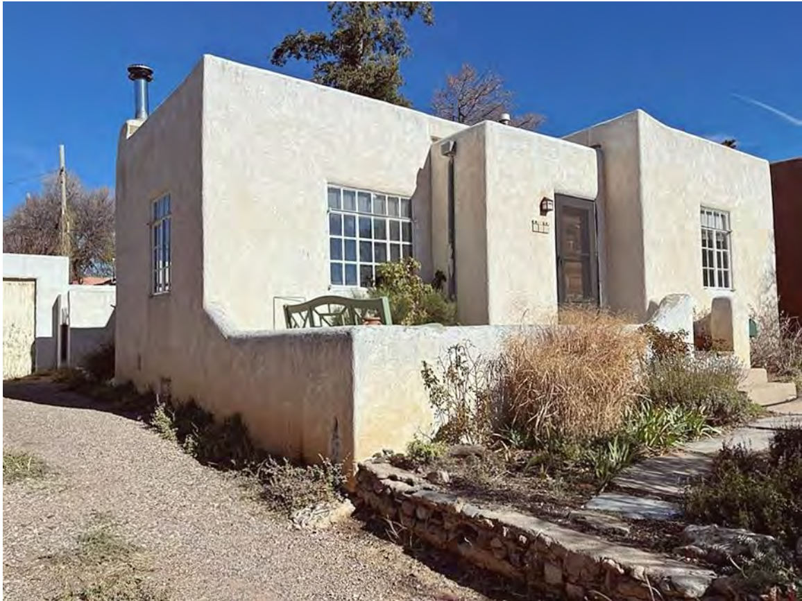
Photo 3: South (front) façade composition. Camera facing northeast.
