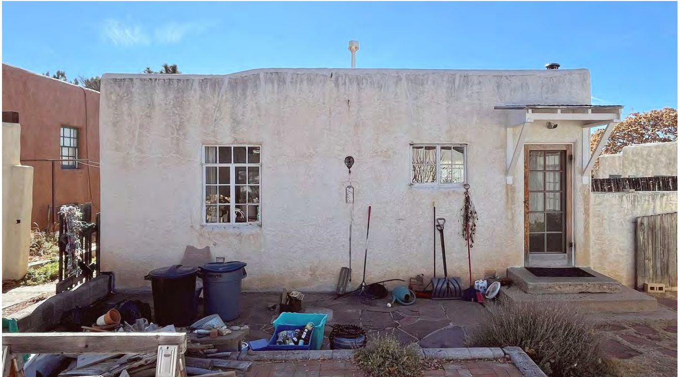
Photo 8: North elevation. Camera facing south.
