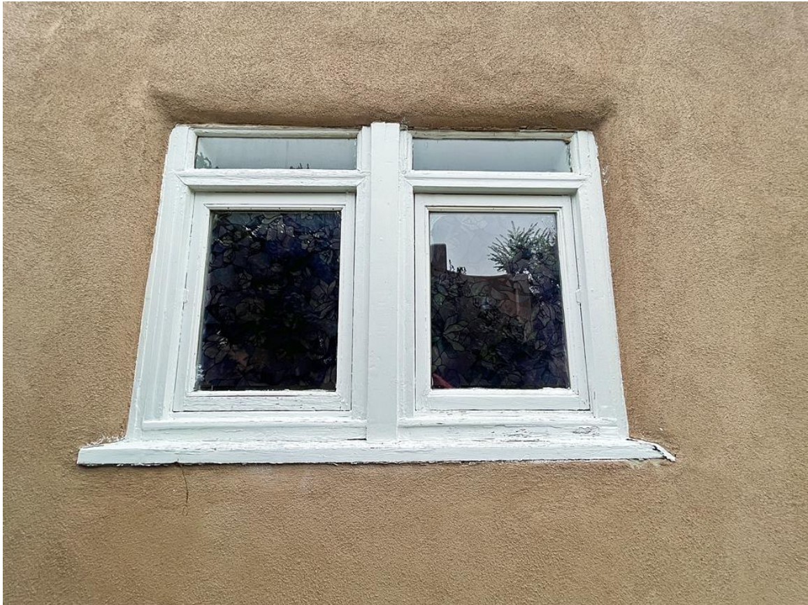
Photo 9: East elevation. North section, window detail. Camera facing west.
