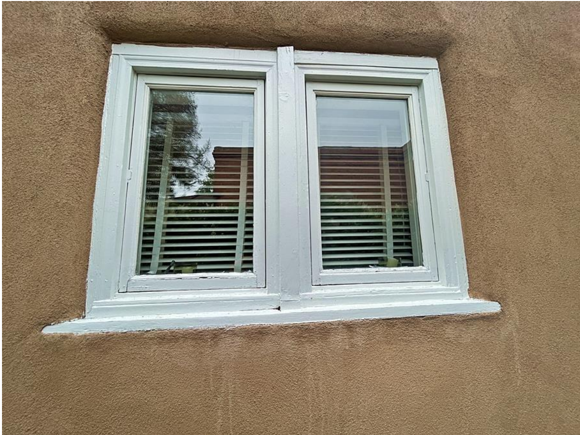
Photo 19: West elevation. North section. Window detail. Camera facing east.
