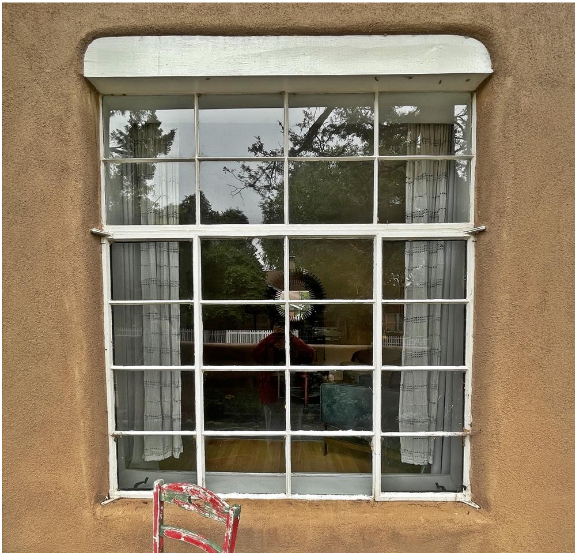
Photo 7: North (front) façade. West window. Camera facing south.
