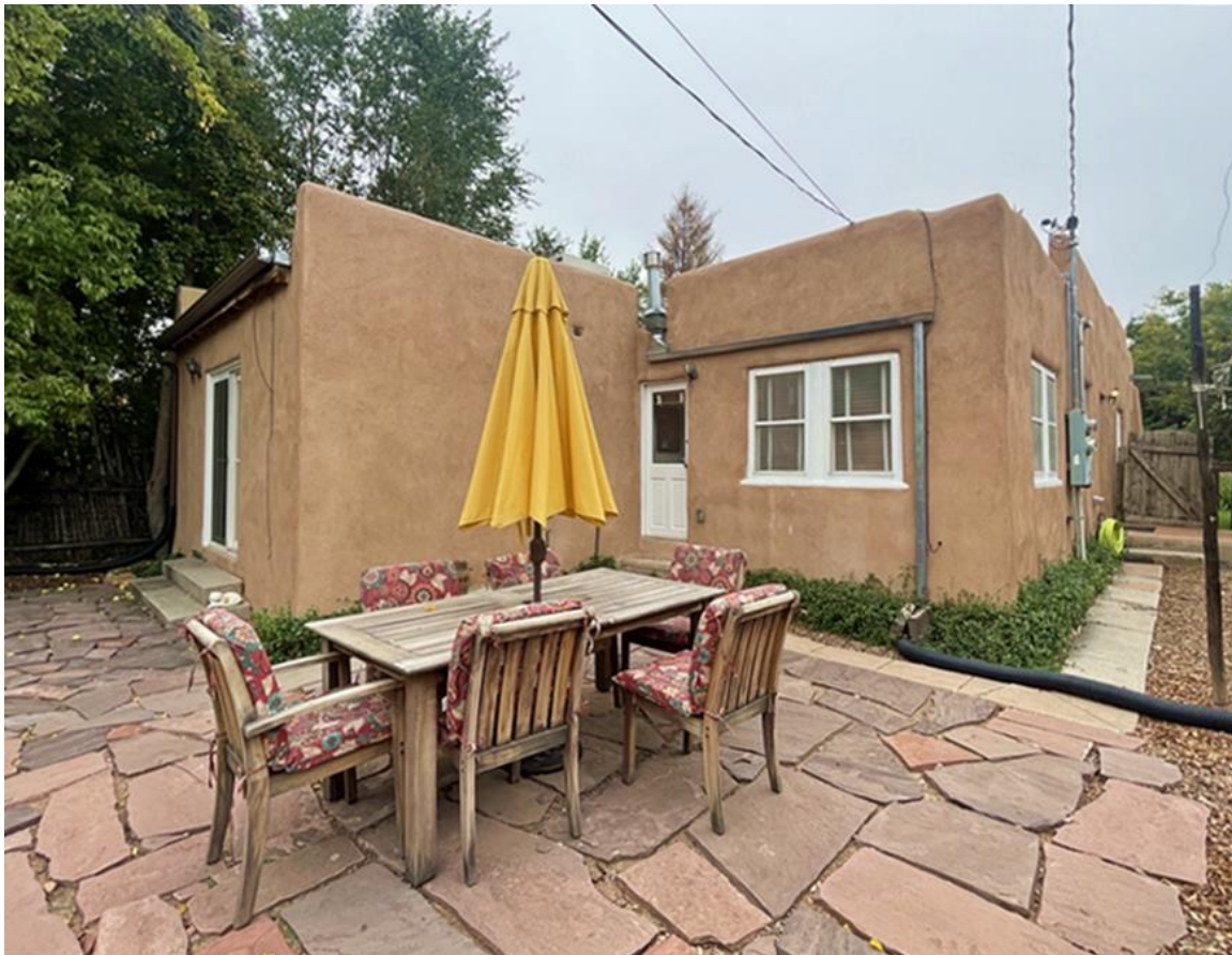
Photo 12: South elevation. Camera facing northwest.
