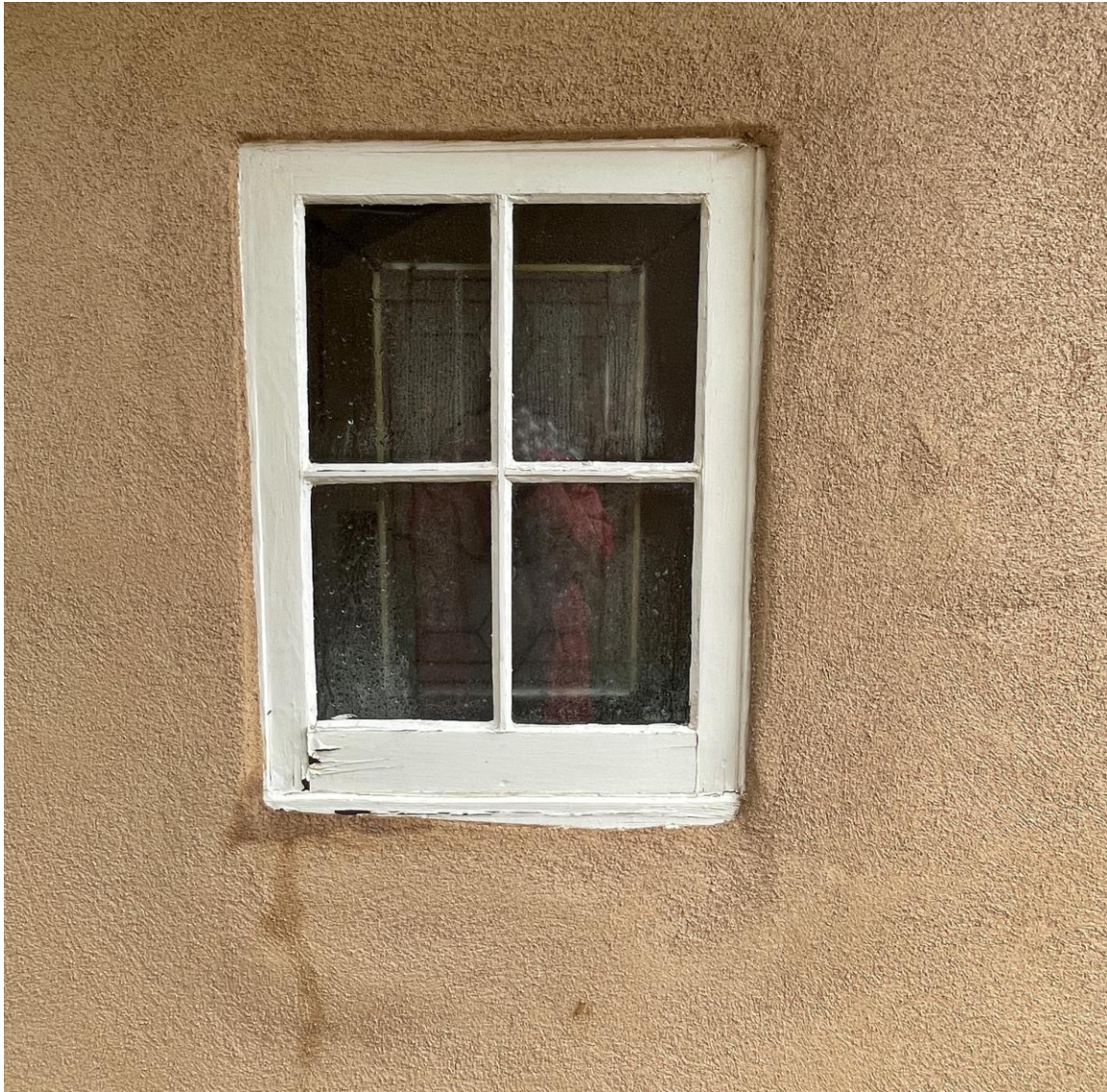
Photo 23: East elevation. Window detail. Camera facing west.
