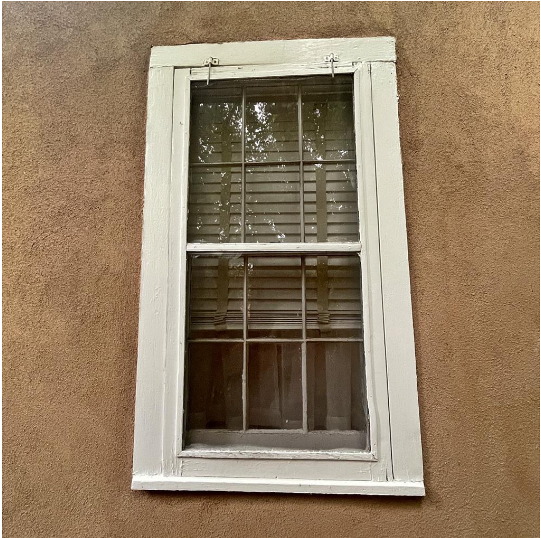
Photo 15: West elevation. South section. Window detail. Camera facing east.
