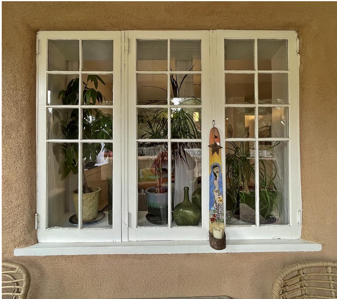
Photo 5: North (front) façade. Porch, casement window. Camera facing south.
