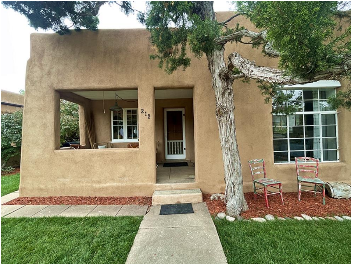
Photo 3: North (front) façade. Camera facing south.
