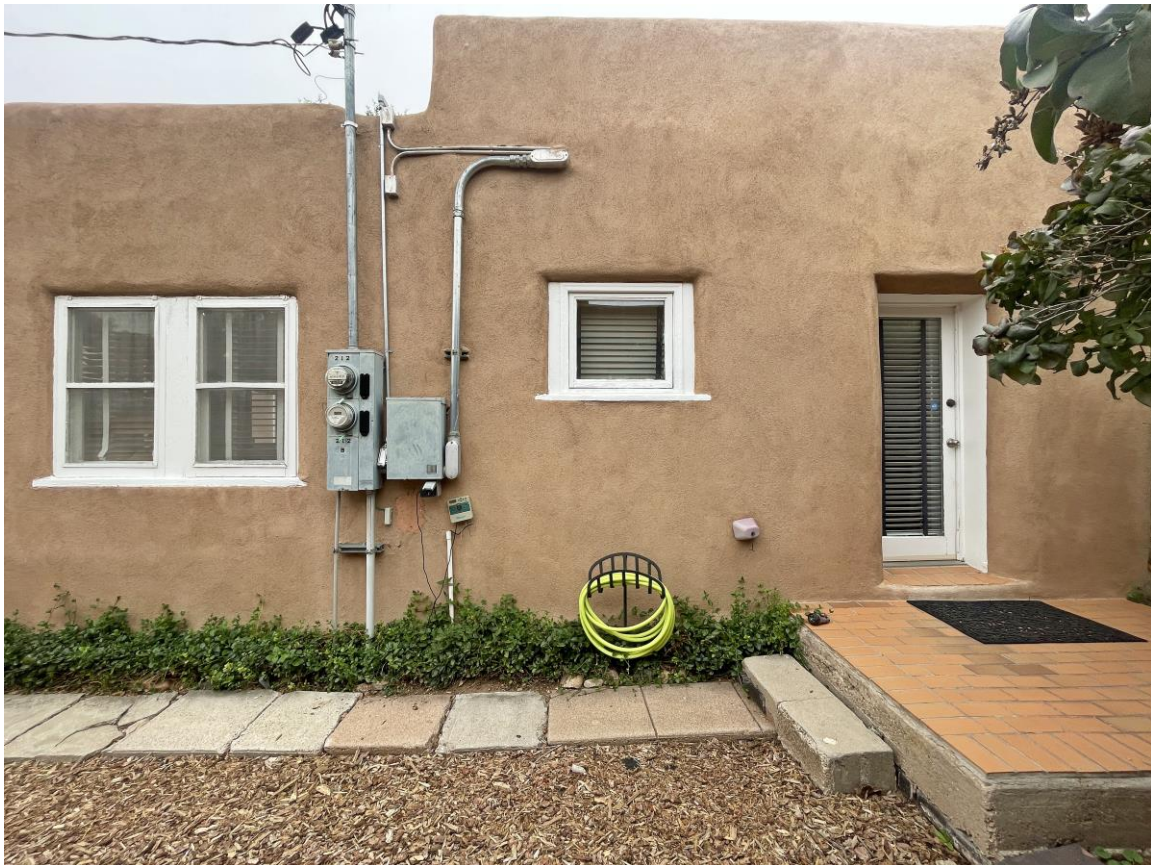
Photo 10: East elevation. Middle and south sections. Camera facing west.
