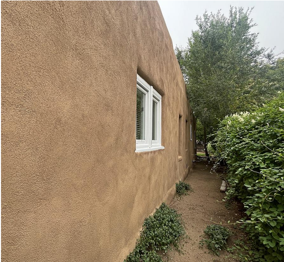
Photo 18: West elevation. North section. Camera facing southeast.
