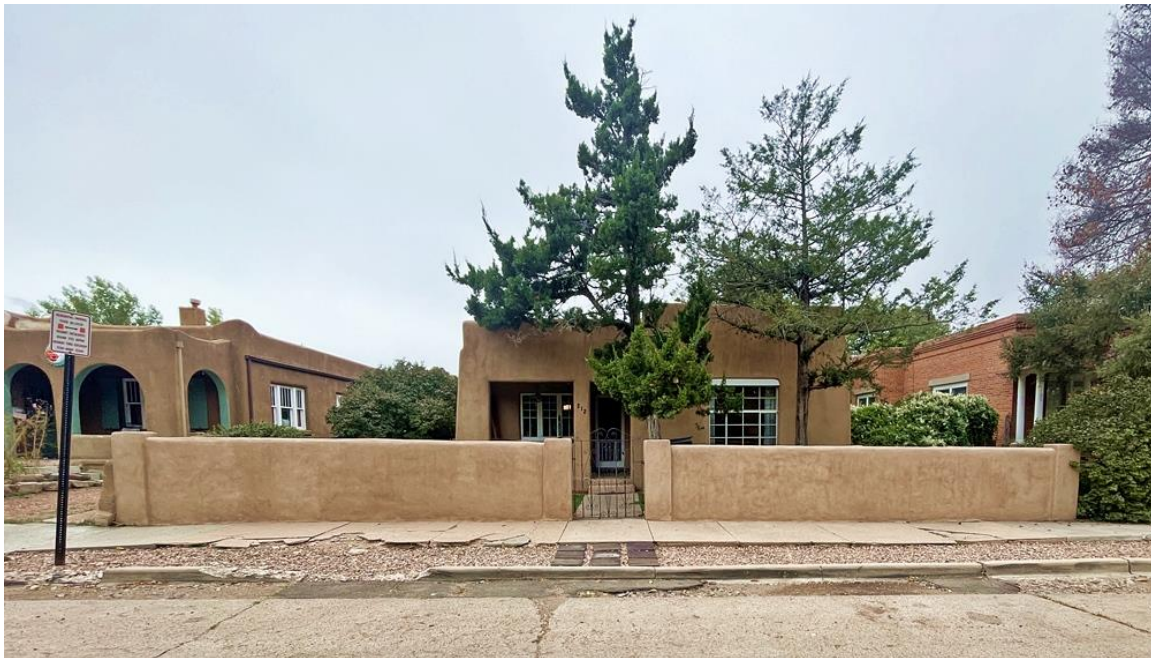
Photo 2: Setting and front yard wall. Camera facing south.
