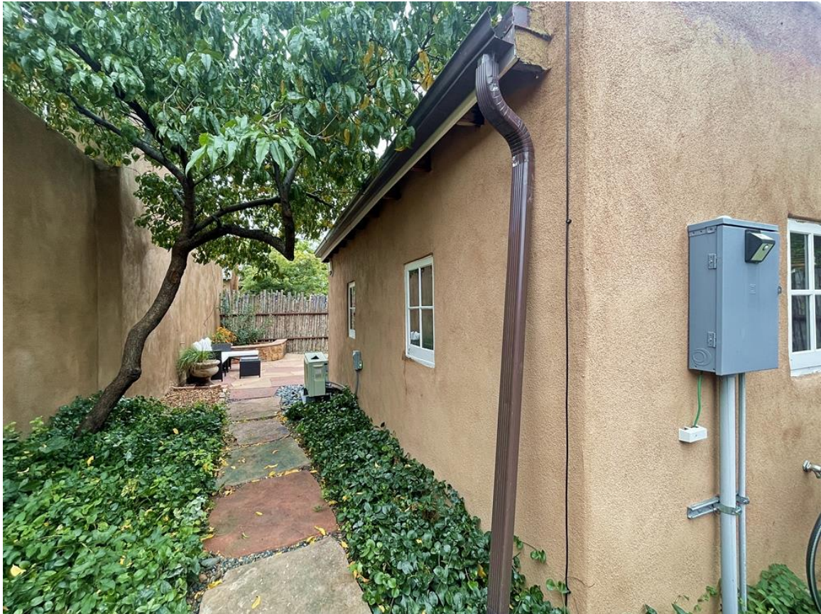
Photo 22: East end of north elevation and east elevation. Camera facing southwest.
