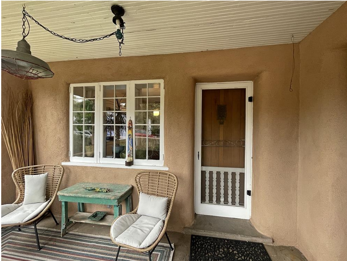
Photo 4: North (front) façade. Porch. Camera facing southeast.
