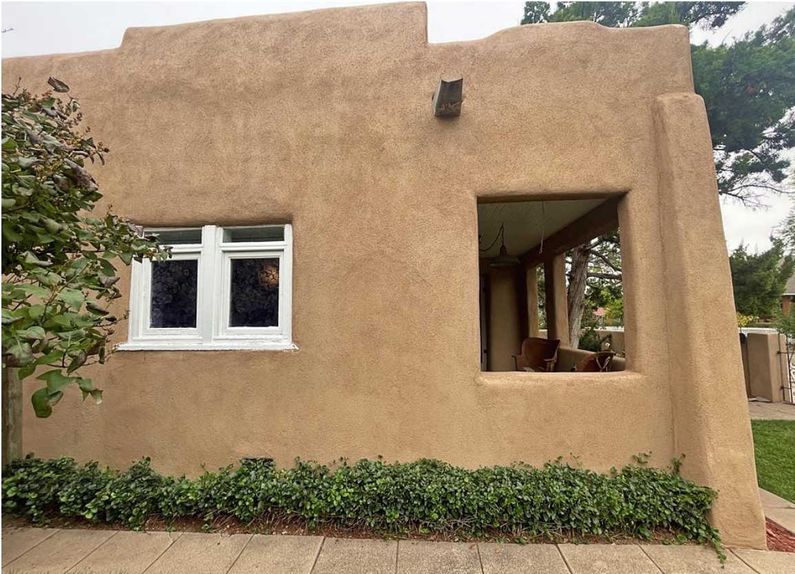
Photo 8: East elevation. North section. Camera facing west.
