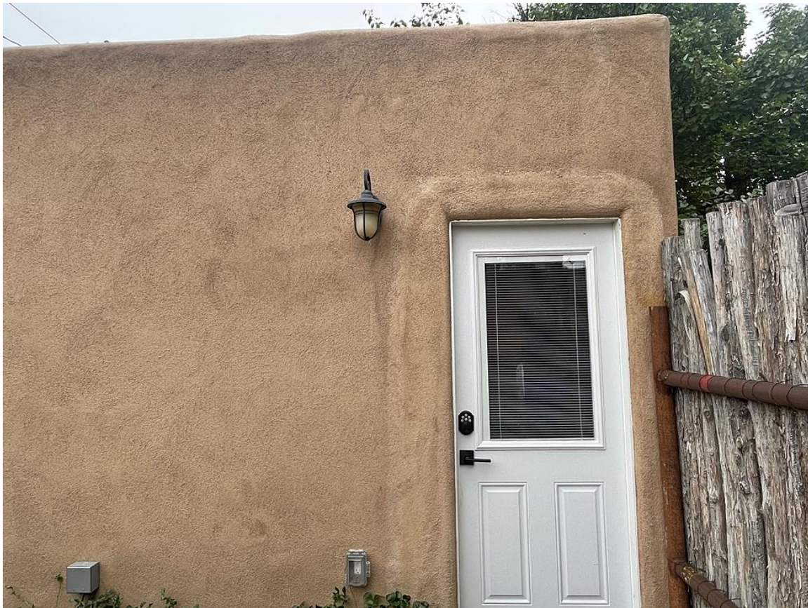
Photo 21: North elevation. West end. Camera facing south.
