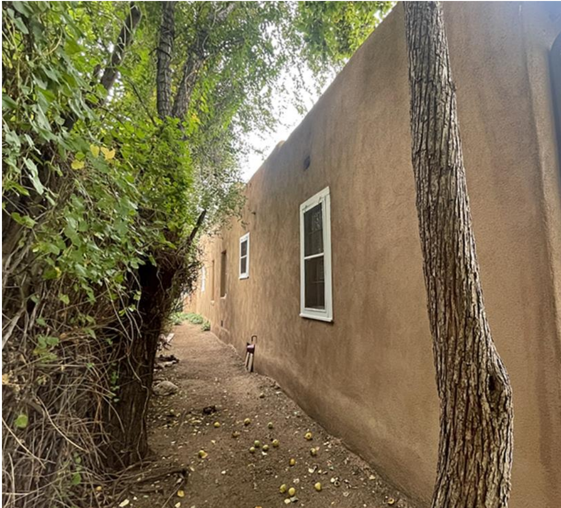
Photo 14. West elevation. South section. Camera facing northeast.
