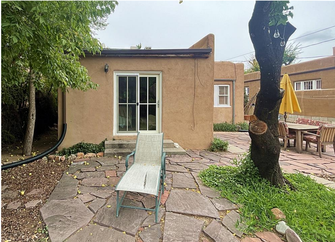
Photo 13: South elevation. Camera facing north.
