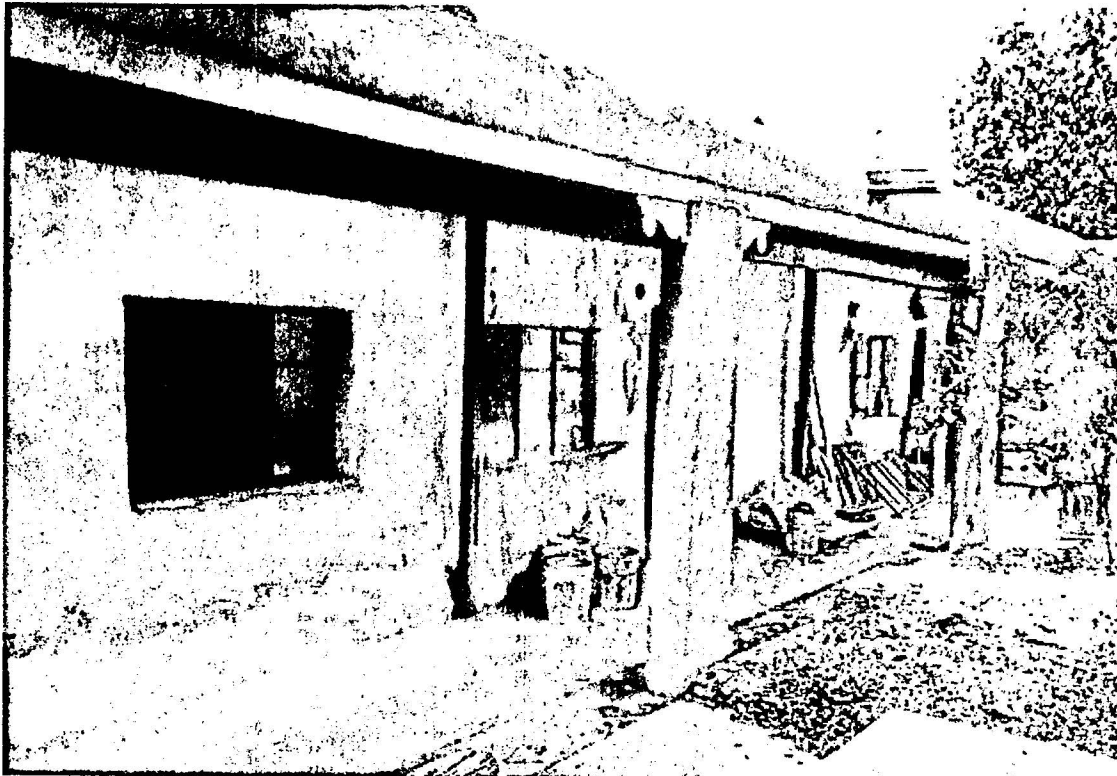
Portal at East Elevation
