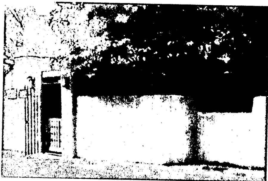
Entrance at West Elevation
