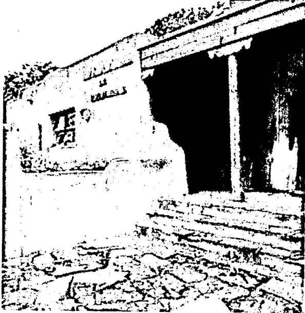
Detail of north entrance
