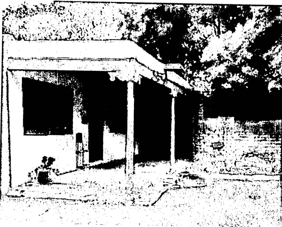
Portal and east elevation
