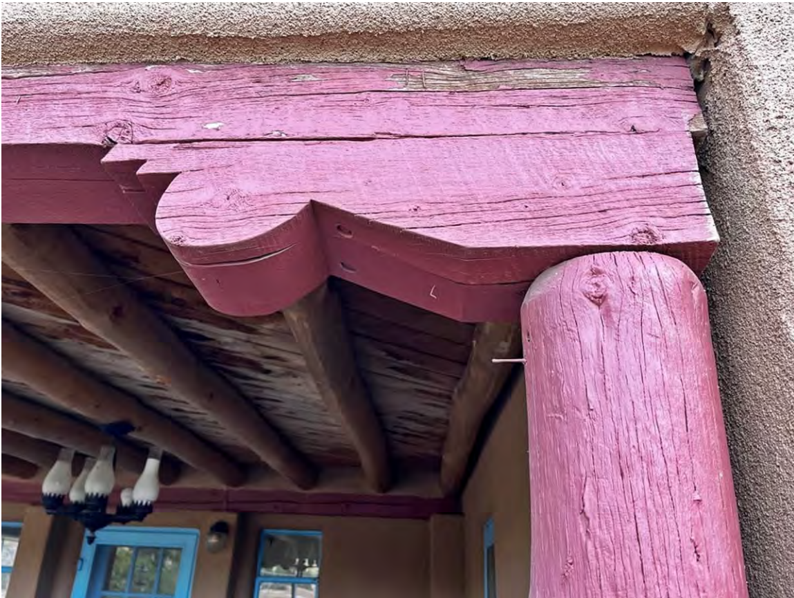
Photo 6: Porch corbel. Camera facing up. October 4, 2023, JWM.
