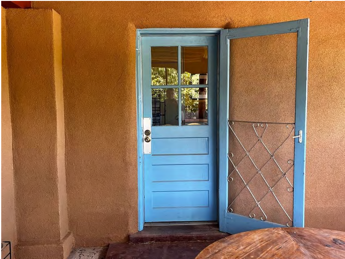
Photo 8. South elevation. Entry door to kitchen. Camera facing northwest. October 4, 2023, JWM.
