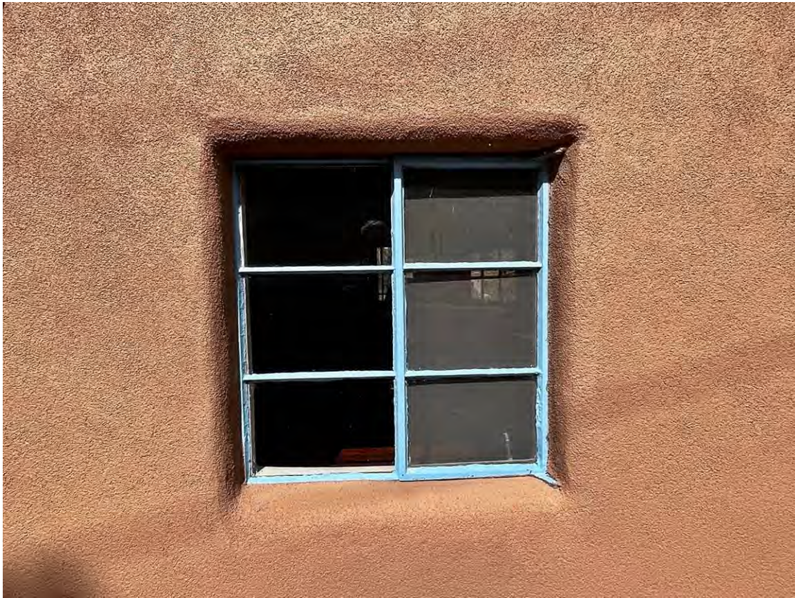
Photo 13: South elevation. Casement window at living room. Camera facing north. October 4, 2023, JWM.
