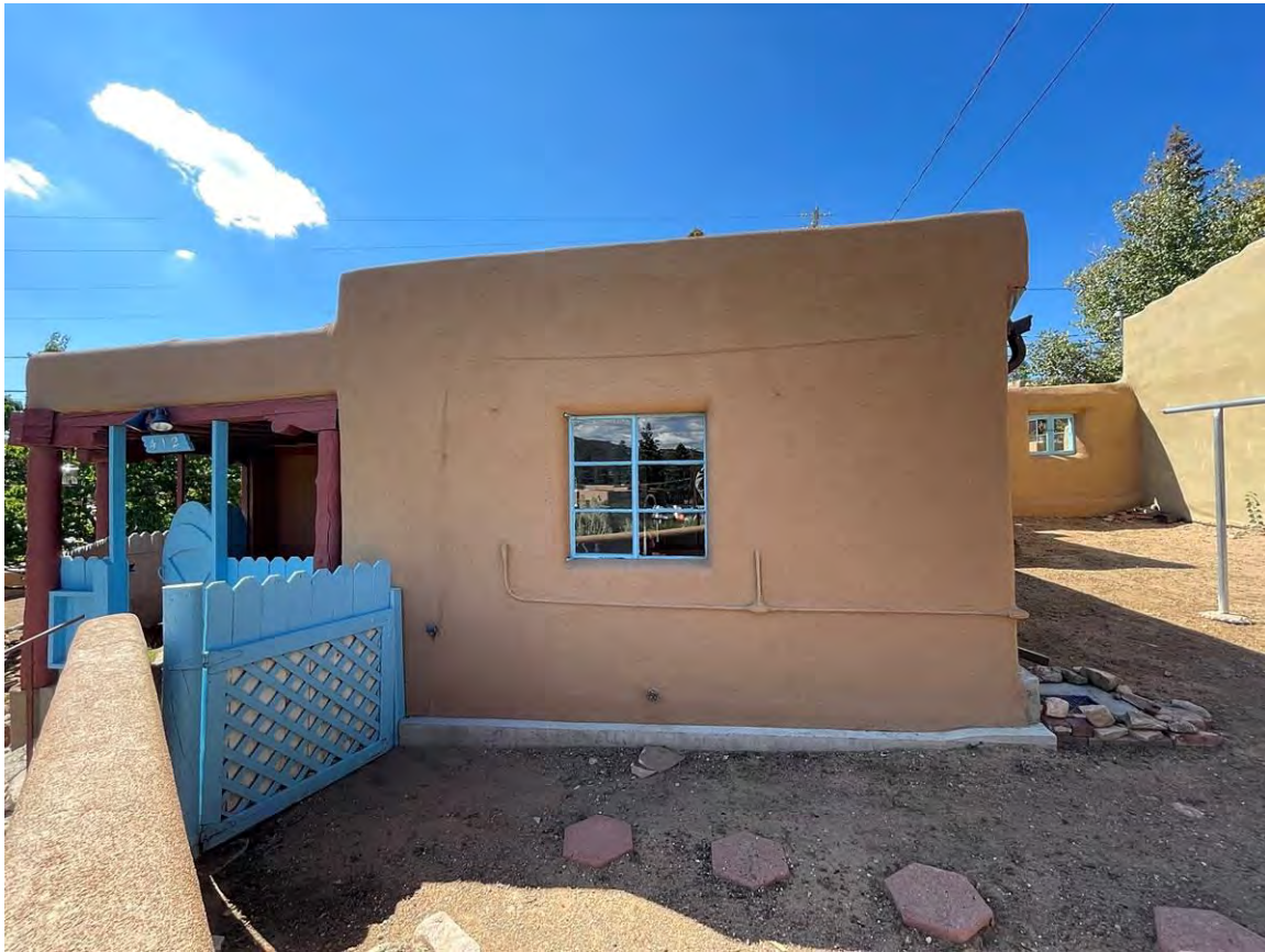
Photo 9: North elevation. Camera facing southwest. September 21, 2023, GC.
