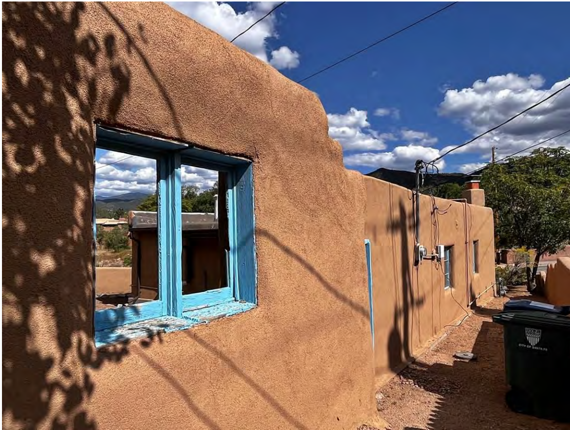
Photo 16: Orphan wall and south elevation of house. Camera facing northeast. October 4, 2023, JWM.
