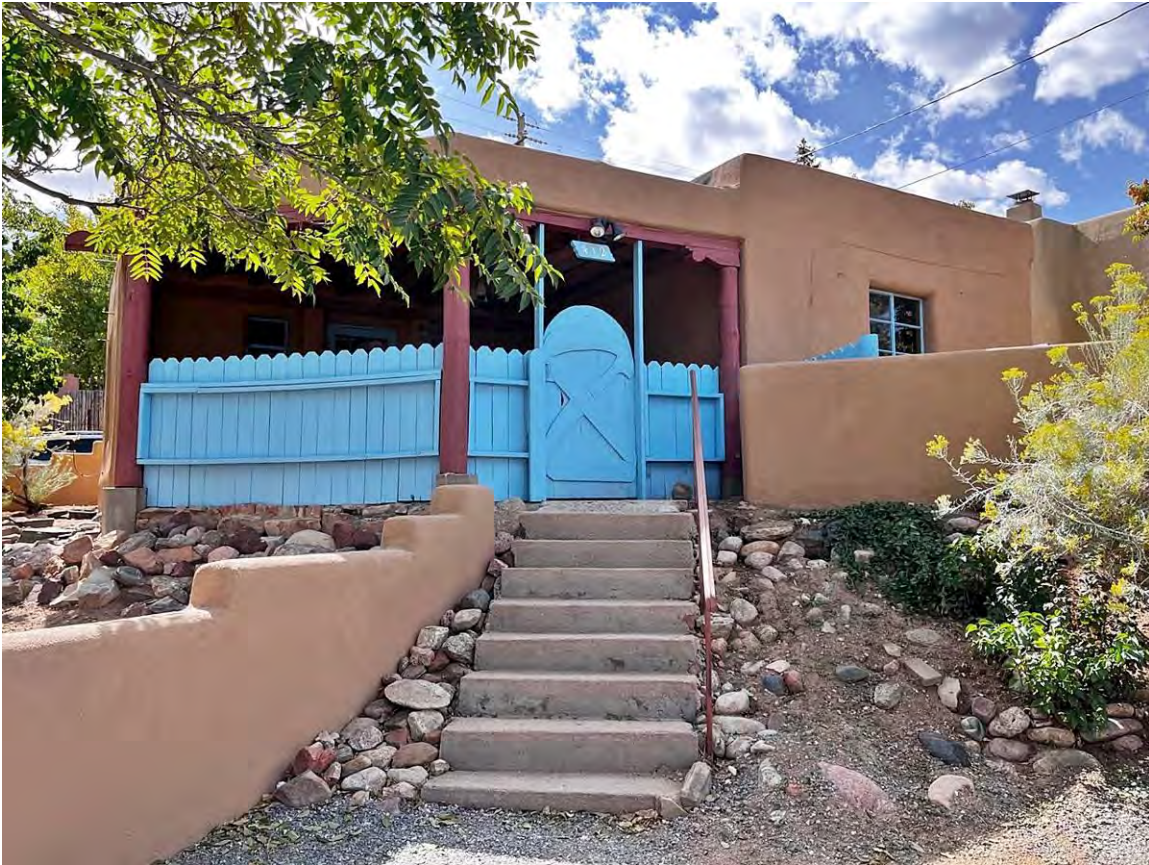
Photo 2: East and north elevations. Camera facing southwest. October 4, 2023, JWM.
