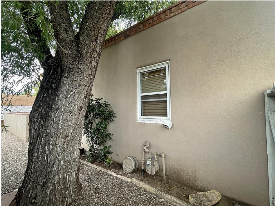
Photo 10: West elevation. Camera facing northeast.
