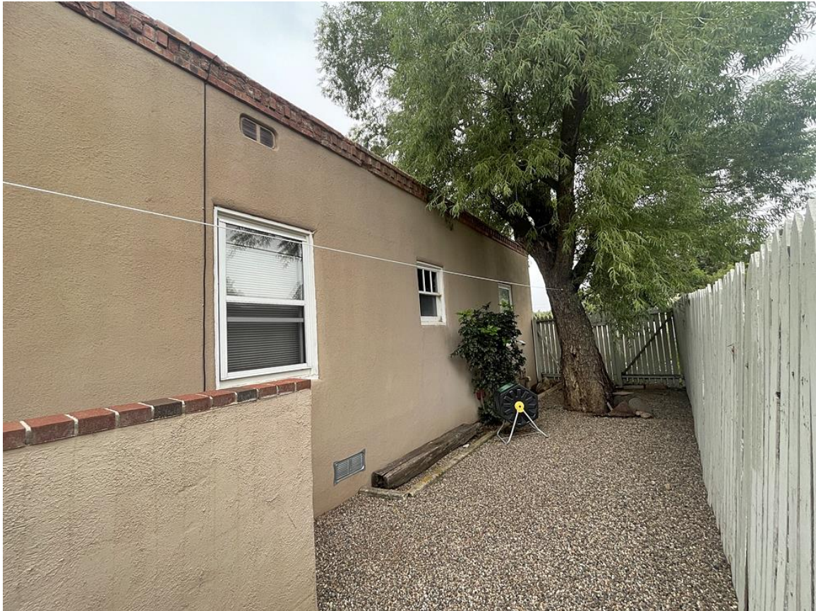
Photo 9: West elevation. Camera facing southeast.
