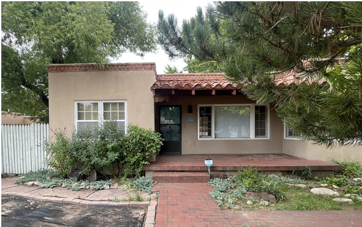
Photo 4: South (front) façade, west and center sections. Camera facing northeast.
