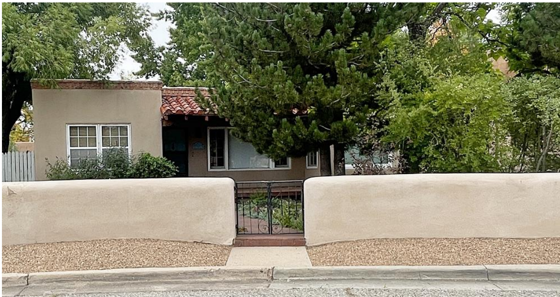
Photo 2: House and setting. Camera facing northeast.
