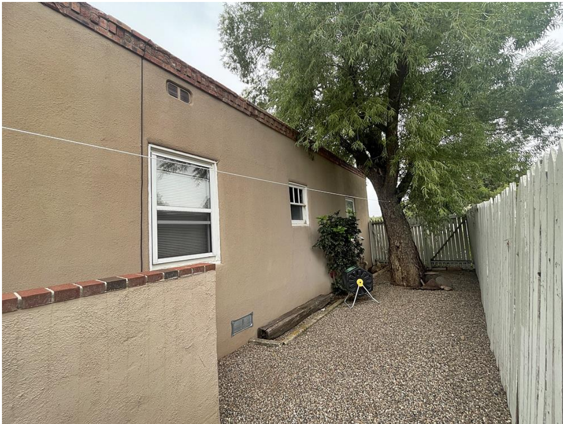
Photo 9: West elevation. Camera facing southeast.
