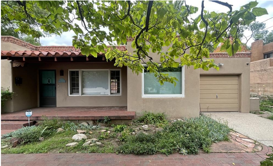
Photo 5: South (front) façade, center and east sections. Camera facing northeast.
