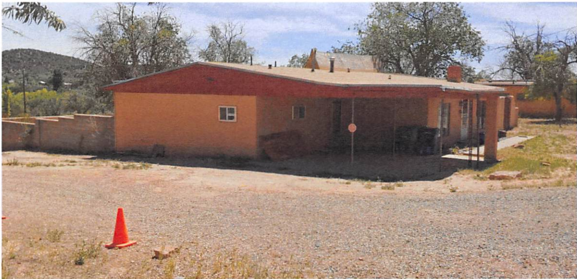
Photo 2: North and east elevations. Camera facing southeast.
