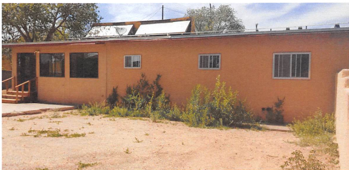
Photo 5: South elevation. Camera facing northwest.
