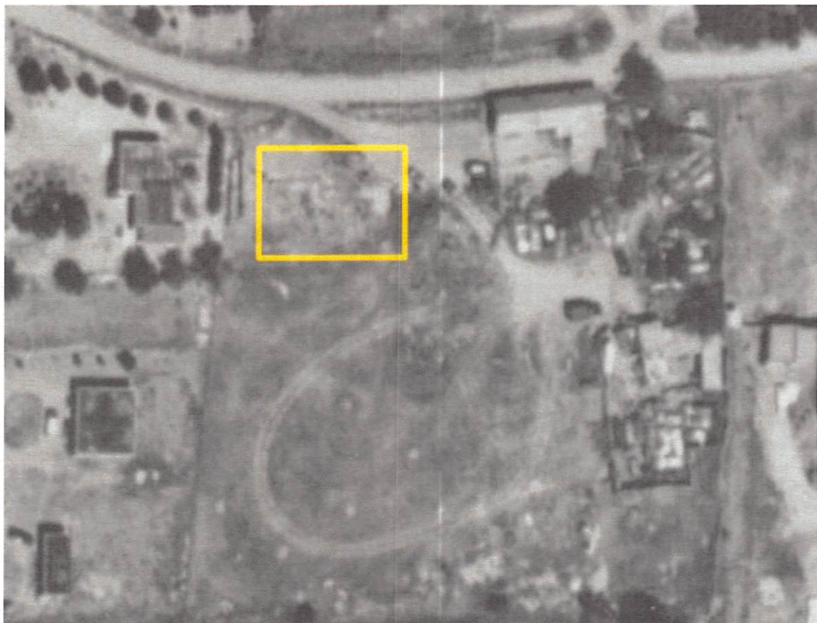
Figure 6: August 18, 1960, aerial photograph. Previous structure removed. Rectangle indicates ground activity; potentially foundation construction. Courtesy City of Santa Fe, GIS.
