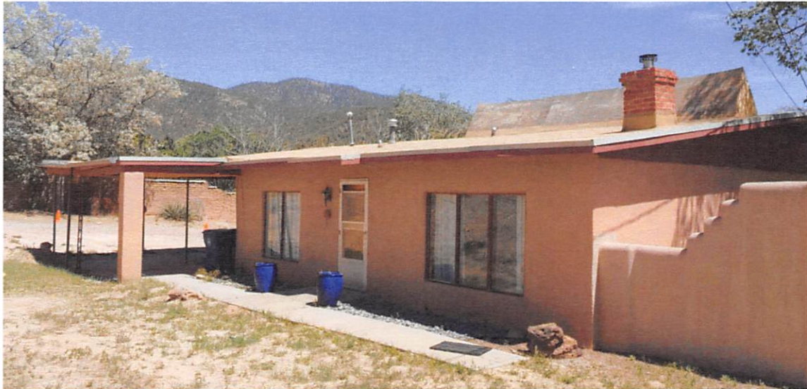
Photo 3: North elevation. Camera facing southeast.
