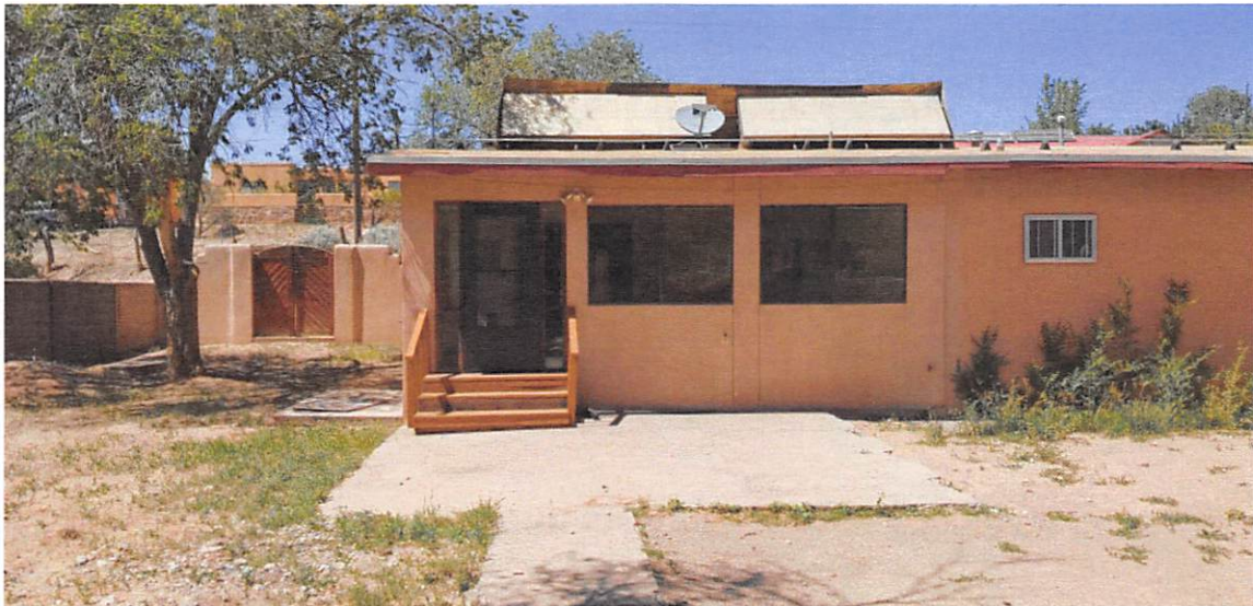
Photo 6: West end of south elevation; enclosed porch. Camera facing north.
