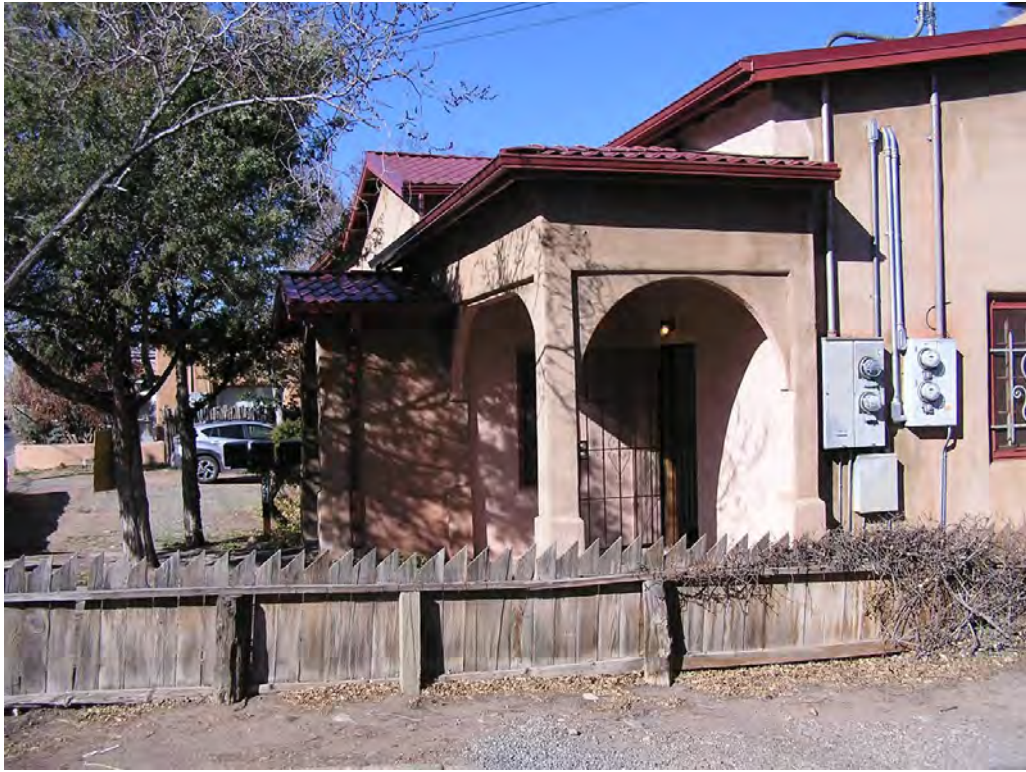
5 - East Façade (southeast corner)
