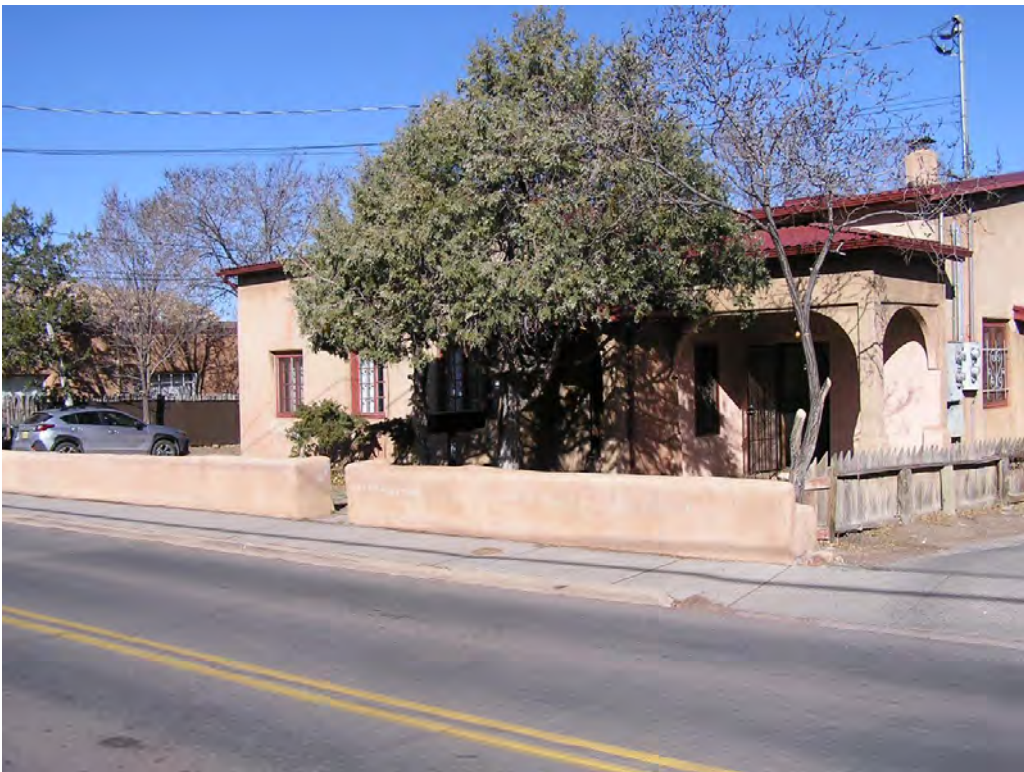
4 - South Façade (facing Agua Fria)
